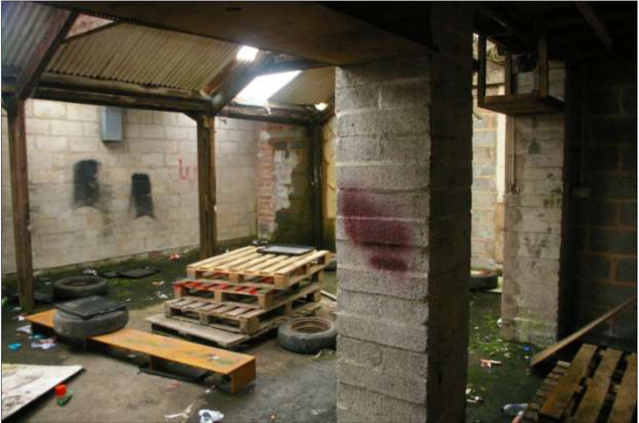
The interior of Building 4; viewed from the north-east.
