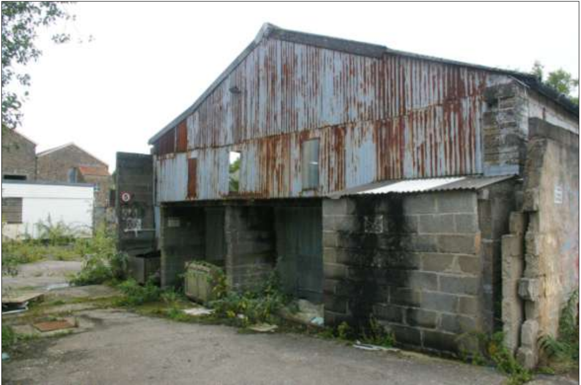
FIGURE 19: THE WEST GABLE OF B1; VIEWED FROM THE SOUTH-WEST.
