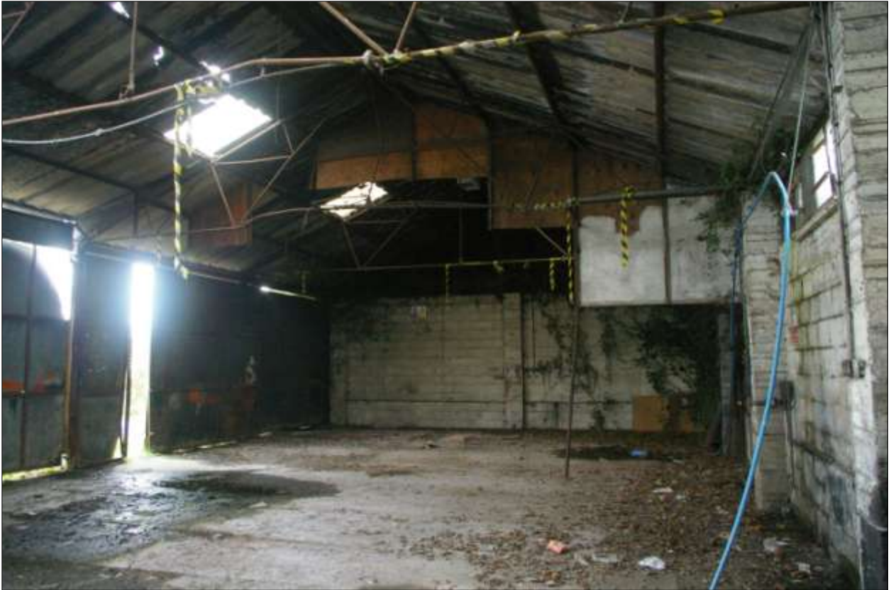
The interior of Building 1, viewed from the west.
