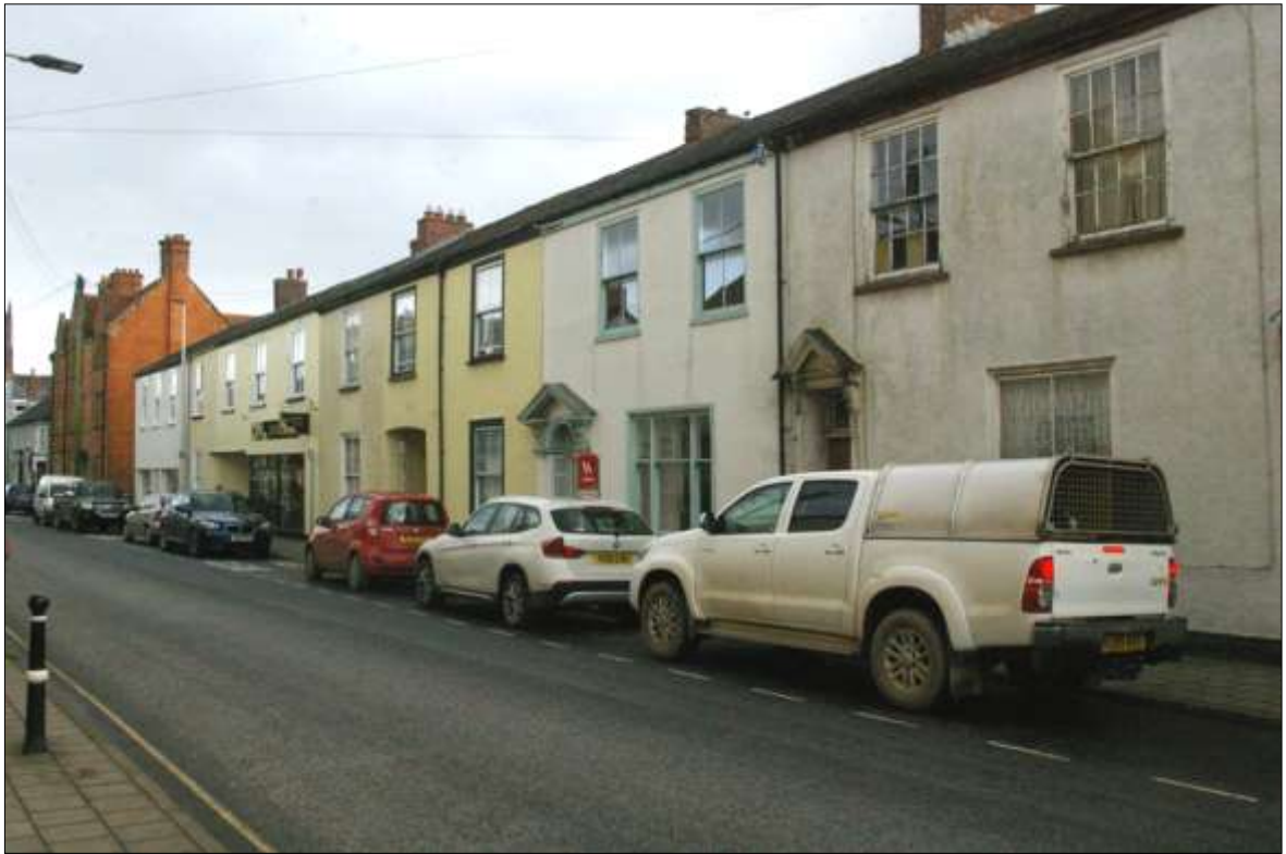
FIGURE 31: NOS. 24-26 SOUTH STREET; VIEWED FROM THE SOUTH-WEST.
