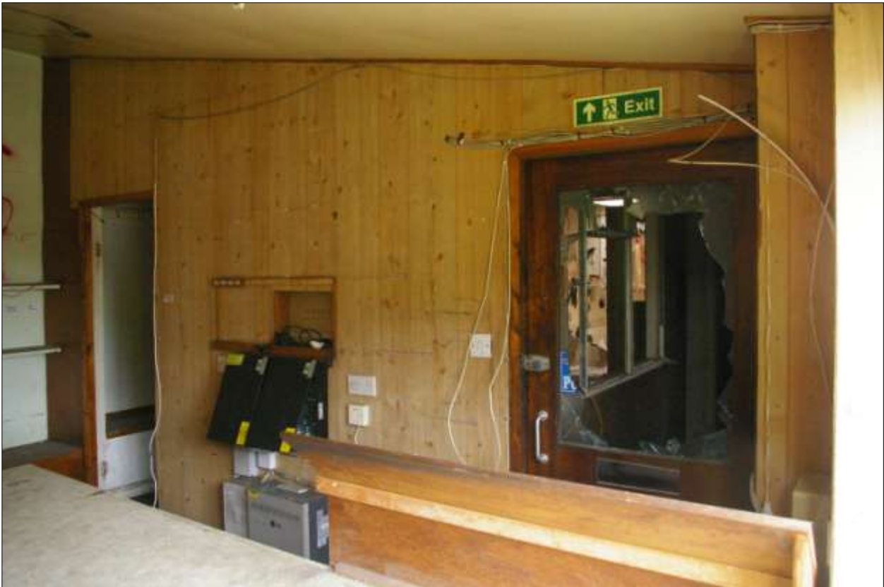
The interior of Building 2; viewed from the south-east.
