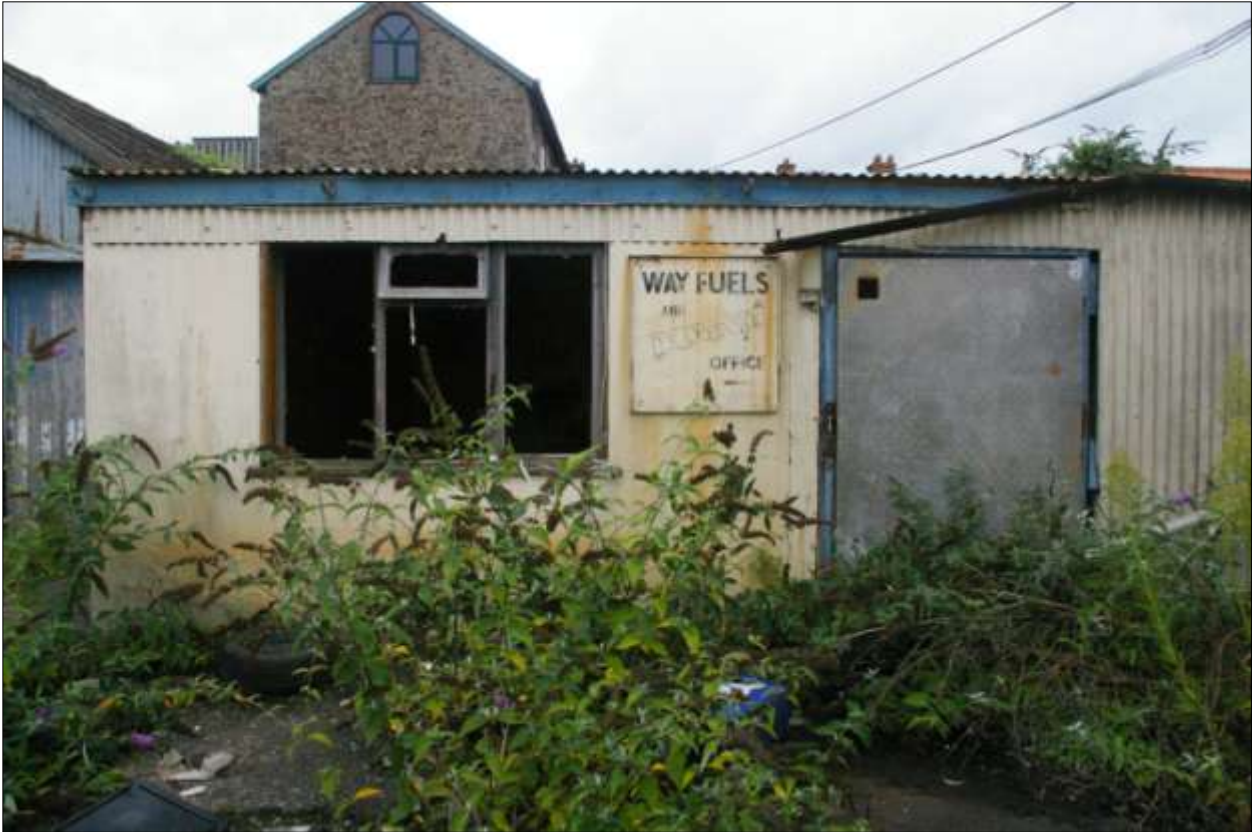
The exterior of Building 2; viewed from the east.
