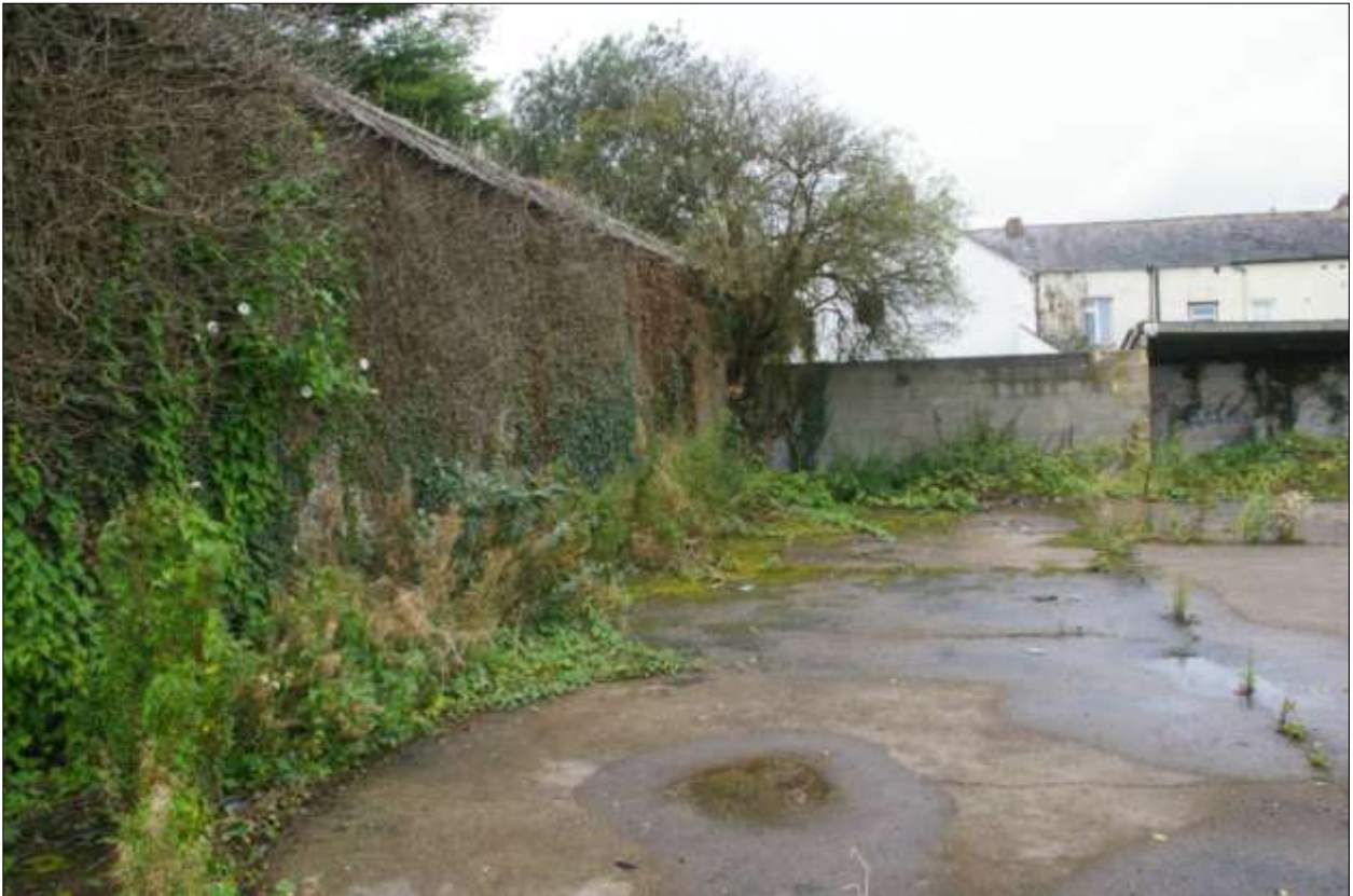
The south wall of the central yard where it extends across the former burgage plots behind South Street; viewed from the ENE.
