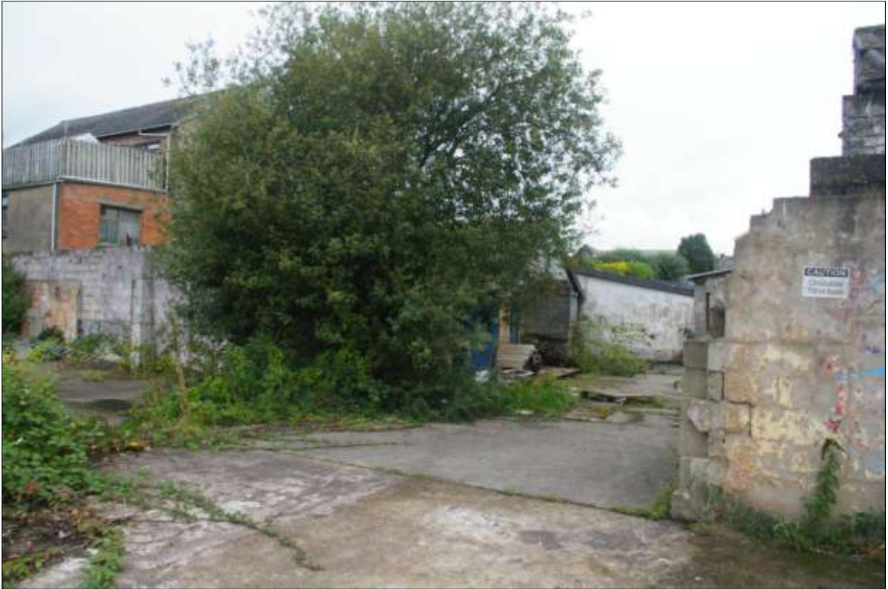
The access between the central and northern yards; viewed from the south-east.
