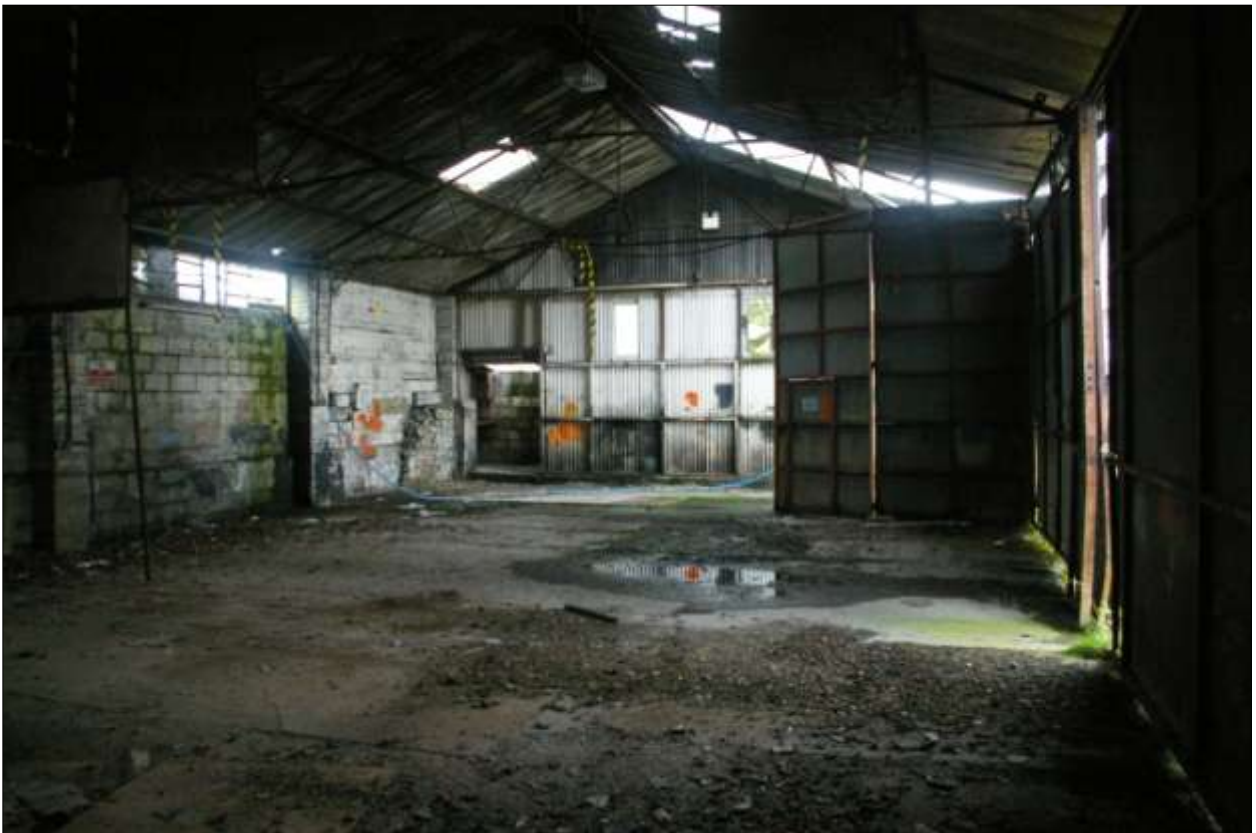
As above, viewed from the east.
