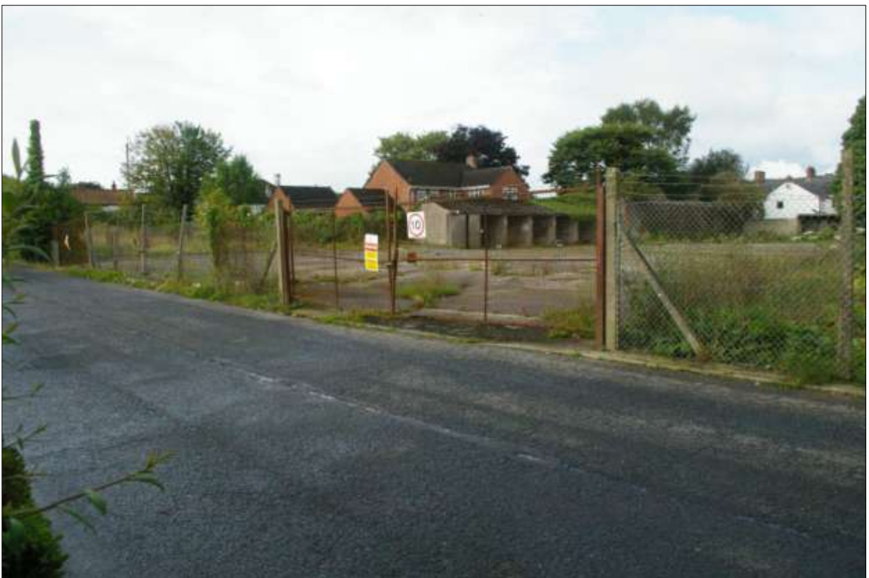
The northern gated entrance that serves the central yard; viewed from the north-east.
