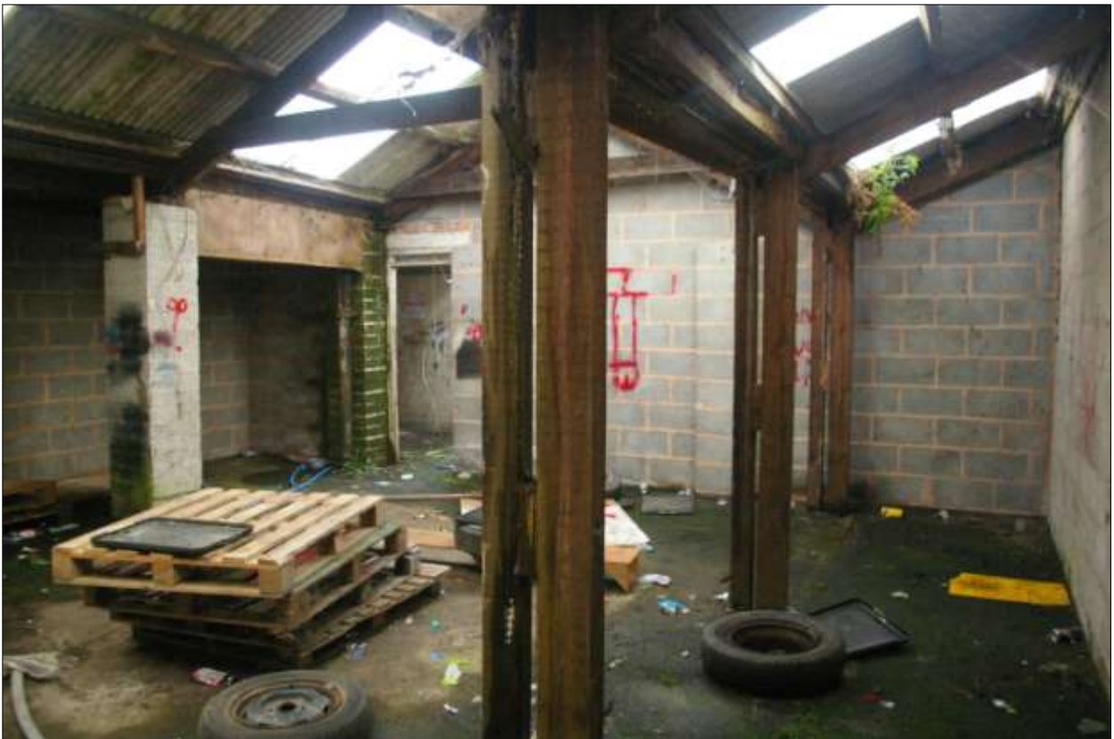
As above; viewed from the south-west.
