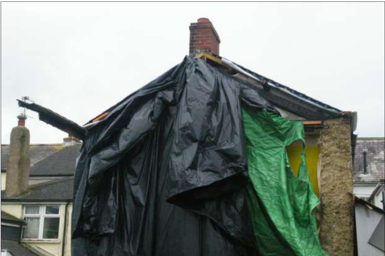
As above, showing the cob wall and burnt roof trusses.
