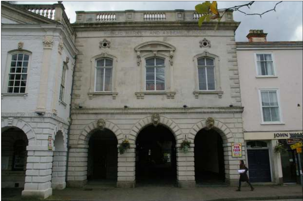
The north elevation of the Markey House on road Street; viewed from the north.
