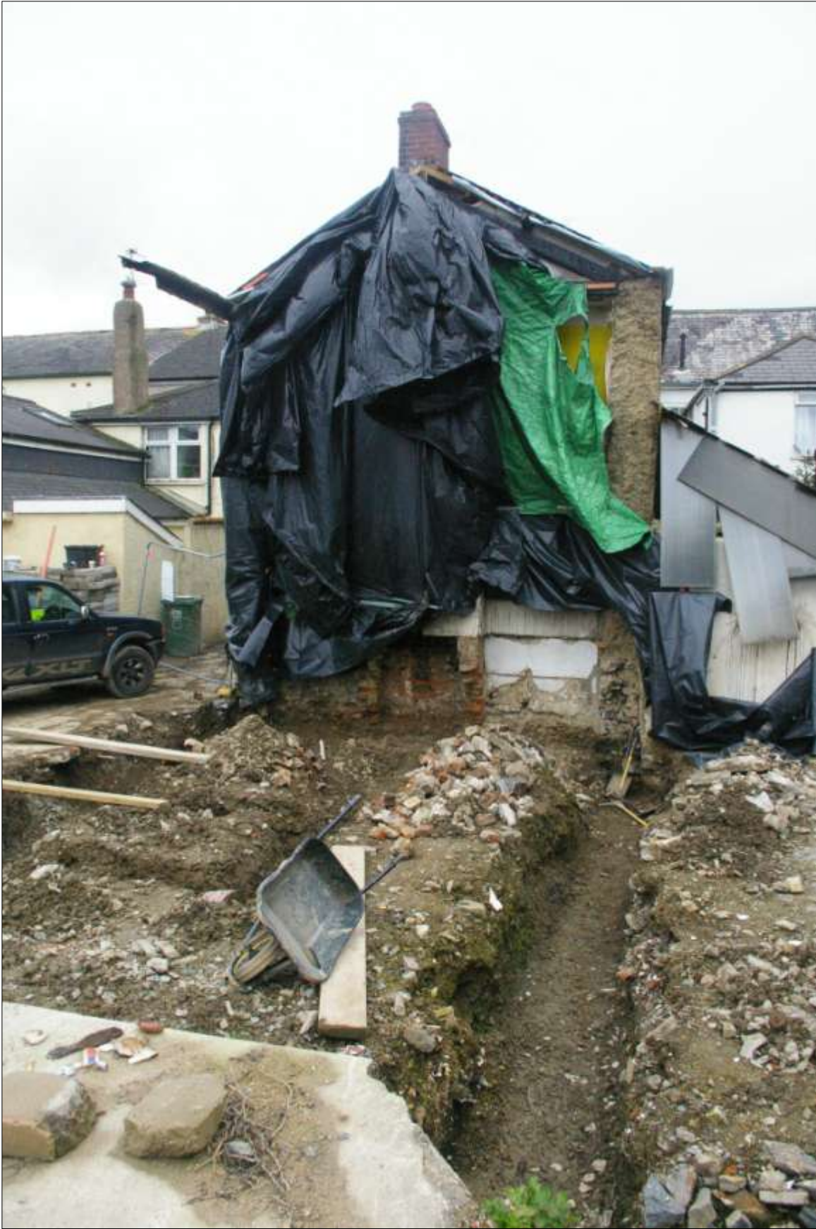
As above, showing the new foundation trenches.
