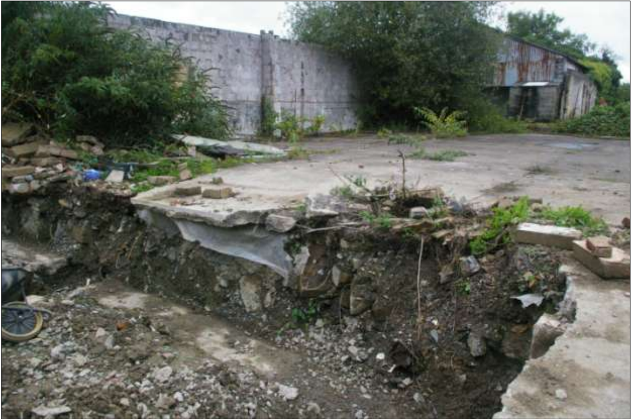
As above, but viewed from the west; showing the depth on made ground across the western part of the central yard.
