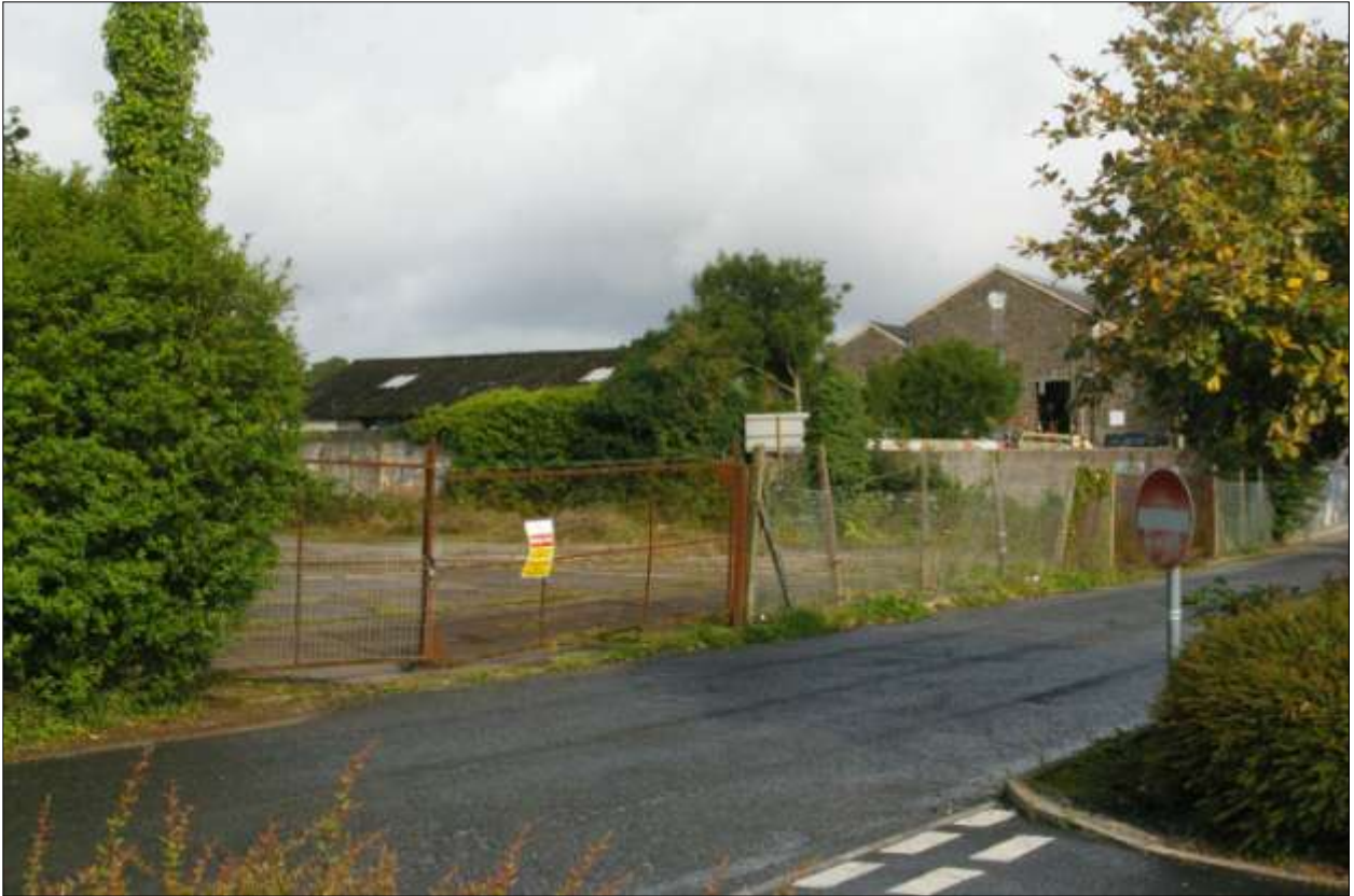
The southern gated entrance that serves the central yard; viewed from the ESE.
