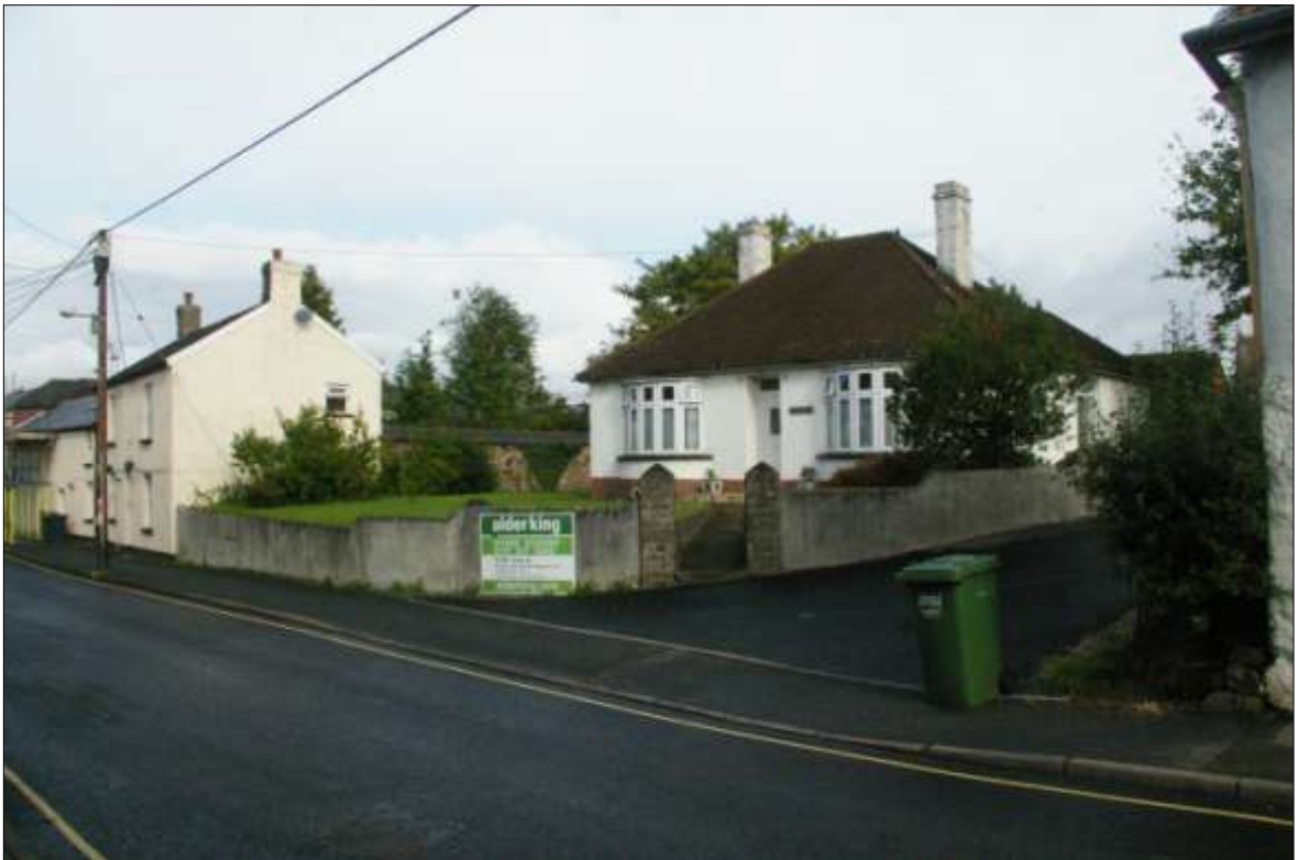
FIGURE 13: THE BUNGALOW (TOWER VIEW), VIEWED FROM THE SOUTH-EAST.
