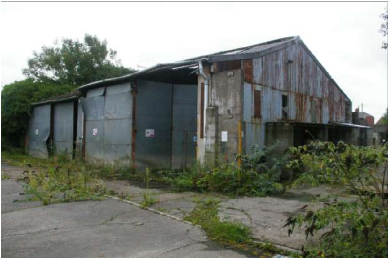
Building 1; viewed from the north-west.
