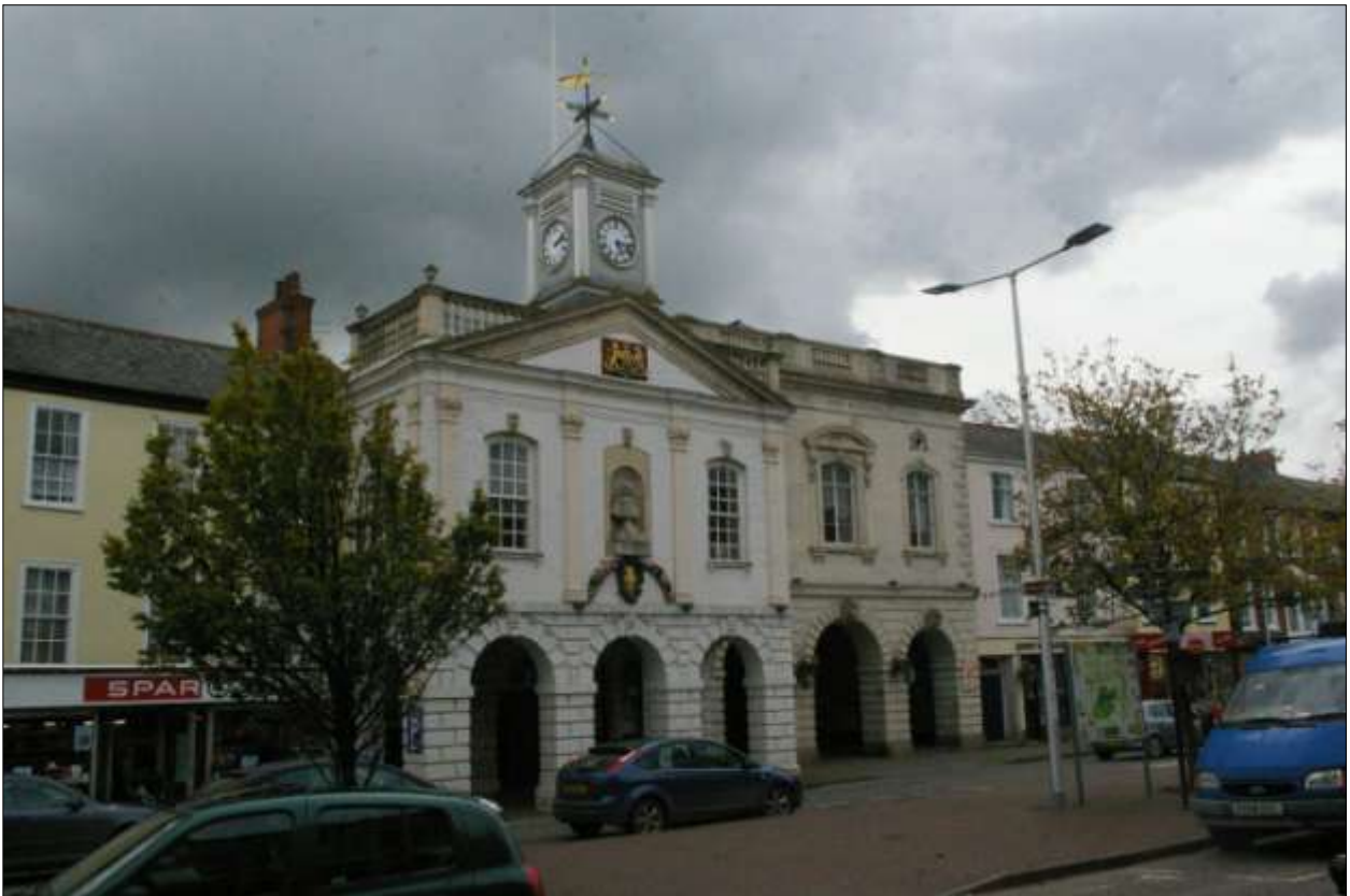
The GI Guildhall on Broad Street, with the GII* Market House to the right; viewed from the north-east.
