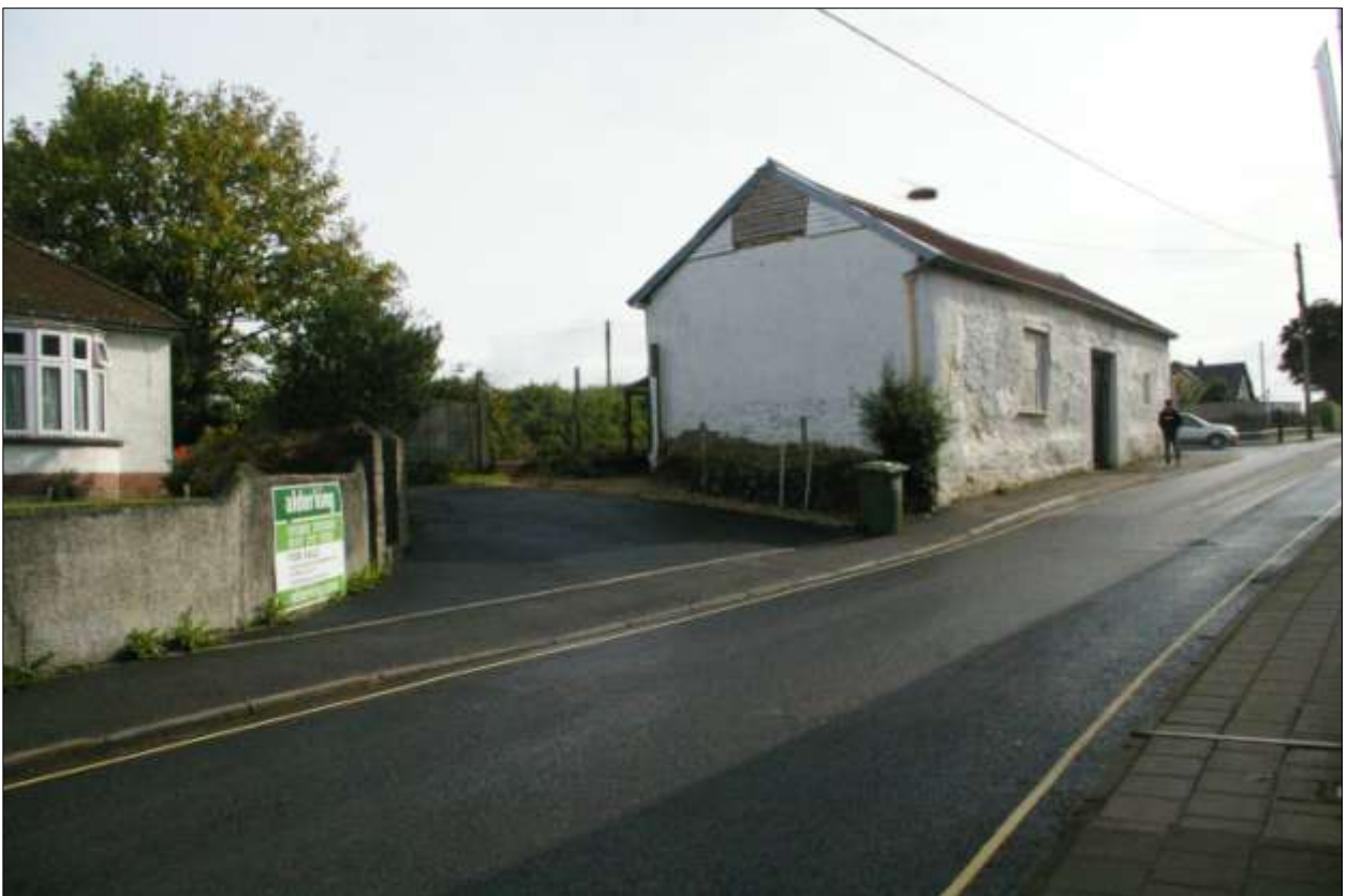
The historic barn next to Tower View on Mill Street; viewed from the south-west.
