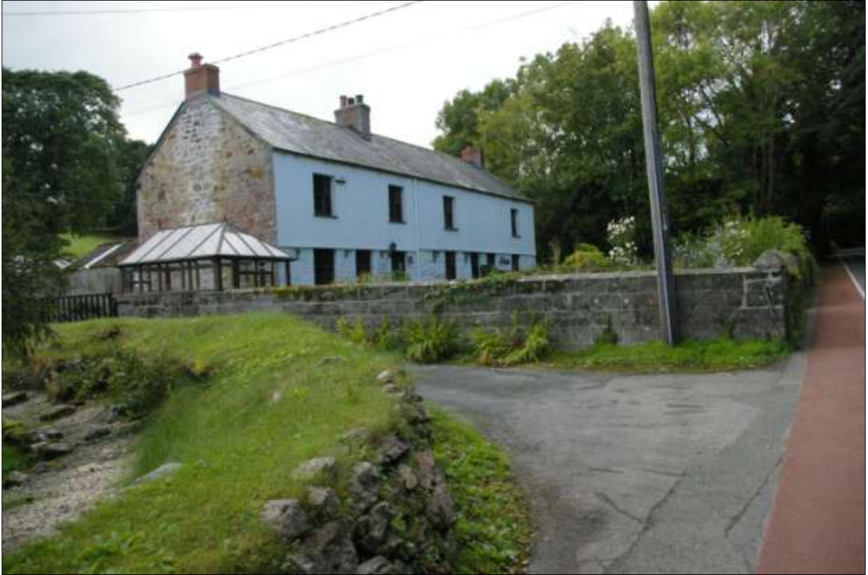
View of 37-38 Duporth Road; viewed from the north-east.
