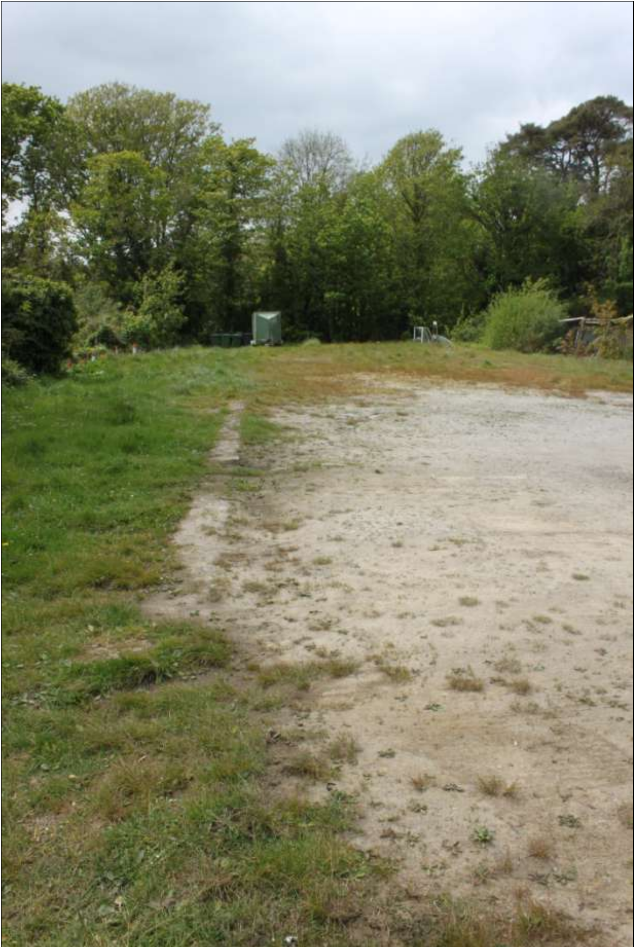
Traces of the former building evident in the south yard, viewed from the east.
