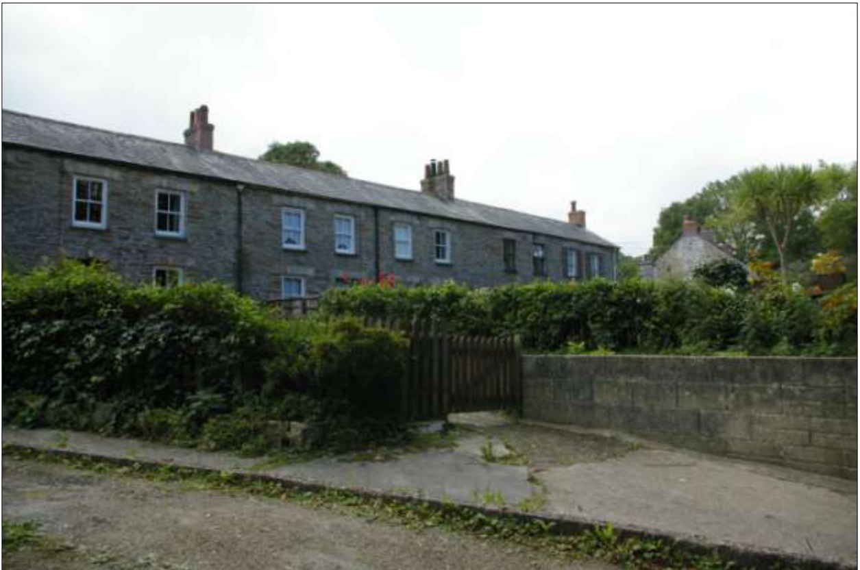
View of 31-36 Duporth Road; viewed from the north-east.
