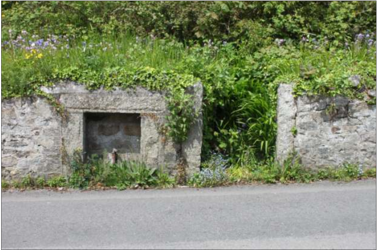
Shot of the water point and adjacent gate opening, viewed from the south.
