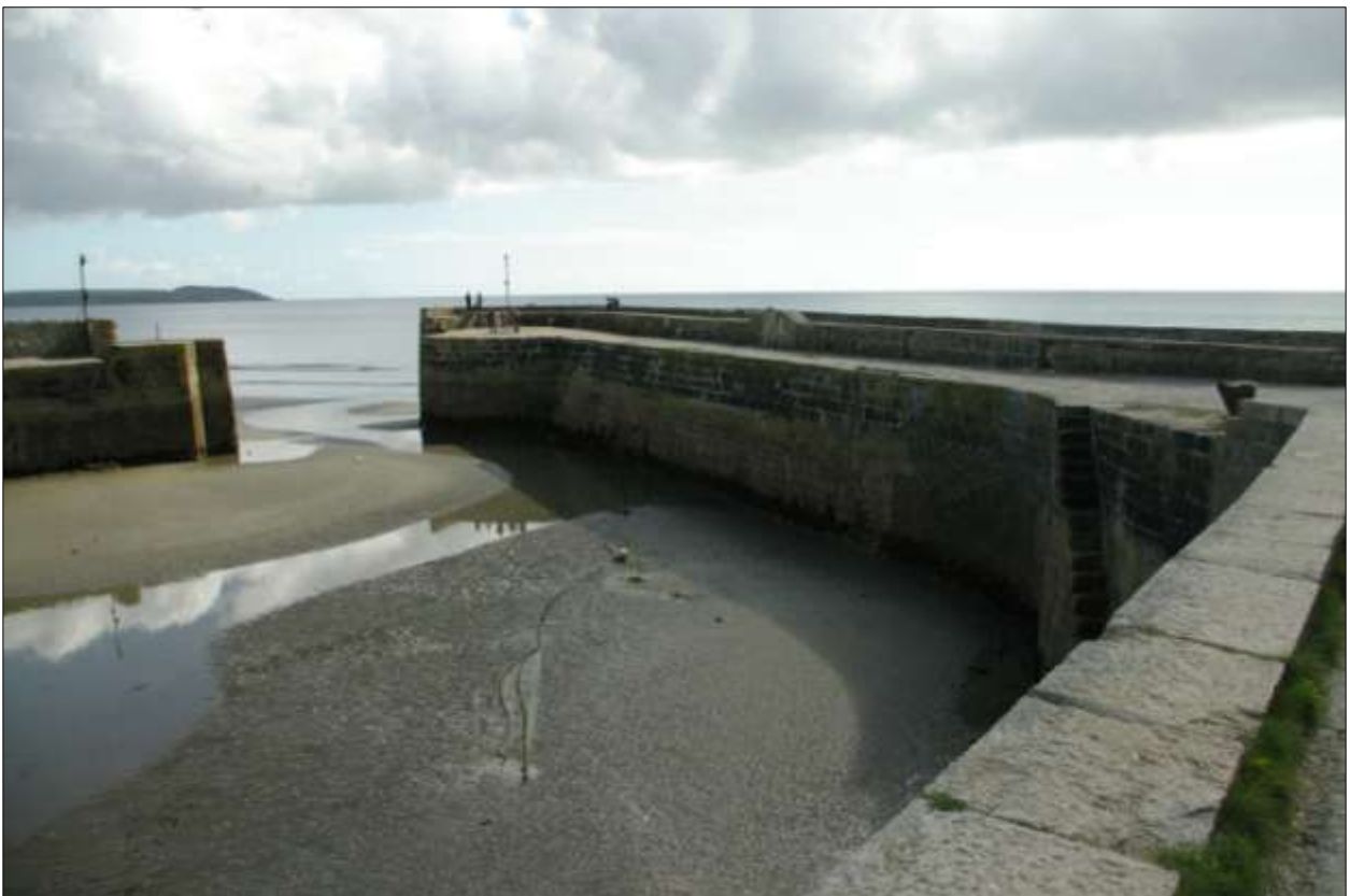
The Charlestown harbour outer basin wall; viewed from the north.
