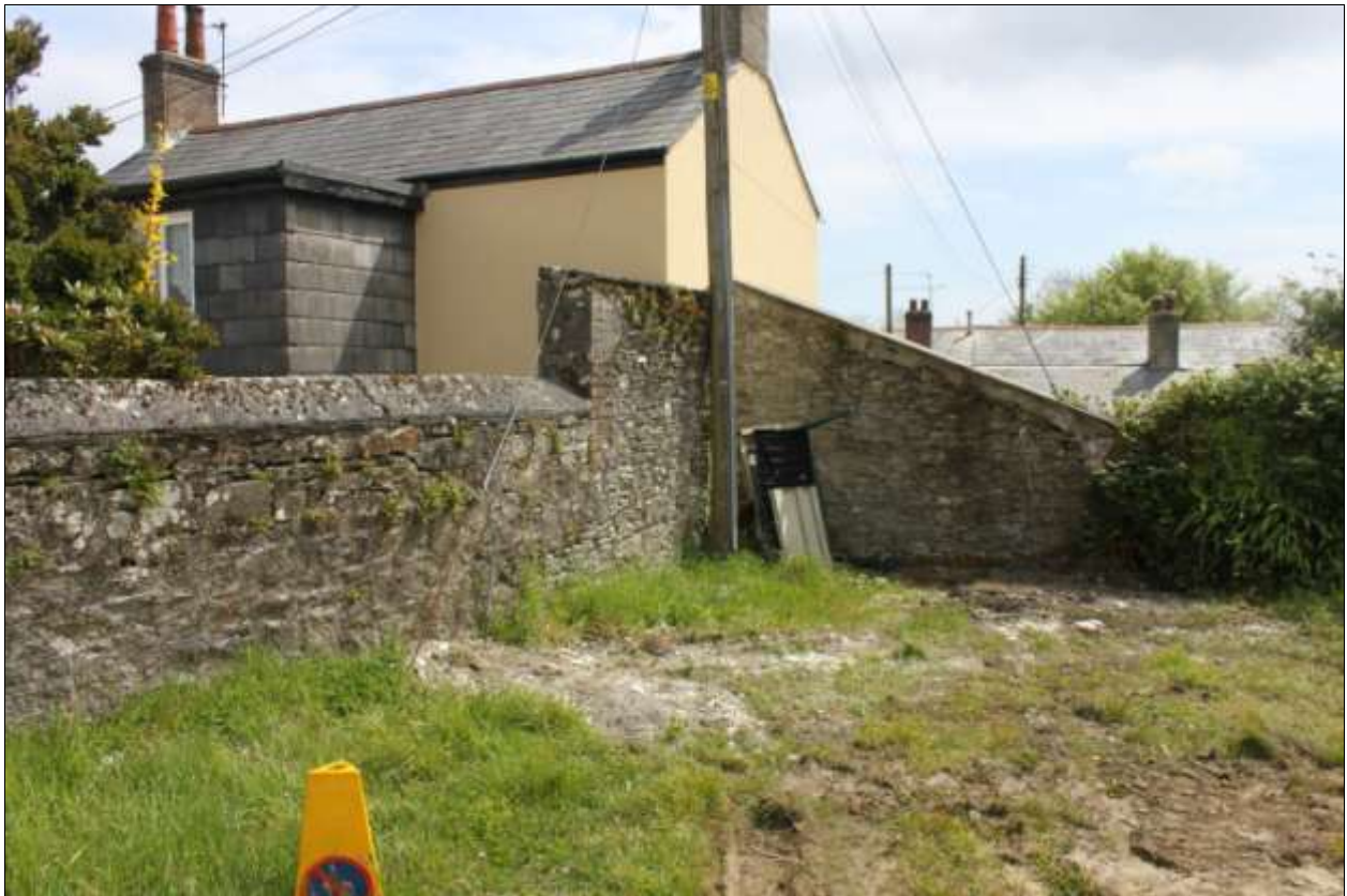
View of the south-eastern corner of the former yard, viewed from the north-west.
