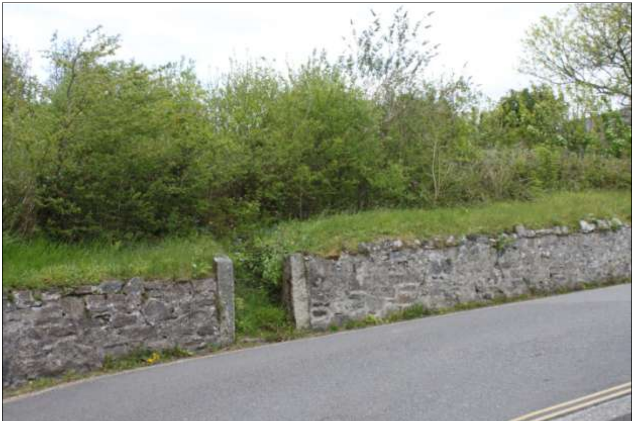
Gateway into the gardens, viewed from the south.
