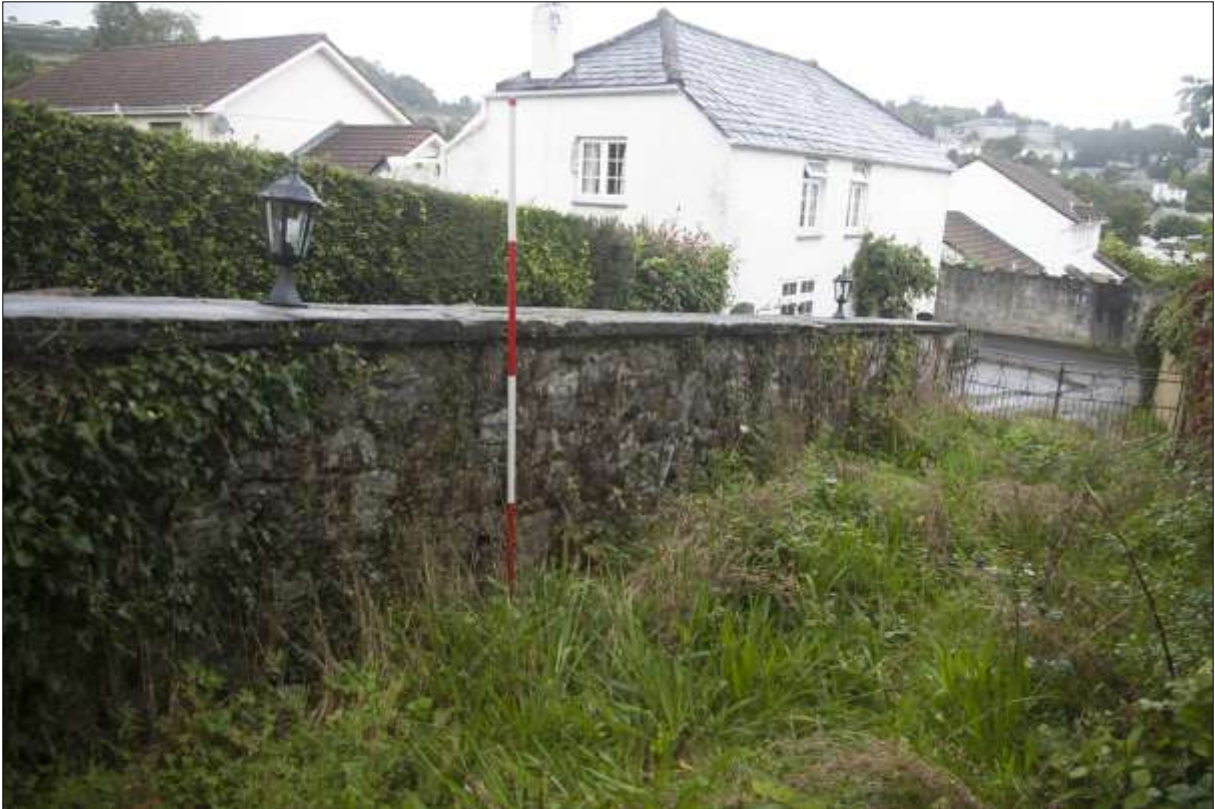
The north-eastern wall of the site; viewed from the south, looking north (scale 2m).
