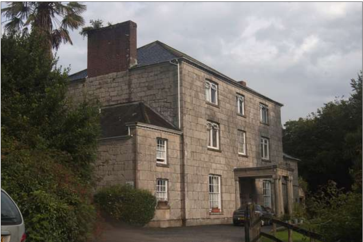
The south-east elevation of Trevarrick House; viewed from the south, looking north.
