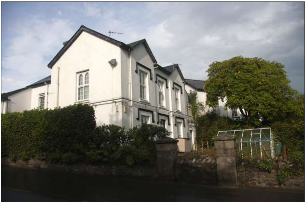
The surviving part of Trevarrick Terrace; viewed from the south-east, looking north-west.
