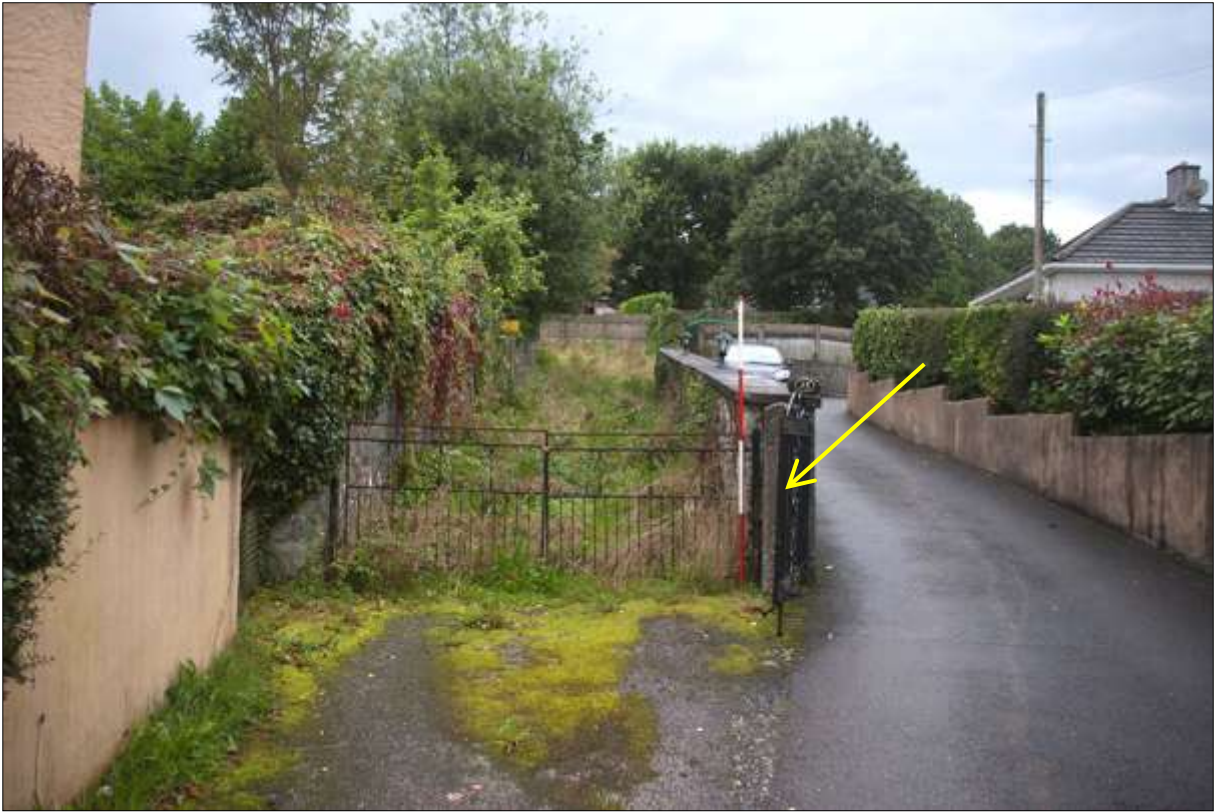
The entrance to the site; viewed from the north-east, looking south-west (scale 2m); the granite gatepost is indicated.
