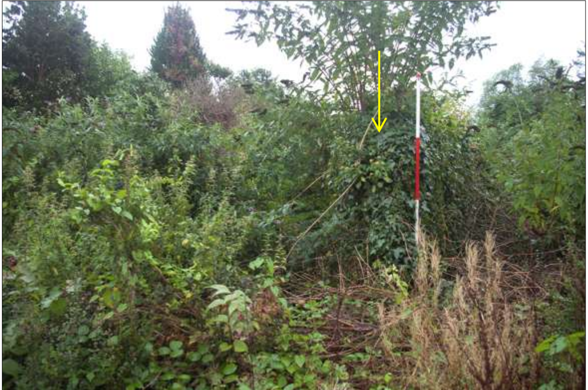
FIGURE 8: THE CENTRAL PART OF THE SITE, WITH THE IVY-COVERED WEST WALL OF B1 INDICATED; VIEWED FROM THE NORTH-WEST, LOOKING SOUTH-EAST (SCALE 2M).
