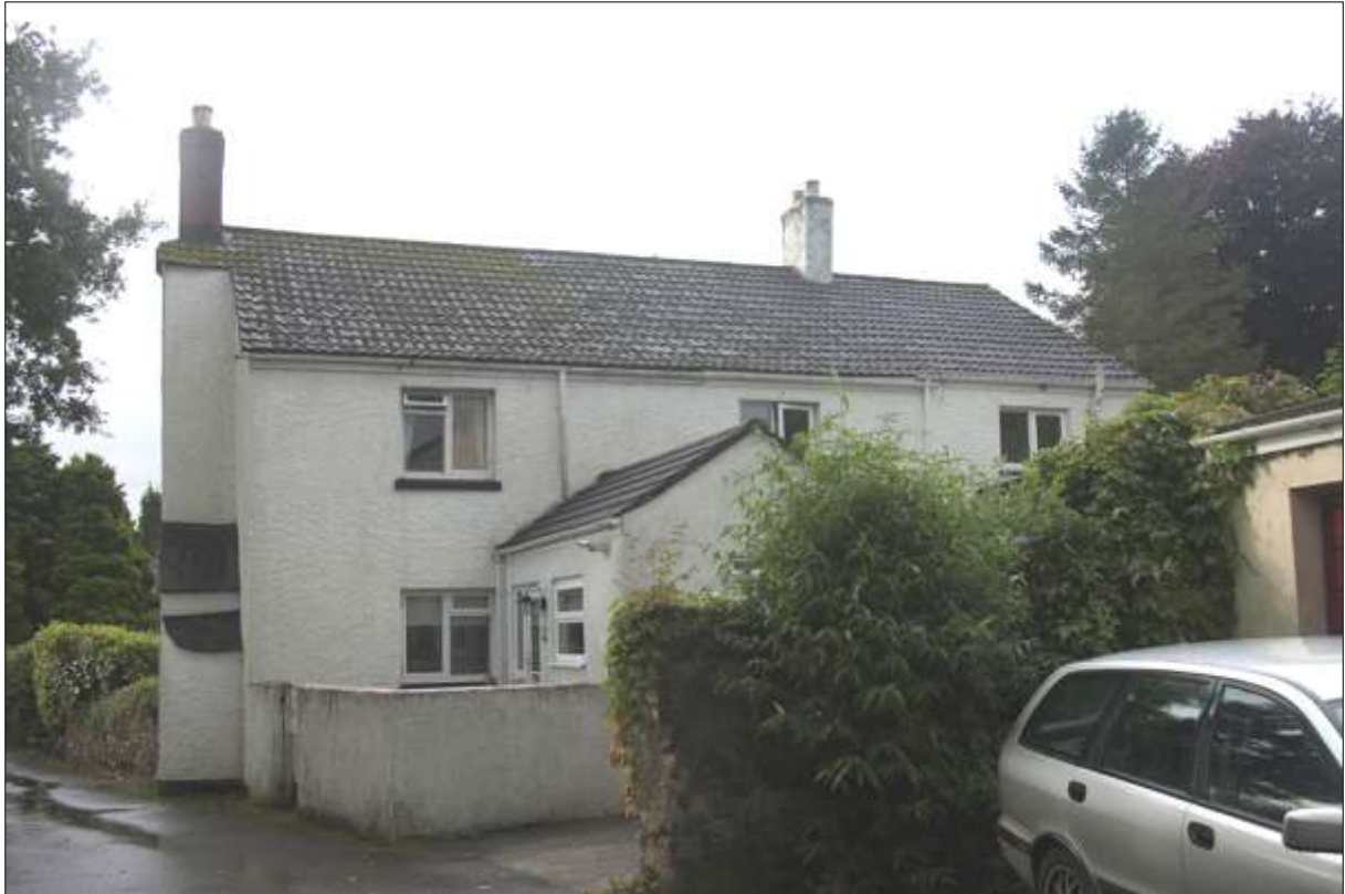
The north elevation of the property adjacent to the east, dated 1826; viewed from the north, looking south. Note the probable bread oven attached to the gable stack, and the change in window height to the right, indicating an extension.
