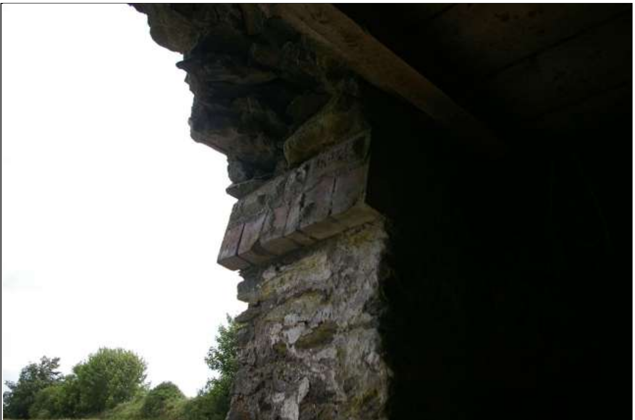
Detail of the collapsed brick arch in the southern opening in Barn 2's west elevation; from the south-east
