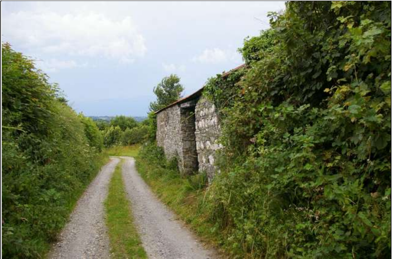
View of the east elevation of the barn range and farm lane; from the north-east.
