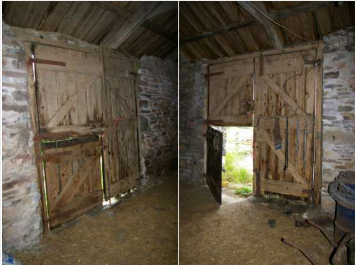
Left: The threshing doors in the east wall of Barn 1; from the north-west. Right: The threshing doors in the west wall of Barn 1; from the north-east.
