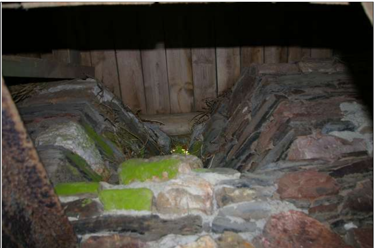
The slit air vent in the east elevation of Barn 2; from the west (below).
