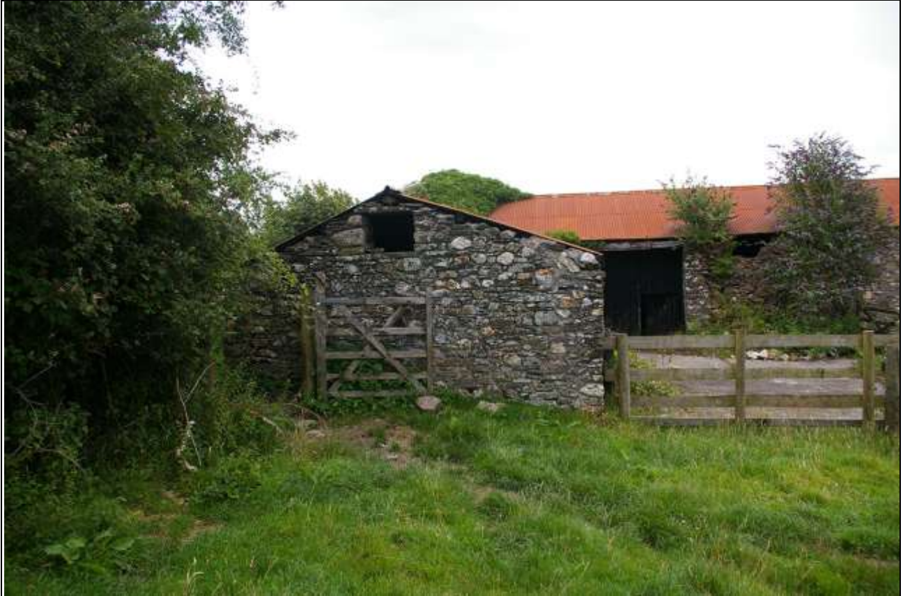
The west gable end of Barn 3; from the west.
