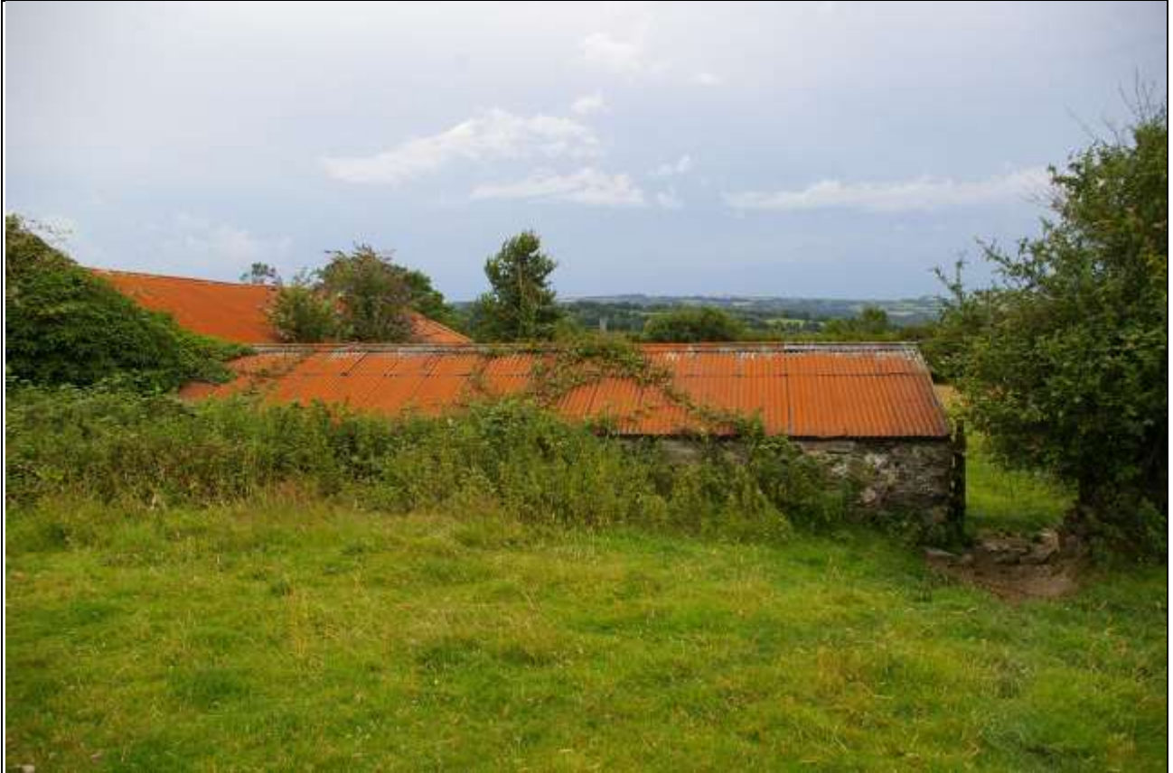
The north side of Barn 3, from the field; from the north-north-west.
