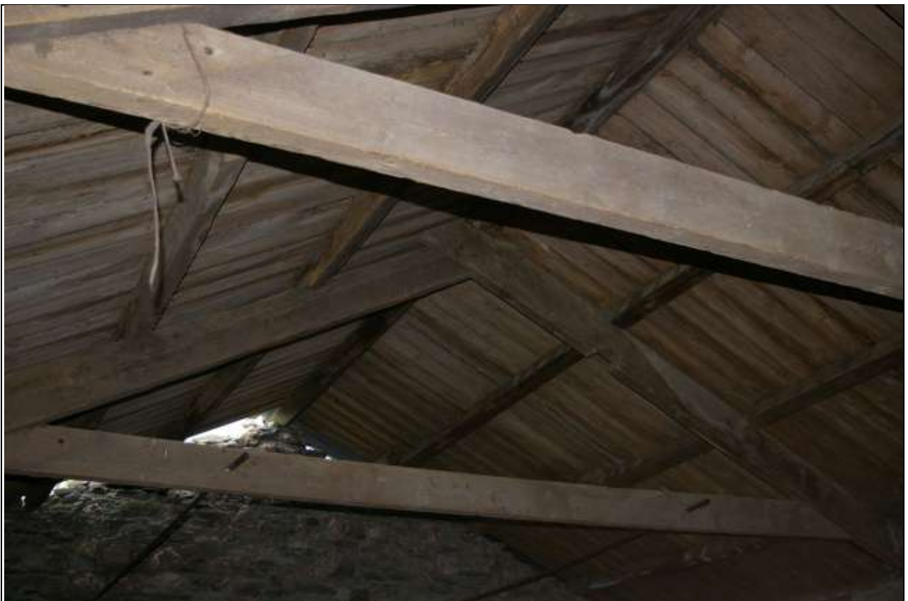
The roof structure over Barn 2; from the north-east.
