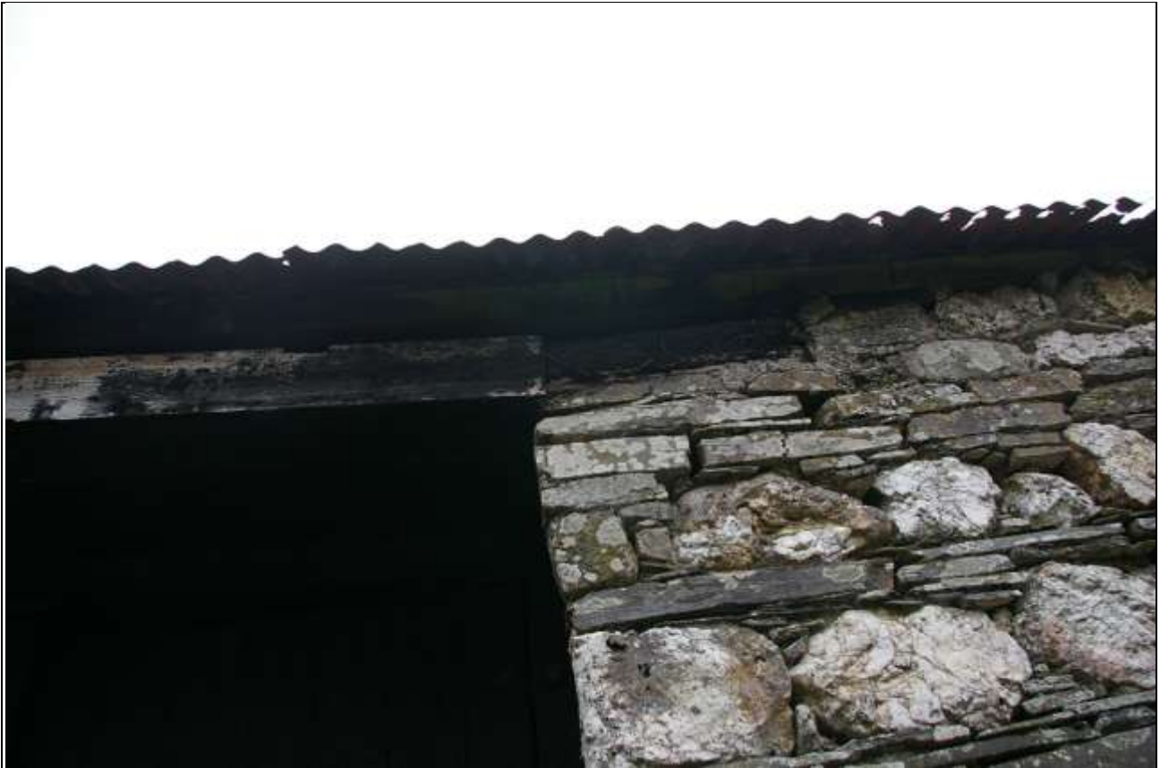
The heavy timber lintel over the opening in the east wall of Barn 1, with possible charring; from the east-south-east.
