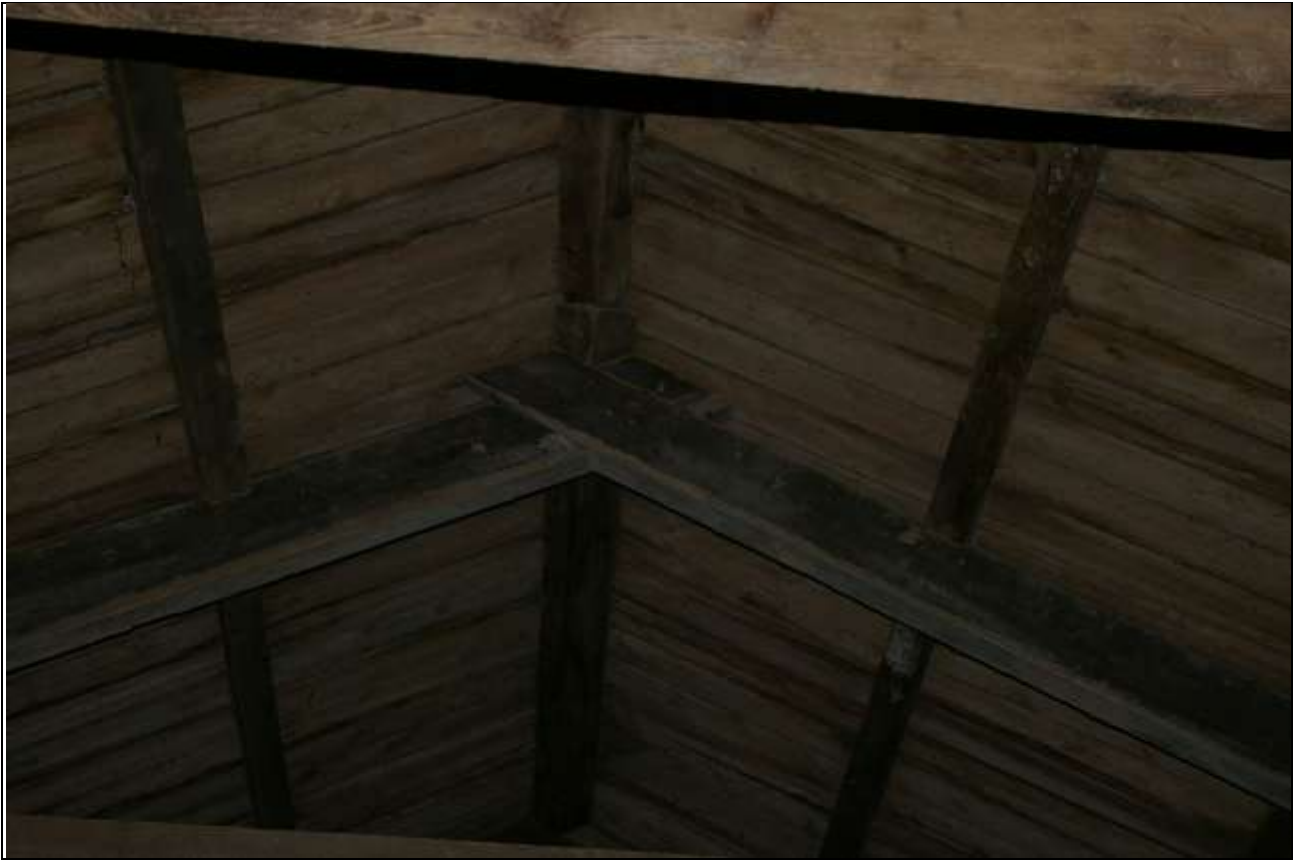
View of the ridge in Barn 1; from the south.
