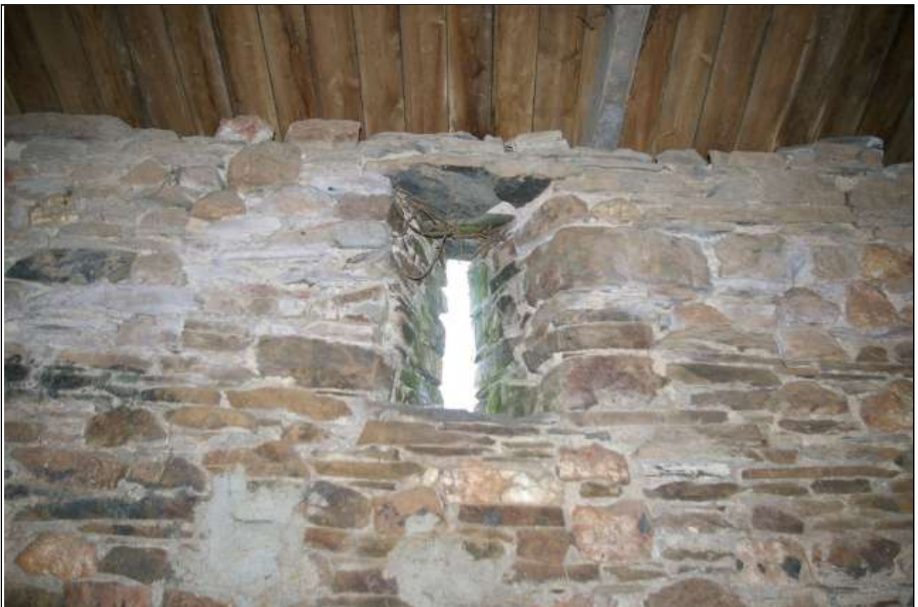
The interior face of the slit air vent in the east wall of Barn 1; from the west.
