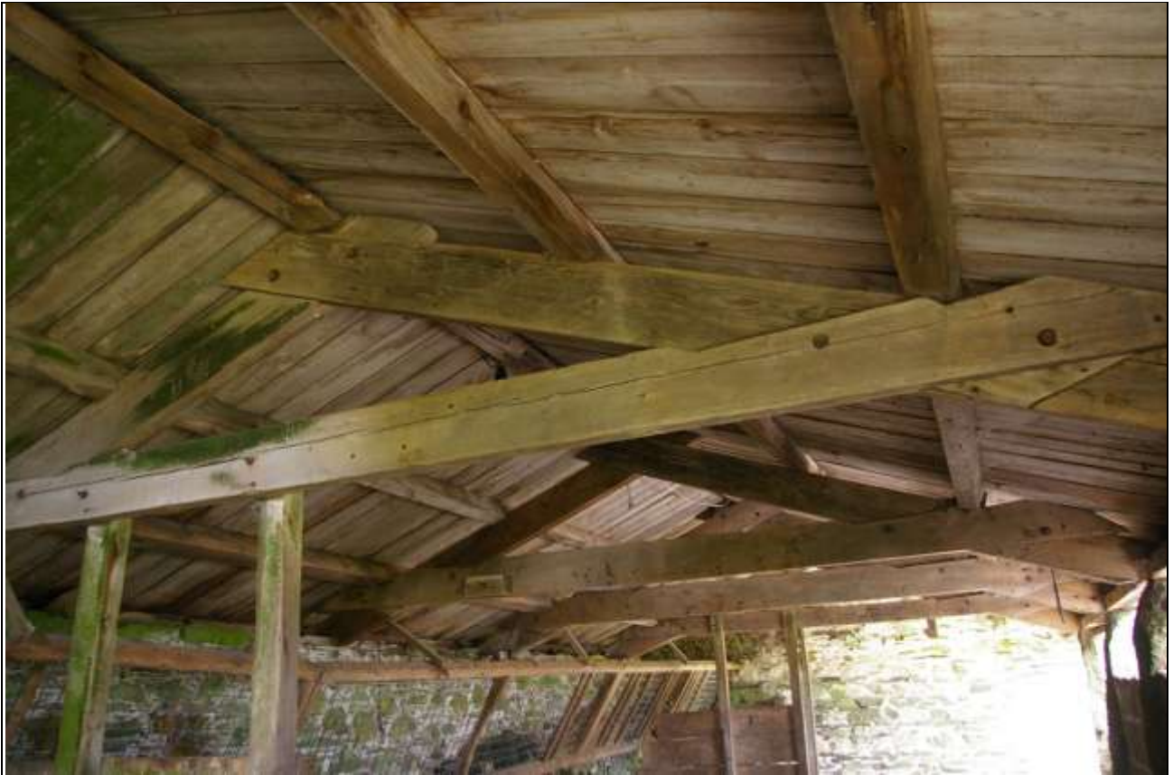
The roof structure in Barn 3; from the south-west corner.
