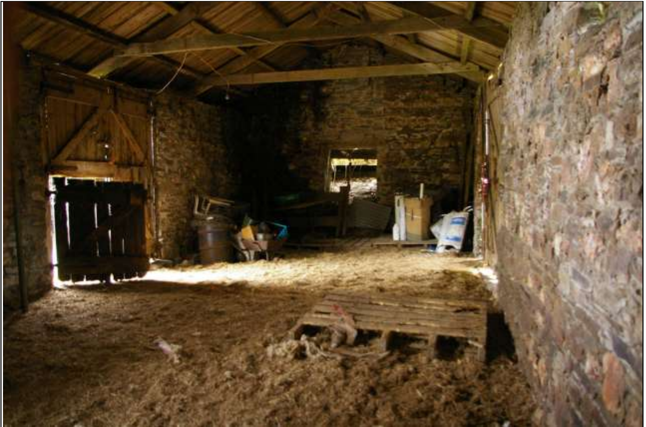
The interior of Barn 1; from the south-east corner.
