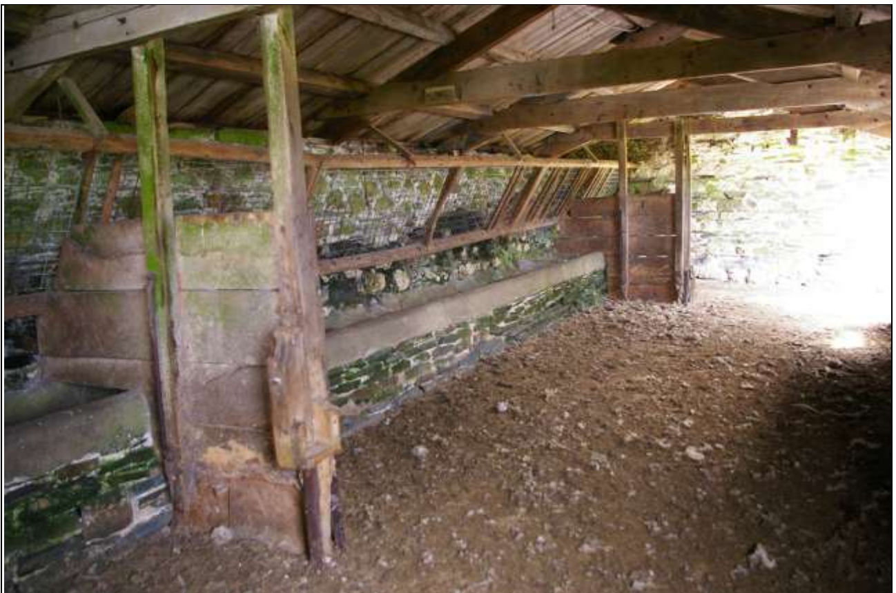
The troughs and partitions in Barn 3; from the south-west corner.
