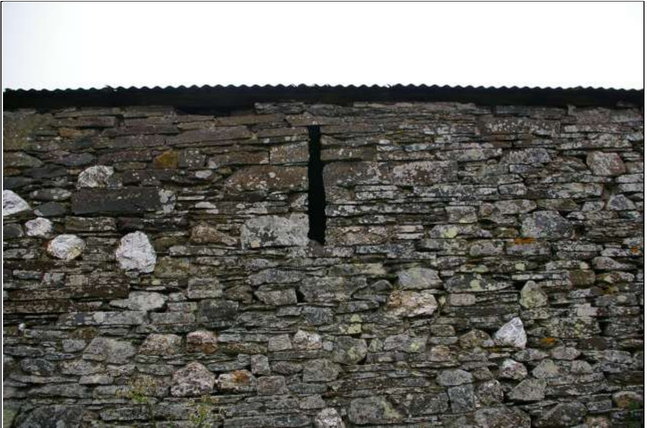
The air vent in the south end of Barn 1's east elevation; from the east.
