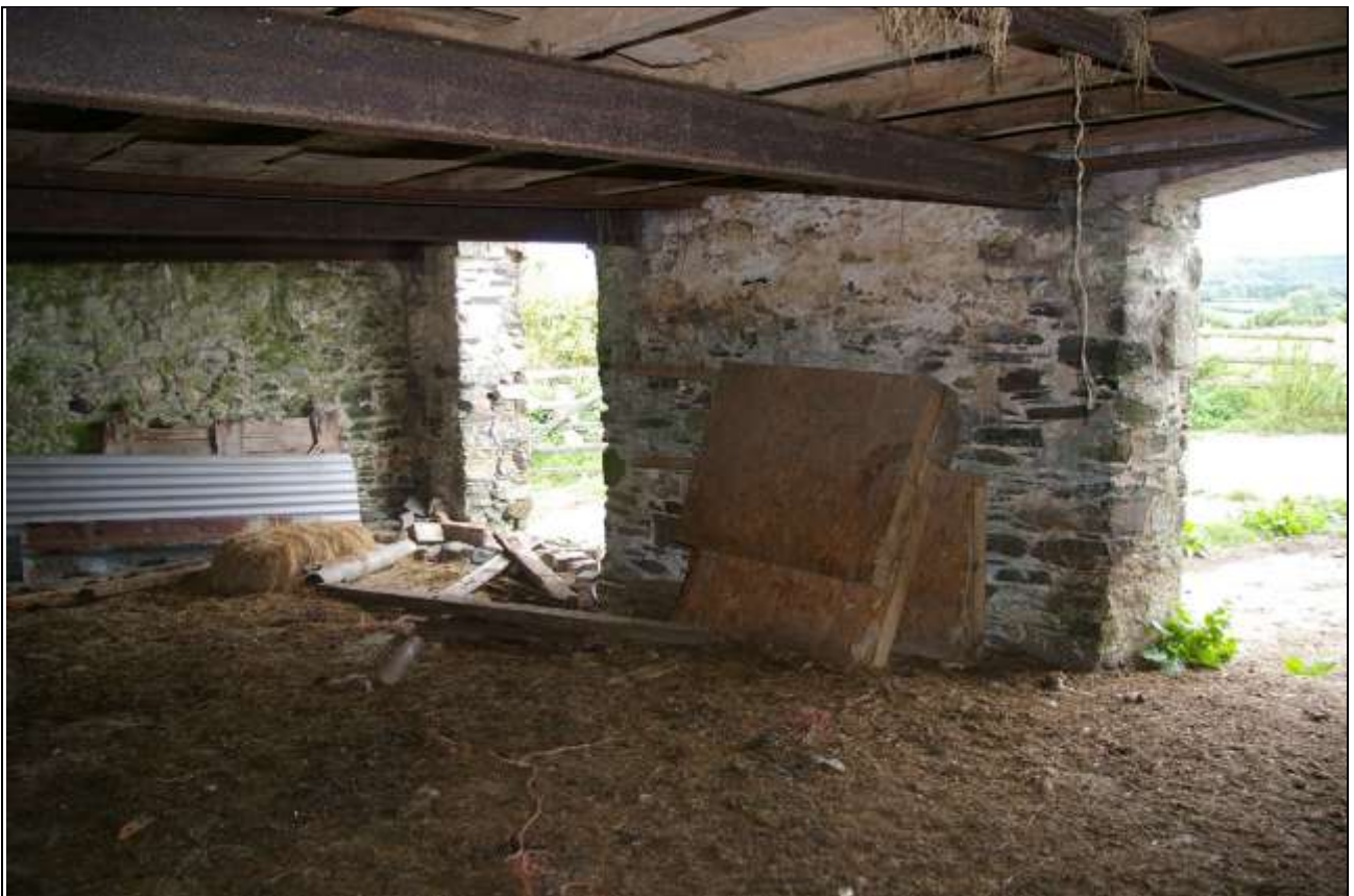
The interior of Barn 2; from the north-east corner.
