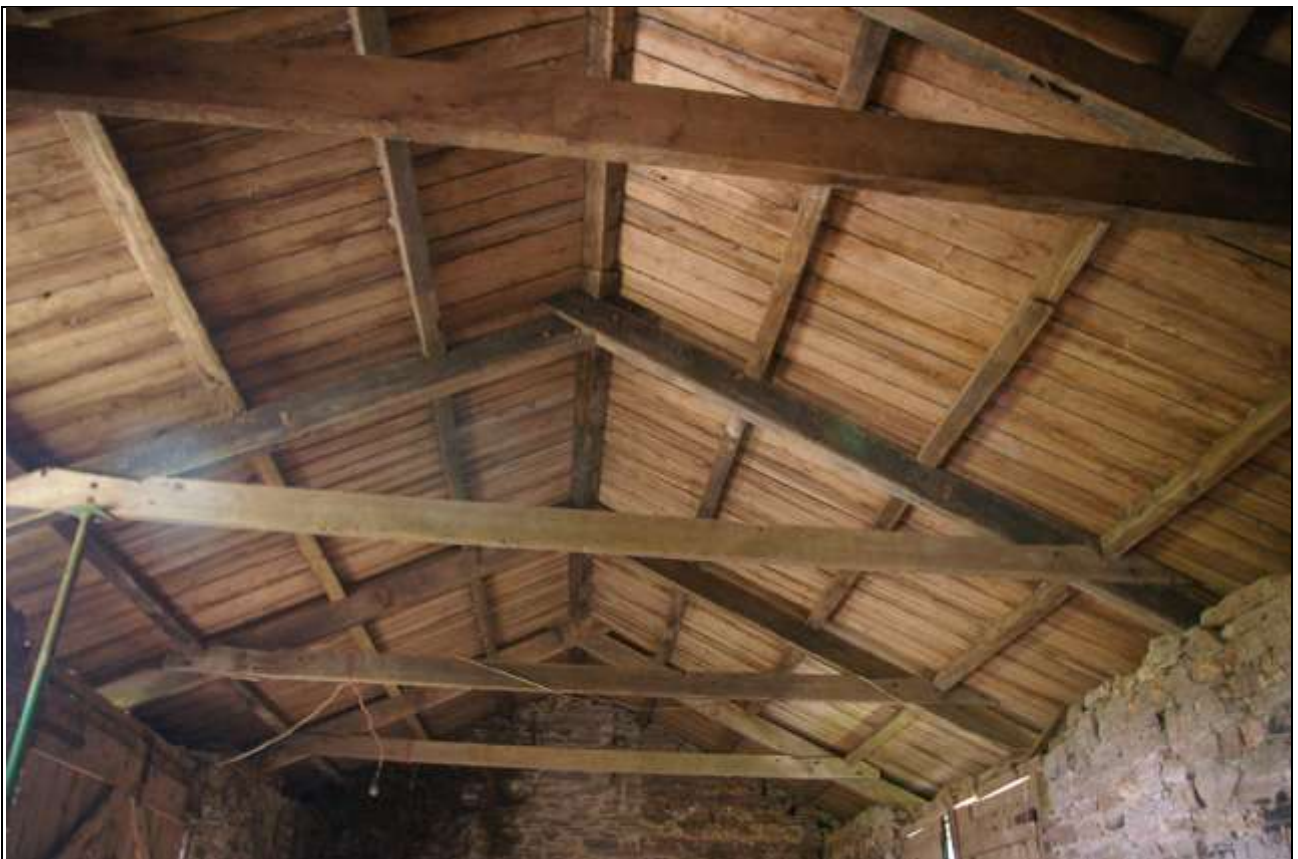
The roof structure in Barn 1; from the south.
