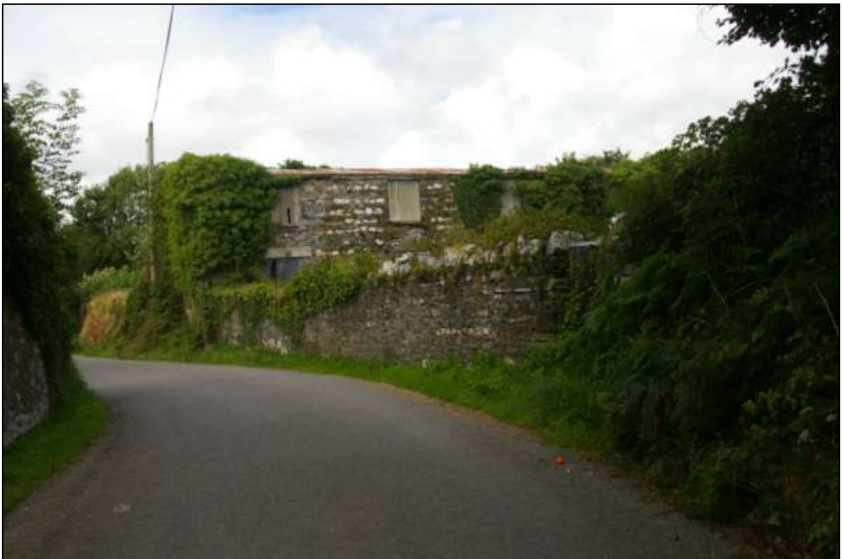
FIGURE 5: ONE OF THE BARNs AT DERRITON, SHOWING THE SAME ALTERNATING COURSES OF SLATE AND QUARTZ.
