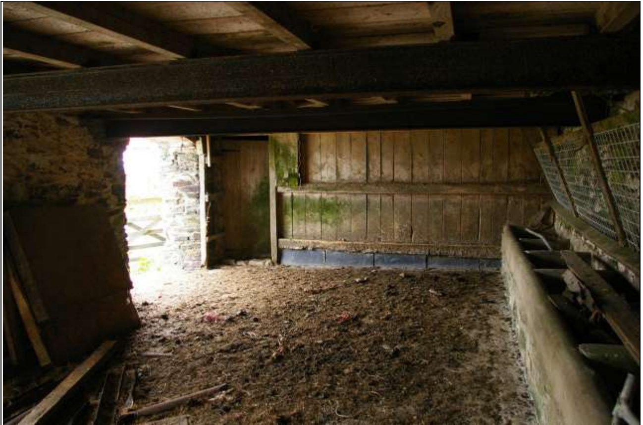
The interior of Barn 2; from the south-east corner.
