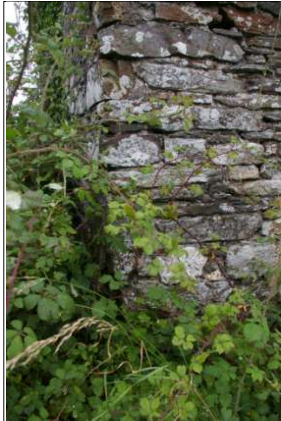
Very large flat slatestone slab used as a quoin in the south-east corner; from the east-south-east.
