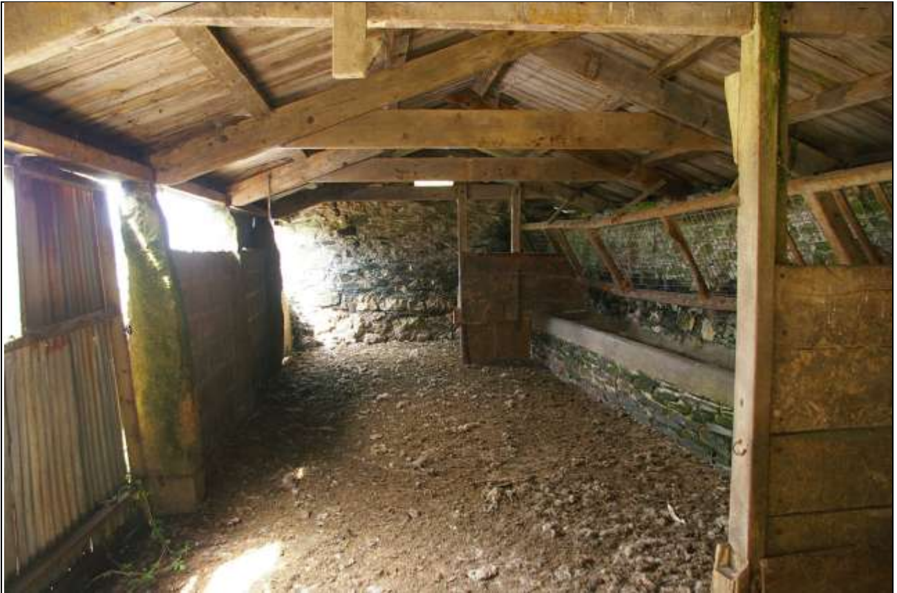
The interior of Barn 3; from the east.
