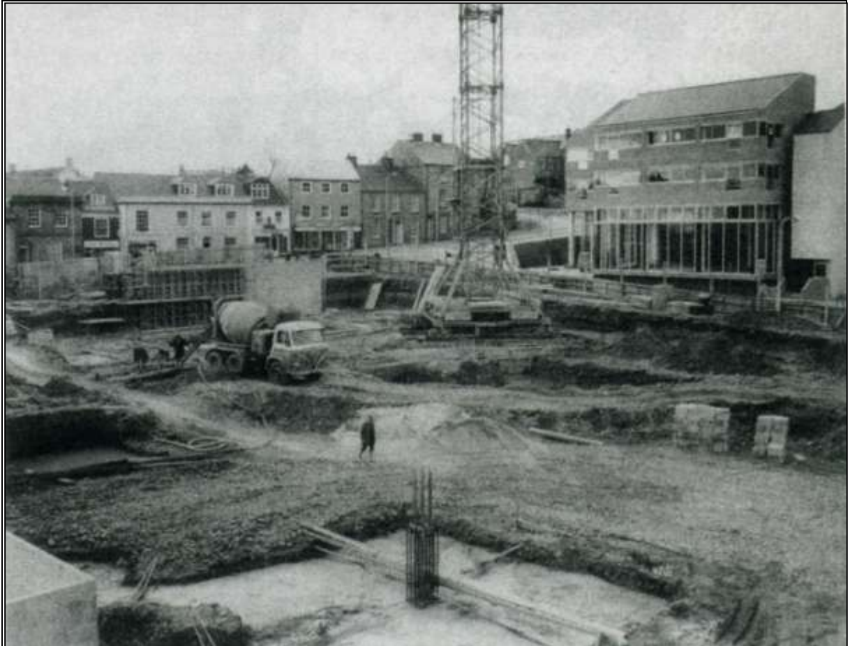
FIGURE 6: 1972 CONSTRUCTION OF ST CLEMENTS ROAD LINKING TRAFALGAR ROUNDABOUT & MORESK (QUEENINCORNWALL.BLOGSPOT.CO.UK).
