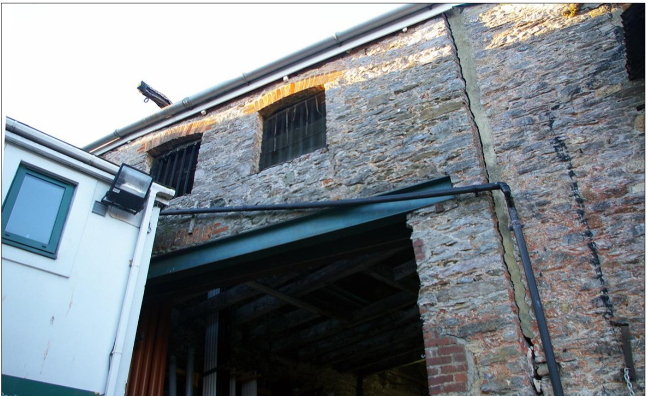
94. THE SOUTH ELEVATION OF B2, WITH LARGE FORCED GF OPENING D12 WITH W18 AND W19 ABOVE; VIEWED FROM THE SSE.
