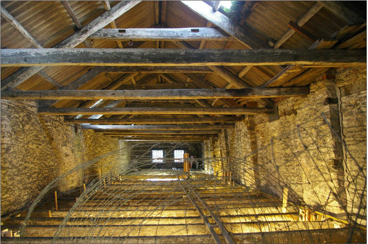
117. B2 SF INTERIOR; VIEWED FROM THE SOUTH.
