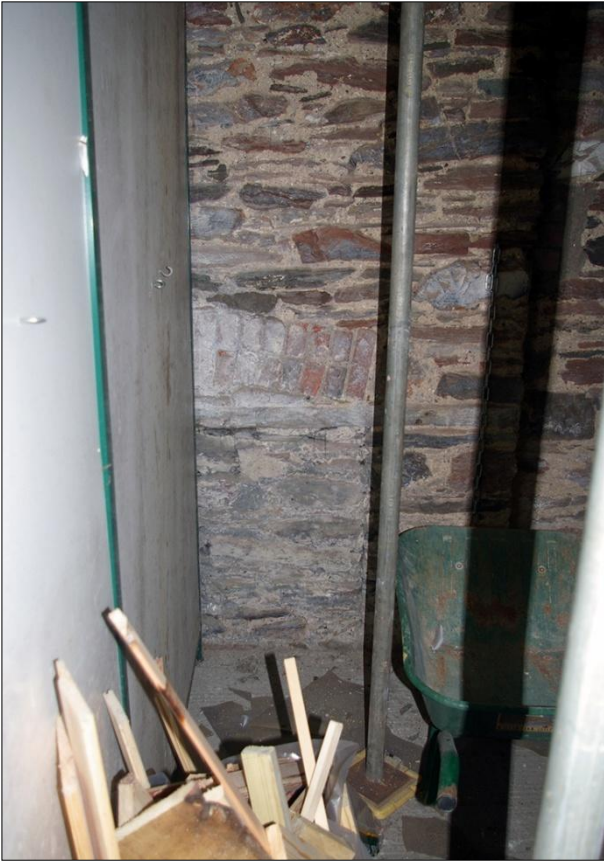
111. AS ABOVE, DETAIL OF FP1; VIEWED FROM THE SOUTH.
