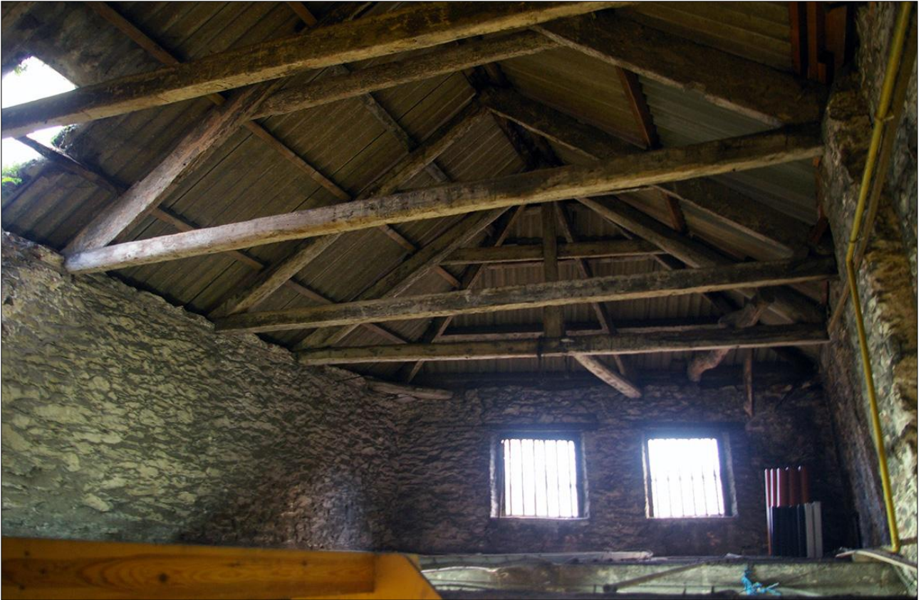
121. B2 SF INTERIOR; THE ROOF STRUCTURE OVER THE SOUTHERN END OF B2, W18 AND W19; VIEWED FROM THE NNW.
