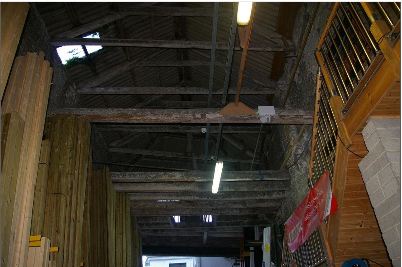
102. B2 INTERIOR, SHOWING THE SF JOISTS AND ROOF STRUCTURE; VIEWED FROM THE NORTH.
