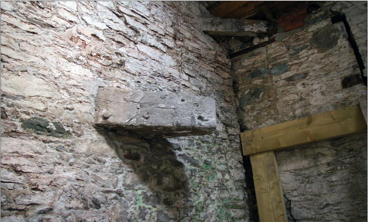
78. B1 FF R2, DETAIL OF THE DRAGON TIE (S11); VIEWED FROM THE WEST.
