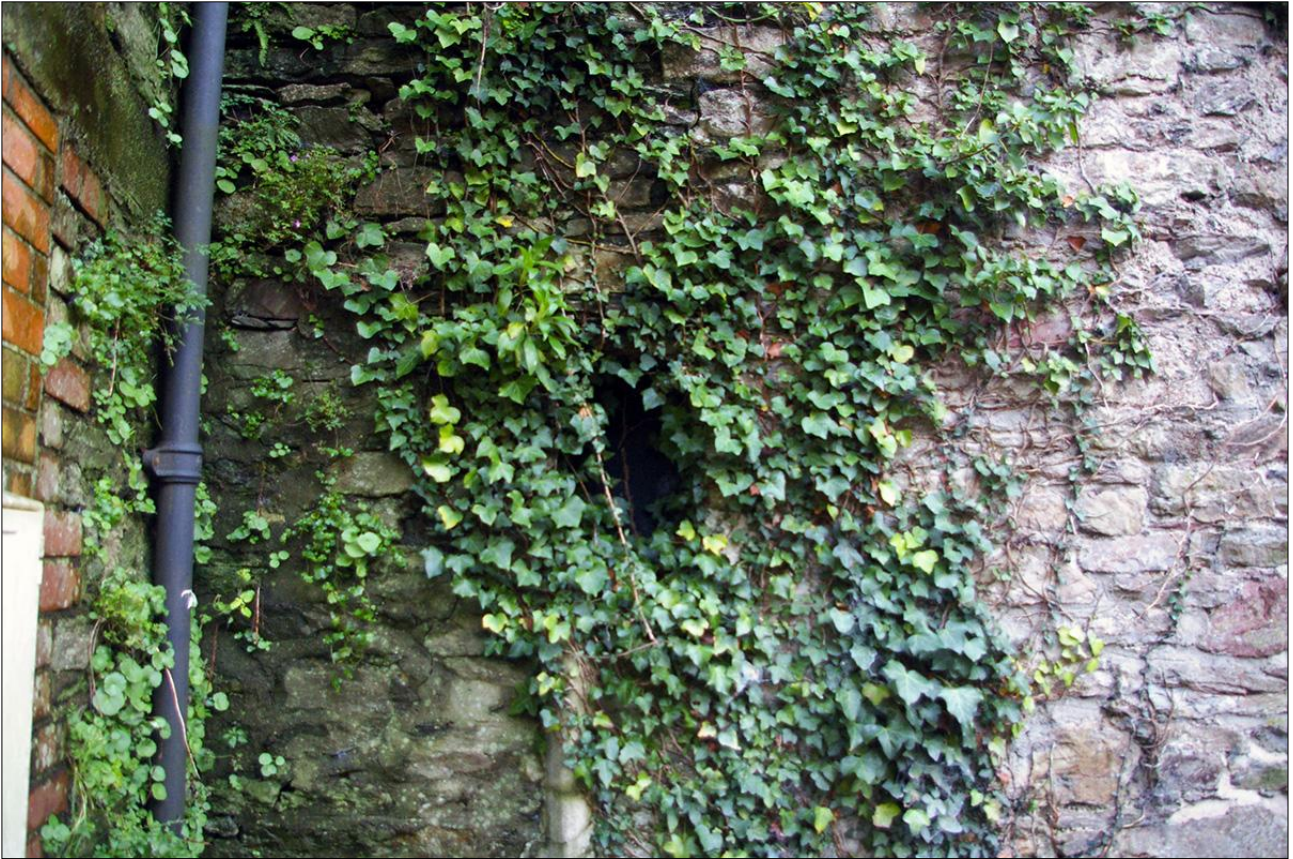
9. THE NORTH WALL OF B1, SHOWING GF WINDOW W8; VIEWED FROM THE NORTH.
