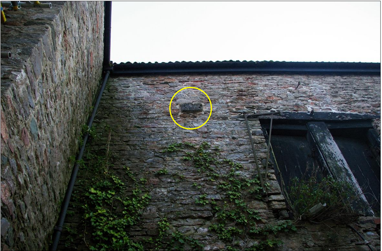
5. THE NORTH WALL OF B1, SHOWING THE SHEERLEGS AND THE PROJECTING STUB OF THE DRAGON TIE S11 (INDICATED); VIEWED FROM THE NORTH.
