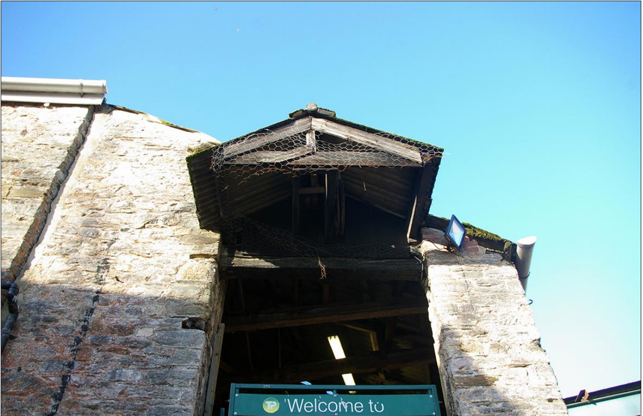
141. THE SOUTH ELEVATION OF B3, WITH FF LOADING DOOR D19 WITH PENTICE AND FLYWHEEL (S23) ABOVE; VIEWED FROM THE SOUTH.
