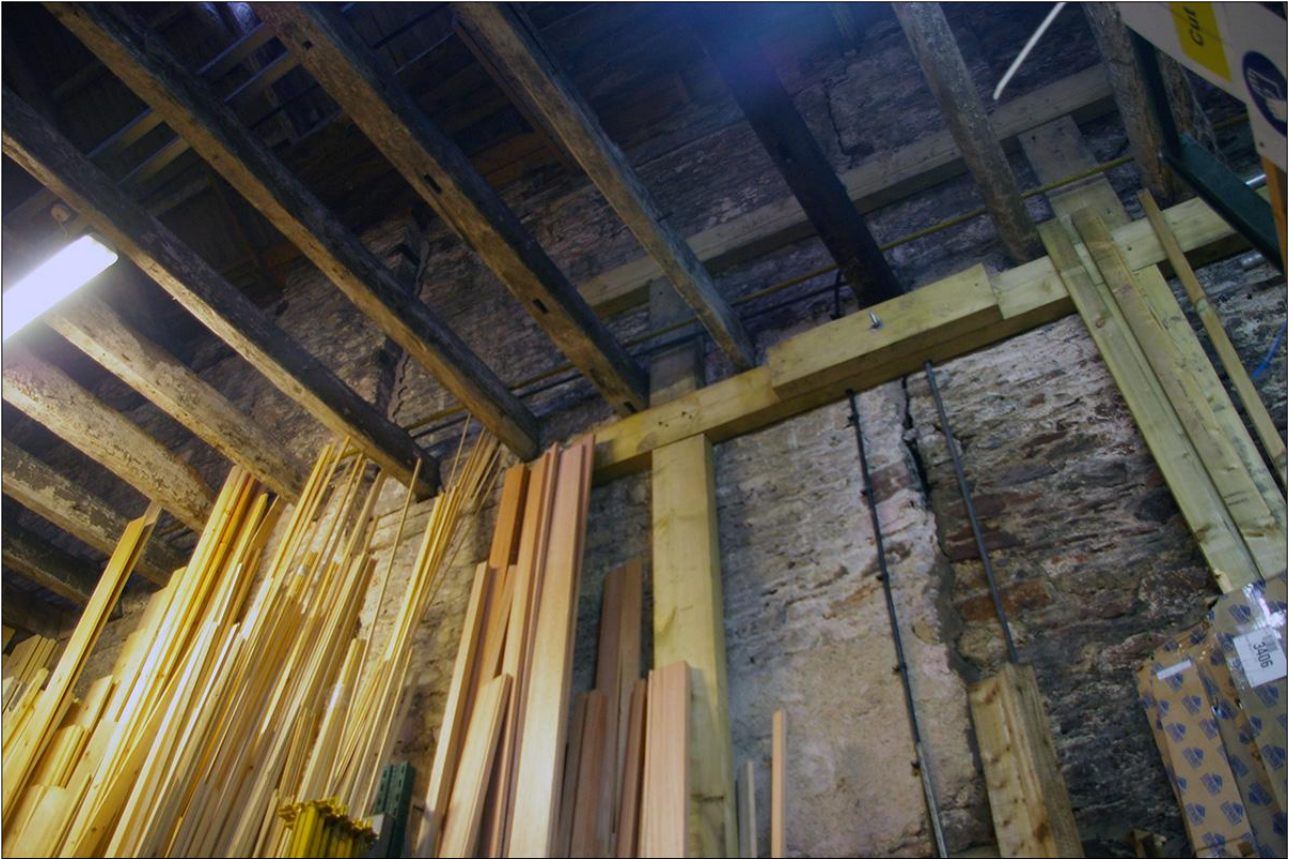
13. THE NORTHERN PART OF THE EAST WALL OF B1; VIEWED FROM THE ENE.
