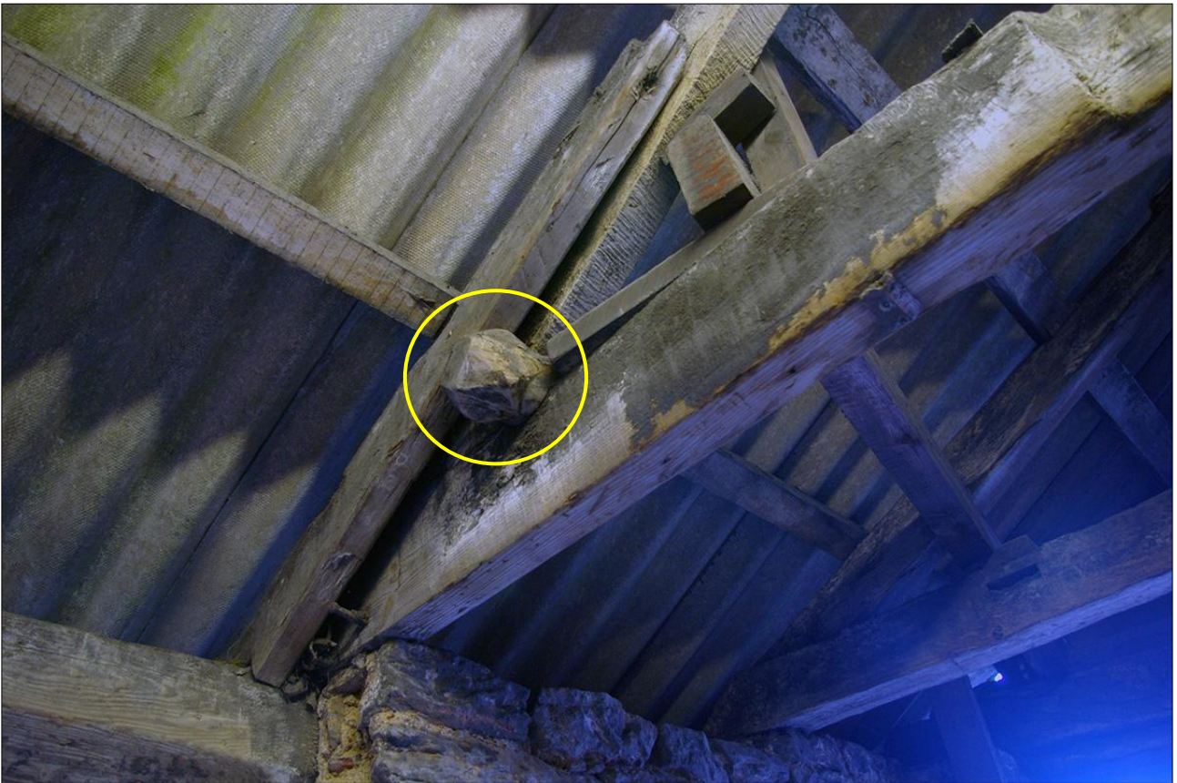
171. B3 ROOF STRUCTURE, SHOWING THE RE-USED SHAPED TIMBER (INDICATED) (S12); VIEWED FROM THE NNW.
