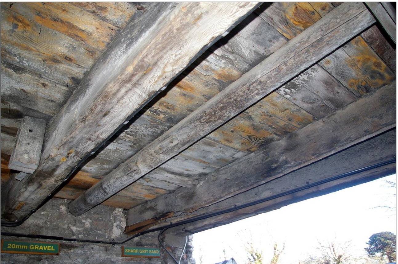
152. AS ABOVE, AT THE ENTRANCE (D13); VIEWED FROM THE WNW.
