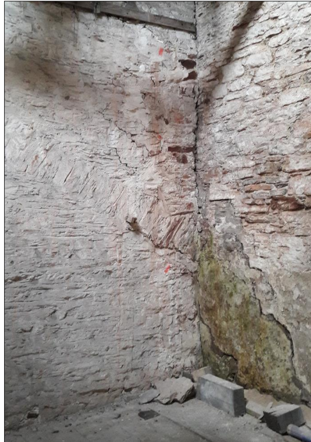
81. RIGHT: B1 FF R3, VIEW OF THE PARTY WALL WITH R1 SHOWING THE RELIEVING ARCH; VIEWED FROM THE NNE.
