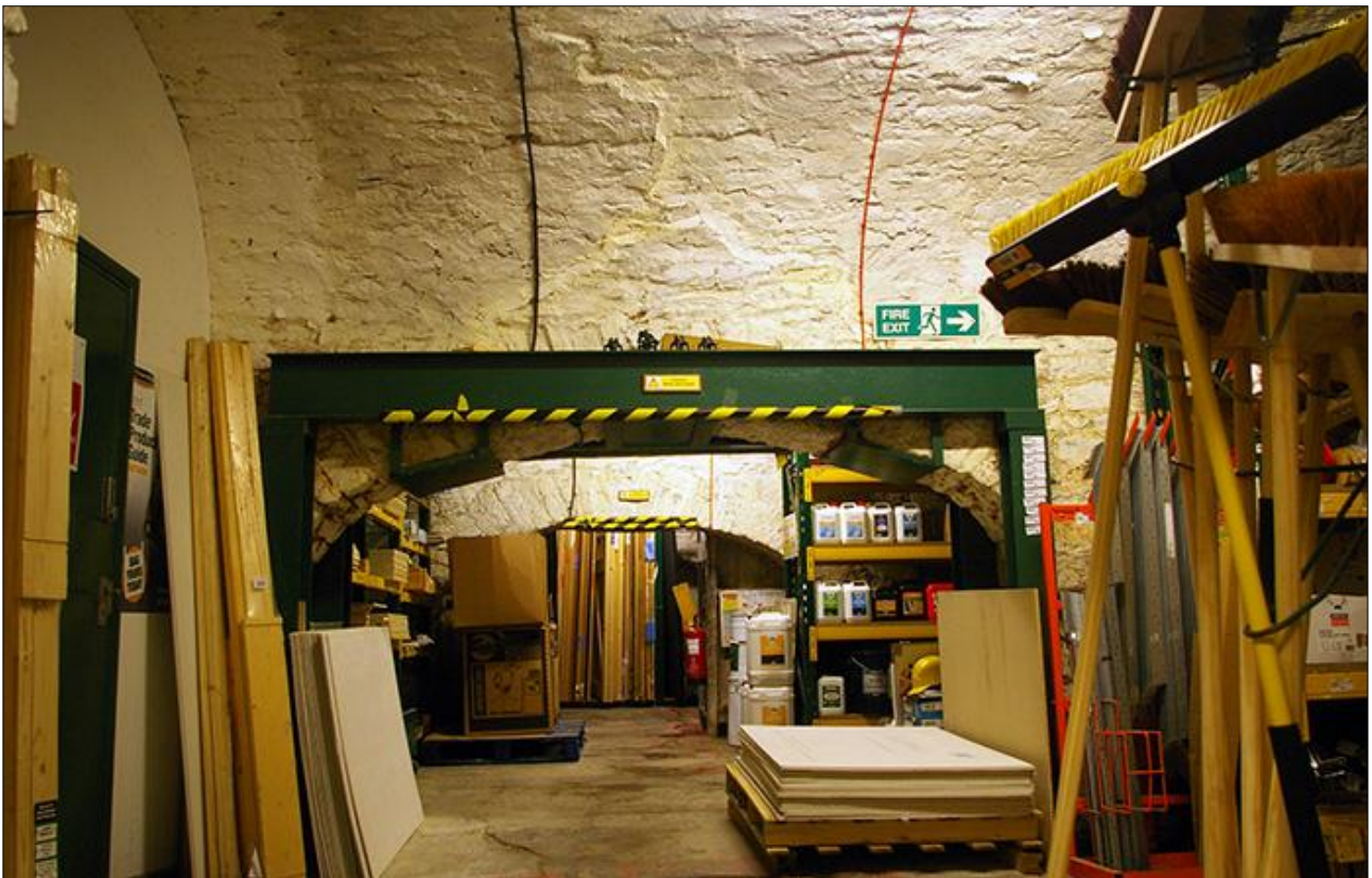
39. B1 GF, LOOKING THROUGH STEEL REINFORCED D4 FROM V3 INTO V4; VIEWED FROM THE SOUTH.
