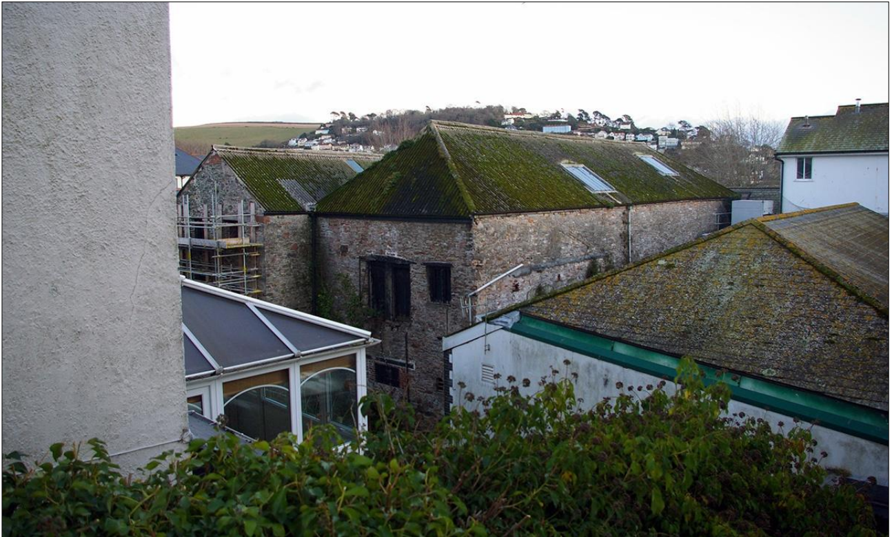
1. THE NORTH AND WEST WALLS OF BUILDING 1 (B1), VIEWED FROM THE NORTH-WEST.
