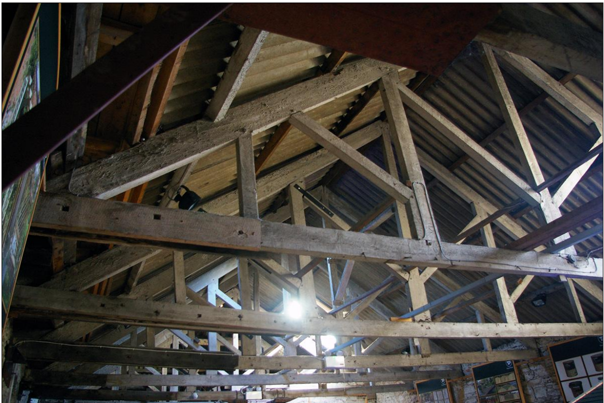
FIGURE 25: THE KINGPOST ROOF IN B1 WITHIN R1; VIEWED FROM THE NORTH-EAST.
