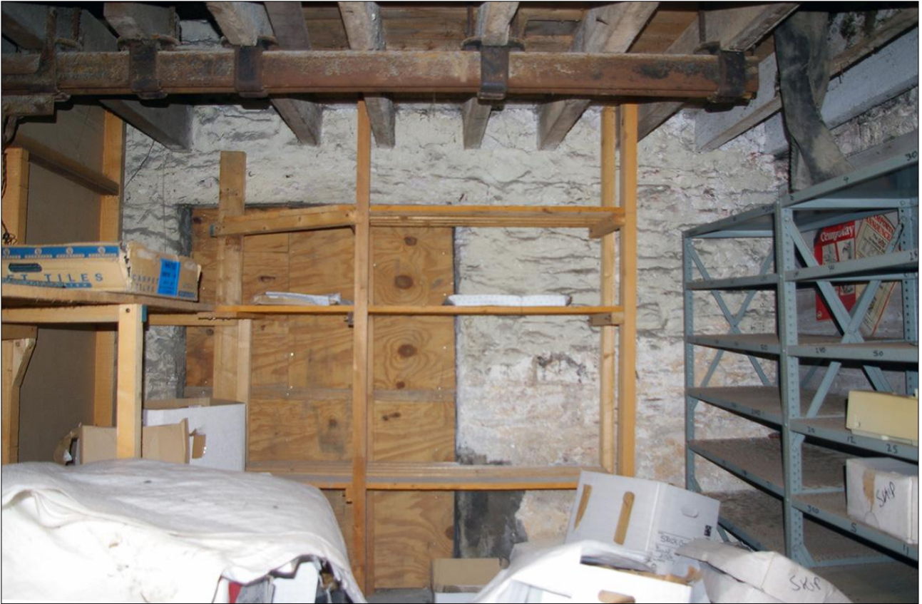
61. B1 FF R1A, VIEW OF BOARDED WINDOW W10, WITH RAIL FOR BAG HOIST AND LEATHER SLEEVE (RIGHT) ABOVE; VIEWED FROM THE NORTH.
