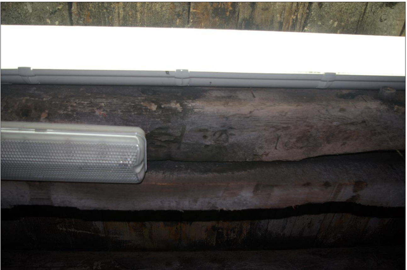
156. AS ABOVE, POSSIBLE GRAFFITI; VIEWED FROM THE SOUTH.
