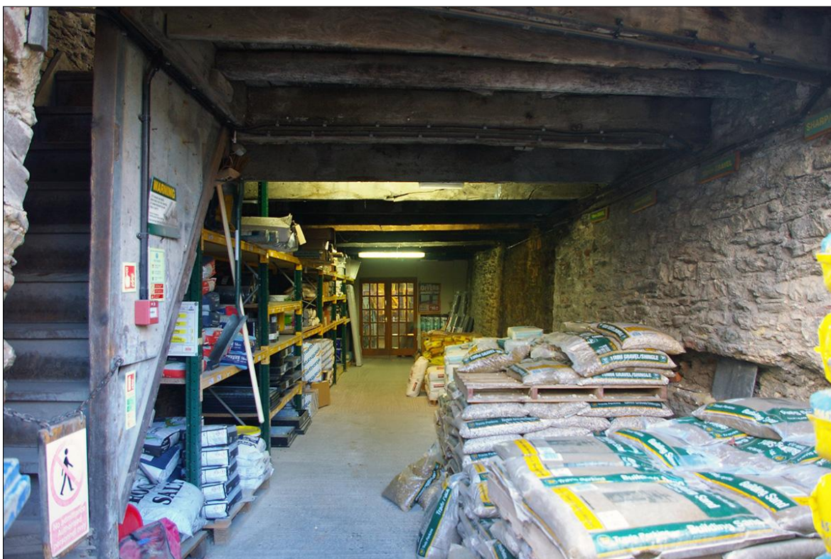
FIGURE 29: THE GROUND-FLOOR INTERIOR OF B3; VIEWED FROM THE SOUTH.
