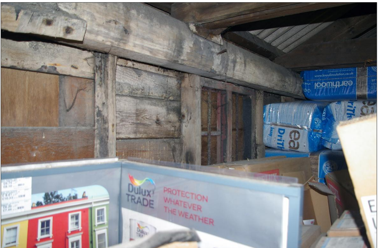
184. AS ABOVE; VIEWED FROM THE NORTH-WEST.
