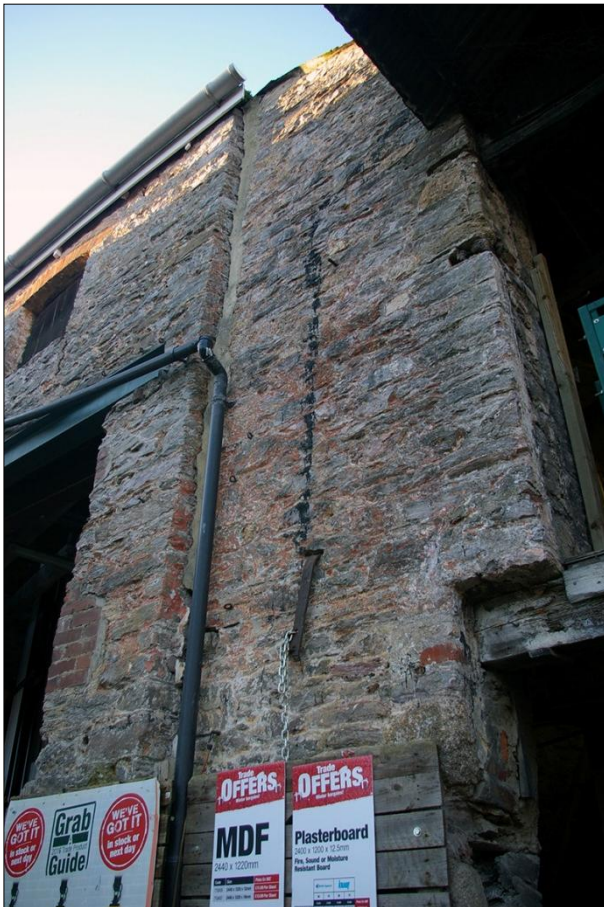
139. LEFT: THE SOUTH ELEVATION OF B3; VIEWED FROM THE SOUTH.
