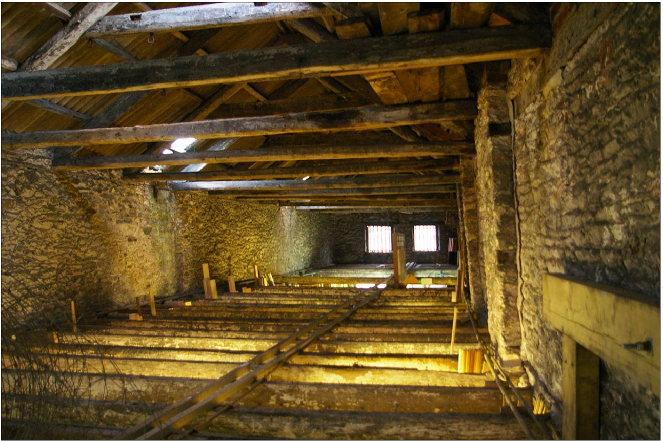
119. AS ABOVE; VIEWED FROM THE NNW.
