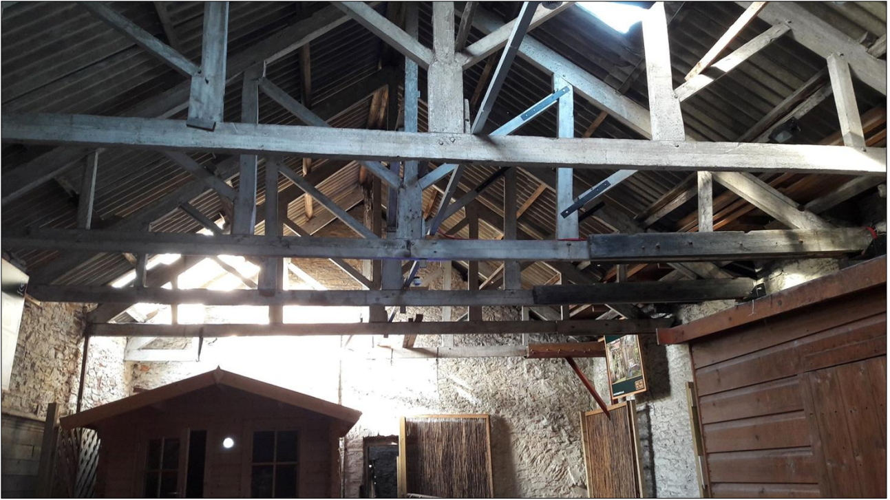
65. B1 FF, DETAIL OF THE ROOF STRUCTURE; VIEWED FROM THE SOUTH.
