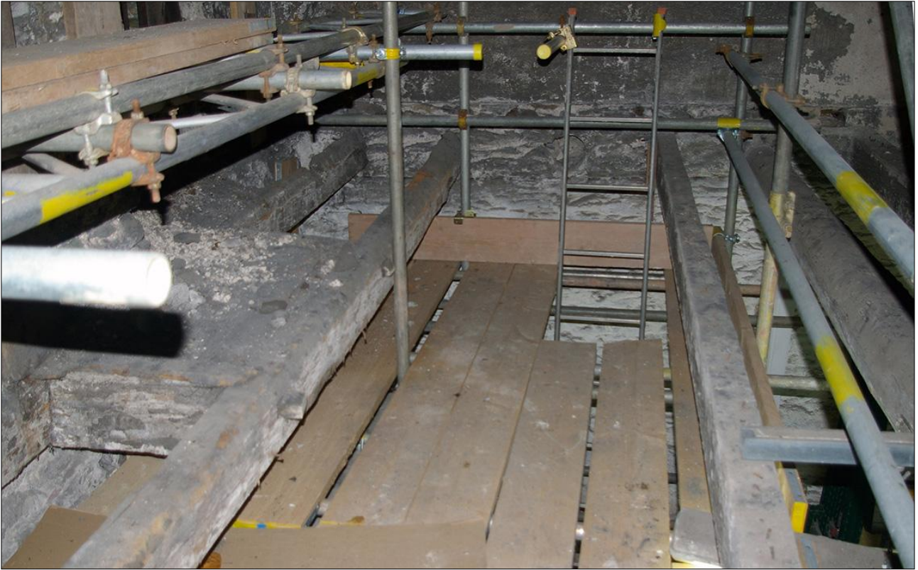
125. B2 SF INTERIOR, DETAIL OF THE BEAMS AT THE SOUTHERN END OF B2; VIEWED FROM THE WEST.
