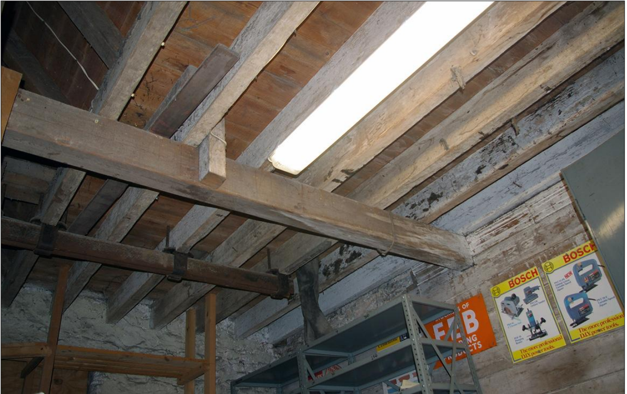
63. B1 FF R1, DETAIL OF THE JOISTS SUPPORTING THE HOPPER ABOVE; VIEWED FROM THE NORTH-EAST.
