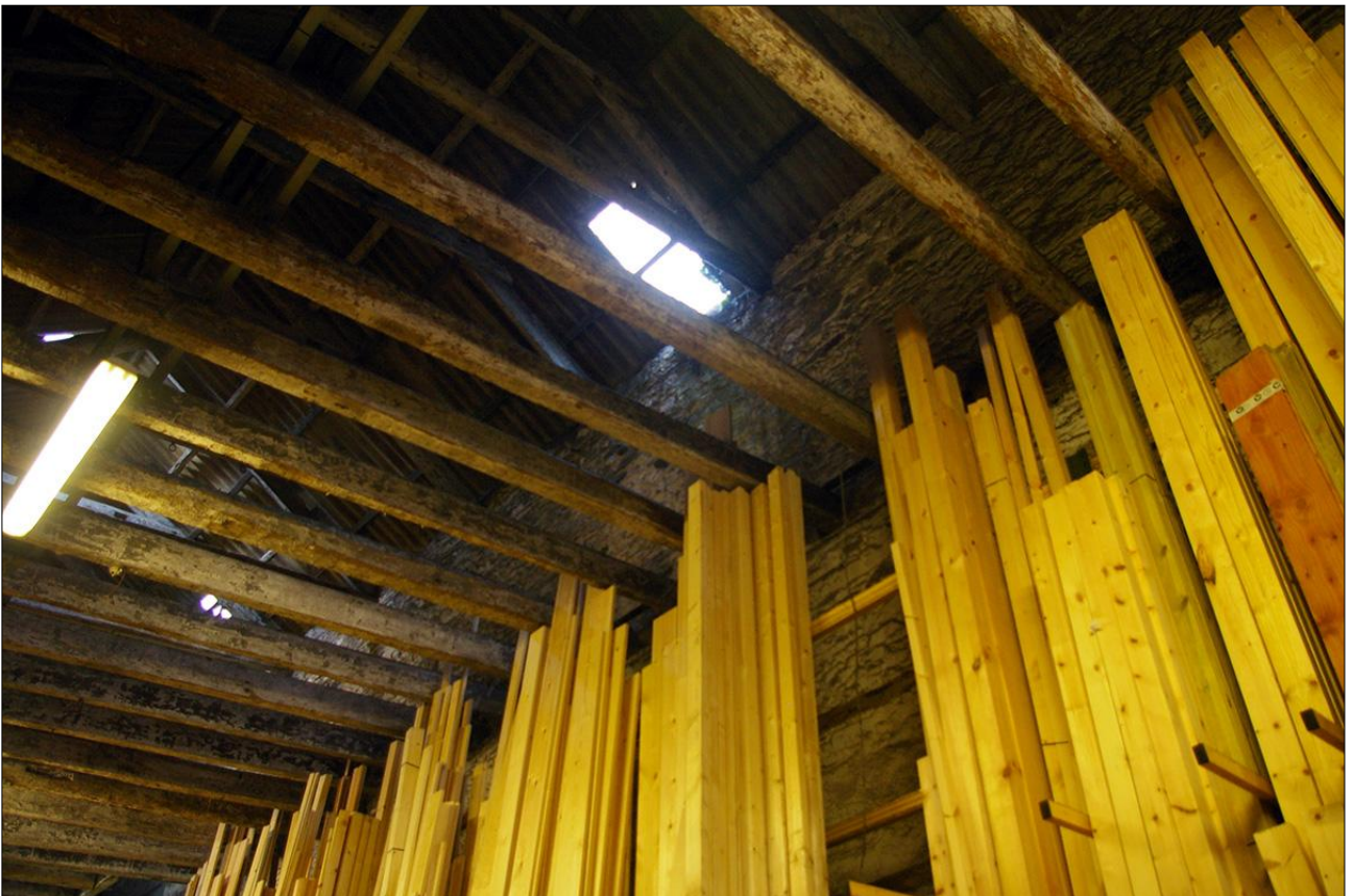
104. B2 INTERIOR, THE WEST WALL OF B2; VIEWED FROM THE SOUTH-WEST.
