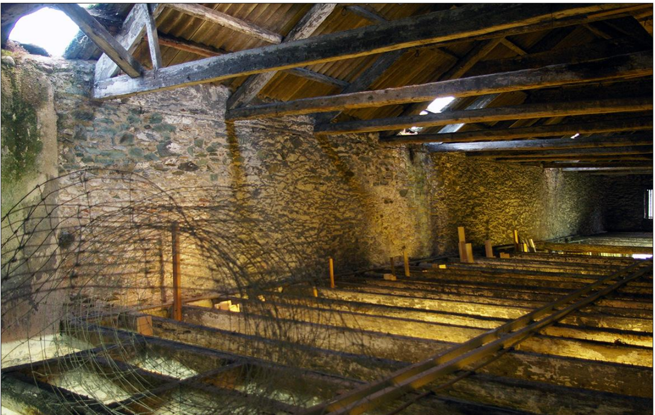
120. B2 SF INTERIOR, THE EAST WALL OF B2; VIEWED FROM THE NNW.
