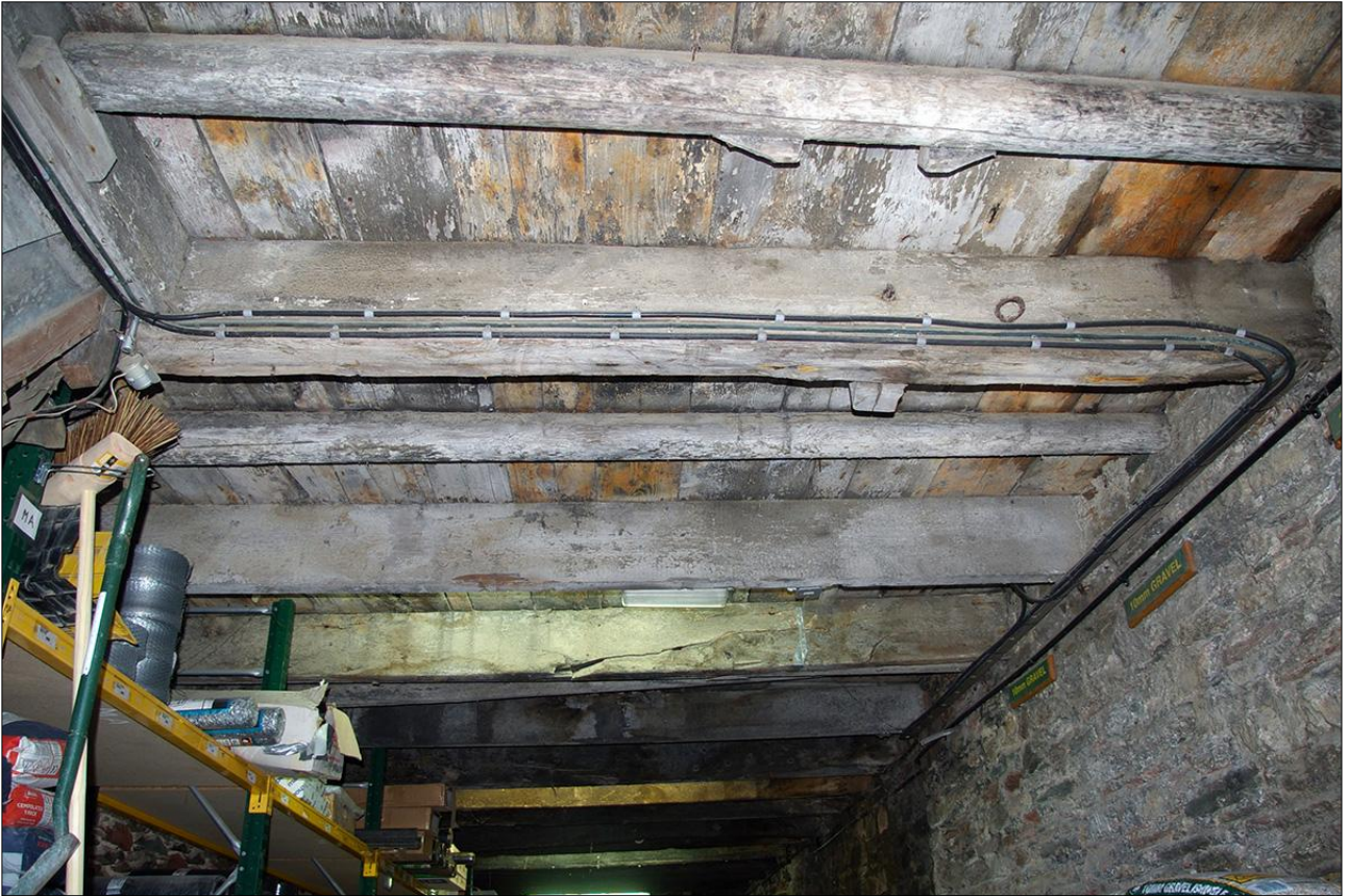
151. AS ABOVE; VIEWED FROM THE SOUTH.
