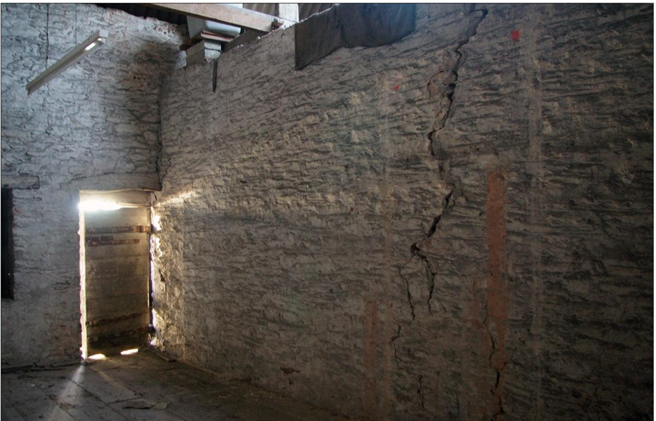
85. B1 FF R3, THE EAST WALL; VIEWED FROM THE SOUTH-WEST.
