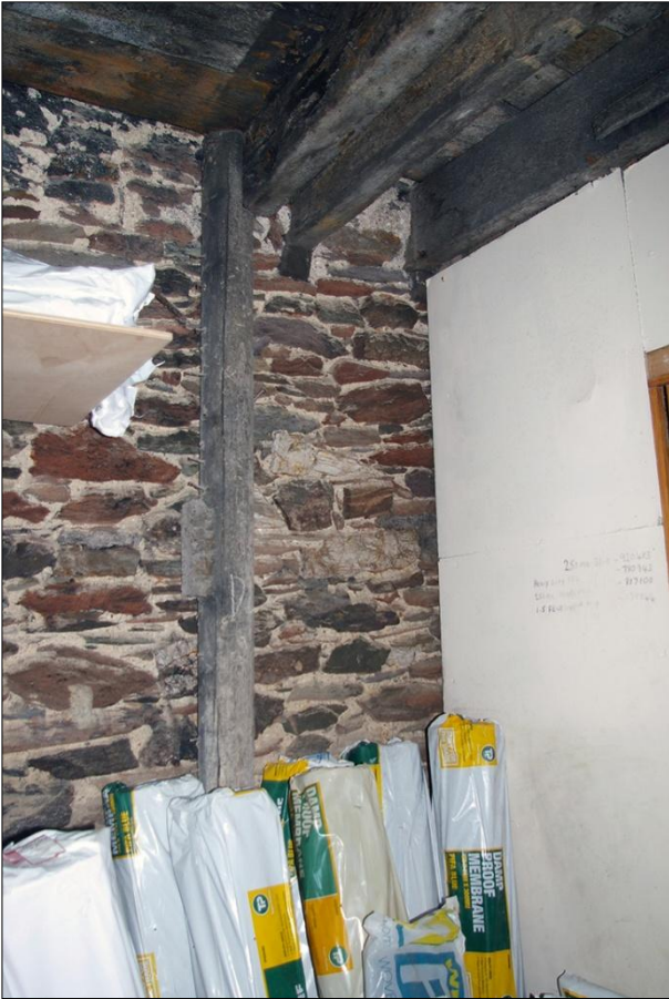
149. AS ABOVE, NEXT TO THE MODERN PARTITION; VIEWED FROM THE EAST.
