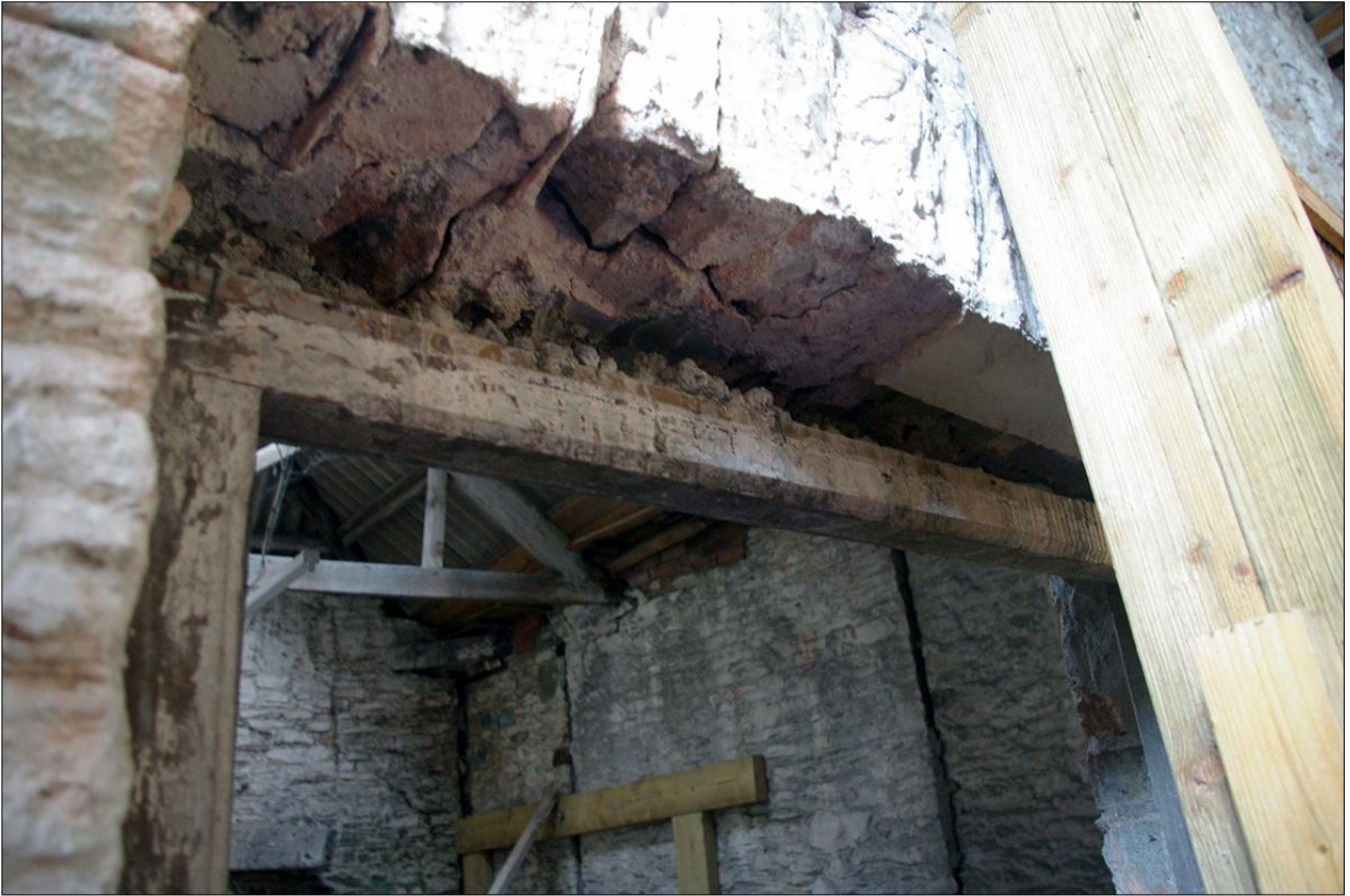
72. B1 FF R1, DETAIL OF THE CHAMFERED DOORFRAME TO D19; VIEWED FROM THE SOUTH-WEST.
