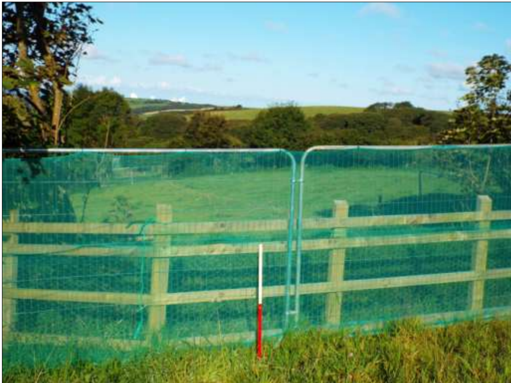
22. Detail of the blocked former entrance into the site in the west site boundary; viewed from the east (1m scale).
