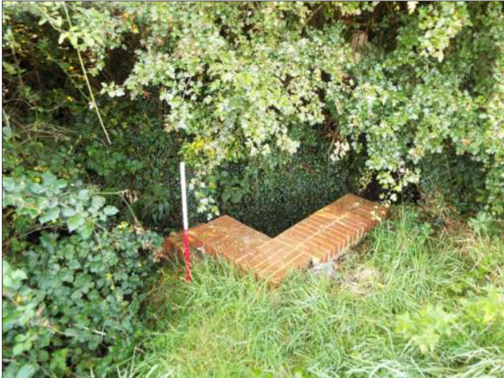
15. Detail of the south-west corner of the site showing the modern brick wall associated with the drainage system which drains into the ditch at the southern site boundary; viewed from the north-north-east (1m scale).
