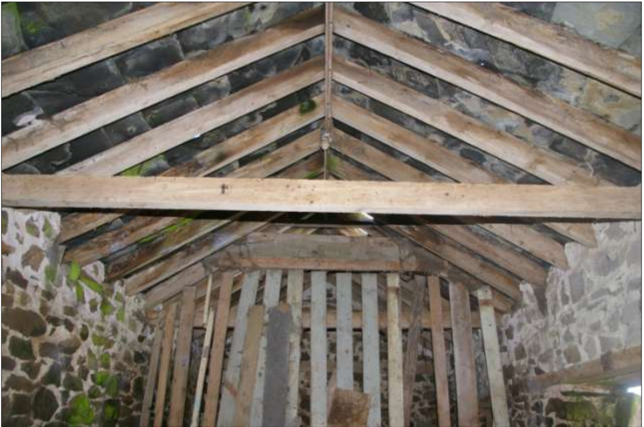
THE ROOF IN THE PIGSTY (BARN 2); FROM THE WEST.
