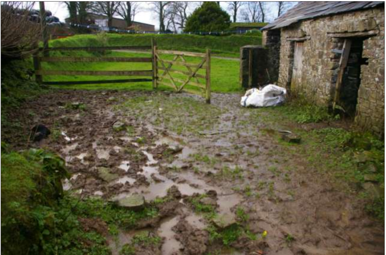
THE YARD TO THE SOUTH OF THE PIGSTY (BARN 2), SHOWING MUD OVER REMAINING COBBLES; FROM THE EAST.
