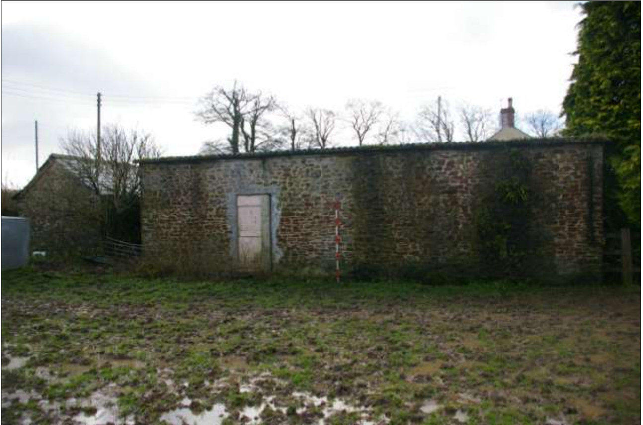
THE EAST ELEVATION OF BARN 1; VIEWED FROM THE EAST-NORTH-EAST (SCALE 2M).
