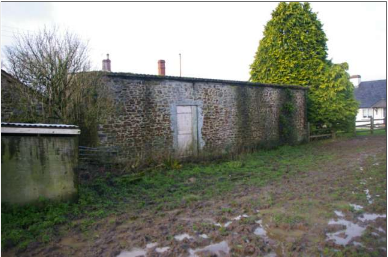
THE EAST ELEVATION OF BARN 1; VIEWED FROM THE SOUTH-EAST.
