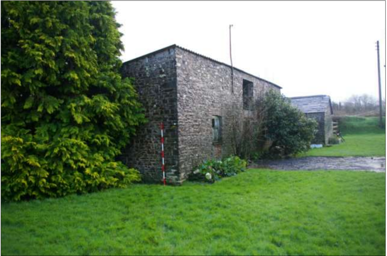
THE NORTH AND WEST ELEVATIONS OF BARN 1; VIEWED FROM THE NORTH-WEST (SCALE 2M).
