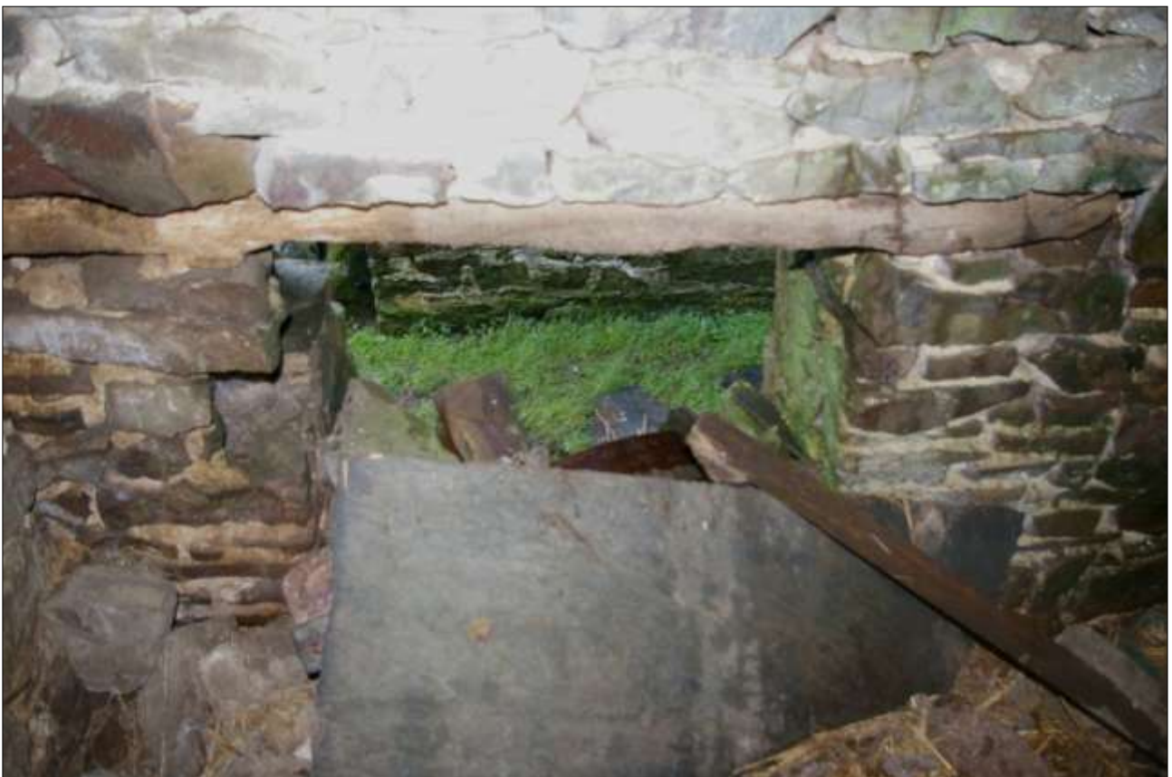
ONE OF THE SMALL FEED HATCHES IN THE NORTH WALL OF THE PIGSTY (BARN 2); FROM THE SOUTH.
