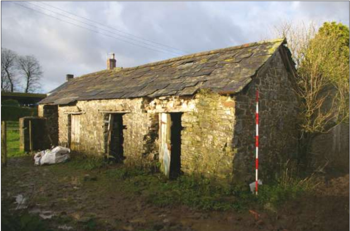
FIGURE 8: BARN 2, VIEWED FROM THE SOUTH-EAST (SCALE 2M).
