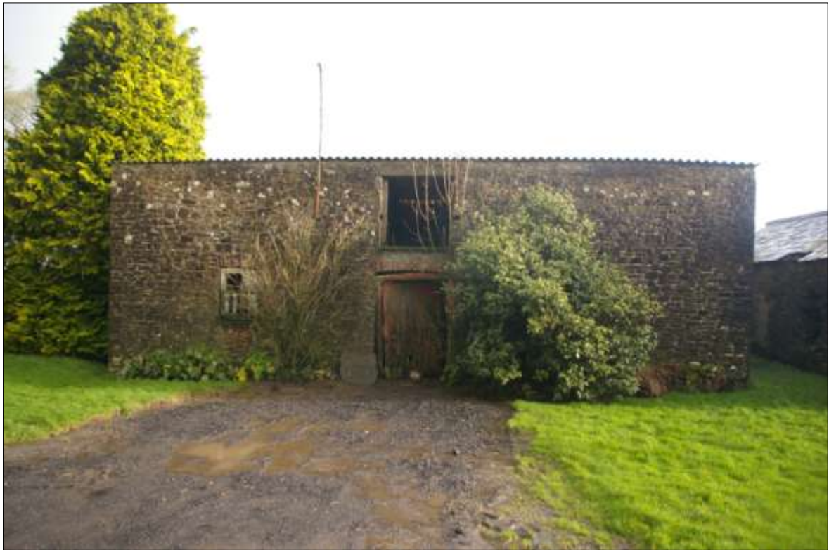
FIGURE 7: BARN 1, VIEWED FROM THE WEST.
