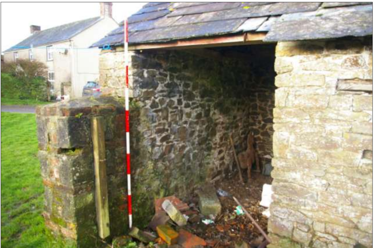
THE BRICK AND CONCRETE BLOCK PIER ADDED TO THE WEST GABLE END WALL OF THE PIGSTY (BARN 2), WITH 2M SCALE; FROM THE SOUTH-EAST.
