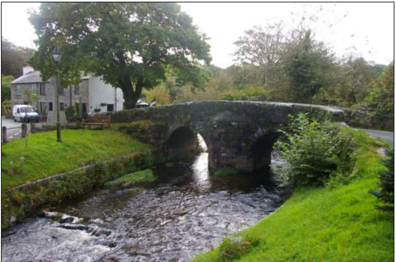
PHOTOGRAPH 14: VIEW OF THE ALTARNUN BRIDGE; TAKEN FACING SOUTH.
