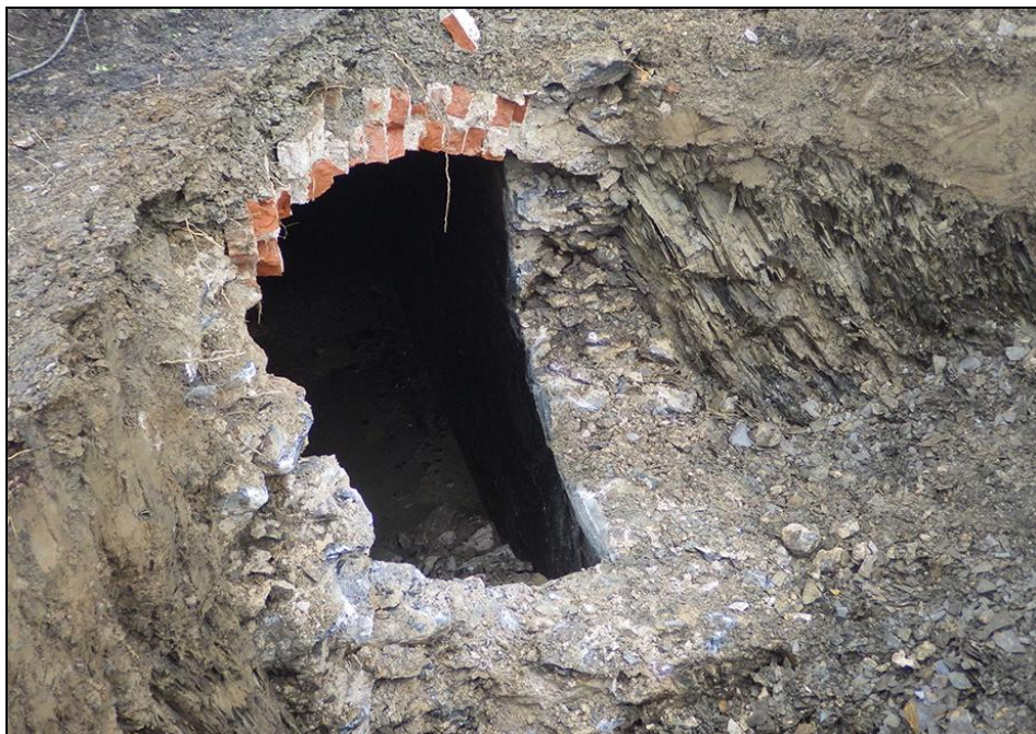
FIGURE 4: VICTORIAN TANK, PARTIAL DEMOLITION; VIEWED FROM THE WEST (NO SCALE).
