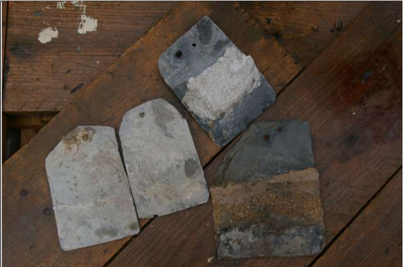
PEG SLATES, SHOWING TWO HOLES, INDICATING AT LEAST ONE REUSE, WITH LIME TORCHING REMOVED FROM THE NAVE AND NORTH AISLE ROOFS, ONE WITH INTACT OAK PEG.
