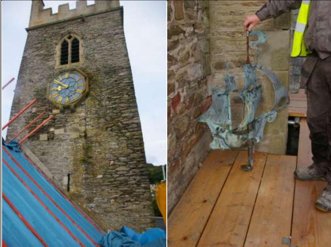
LEFT: DETAILED VIEW OF THE TOWER, SHOWING THE EAST SIDE AND BLOCKED OPENINGS, INDICATING PHASING, ALSO SHOWING ODD ANGLE OF ROOFLINE WHERE ATTACHED TO TOWER; FROM THE EAST, NORTH-EAST.
