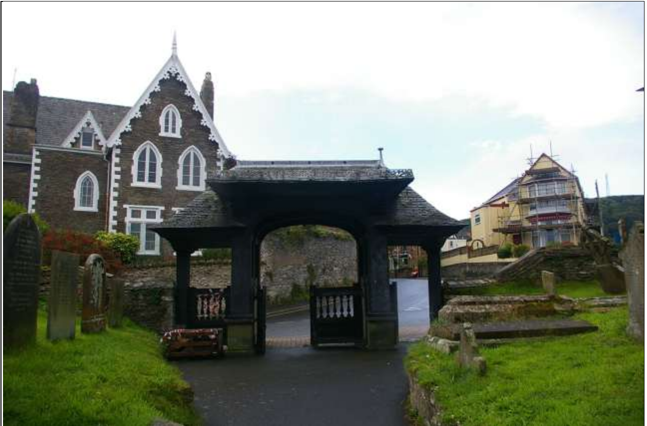
ELABORATE LYCH GATE WITH SCANTLE SLATE ROOF AND PEGGED TIMBER FRAME, DATED 1836; FROM THE NORTH-WEST.
