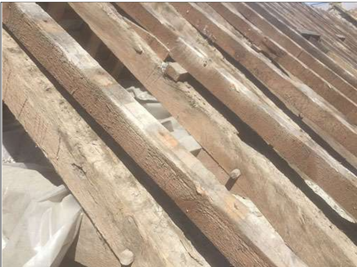
CARPENTERS NUMBERING MARKS ON THE SOUTH AISLE TRUSSES.
