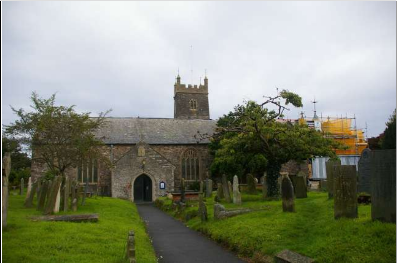
VIEW OF THE CHURCH, FROM THE LYCHGATE, SHOWING SOUTH PORCH, SOUTH AISLE AND THE LARGE 19 TH CENTURY REPLACEMENT PERPENDICULAR STYLE STONE WINDOWS; FROM THE SOUTH-WEST.
