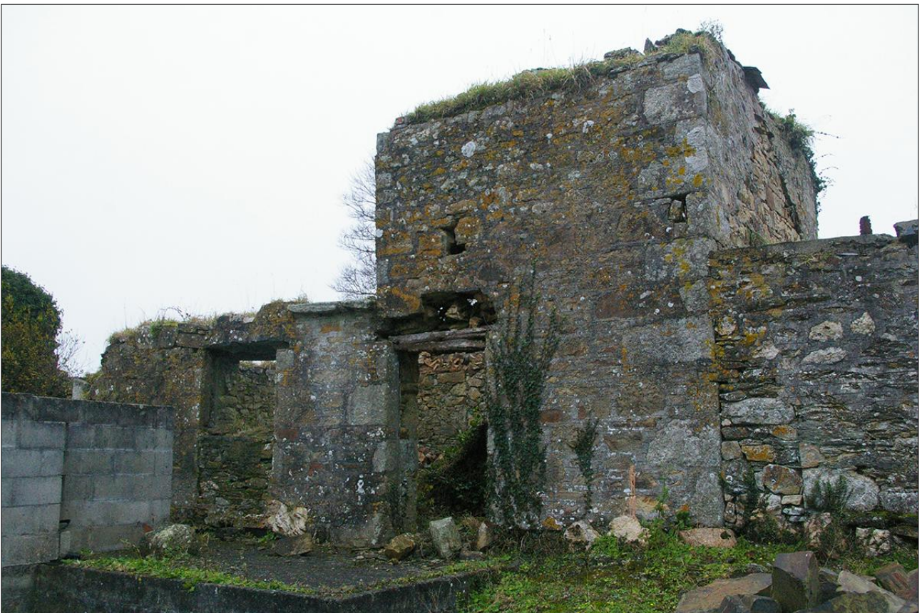
THE SOUTH-WEST ELEVATION OF B4B; VIEWED FROM THE SOUTH.
