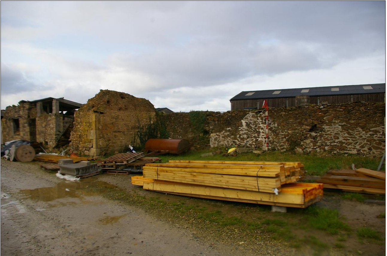
B1 & B2; VIEWED FROM THE SOUTH-EAST (SCALE 2M).
