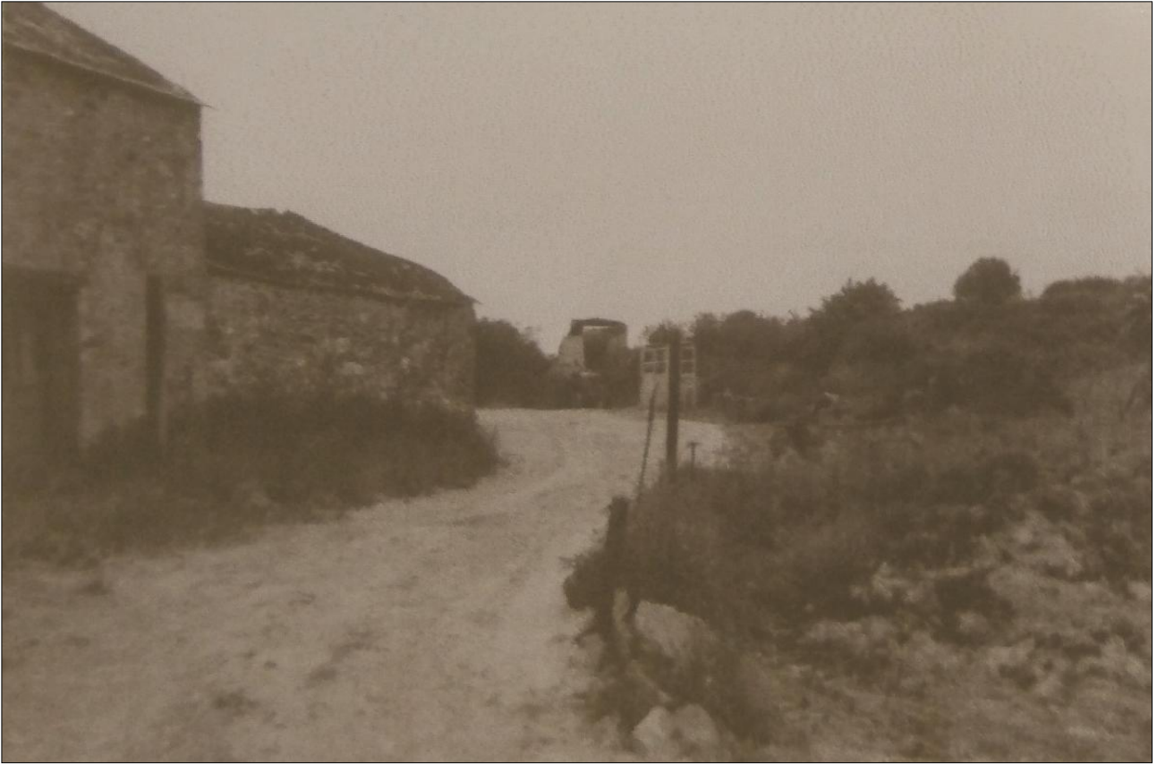
THE SOUTH ELEVATION OF B4B AND B4C, VIEWED FROM THE WEST.
