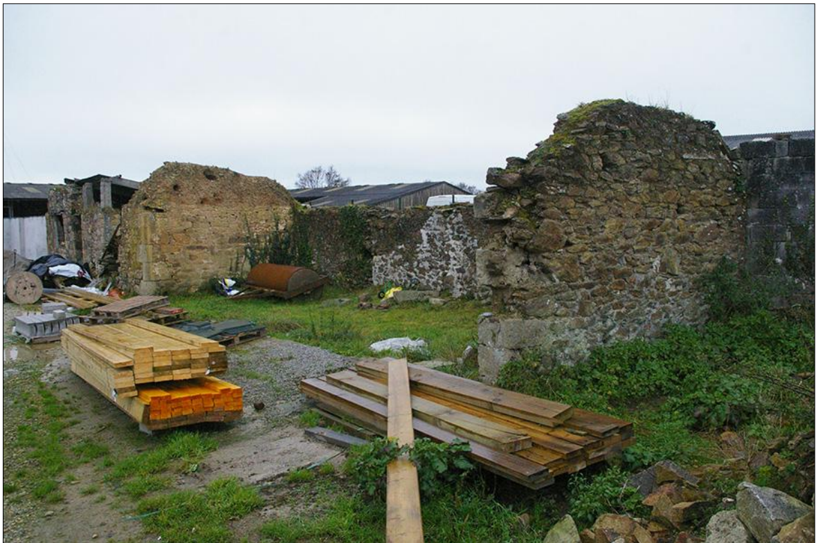
FIGURE 13: B2, VIEWED FROM THE SOUTH-EAST.
