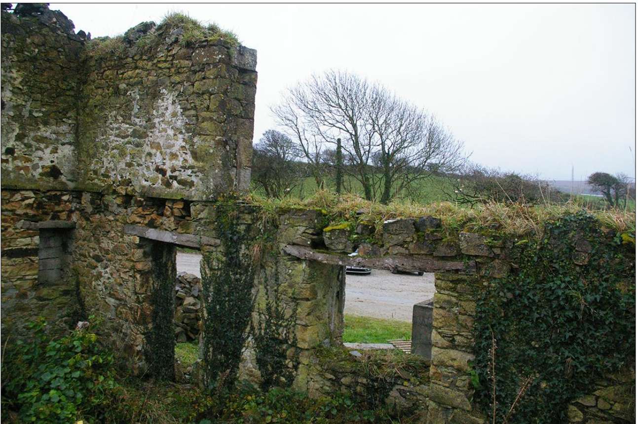
THE INTERIOR OF B4B (SOUTH-WEST CORNER) SHOWING THE OPENINGS; VIEWED FROM THE NORTH.
