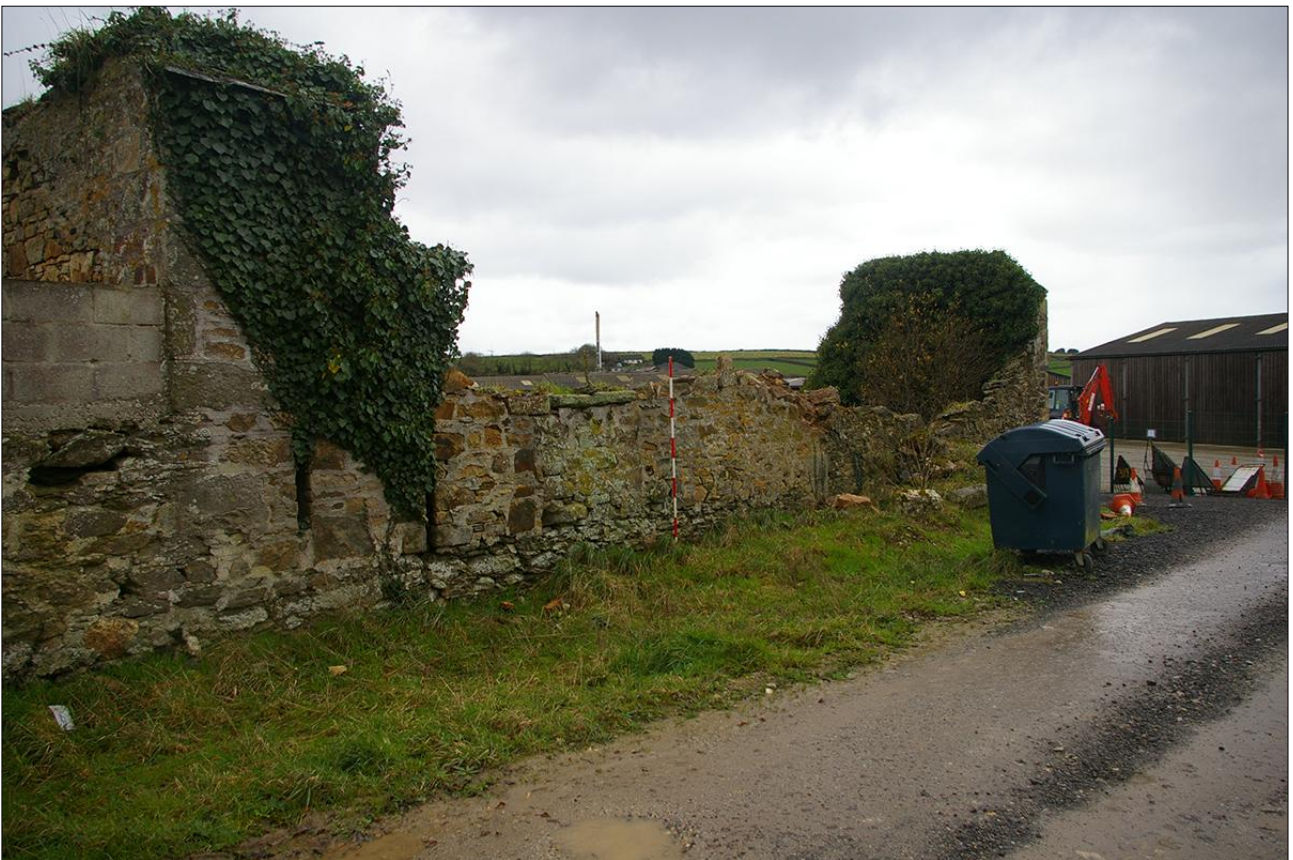
THE NORTH-EAST ELEVATION OF B4B; VIEWED FROM THE EAST (SCALE 2M).
