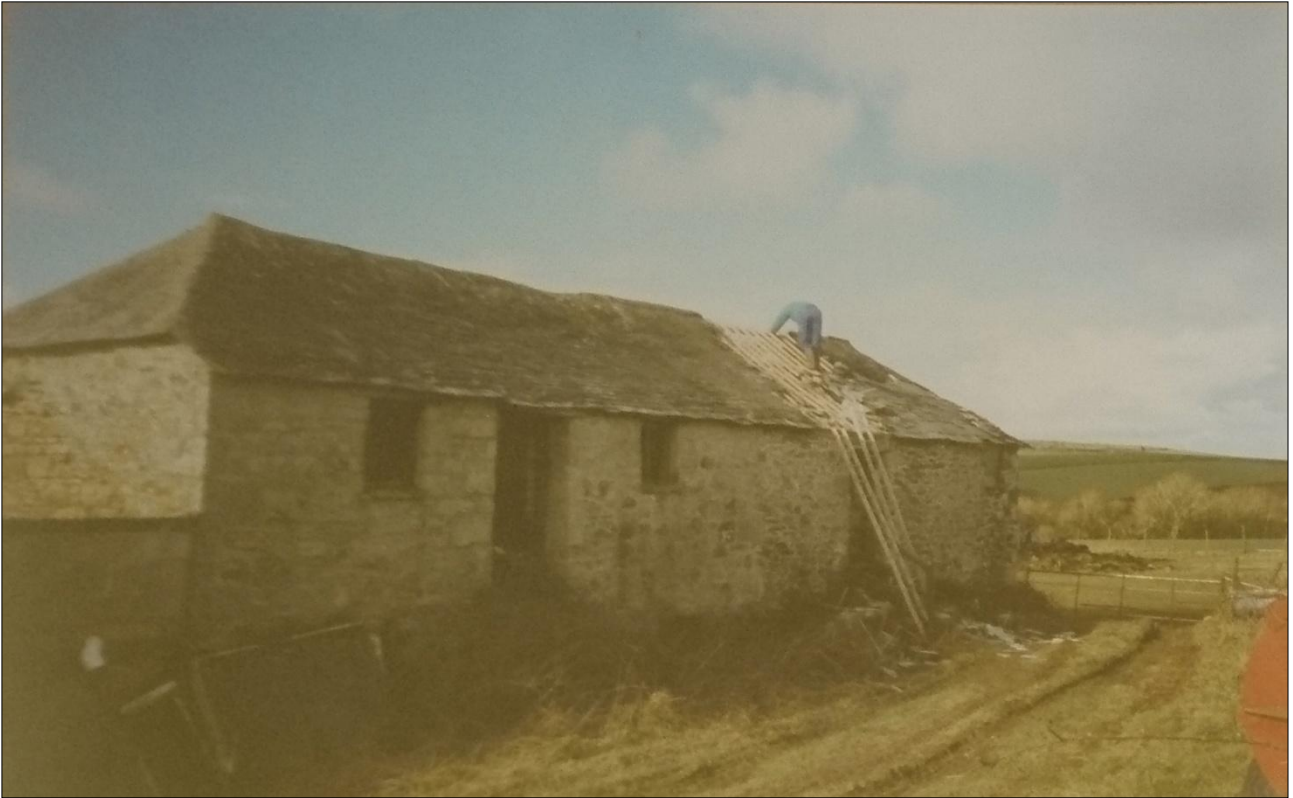
THE REAR (NORTH-EAST) ELEVATION OF B4, VIEWED FROM THE EAST.
