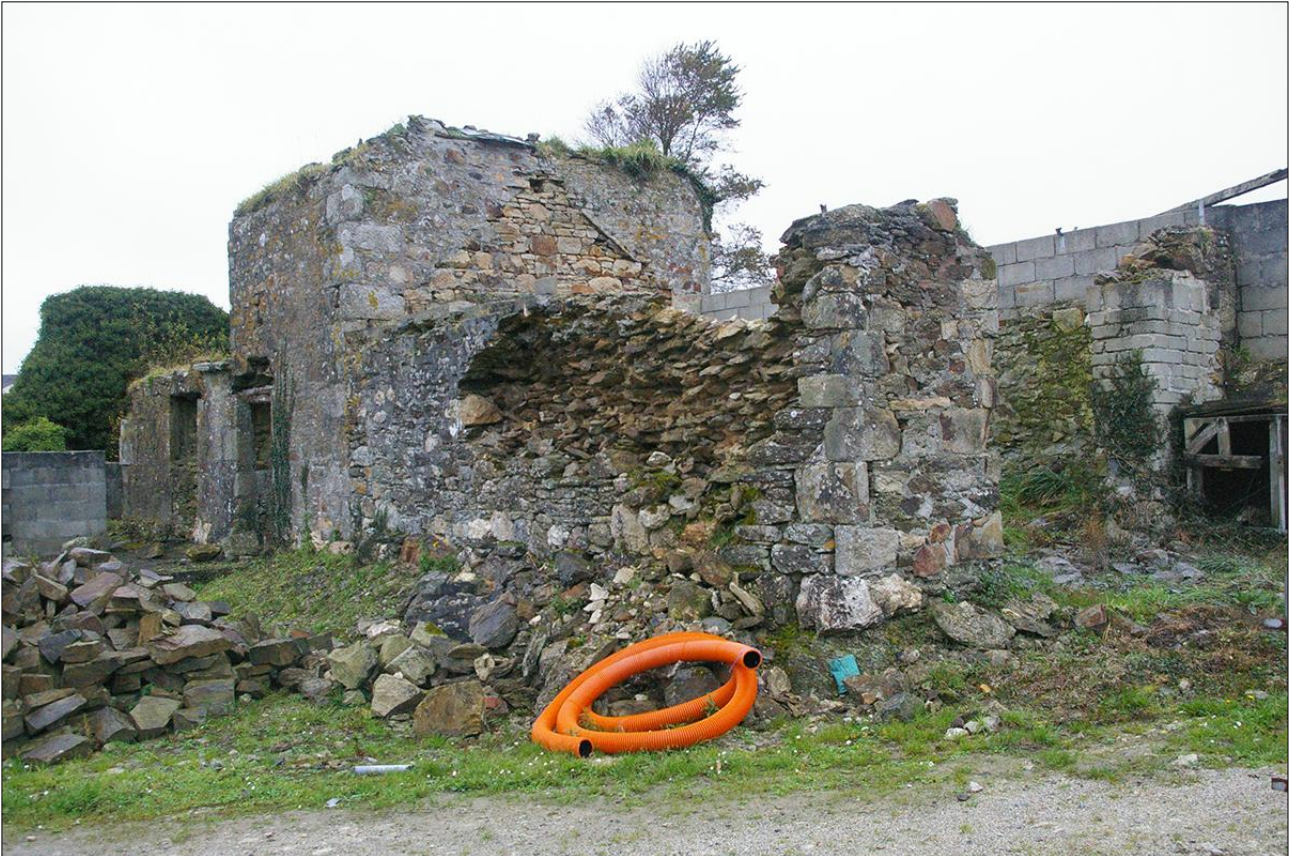
THE SOUTH-WEST ELEVATION OF B4C; VIEWED FROM THE SOUTH.
