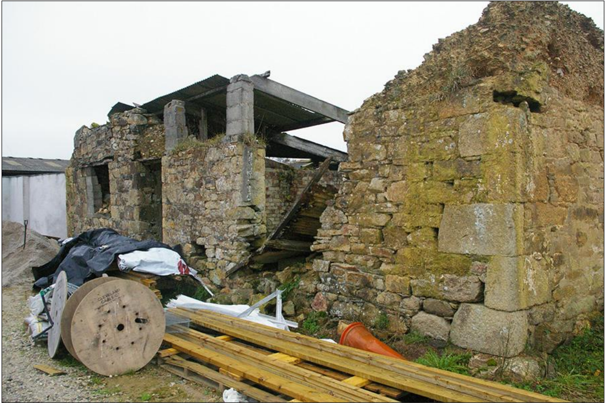
FIGURE 11: THE SOUTH ELEVATION OF B1; VIEWED FROM THE SOUTH-EAST.
