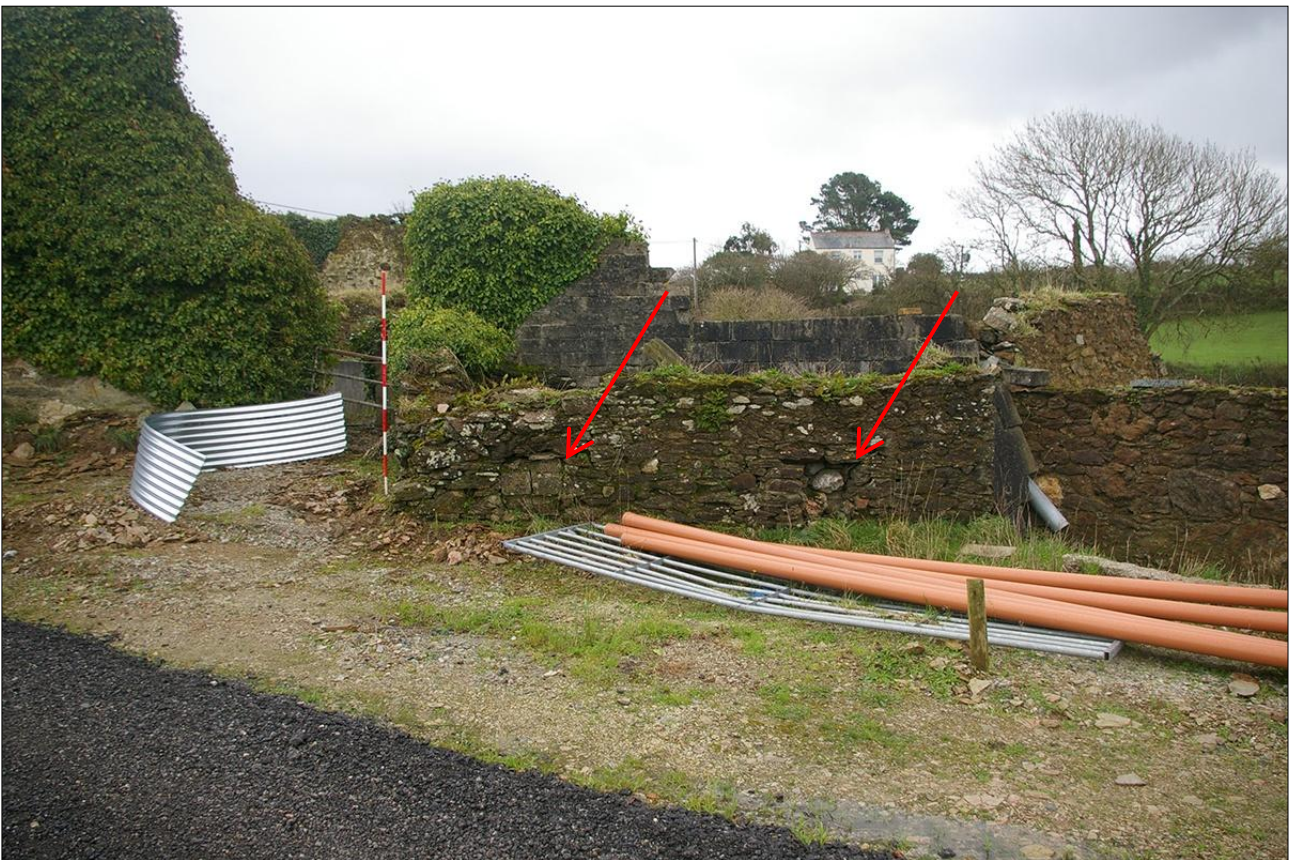
THE NORTH-WEST ELEVATION OF B3, WITH FEEDING HATCHES INDICATED; VIEWED FROM THE NORTH-WEST (SCALE 2M).
