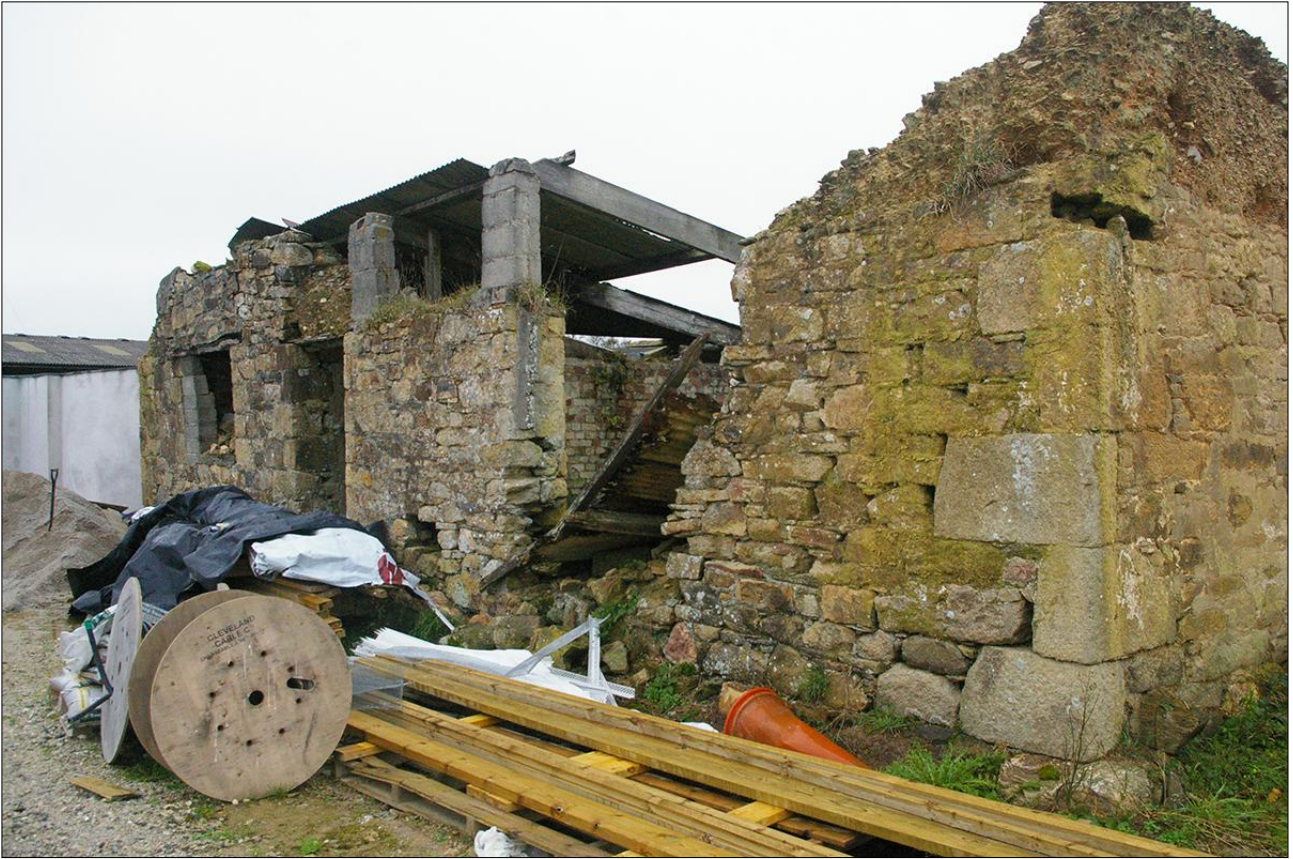
THE SOUTH ELEVATION OF B1; VIEWED FROM THE SOUTH-EAST.
