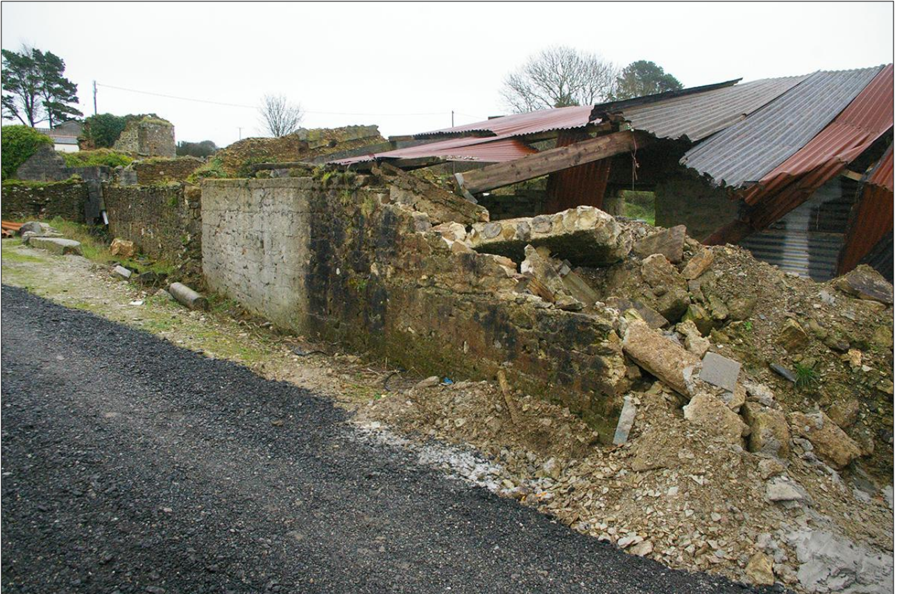
THE SHUTTERED CONCRETE NORTH WALL OF B1; VIEWED FROM THE NORTH-WEST.
