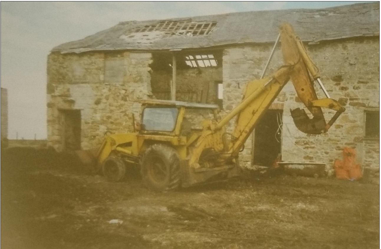
THE FRONT (SOUTH-WEST) ELEVATION OF B4A, VIEWED FROM THE SOUTH-WEST.
