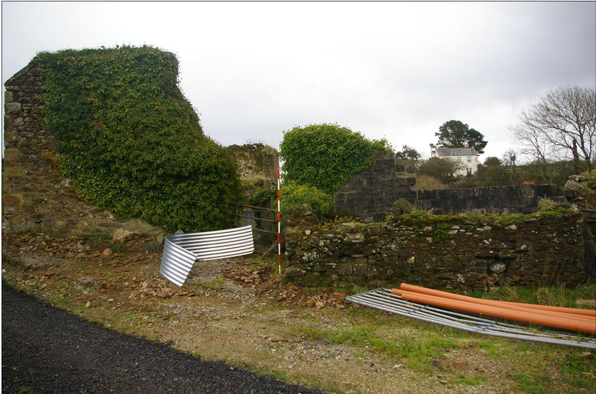
FIGURE 14: B3, VIEWED FROM THE NORTH (SCALE 2M).
