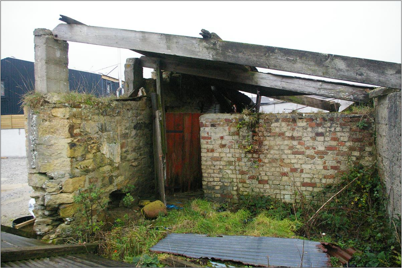
B1, EAST CELL AND DIVIDING WALL; VIEWED FROM THE EAST.
