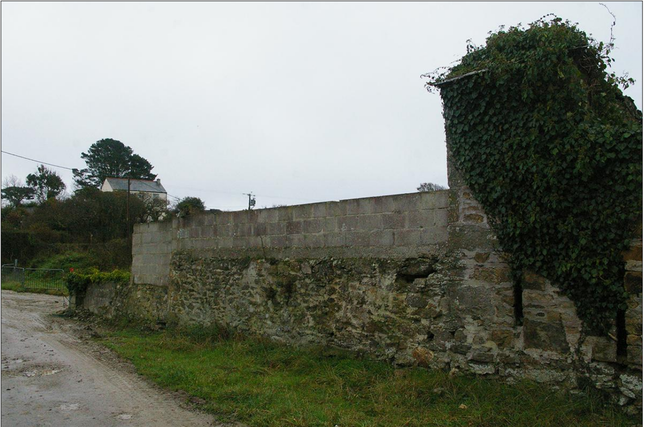
THE NORTH-EAST ELEVATION OF B4C; VIEWED FROM THE NORTH.
