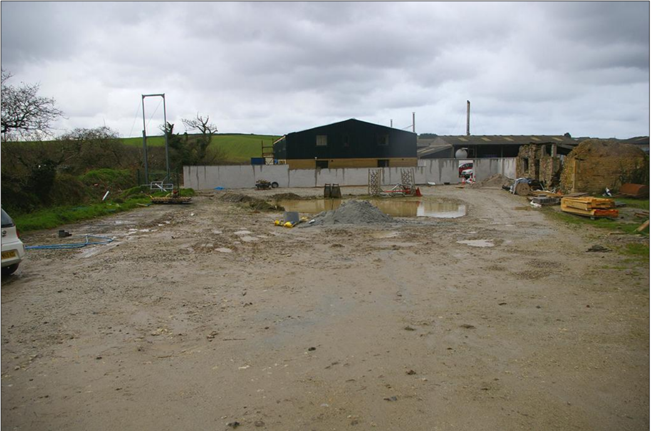
THE FORMER HISTORIC YARD AREA; VIEWED FROM THE EAST.
