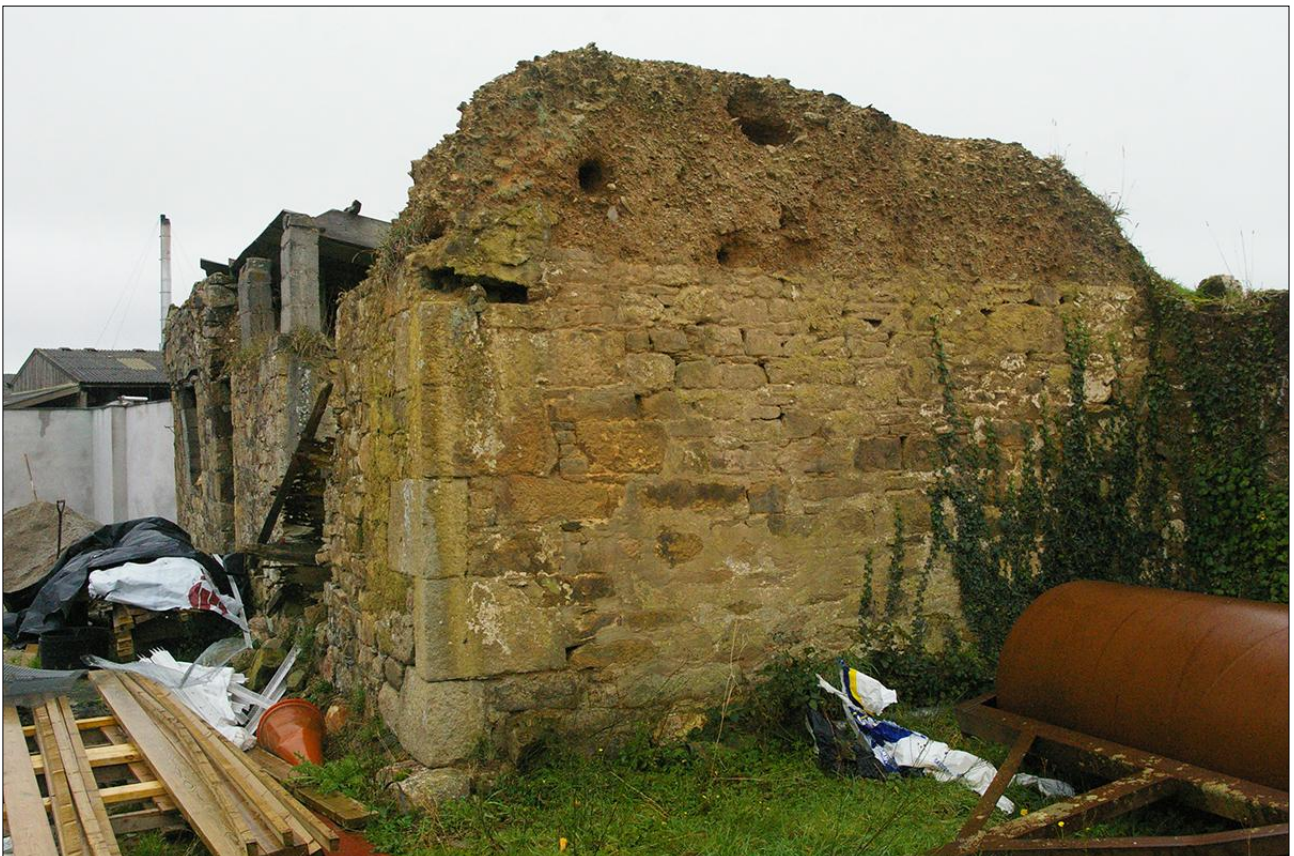
THE EAST GABLE OF B1; VIEWED FROM THE SOUTH-EAST.
