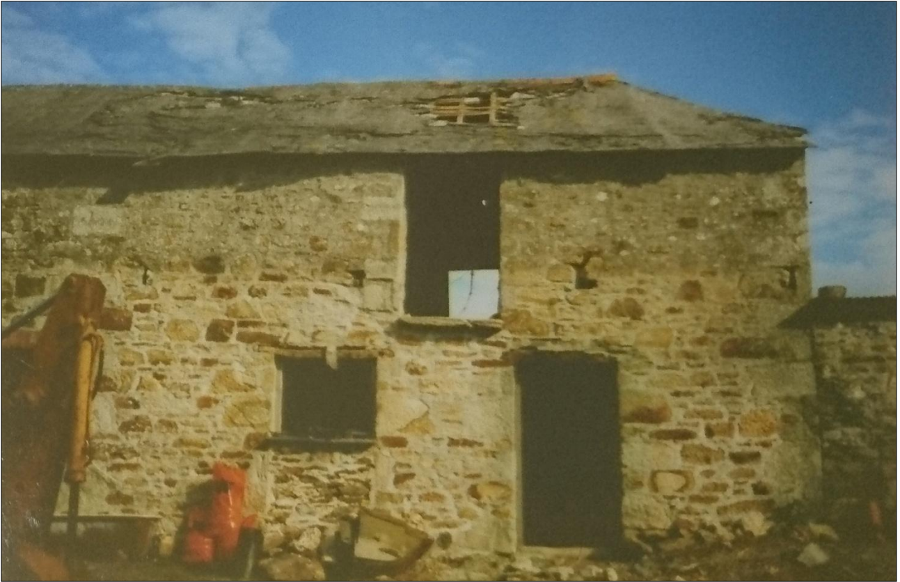
THE FRONT (SOUTH-WEST) ELEVATION OF B4B, VIEWED FROM THE SOUTH-WEST.
