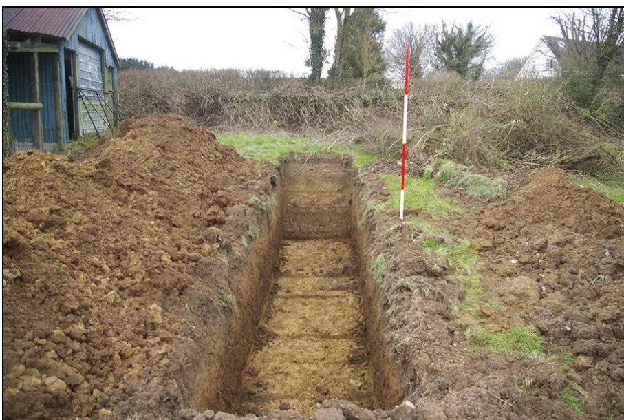
FIGURE 5: TRENCH 6; VIEWED FROM THE EAST (2M SCALE).
