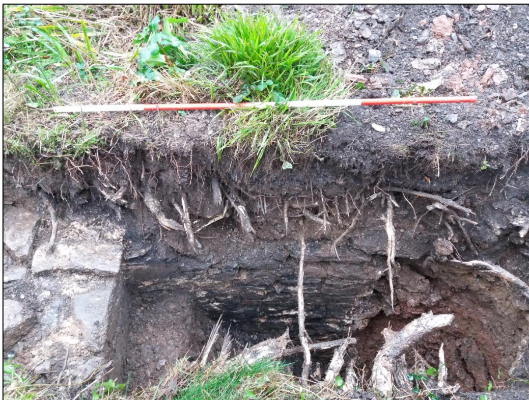
TEST-PIT 04, DETAIL OF WALL {405} NORTH-WEST FACING ELEVATION; VIEWED FROM THE NORTH-WEST (2M SCALE).
