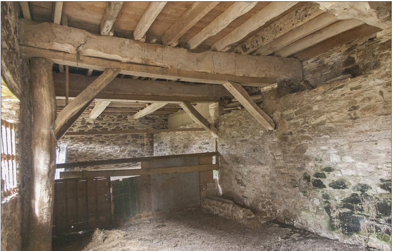
THE GROUND-FLOOR INTERIOR OF B2.1; VIEWED FROM THE SOUTH.
