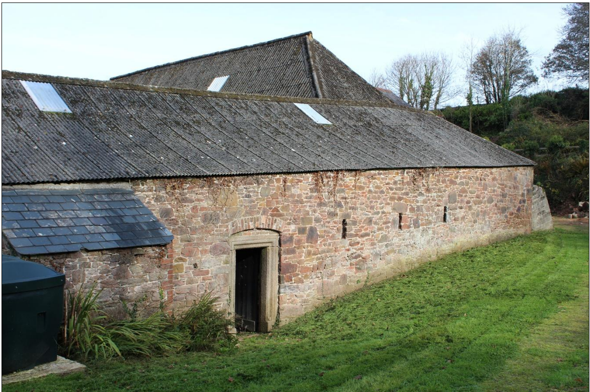
FIGURE 19: THE REAR (SOUTH) ELEVATION OF B1.1; VIEWED FROM THE SOUTH-WEST.
