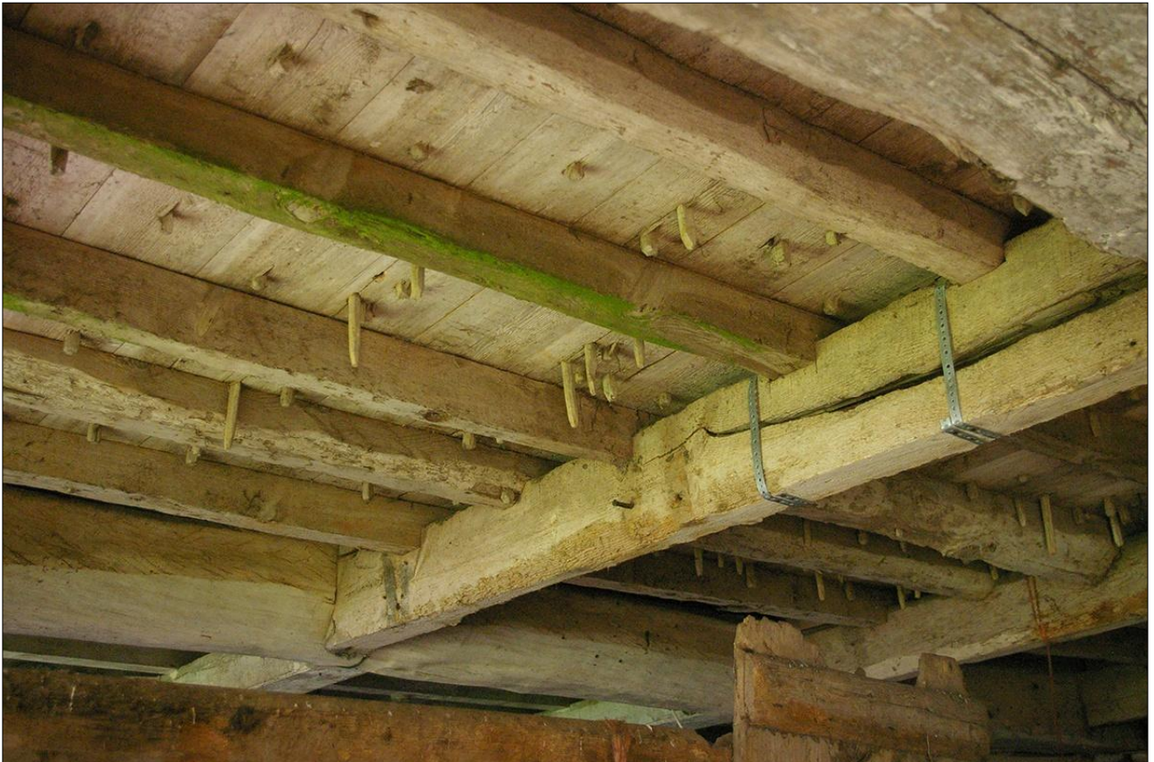
THE MANY TRUNNELS IN THE FLOOR BENEATH THE SOUTH THRESHING DOORS IN B5; VIEWED FROM THE NORTH-EAST.
