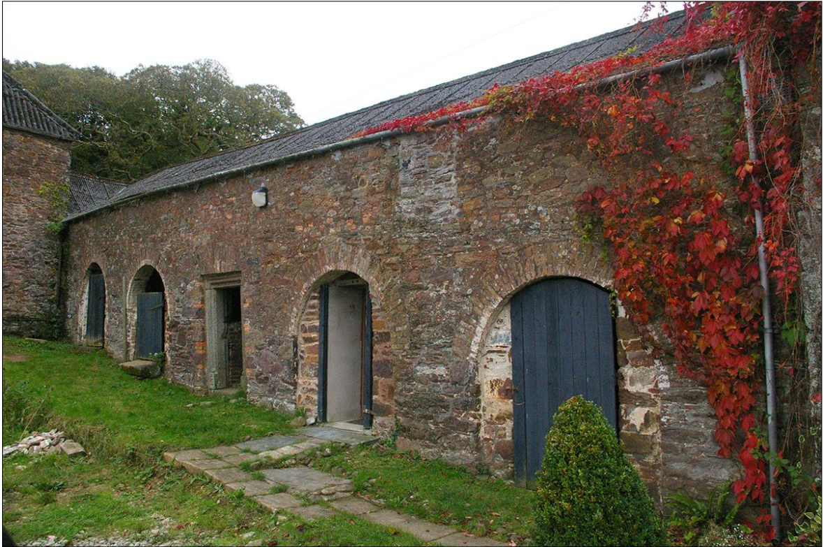
FIGURE 18: THE FRONT (NORTH) ELEVATION OF B1.1; VIEWED FROM THE NORTH-WEST.
