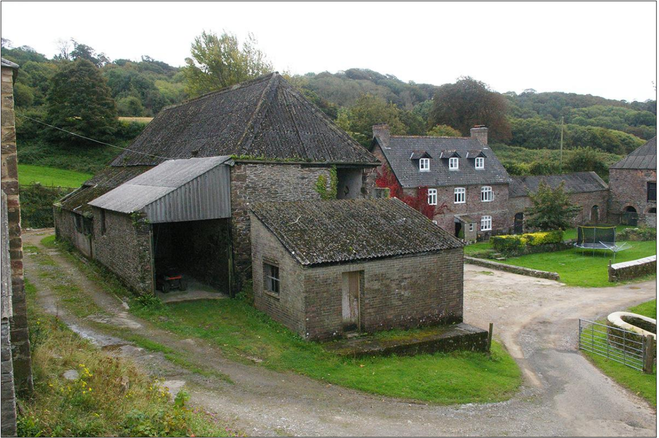
THE EAST AND NORTH ELEVATIONS OF B1.3, B1.4 AND B1.5, WITH B3 AND B4 IN THE BACKGROUND; VIEWED FROM THE NNE.
