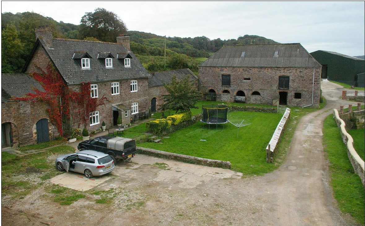
FIGURE 30: THE CENTRAL YARD FROM THE TOP OF THE EXTERNAL STAIRS TO B1.3; VIEWED FROM THE NORTH-EAST.
