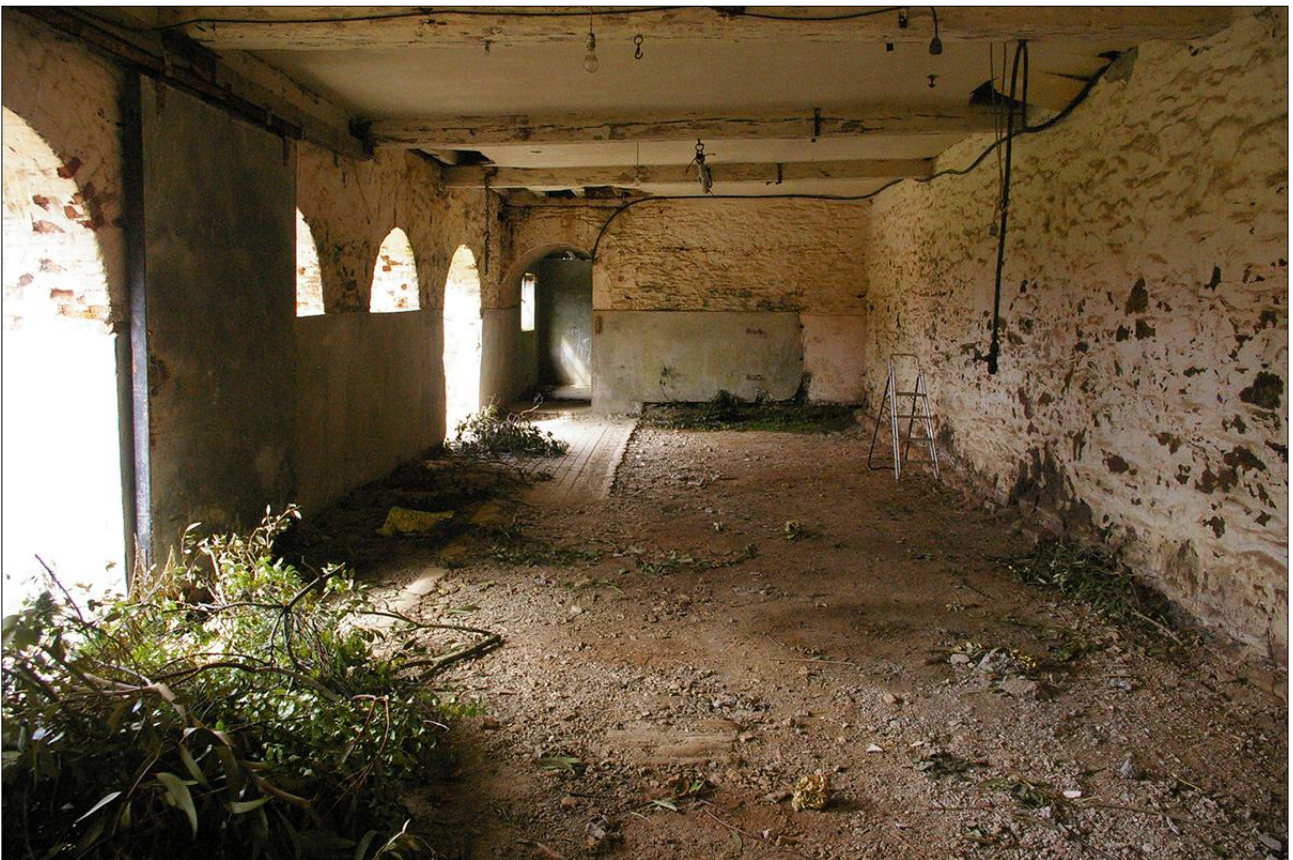
THE GROUND-FLOOR INTERIOR OF B1.3; VIEWED FROM THE SOUTH.
