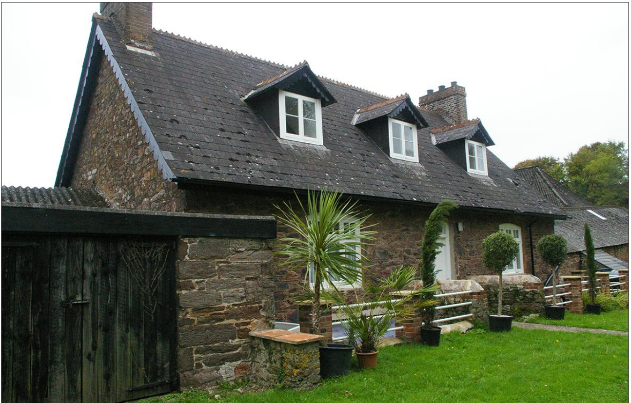
THE REAR (SOUTH) ELEVATION OF B3, WITH SHED ABUTTING B4 TO THE LEFT; VIEWED FROM THE SOUTH-WEST.
