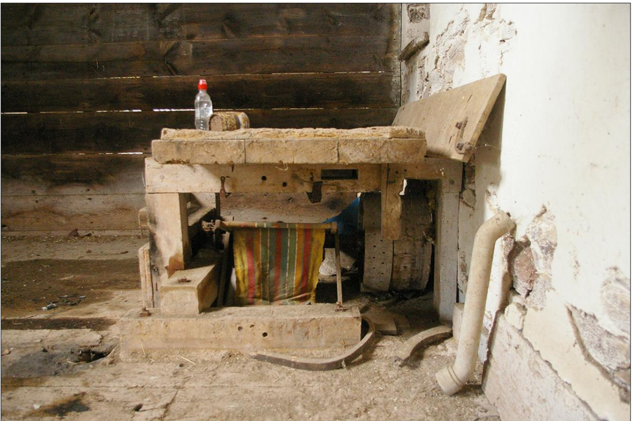
THE FLYWHEEL AT FIRST-FLOOR LEVEL IN B1.3, WITH SCREEN BEHIND; VIEWED FROM THE SOUTH.
