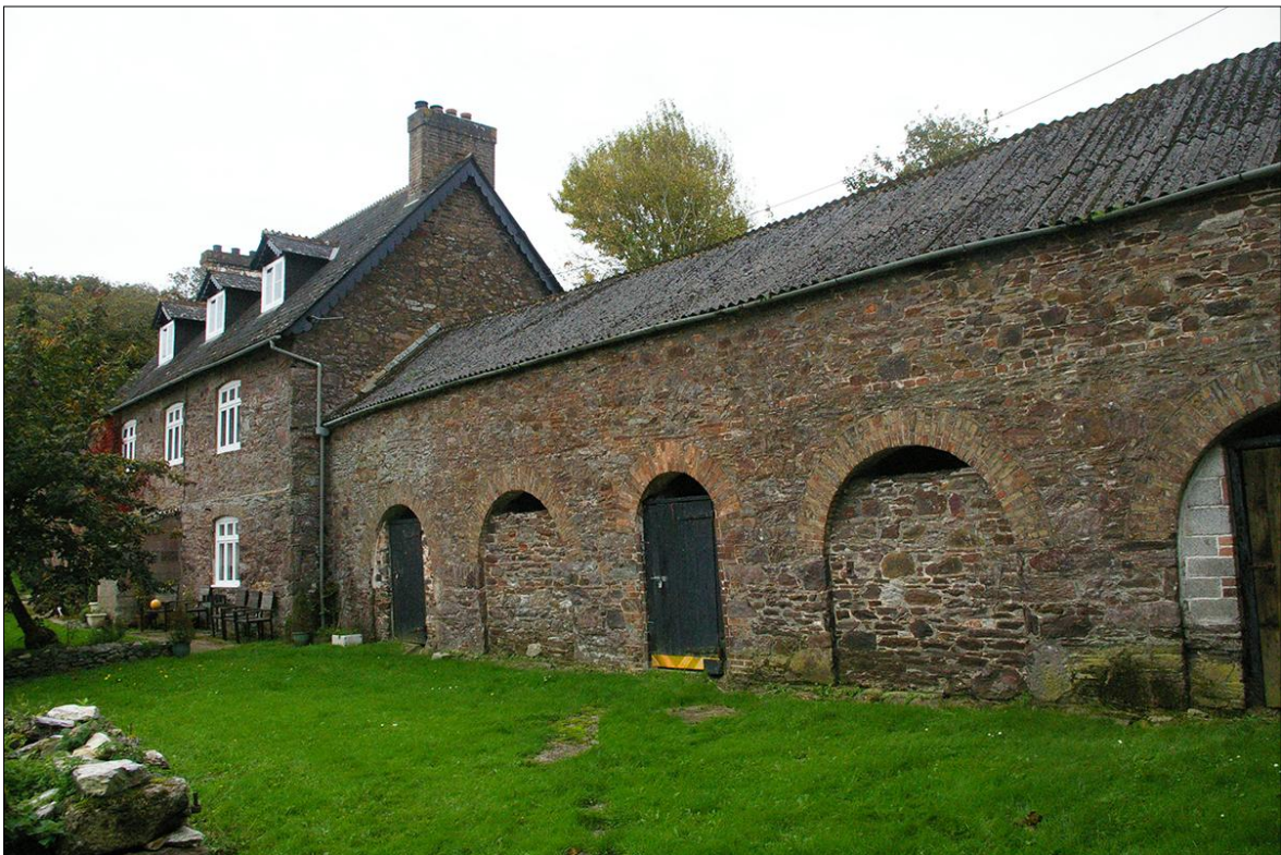
FIGURE 28: THE FRONT (NORTH) ELEVATION OF B4; VIEWED FROM THE NORTH-WEST.
