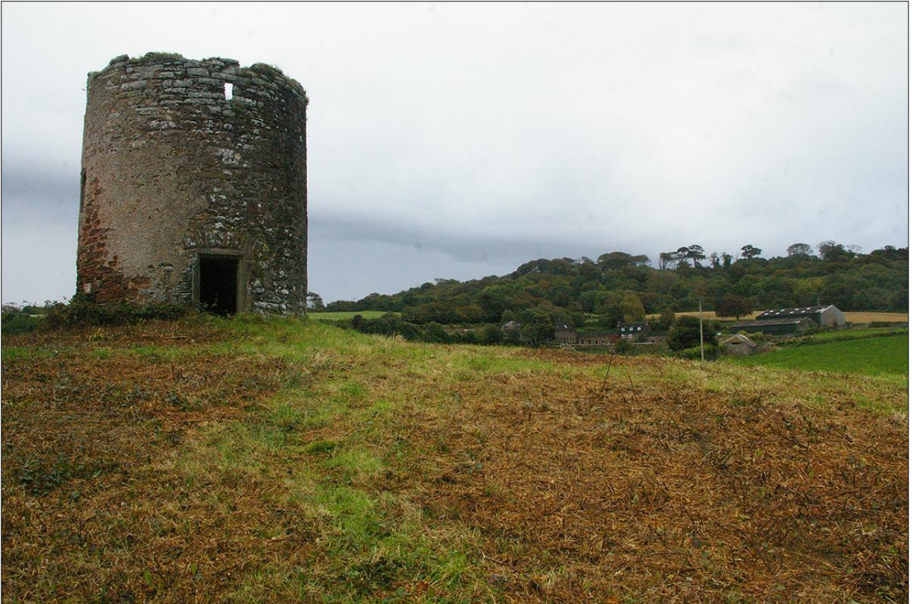
THE RUINED WINDMILL TOWER WITH THE FARM IN THE BACKGROUND; VIEWED FROM THE NORTH-WEST. NOTE THE USE OF INSERTED GRANITE WINDOW AND DOOR FRAMES.
