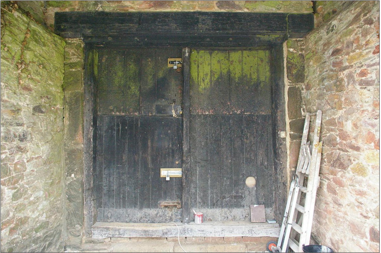
DETAIL OF THE SOUTH PORCH DOOR; VIEWED FROM THE WEST.
