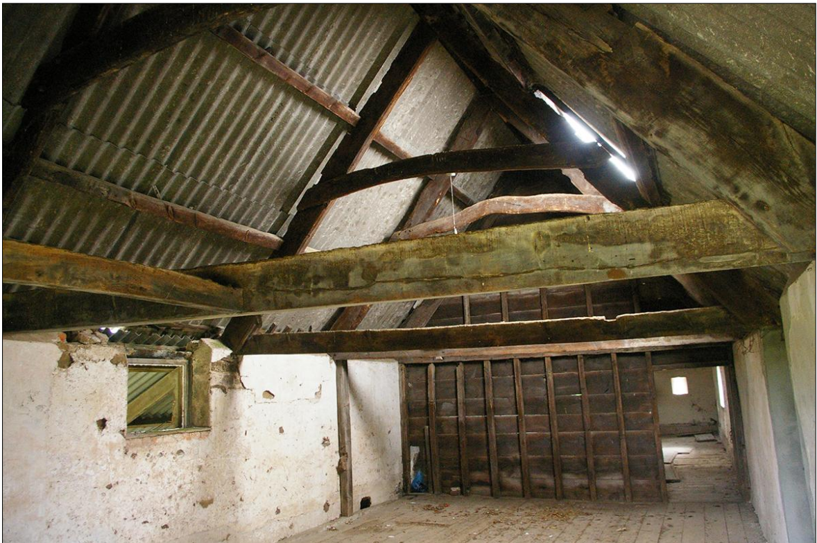
FIGURE 22: THE FIRST-FLOOR INTERIOR OF B1.3; VIEWED FROM THE NORTH.
