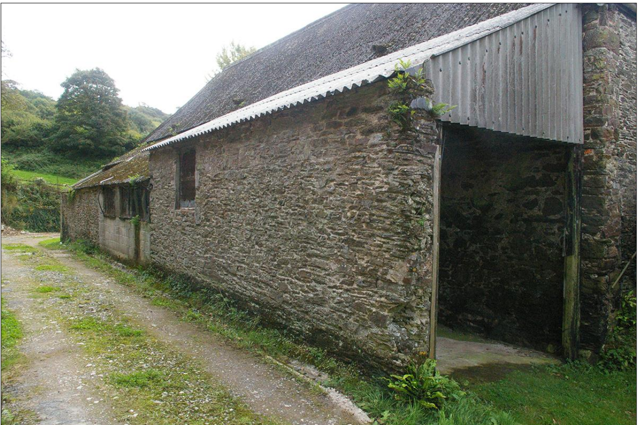
THE EAST WALL OF B1.5A; VIEWED FROM THE NORTH-EAST.
