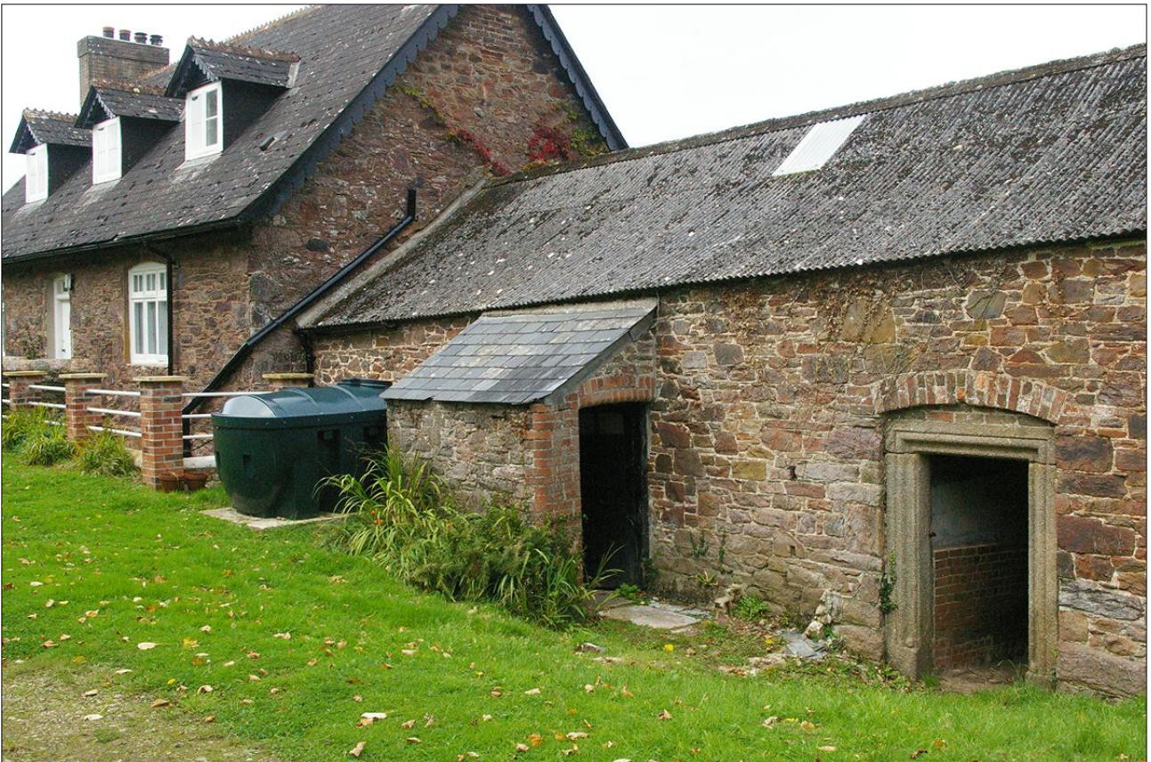
THE REAR (SOUTH) WALL AND DOORWAY OF B1.1, WITH LEAN-TO AND B3; VIEWED FROM THE SOUTH-EAST.
