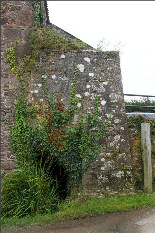
STRUCTURE ABUTTING THE NORTH-WEST WALL OF B5; VIEWED FROM THE NORTH.
