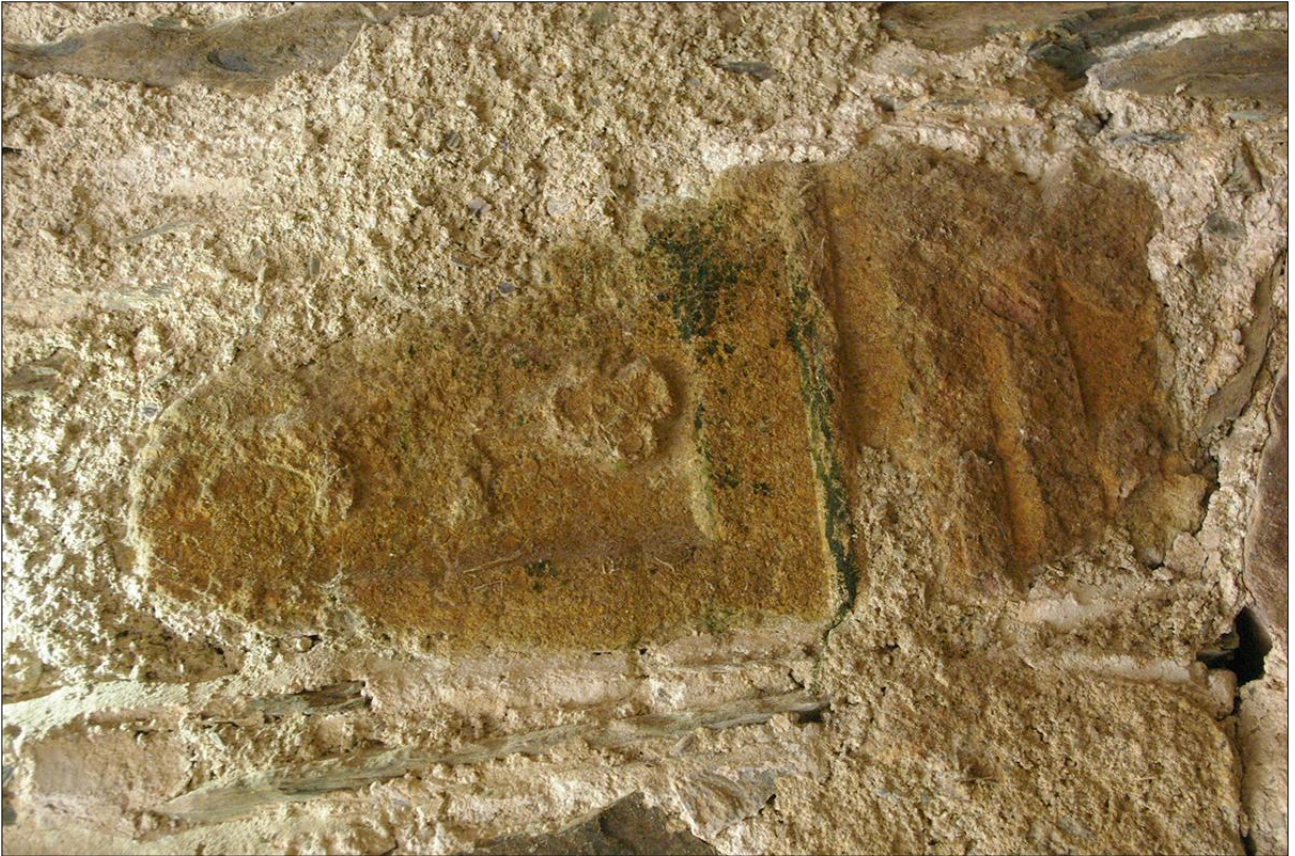
THE ARCHITECTURAL FRAGMENT BUILT INTO THE SOUTH WALL OF B2.1.
