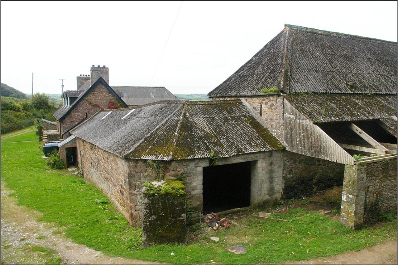
B1.1 AND B1.2 VIEWED FROM THE EAST.
