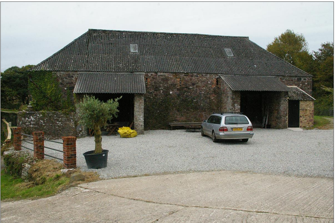
THE WEST ELEVATION OF B5, SHOWING THE TWO PORCHES; VIEWED FROM THE WEST.
