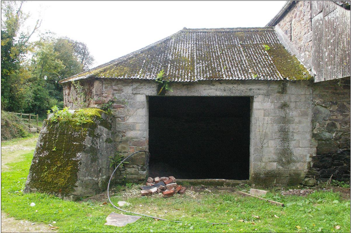
FIGURE 20: THE EAST ELEVATION OF B1.2; VIEWED FROM THE EAST.
