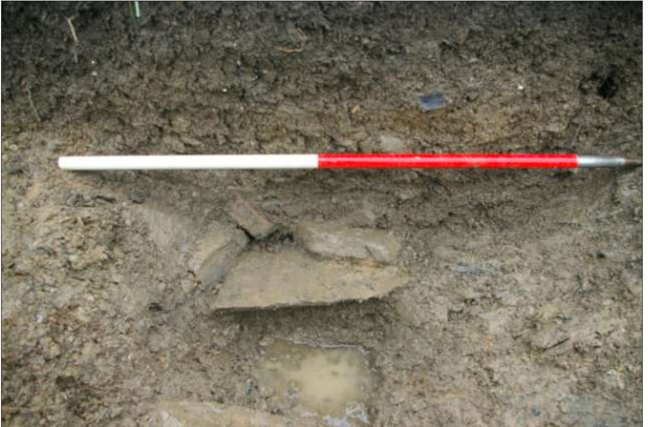
13. DRAIN [208], DETAIL OF NORTH FACING SECTION SHOWING DRAIN CONSTRUCTION AND INFILL, NOTE THE INGRESS OF WATER; VIEWED FROM THE NORTH (1M SCALE).
