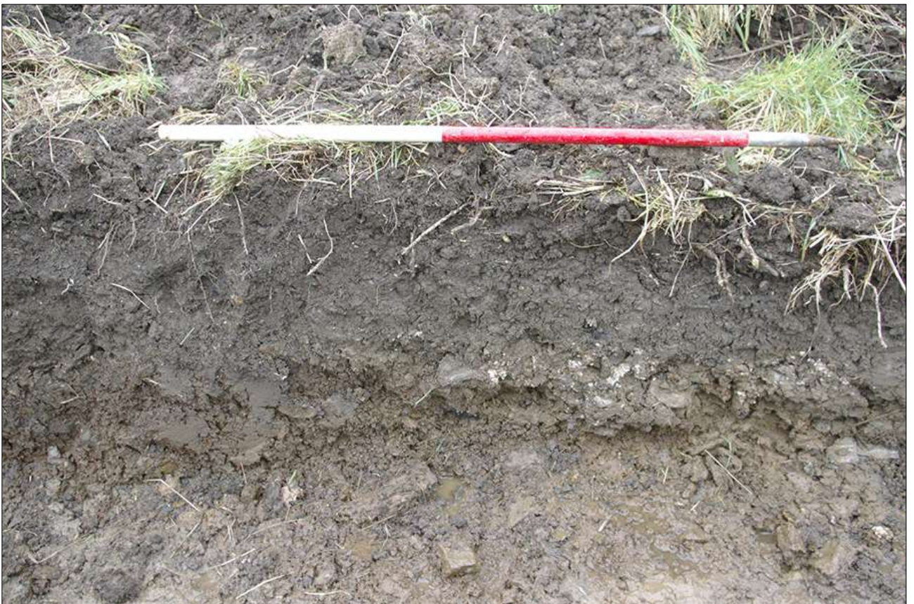
6. TRENCH 01, EAST-FACING REPRESENTATIVE SECTION, NORTH END, SHOWING SOIL LAYERS OVER MADE GROUND, WITH INGRESS OF WATER; VIEWED FROM THE EAST (1M SCALE).
