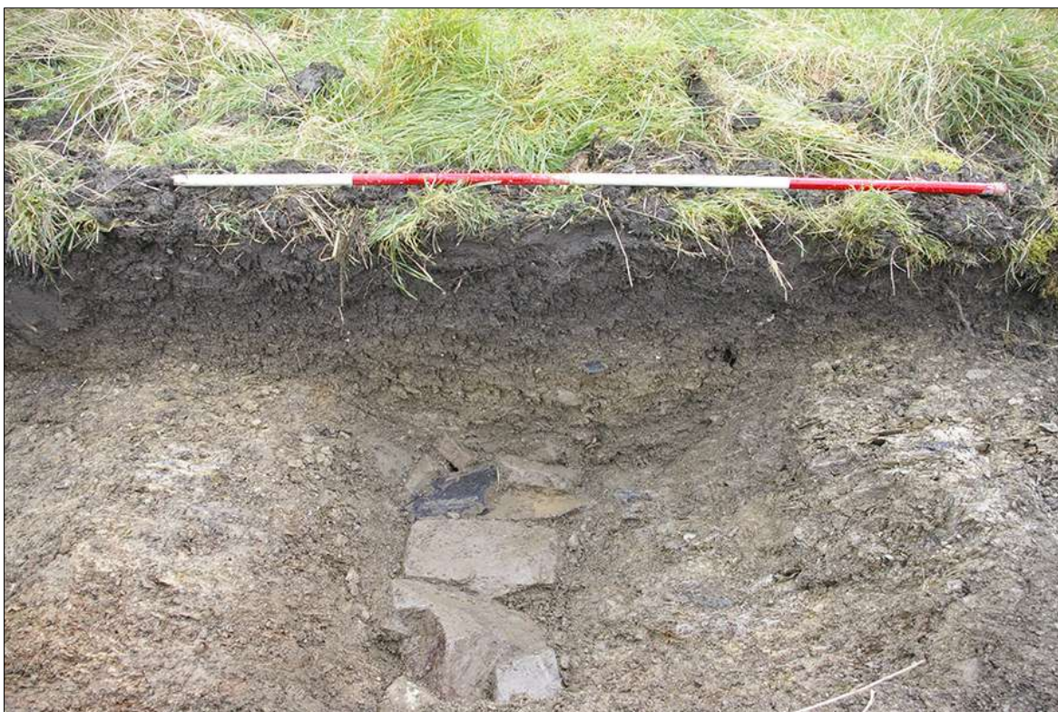
FIGURE 8: DRAIN [208], NORTH-FACING SECTION SHOWING FEATURE FILLS AND OVERLYING SOIL LAYERS; VIEWED FROM THE NORTH (2M SCALE).
