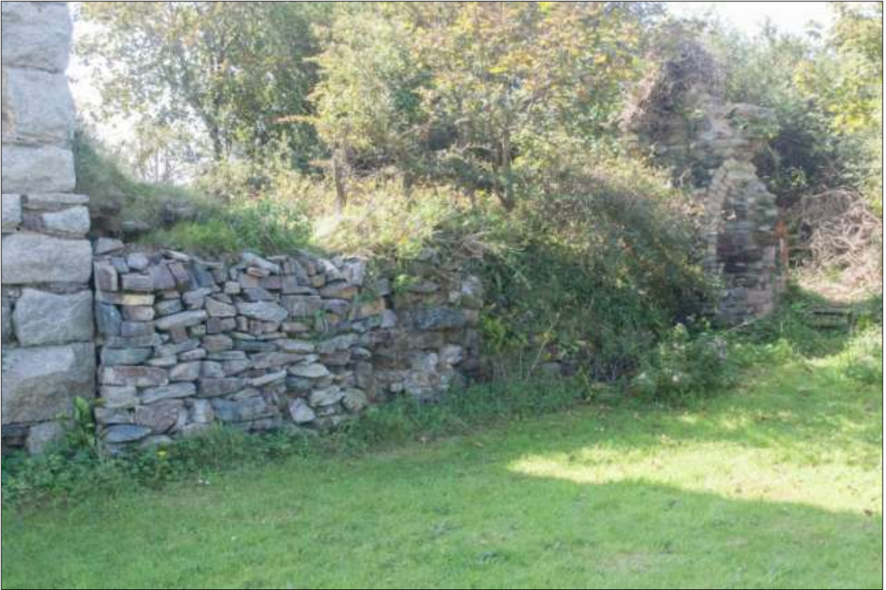
THE SURVIVING REMNANT OF THE BOILERHOUSE WALL; VIEWED FROM THE NORTH-NORTH-WEST.
