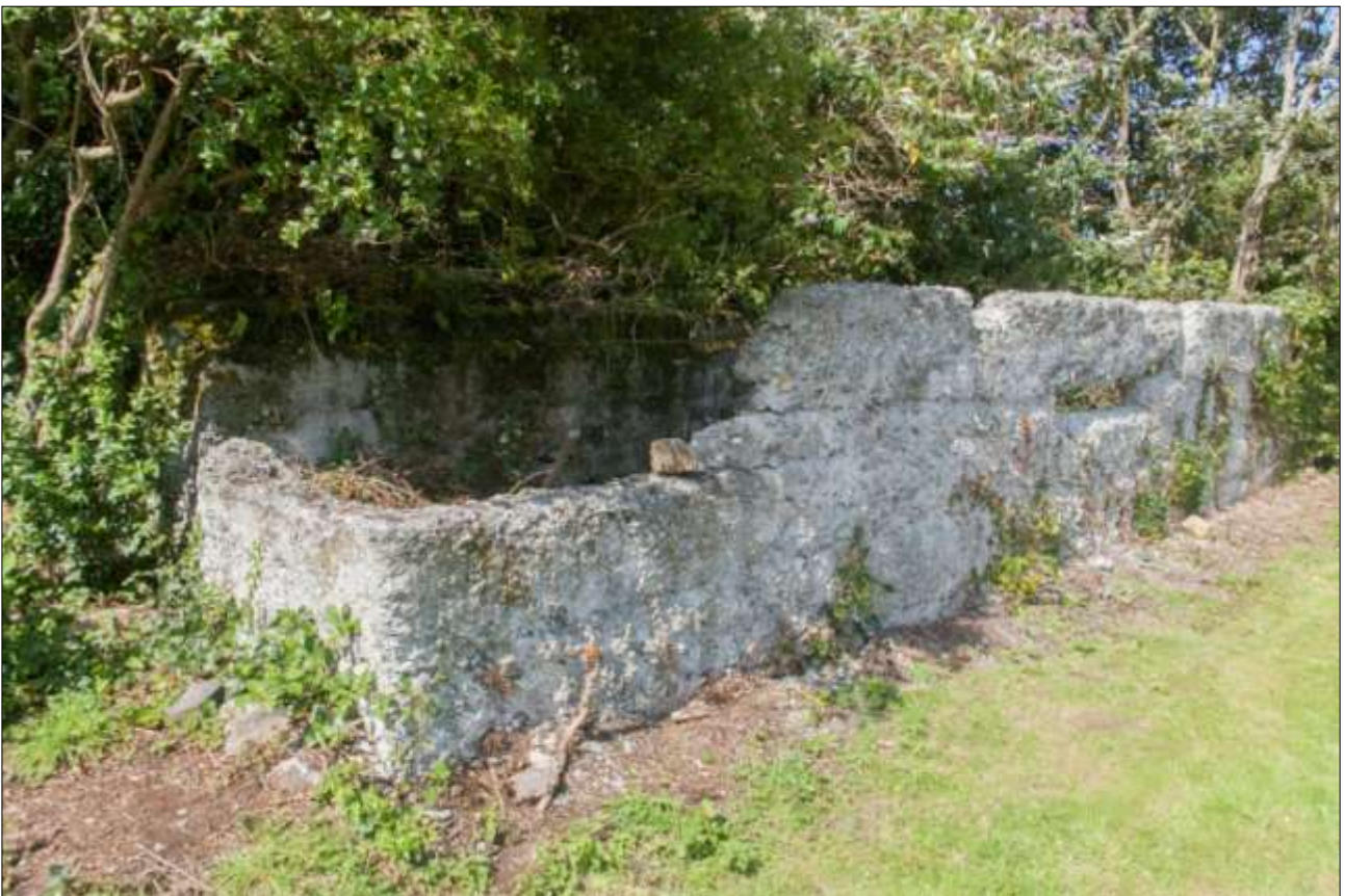
AS ABOVE, THE SOUTH-EAST ANGLE; VIEWED FROM THE SOUTH-EAST.
