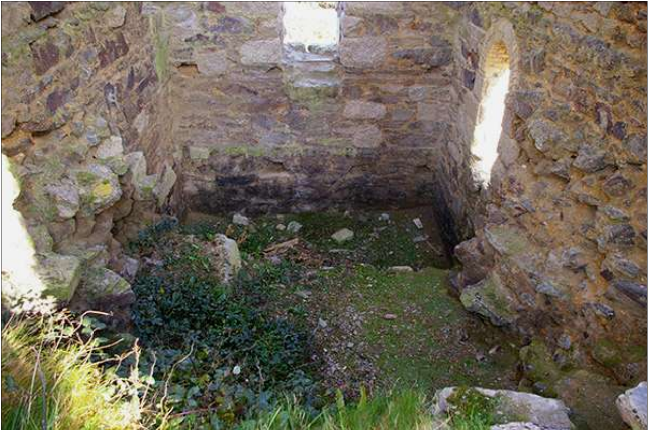
THE FLOOR OF THE ENGINE HOUSE SHOWING DEEP ENGINE PIT TO THE NORTH END; FROM THE SOUTH-WEST.
