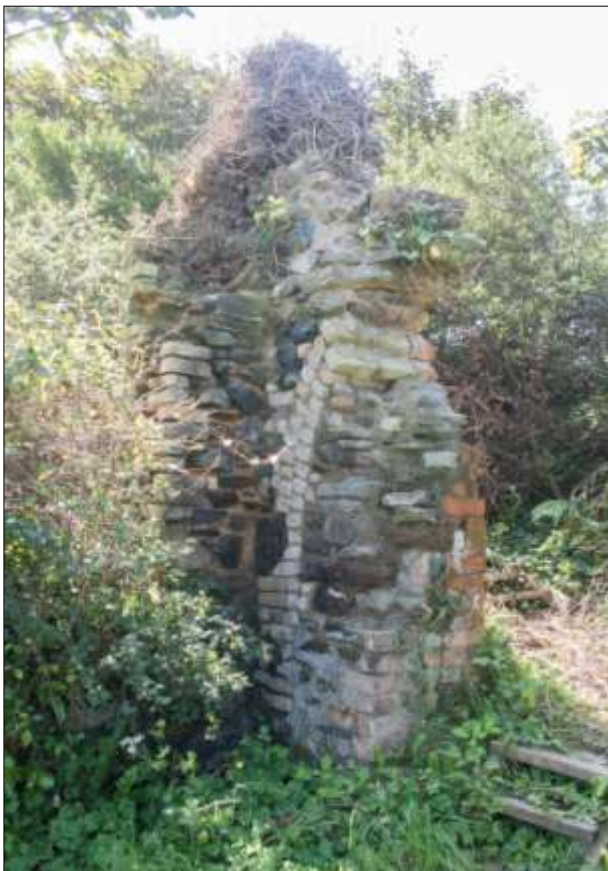
THE SOUTH-EAST INTERNAL CORNER OF THE BOILERHOUSE, SHOWING THE NARROWED PHASE 3 OPENING WITHIN A PARTLY-BLOCKED PHASE 2 OPENING; VIEWED FROM THE NORTH-WEST.
