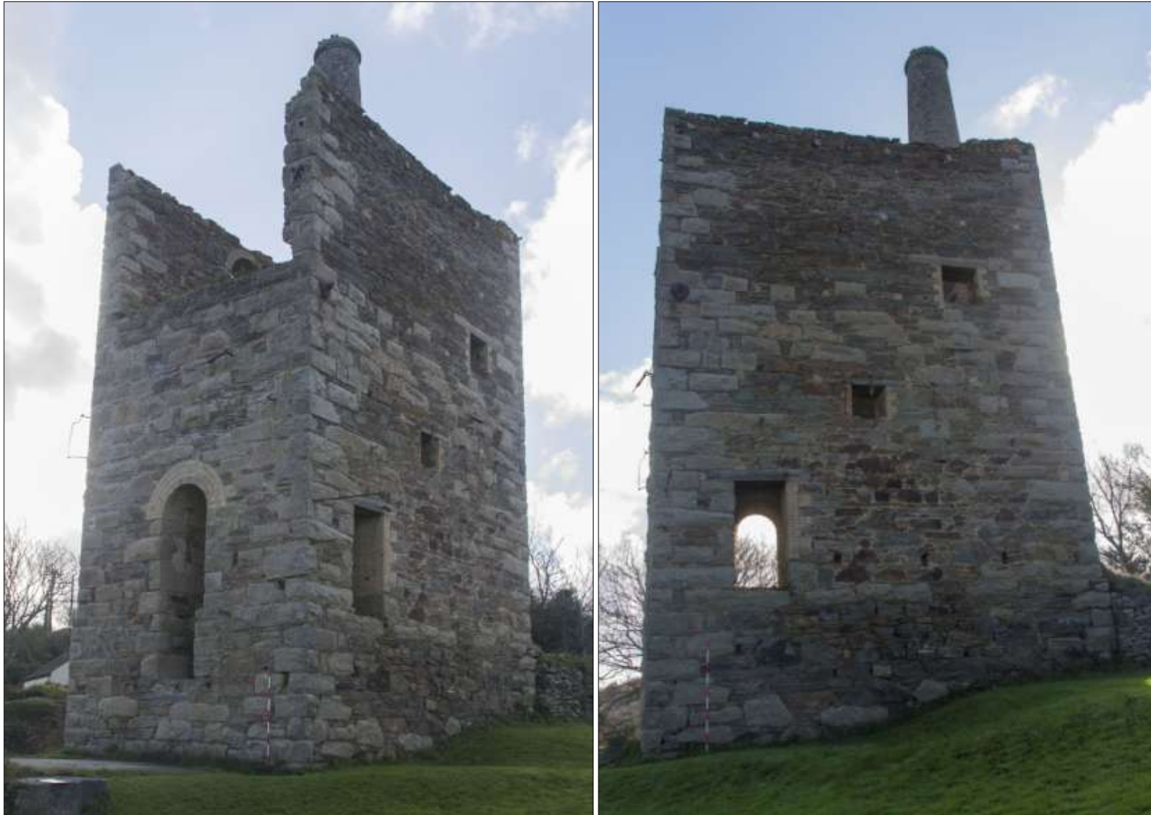
LEFT: THE NORTH-WEST AND NORTH-EAST ELEVATIONS OF THE ENGINE HOUSE; VIEWED FROM THE NORTH (SCALE 2M).
