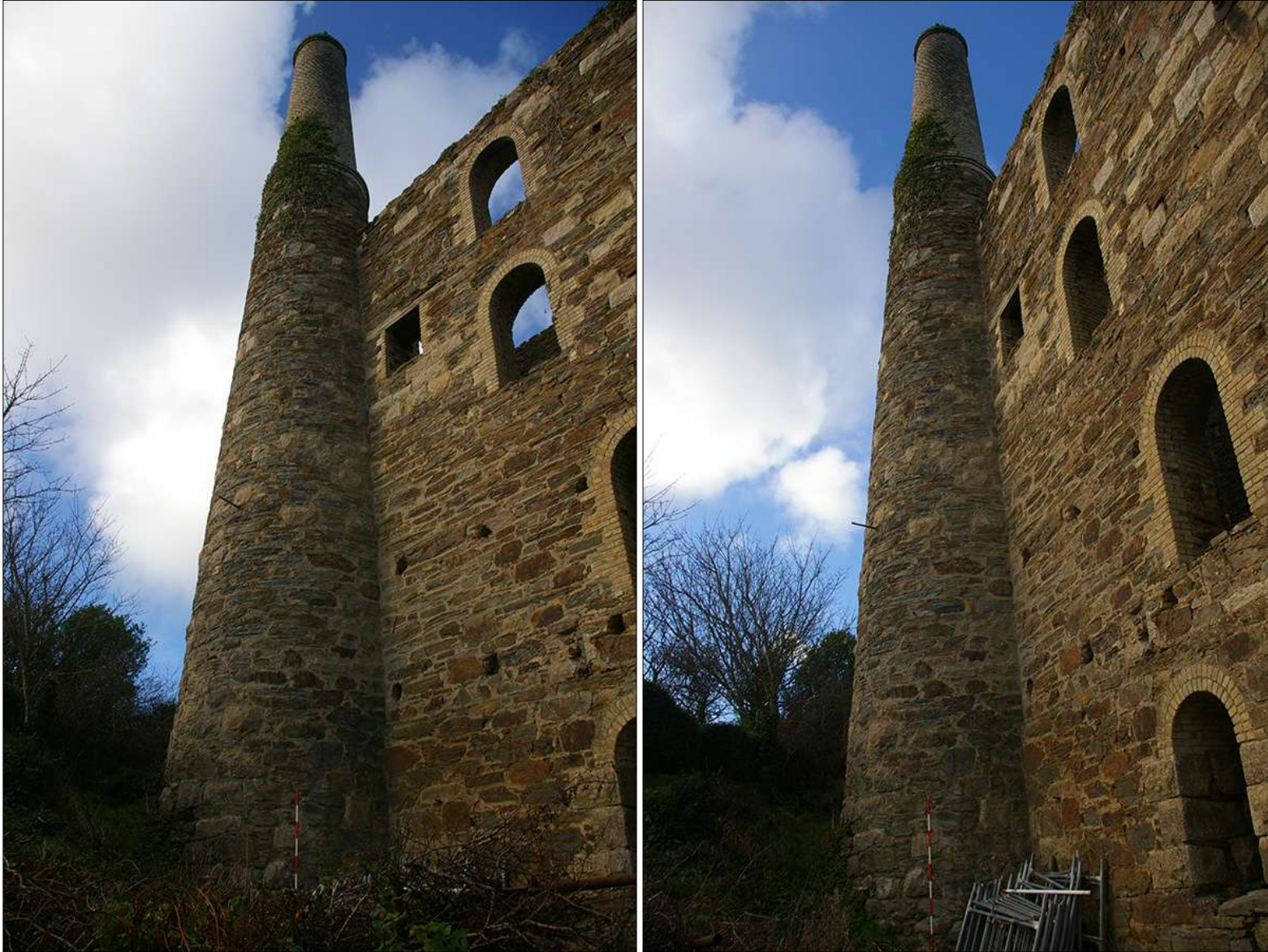
THE SOUTH-EAST ELEVATION AND CHIMNEY STACK; FROM THE EAST (SCALE 2M).
