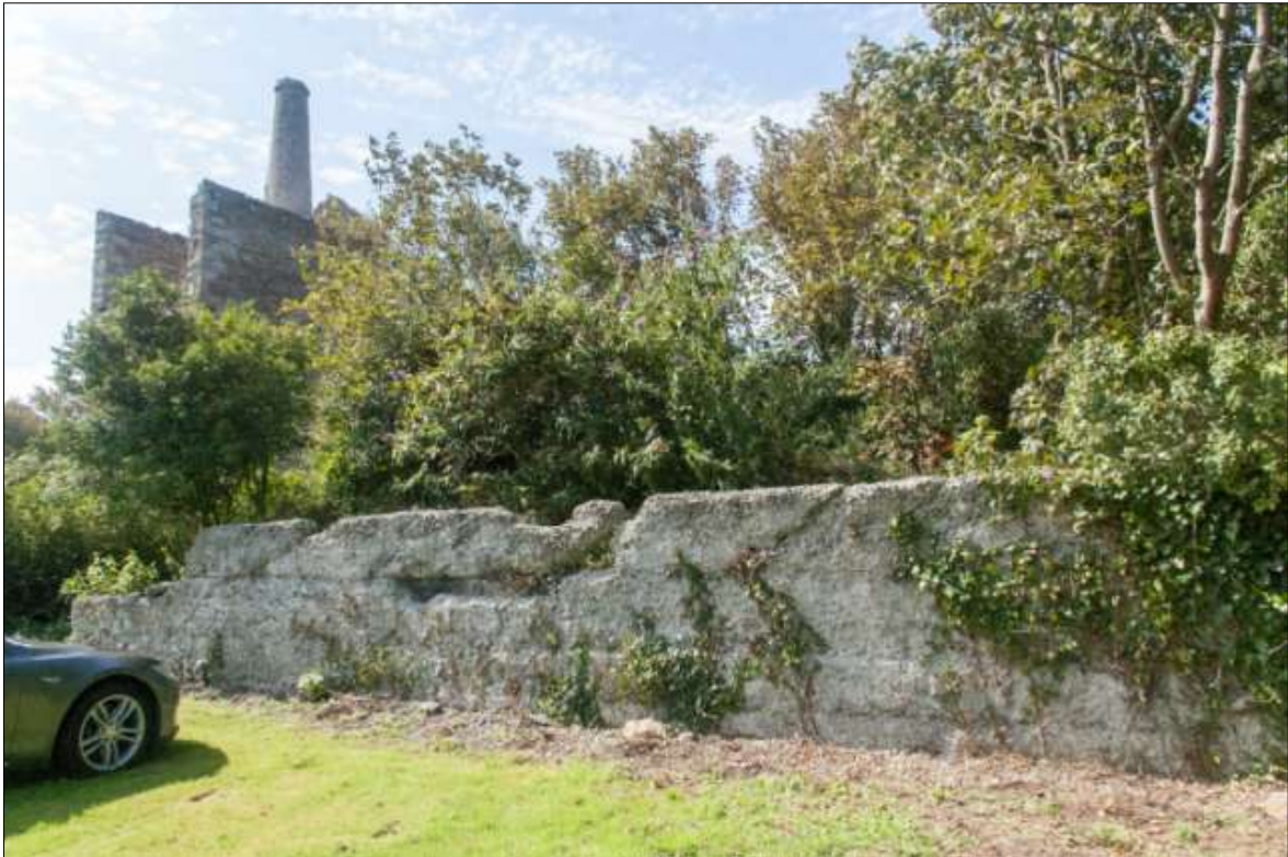
FIGURE 11: THE NORTH-EAST WALL OF THE STAMPS; VIEWED FROM THE NORTH-EAST.
