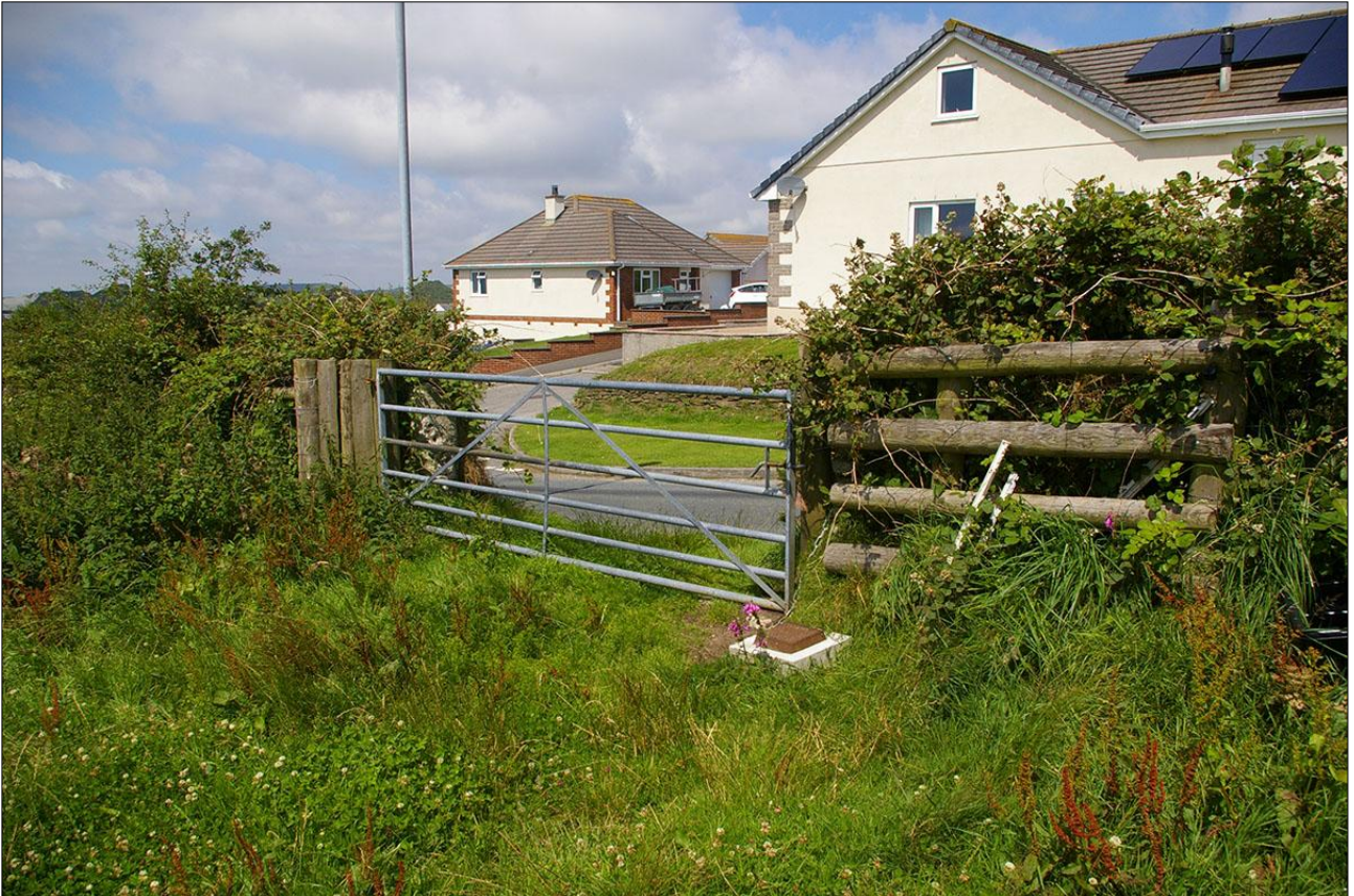
THE GATEWAY ONTO THE ROAD; VIEWED FROM THE SOUTH-EAST, LOOKING NORTH-WEST.
