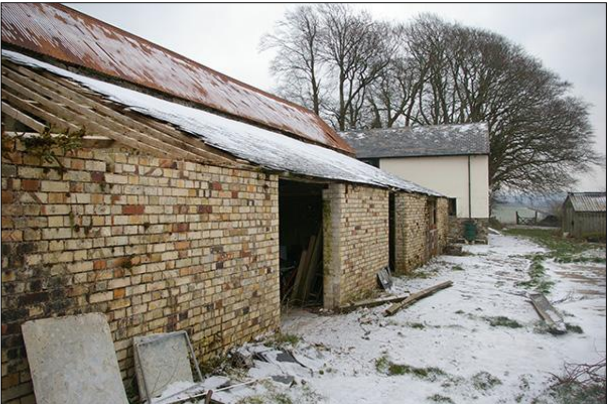
THE BRICK LEAN-TO, FROM THE NORTH-NORTH-WEST (2M SCALE).
