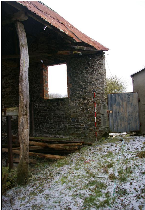
LEFT: THE NORTH ELEVATION OF THE LINHAY BARN, WITH LARGE LOADING DOOR WITH BRICK REVEALS, FROM THE EAST-SOUTH-EAST (2M SCALE).
