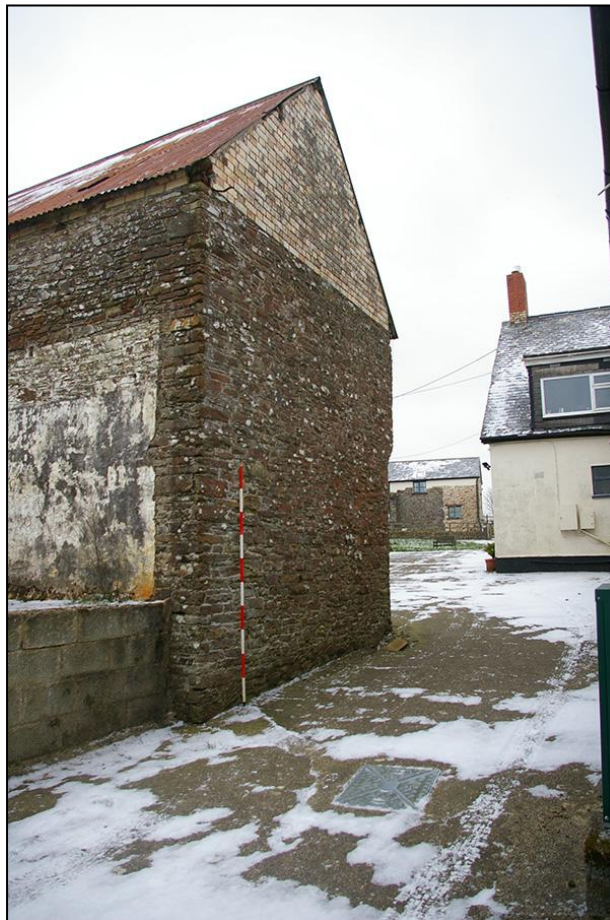
THE SOUTH ELEVATION OF THE LINHAY BARN, GOOD SLATESTONE STONEMWORK, WITH IN FILLED APEX, PROBABLY REPLACING WEATHER BOARDING, WITH BRICK, FROM THE SOUTH-WEST (2M SCALE).
