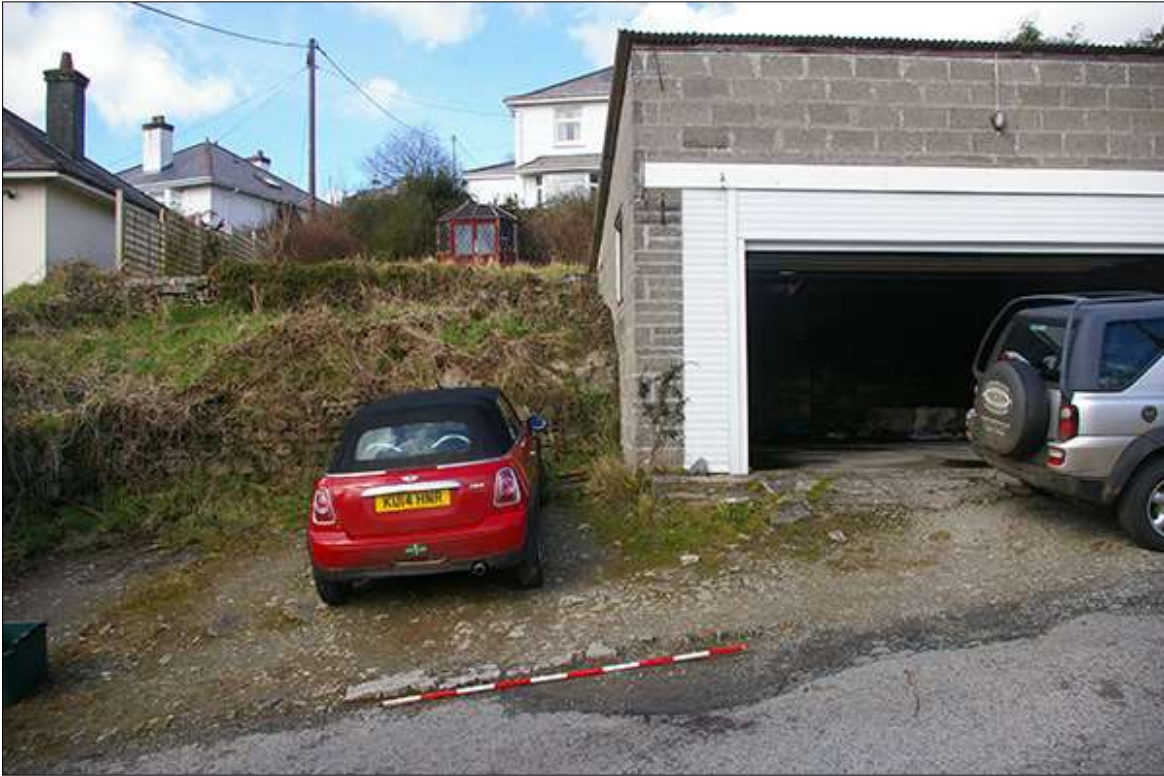
20. THE PLOT ACROSS THE ROAD, WITH RAISED KERB OF SLATE COBBLED AND SOME GRANITE AND SLATESTONE RUBBLE WALLING, INDICATING THERE MAY HAVE BEEN ANOTHER WALL ENCLOSING THAT SITE (POSSIBLY THE WORKHOUSE GARDEN WALL) OR ANOTHER BUILDING AT SOME POINT, WITH 2M SCALE; FROM THE SOUTH-EAST.
