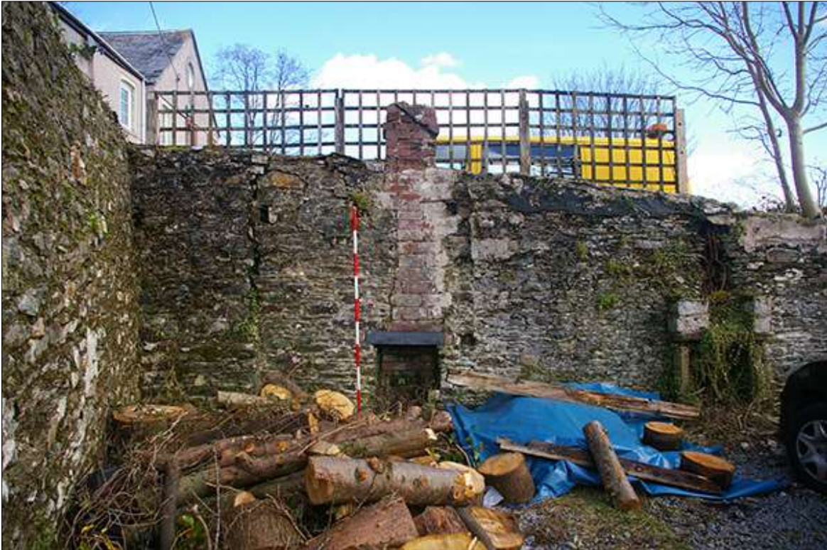
13. THE LOWER SITE; THE NORTH-EAST WALL, SHOWING THE INSERTED FLUE AND FIREPLACE, AND CLEAR BUILD LINE TO THE LEFT; VIEWED FROM THE SOUTH-SOUTH-WEST (SCALE 2M).
