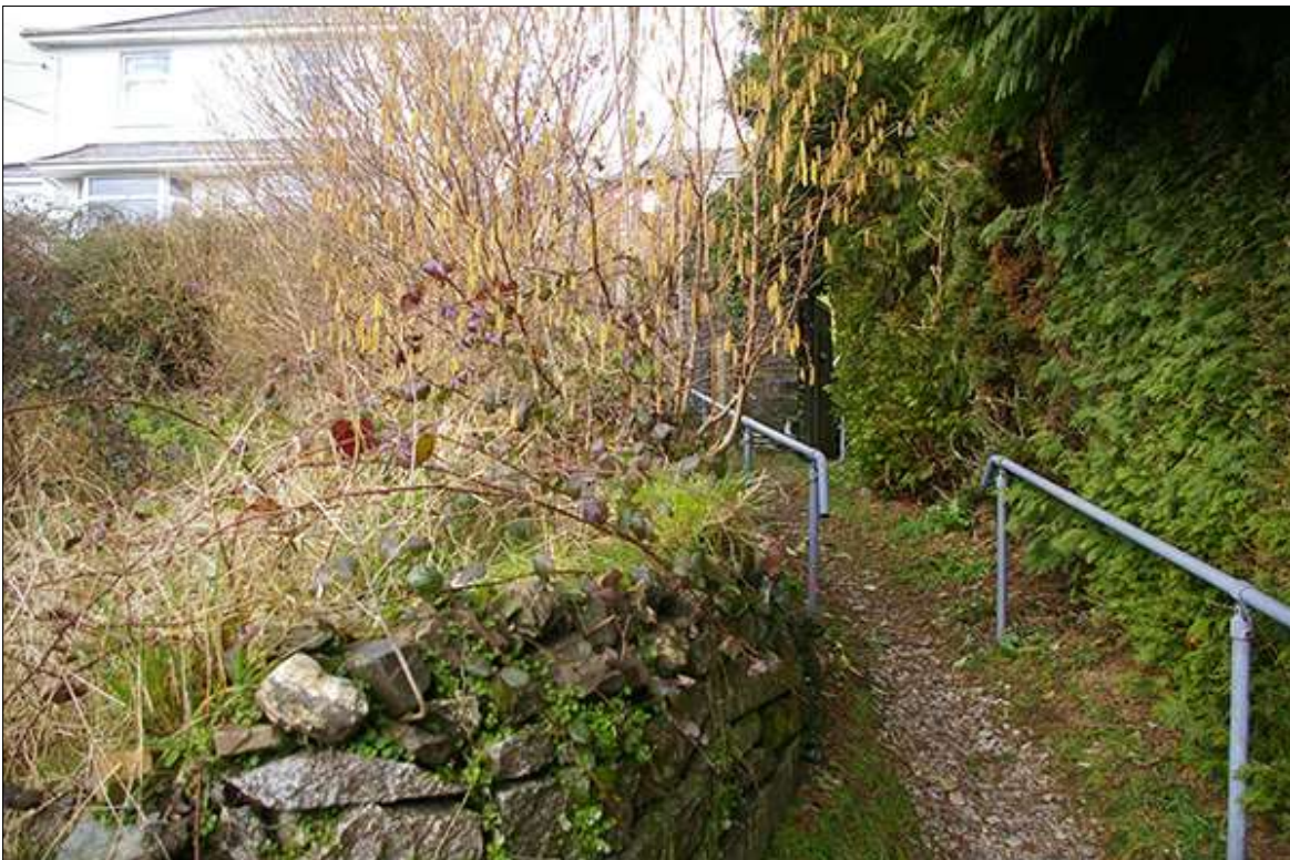
23. THE TOP PLOT, WITH LESS TERRACING AND ACCESS PATH ALONGSIDE THE CONCRETE GARAGE.
