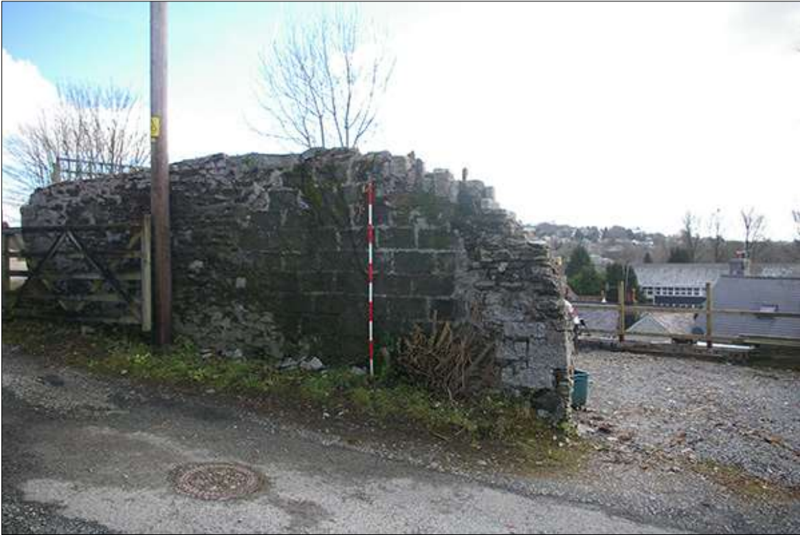
7. THE LOWER SITE, THE NORTH-WEST WALL FACING ONTO MAUDLINS PARK; VIEWED FROM THE WEST (SCALE 2M).
