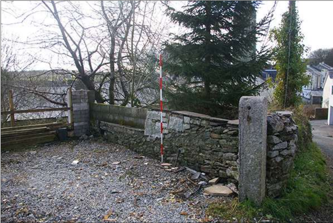
9. THE LOWER SITE, THE SOUTH-WEST WALL, SHOWING HOW THE SLOPING TOP OF THE WALL HAS BEEN BUILT UP WHICH REUSED GRANITE BLOCKS AND CONCRETE BLOCK; VIEWED FROM THE NORTH (SCALE 2M).
