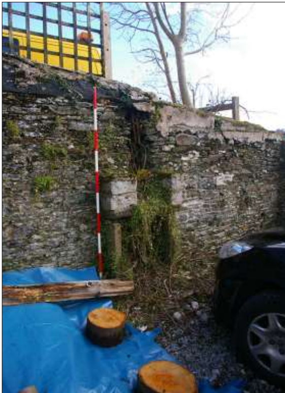
14. (LEFT) THE LOWER SITE; VIEW OF THE TERRACOTTA PIPE USED AS A FLUE SERVING A SMALL GRATE OR COPPER, CUT INTO THE NORTH-EAST WALL; VIEWED FROM THE WEST (SCALE 2M).
