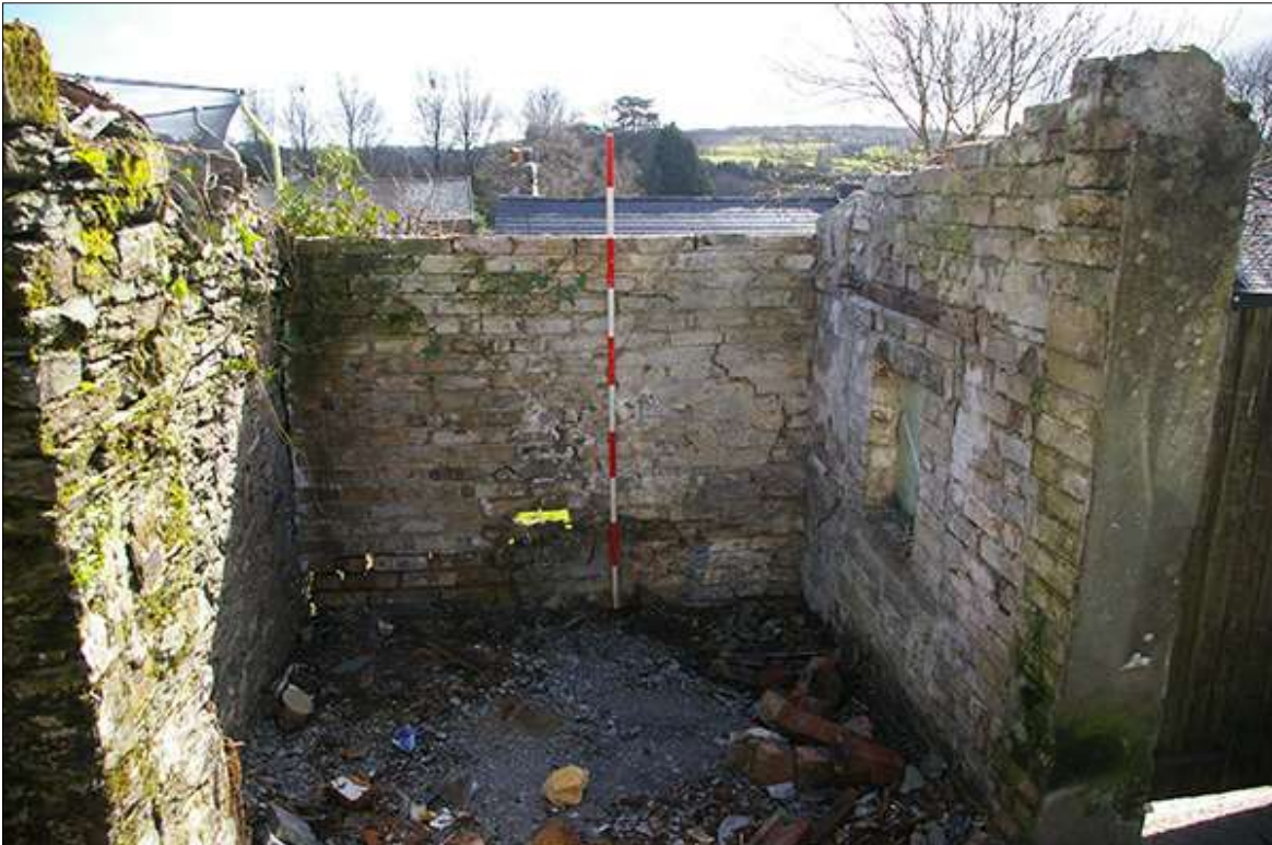
17. THE SMALL SUB-SQUARE BUILDING, FORMED FROM TWO BRICK WALLS ABUTTING THE EARLIER STONE RUBBLE BUILDING, WITH 2M SCALE; FROM THE NORTH-WEST.
