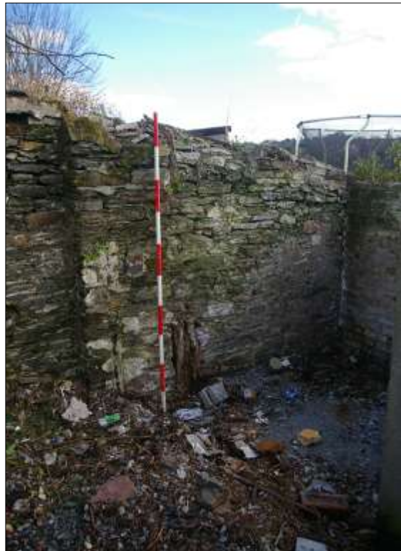
14. (LEFT) THE LOWER SITE; VIEW OF THE TERRACOTTA PIPE USED AS A FLUE SERVING A SMALL GRATE OR COPPER, CUT INTO THE NORTH-EAST WALL; VIEWED FROM THE WEST (SCALE 2M).
