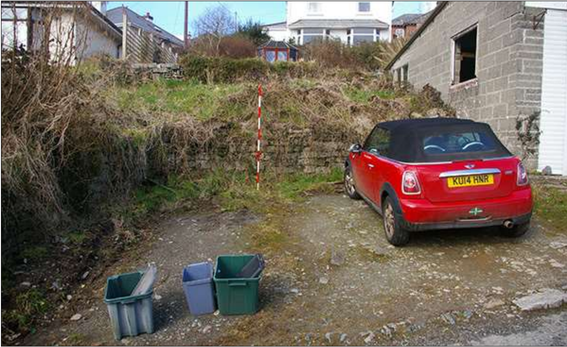
22. THE STEEP TERRACING WHICH CUTS INTO THE SLOPE OF THE HILLSIDE, OF 19 TH AND 20 TH CENTURY DATE. MUCH OF THIS AREA TO THE WEST WAS DEVELOPED IN THE 1920S AND 1930S BUILDING SPACIOUS CHALET BUNGALOW STYLE HOUSES; FROM THE EAST, NORTH-EAST.
