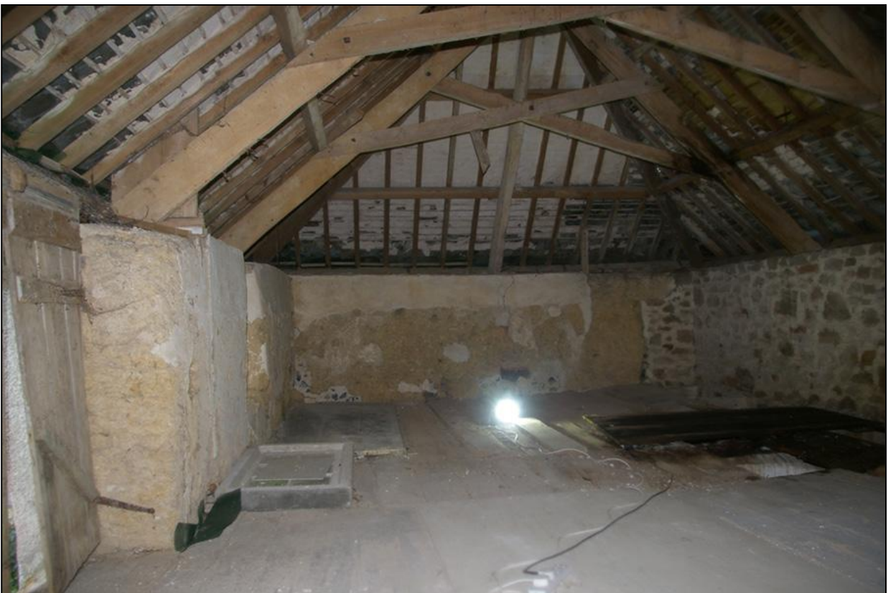
THE EAST END OF THE LOFT, BUILDING 1; FROM THE EAST, NORTH-EAST.
