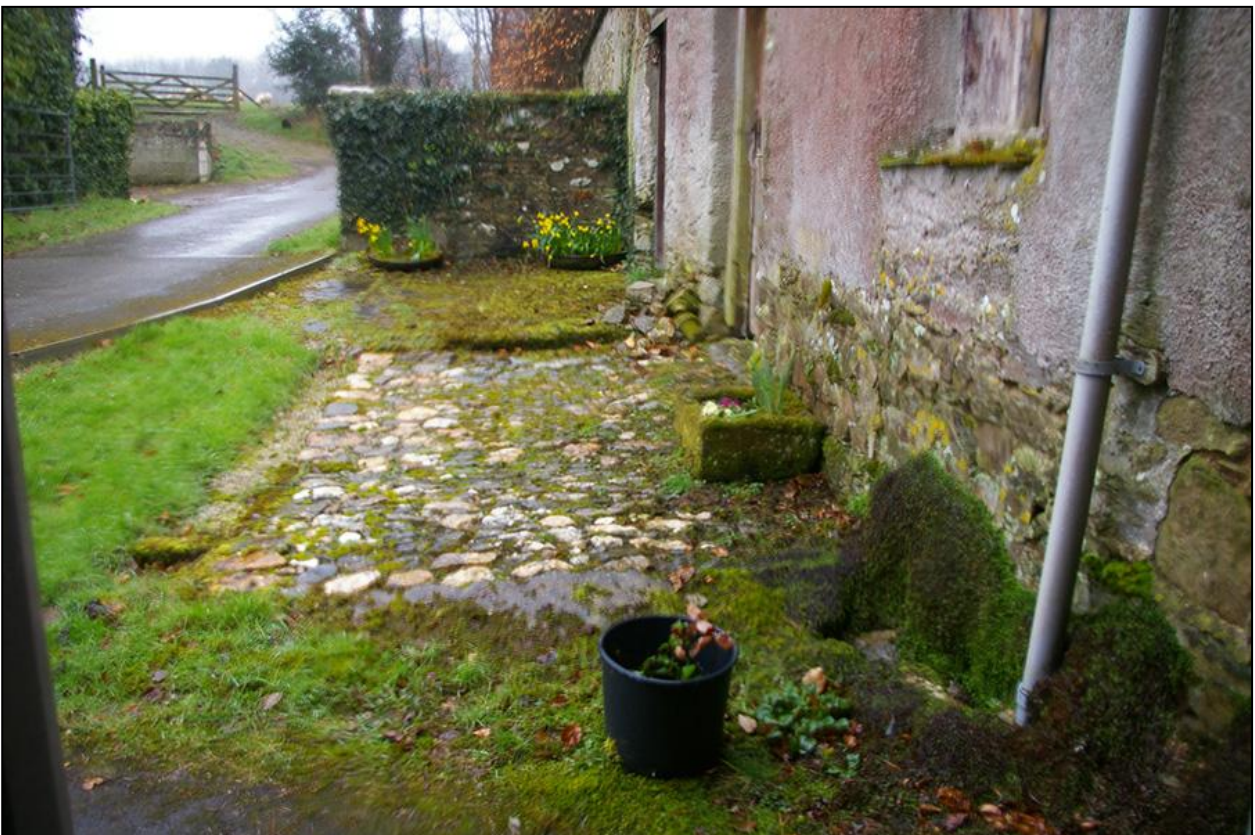
THE COBBLED AND QUARTZ PEBBLE FORMER YARD SURFACE WHICH SURVIVES ALONG THE NORTH ELEVATION OF BUILDING 1; FROM THE WEST.
