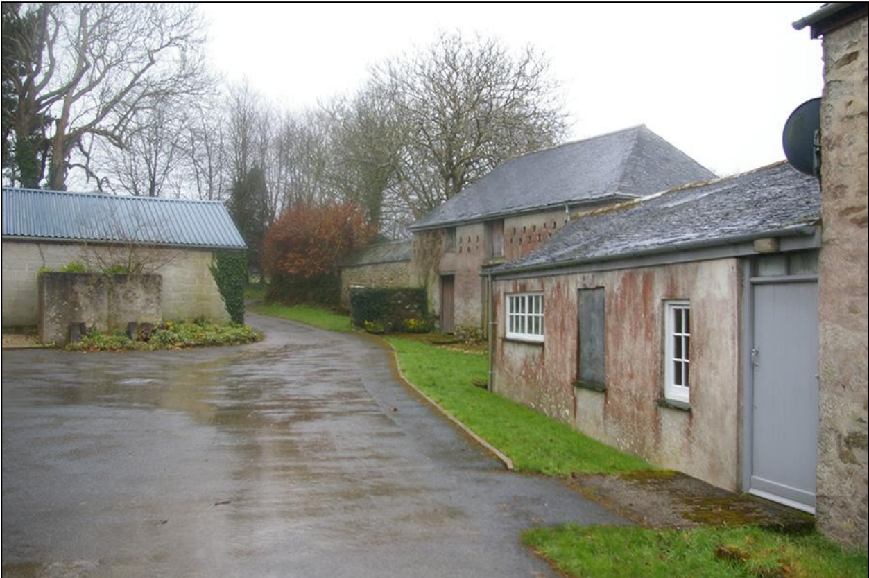
BUILDINGS 1 AND 2, IN THE CONTEXT OF THE CARRIAGE DRIVE AND FARMYARD; FROM THE WEST, NORTH-WEST.
