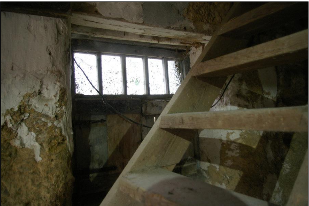
THE WINDOW IN THE WEST COMPARTMENT, WITHIN A BLOCKED DOORWAY, SCREENED BY THE RELATIVELY MODERN STAIRS TO THE LOFT SPACE; FROM THE SOUTH-WEST.
