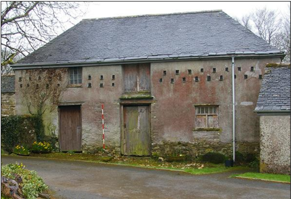
FIGURE 7: BUILDING 1, VIEWED FROM THE NORTH
