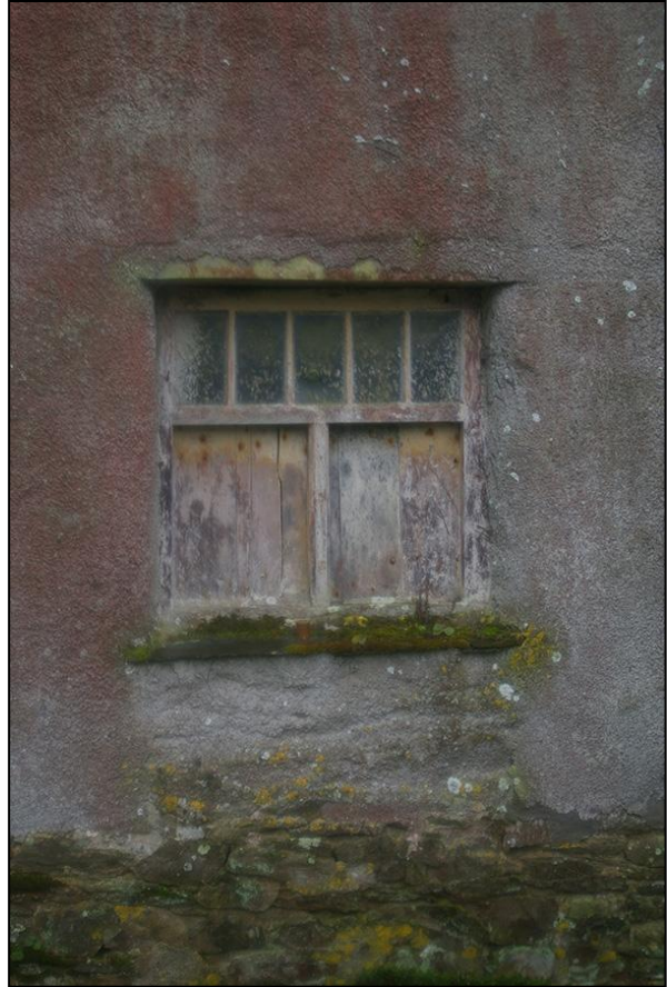
THE CENTRAL DOOR IN THE NORTH ELEVATION OF BUILDING 1 AND THE LOADING DOOR ABOVE; FROM THE NORTH [LEFT]. THE WINDOW TO THE WEST, GROUND FLOOR OF BUILDING 1, SET INTO A BLOCKED DOORWAY; FROM THE NORTH [RIGHT].
