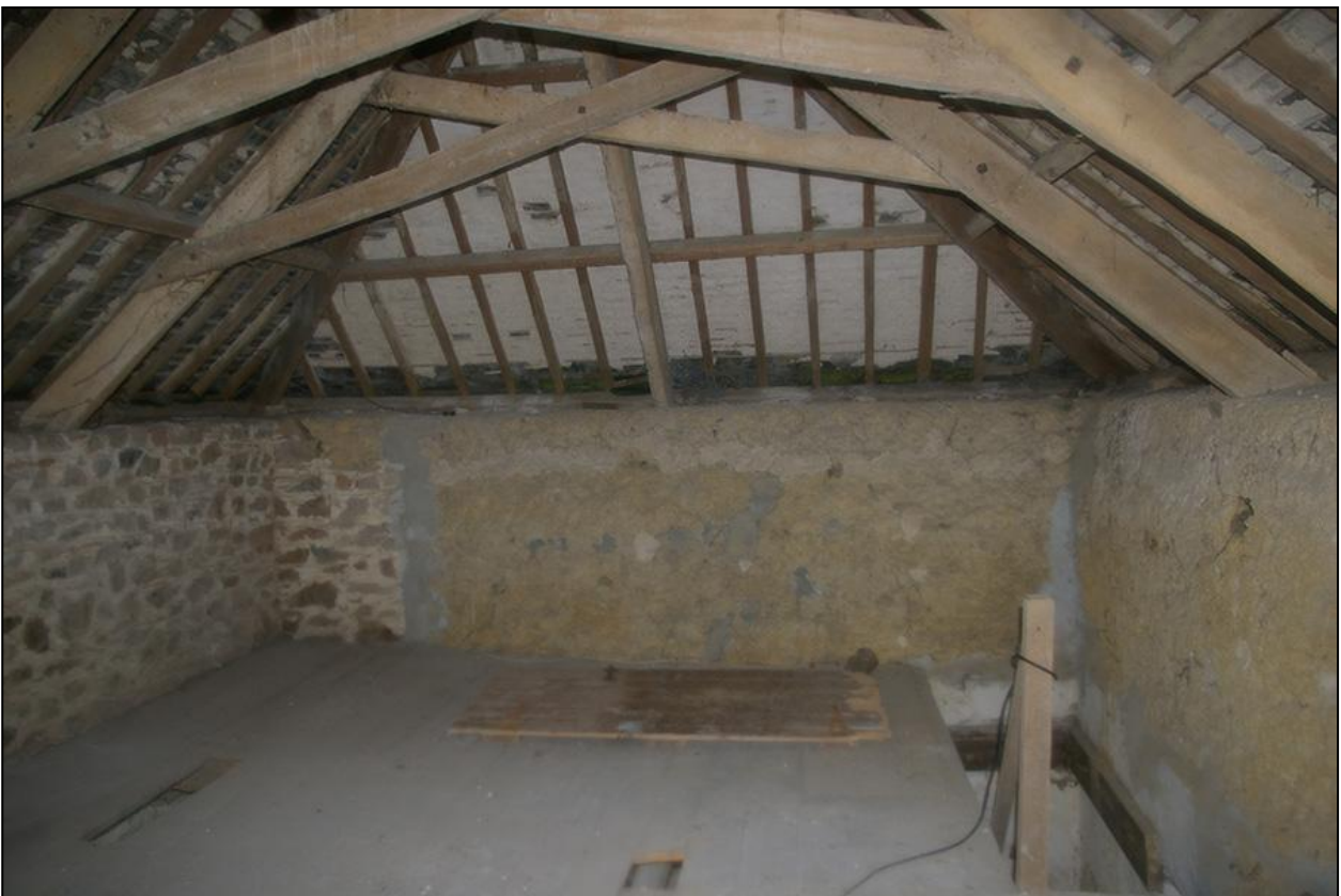
THE WEST END OF THE LOFT; FROM THE EAST, NORTH EAST.
