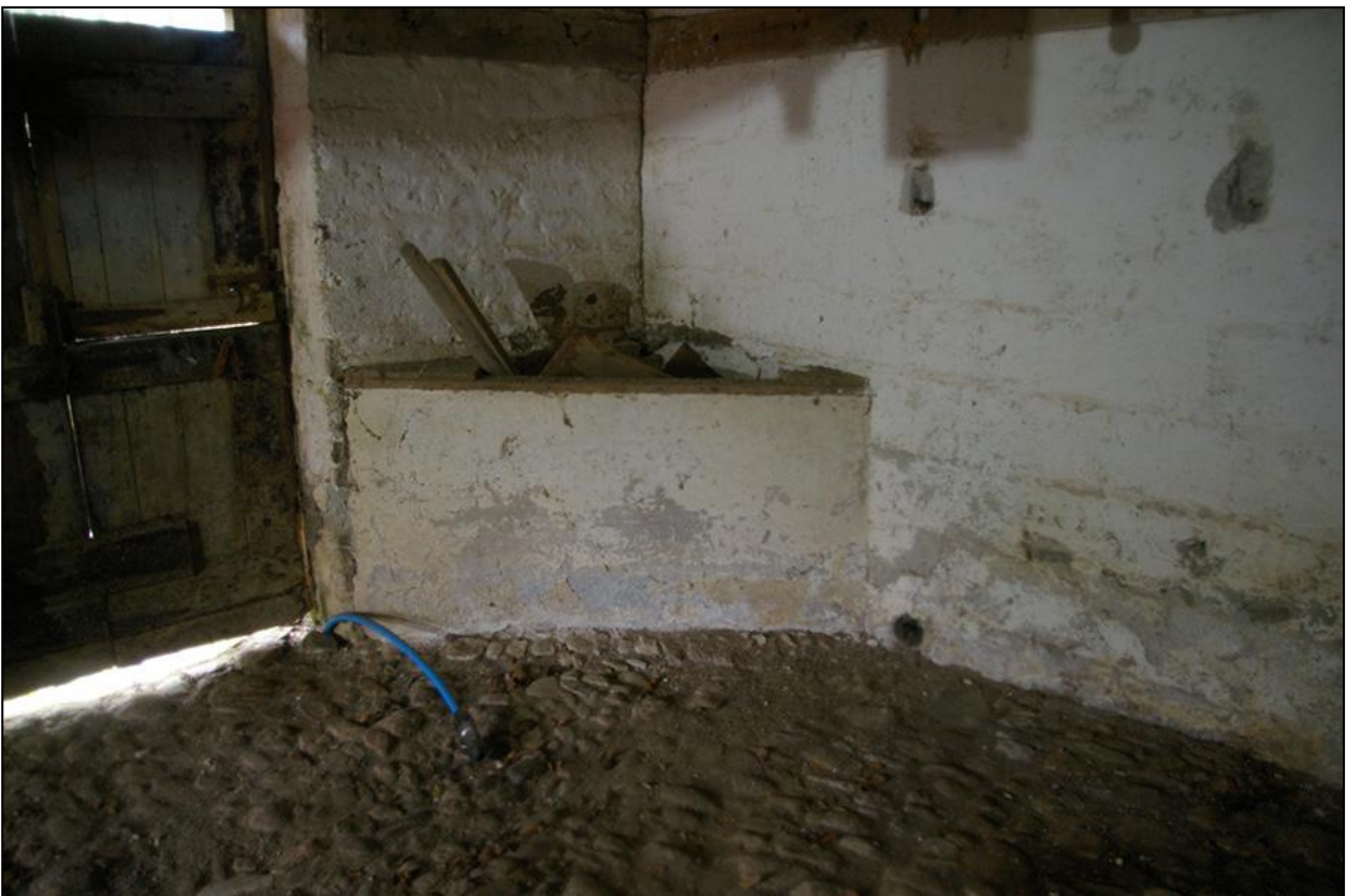
THE DOOR IN THE NORTH WALL, SERVING THE WEST COMPARTMENT AND THE HAYRACK BUILT INTO THE NORTH-EAST CORNER; FROM THE SOUTH AND SOUTH-WEST.
