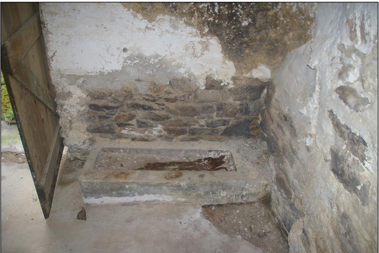
TROUGH IN THE NORTH-EAST CORNER OF BUILDING 1; FROM THE SOUTH.
