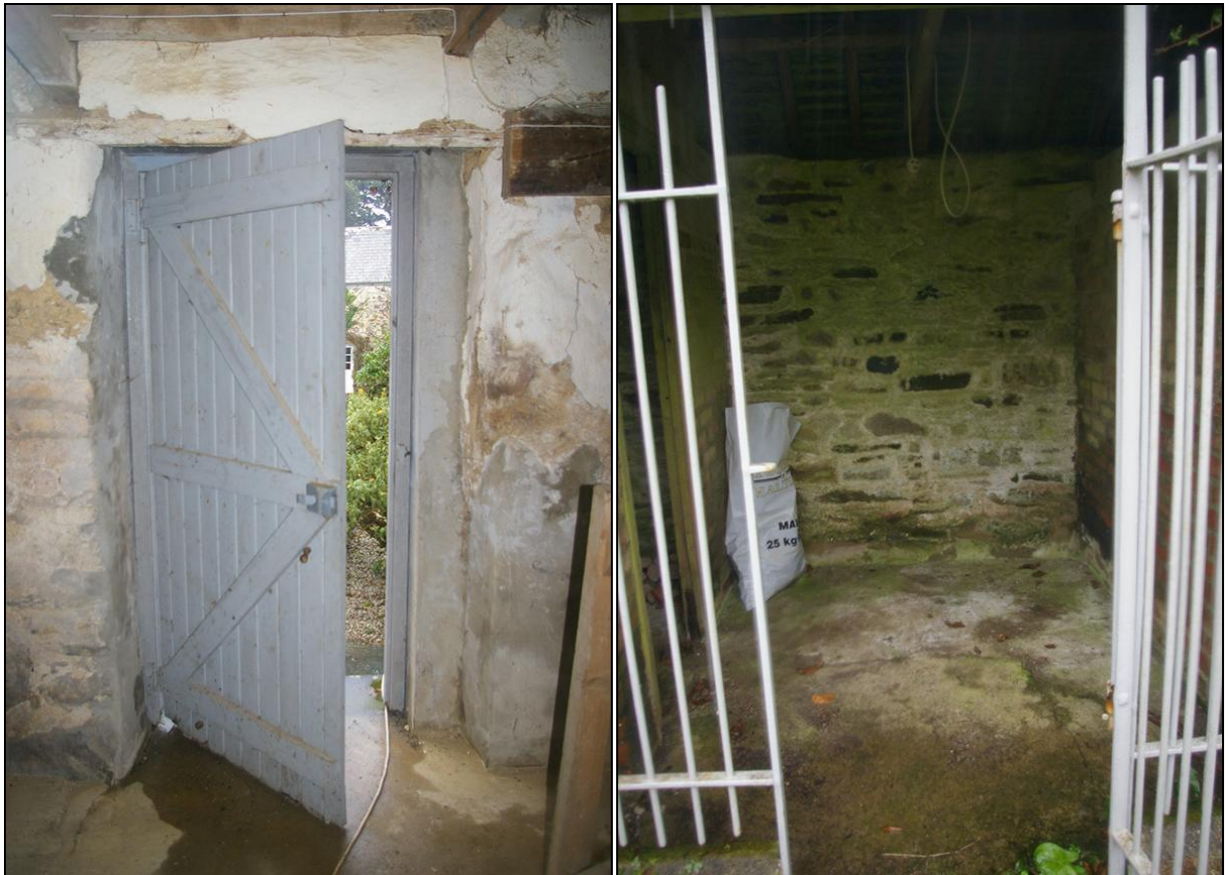
THE WEST DOOR IN THE WEST WALL OF BUILDING 1, SHOWING THE FORCED AND REPAIRED SIDES AND INSERTED RECYCLED TIMBER LINTEL; FROM THE EAST [LEFT]. THE KENNELS, AN OUTER PEN AND INNER CLOSED ROOM, SET WITHIN BUILDING 2, TO THE WEST END, AGAINST BUILDING 1; FROM THE SOUTH, SOUTH-EAST AND NORTH-EAST [RIGHT].
