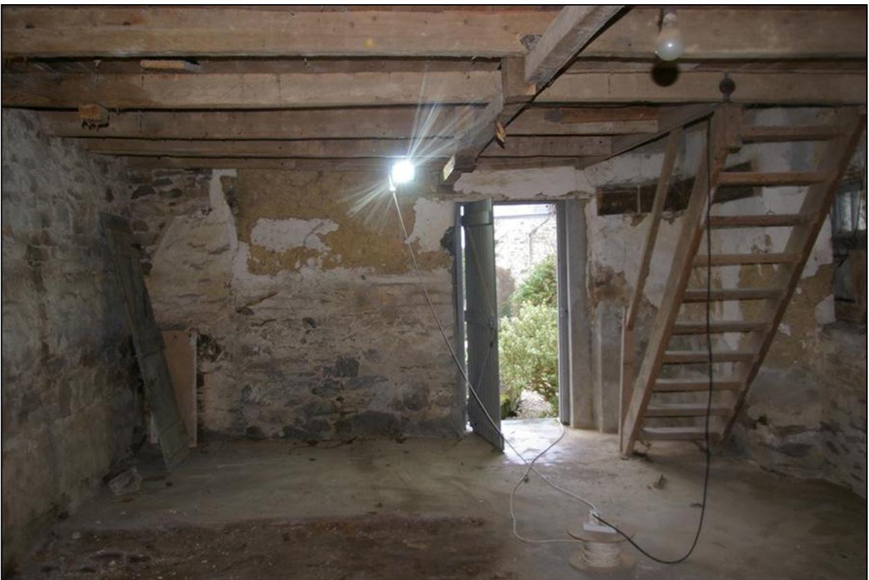
THE WEST WALL OF BUILDING 1, FROM THE INTERIOR; FROM THE EAST.
