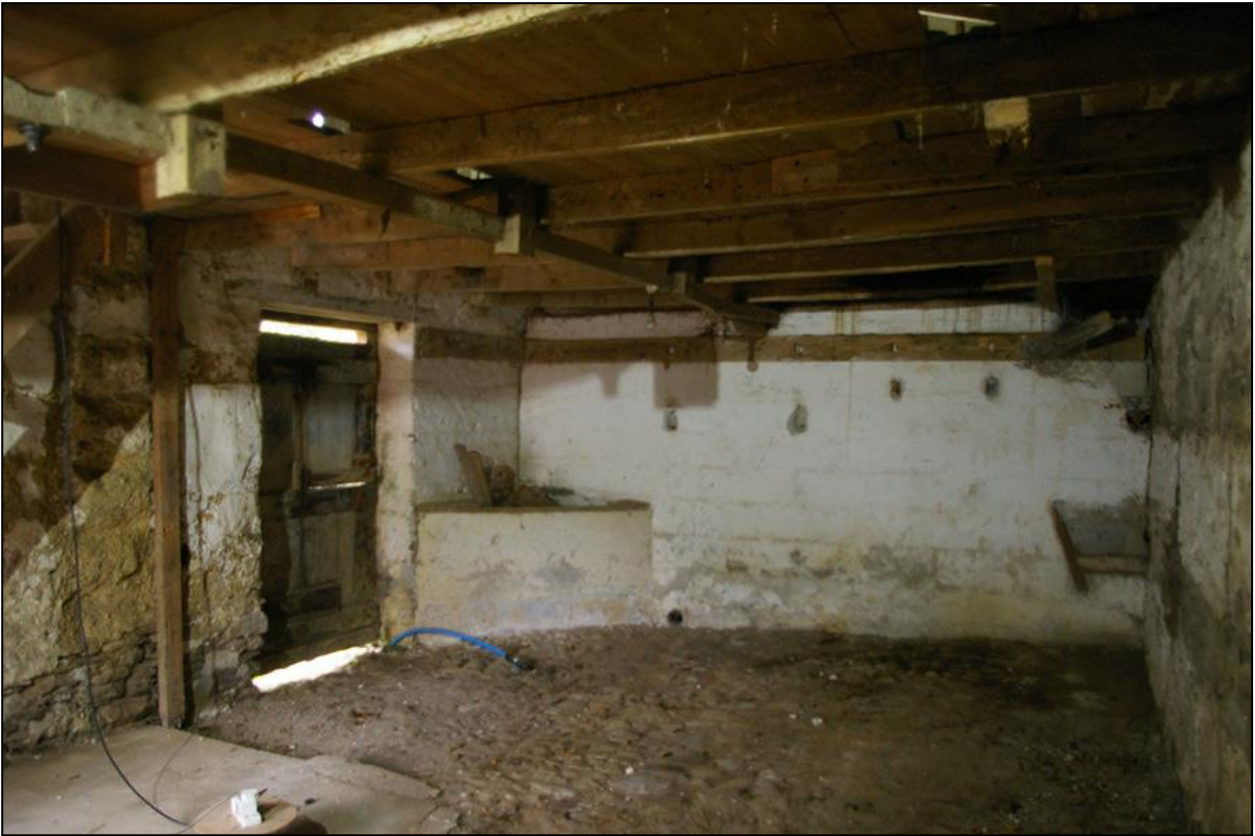
THE WEST COMPARTMENT, VIEWED FROM THE SOUTH-WEST CORNER.
