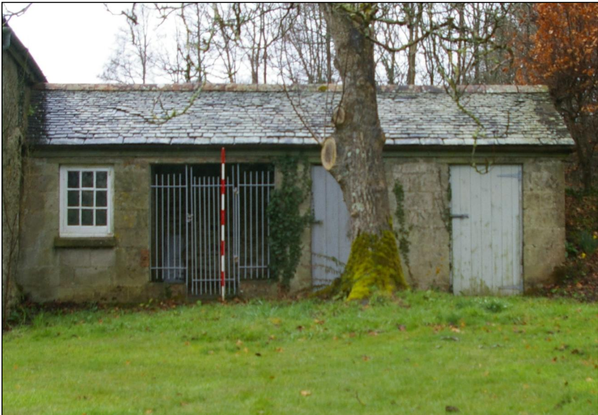
FIGURE 8: BUILDING 2, VIEWED FROM THE SOUTH, 2M SCALE
