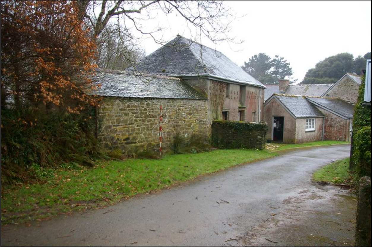
THE APPROACH TO THE FARMYARD ALONG THE HISTORIC FORMER CARRIAGE DRIVE, WITH 2M SCALE; FROM THE EAST, NORTH-EAST.
