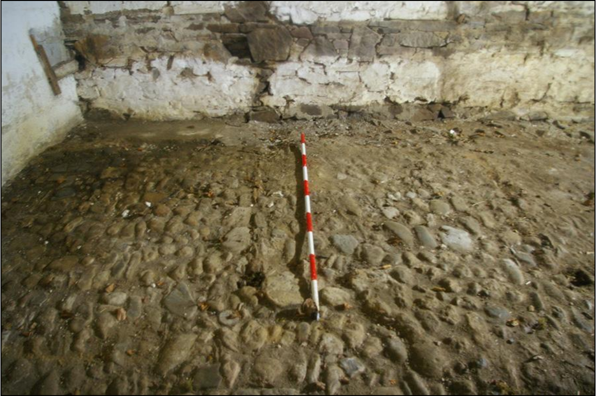
THE PARTITION SLOTS AND SOCKETS, INDICATING THE FORMER WIDE STALLS IN THE COBBLED FLOOR OF BUILDING 1, WITH 2M SCALES; FROM THE NORTH.
