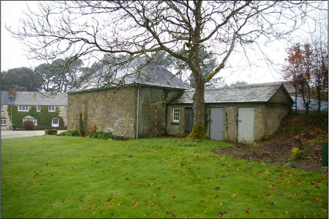
THE EAST ELEVATION OF BUILDING 1, WITH 2M SCALE; FROM THE SOUTH-EAST.
