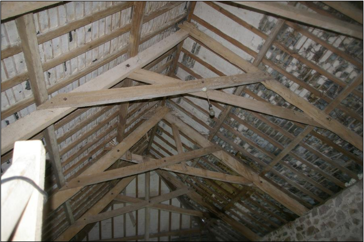
THE ROOF OF BUILDING 1; FROM THE NORTH-WEST CORNER.
