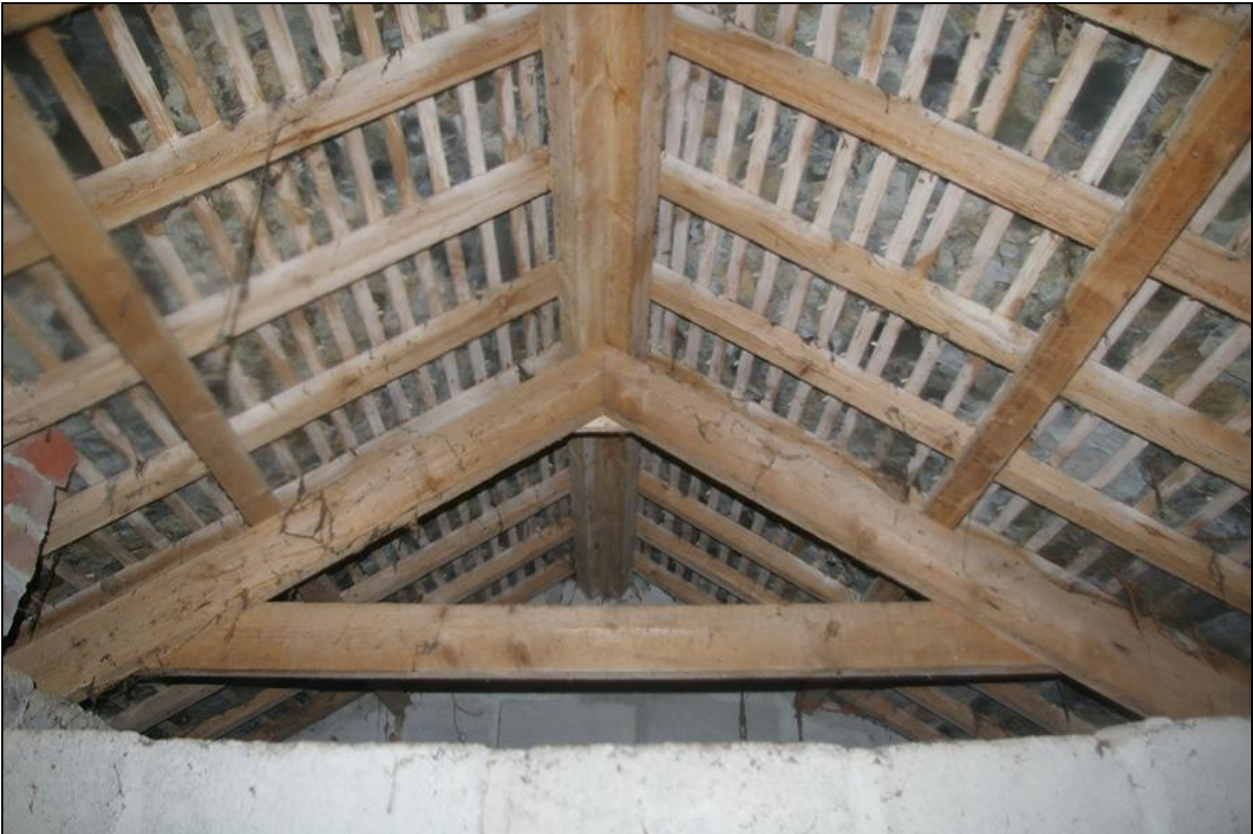
THE BASIC A-FRAME ROOF STRUCTURE IN BUILDING 2; FROM THE WEST.
