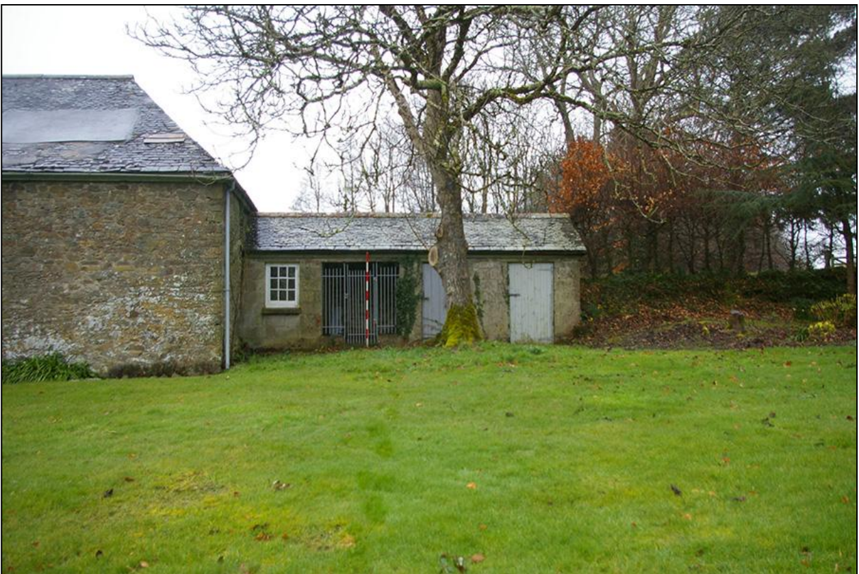
THE SOUTH ELEVATION OF BUILDING 2, WITH 2M SCALE; FROM THE SOUTH.
