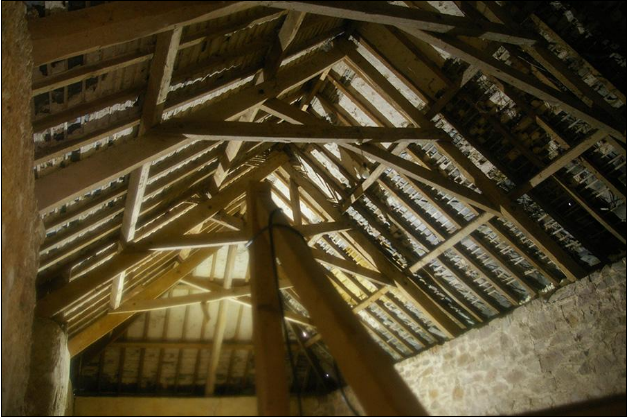
ROOF OF BUILDING 1; FROM THE NORTH-WEST CORNER.
