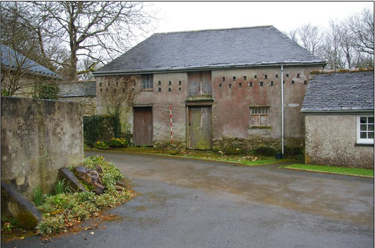
THE NORTH ELEVATION OF BUILDING 1, WITH 2M SCALE; FROM THE NORTH.
