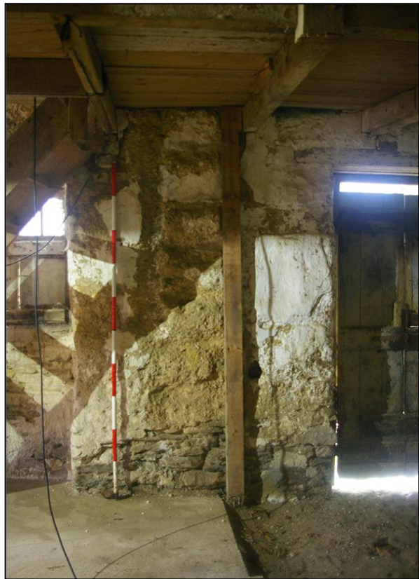
THE DRAIN WITHIN THE COBBLES, TO THE NORTH SIDE OF THE SURVIVING COBBLED FLOOR IN BUILDING 1, WITH 2M SCALE; FROM THE WEST [LEFT]. THE SCARRING AND MARKS IN THE LIME WASH AND PLASTER WHERE THE FORMER LOFT LADDER WAS ATTACHED TO THE NORTH WALL OF BUILDING 1, WITH 2M SCALE; FORM THE SOUTH [RIGHT].
