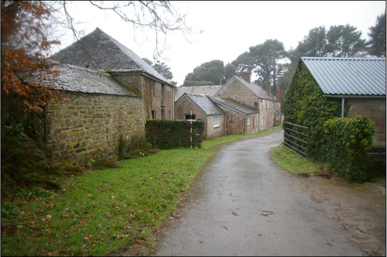
THE ENTRANCE TO THE FARMYARD: A LOOSE SLATESTONE RUBBLE WALL ENCLOSES THE DRIVEWAY NOW, REDUCING THE OPENING, WITH 2M SCALE; FROM THE EAST.
