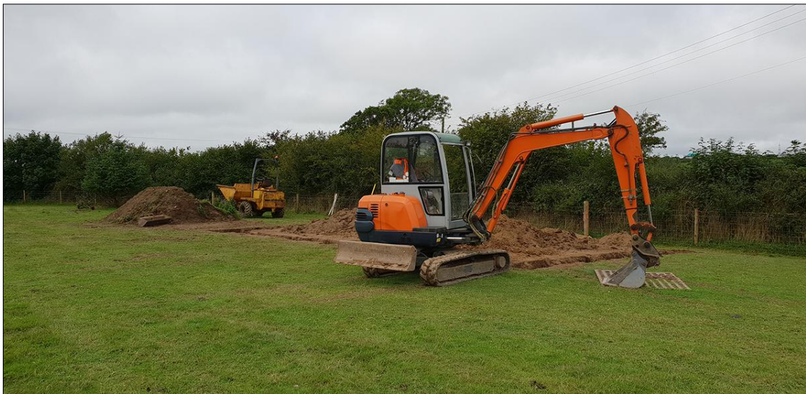
21. GENERAL POST-EXCAVATION SITE VIEW; VIEWED FROM THE SOUTH-EAST (NO SCALE).
