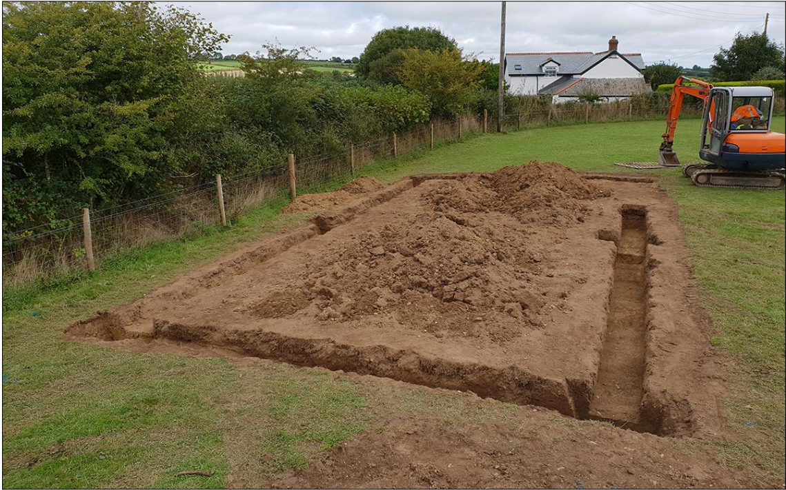
22. GENERAL POST-EXCAVATION SITE VIEW; VIEWED FROM THE WEST (NO SCALE).
