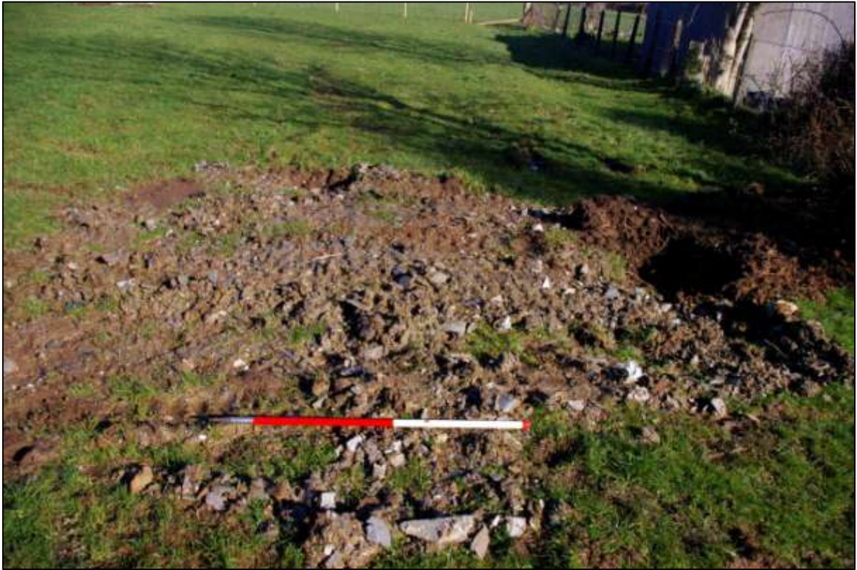
THE GEOTECHNICAL TEST PIT NEAR THE SOUTH CORNER OF THE SITE (SCALE 1M).
