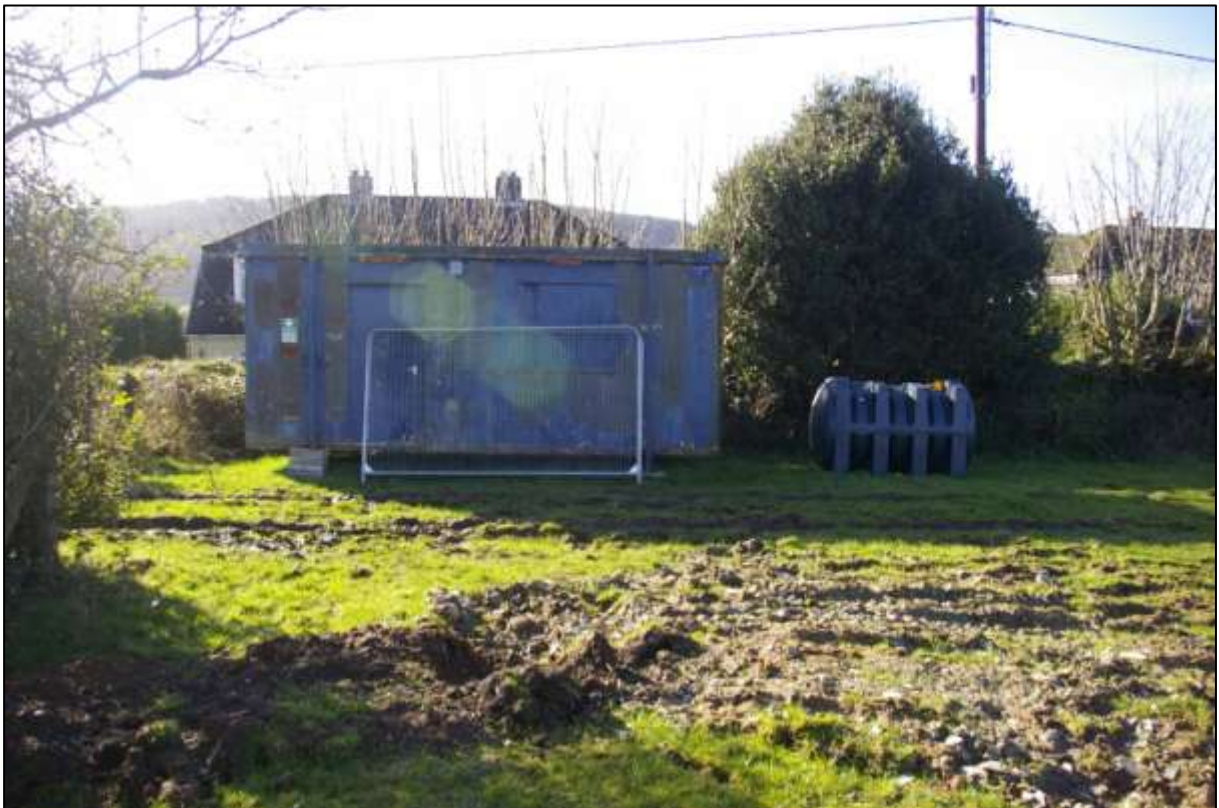
THE SOUTHERN CORNER OF THE SITE, SHOWING THE SITE CABIN AND HERAS FENCING.
