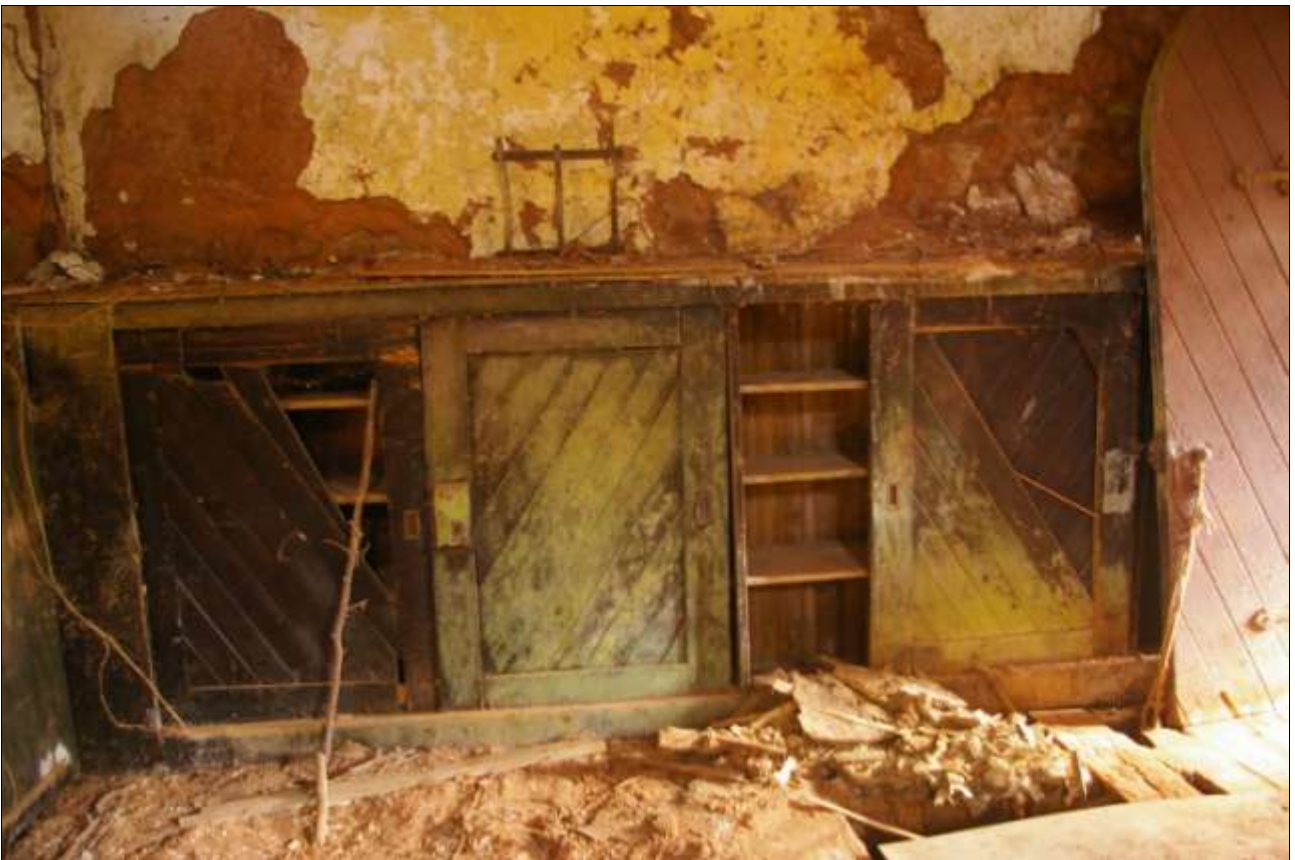
SURVIVING CUPBOARDS, VIEWED FROM THE WEST (NO SCALE).
