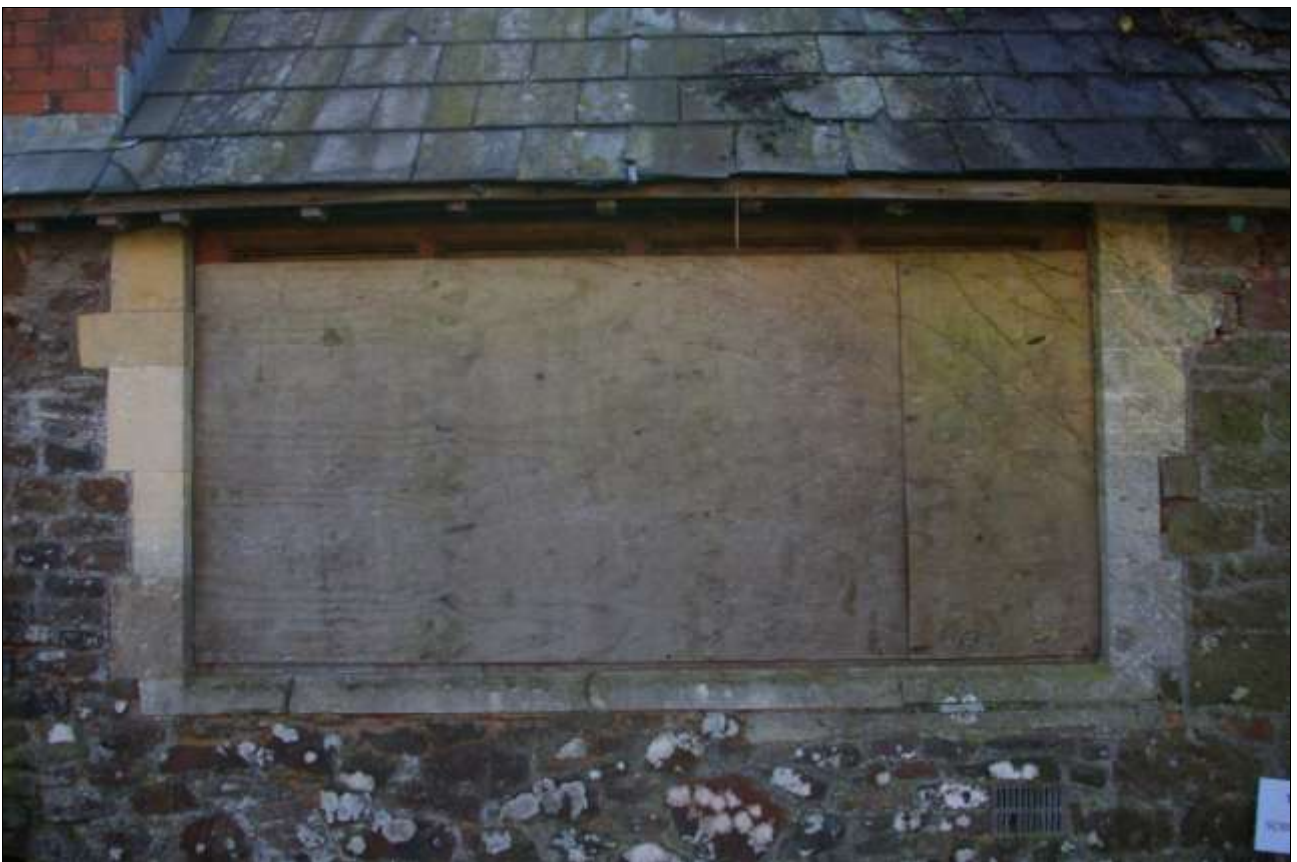
LARGE WINDOW IN NORTH ELEVATION, VIEWED FROM THE NORTH (NO SCALE).
