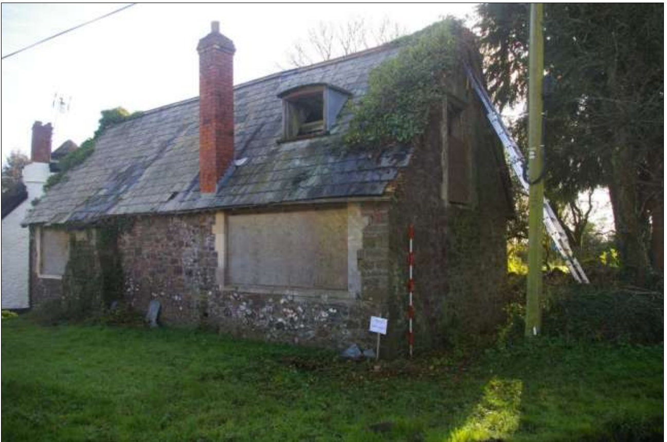
NORTH AND WEST ELEVATIONS. VIEWED FROM THE NORTH (2M SCALE).
