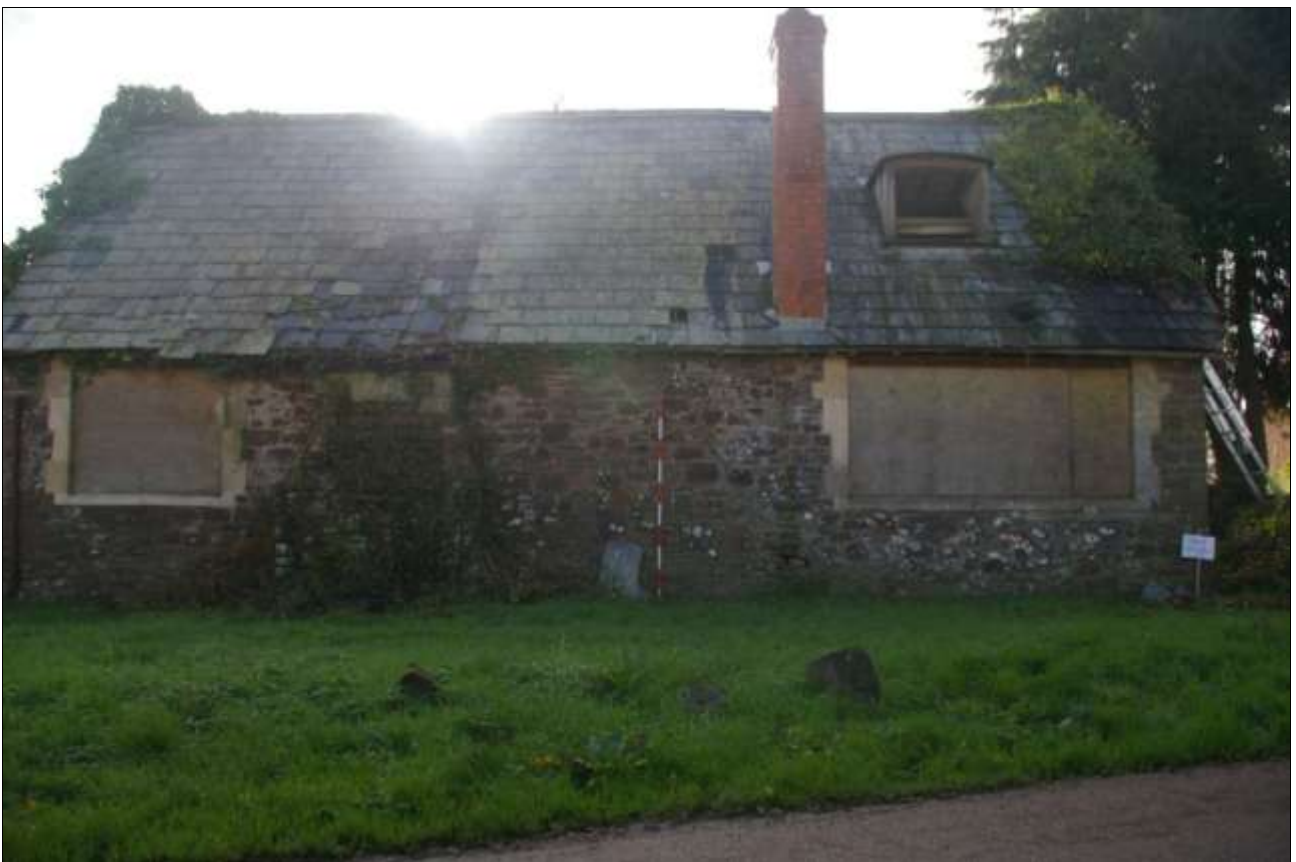
NORTH ELEVATION, VIEWED FROM THE NORTH (2M SCALE).
