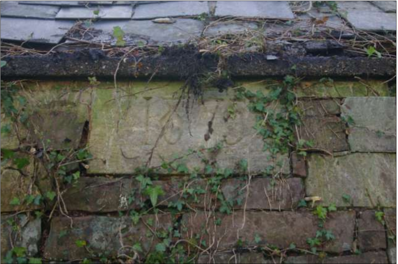
DATESTONE IN THE NORTH ELEVATION, VIEWED FROM THE NORTH (NO SCALE).
