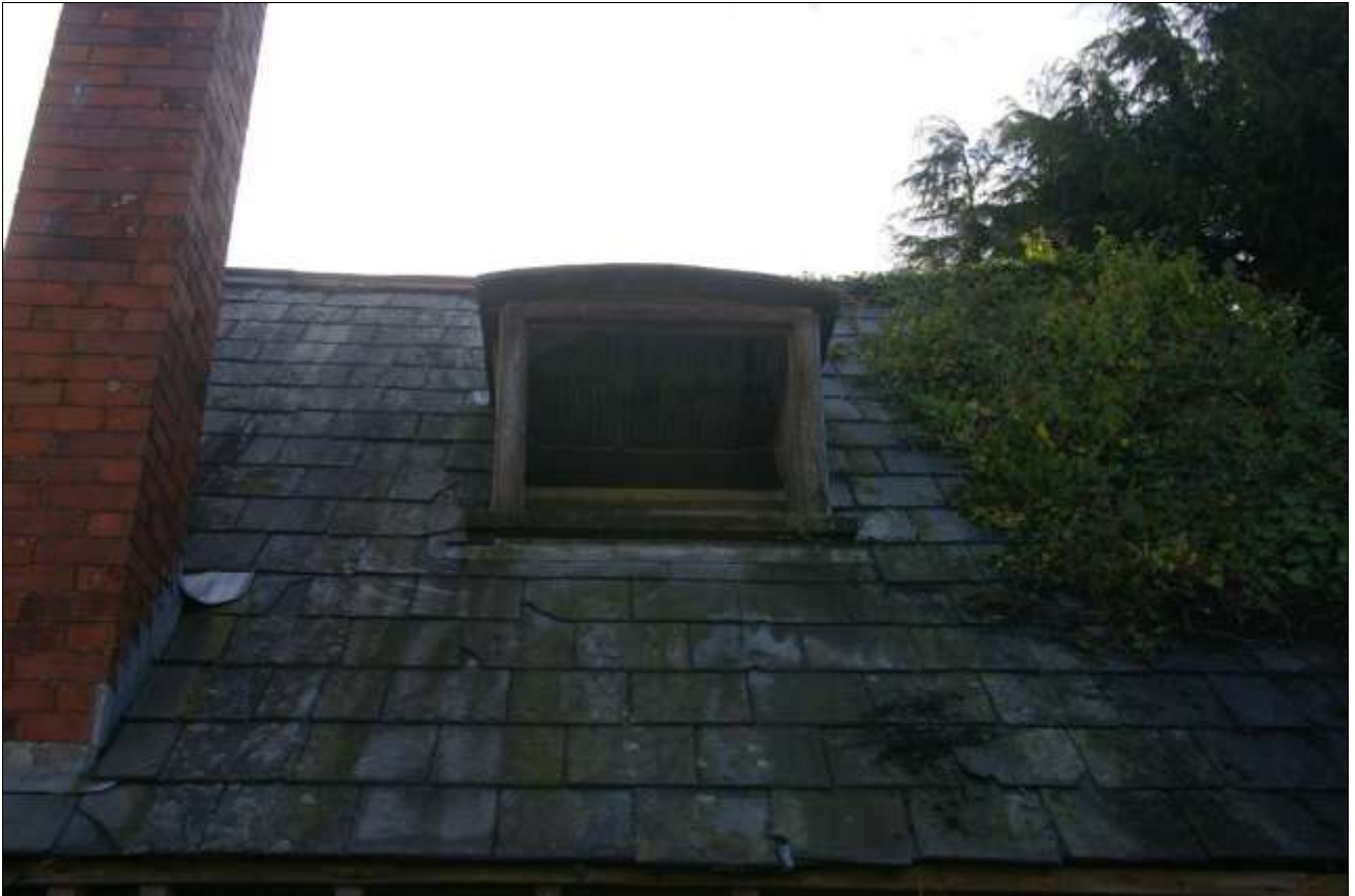
ROOF LIGHT IN NORTH ELEVATION, VIEWED FROM THE NORTH (NO SCALE).
