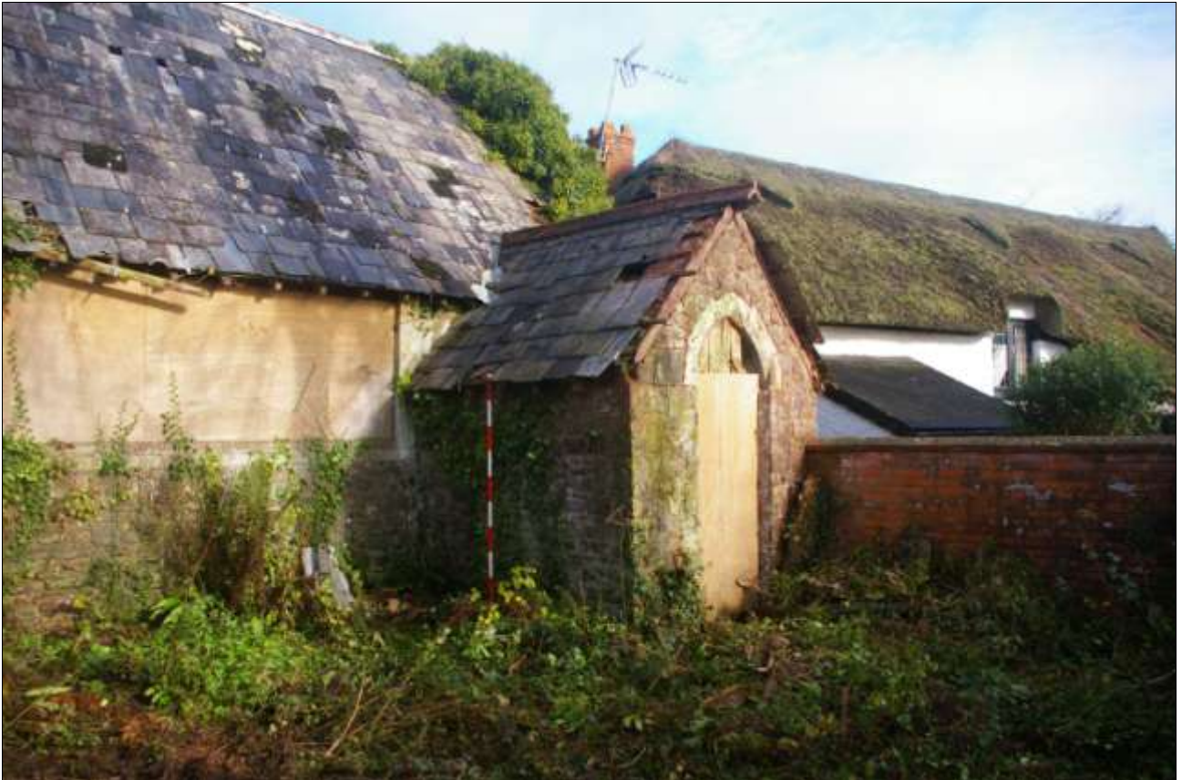
EASTERN PORCH ON SOUTHERN ELEVATION, VIEWED FROM THE SOUTH-WEST (2M SCALE).
