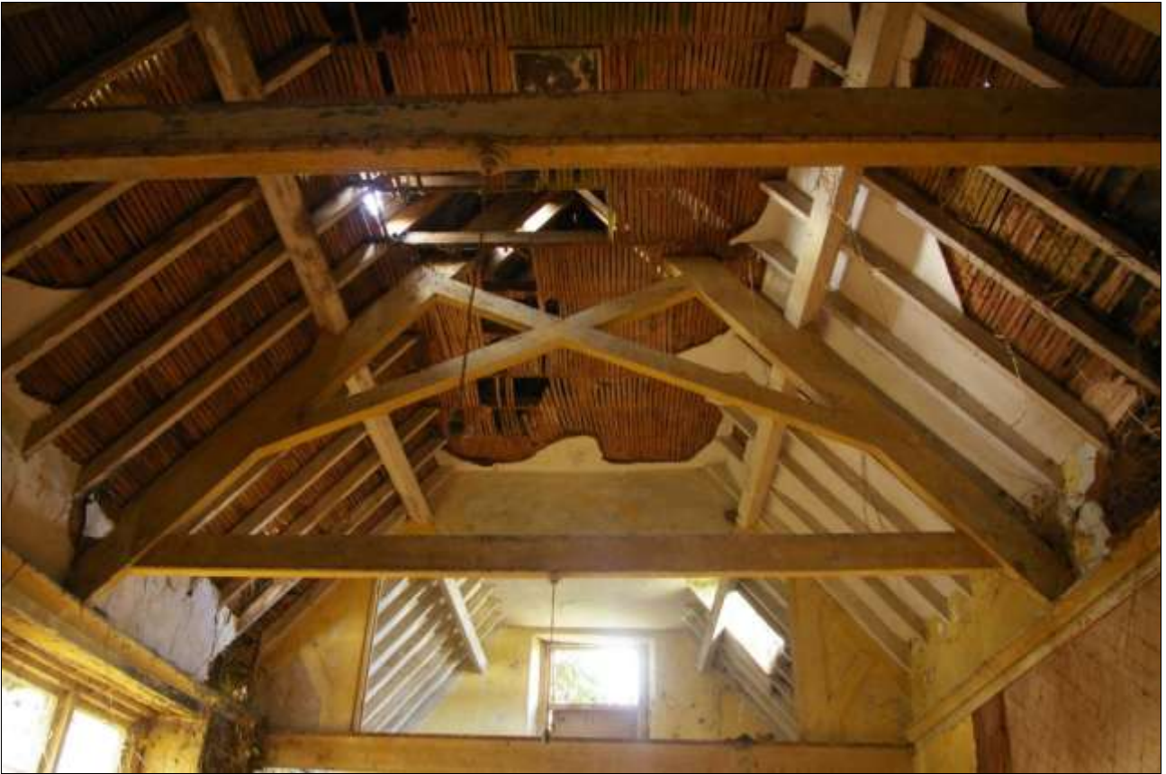
SHOT OF ROOF TIMBERS VIEWED FROM THE EAST (NO SCALE).
