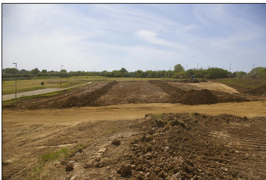
FIGURE 5: SITE SHOT, POST-EXCAVATION; VIEWED FROM THE NORTH-EAST (NO SCALE).
