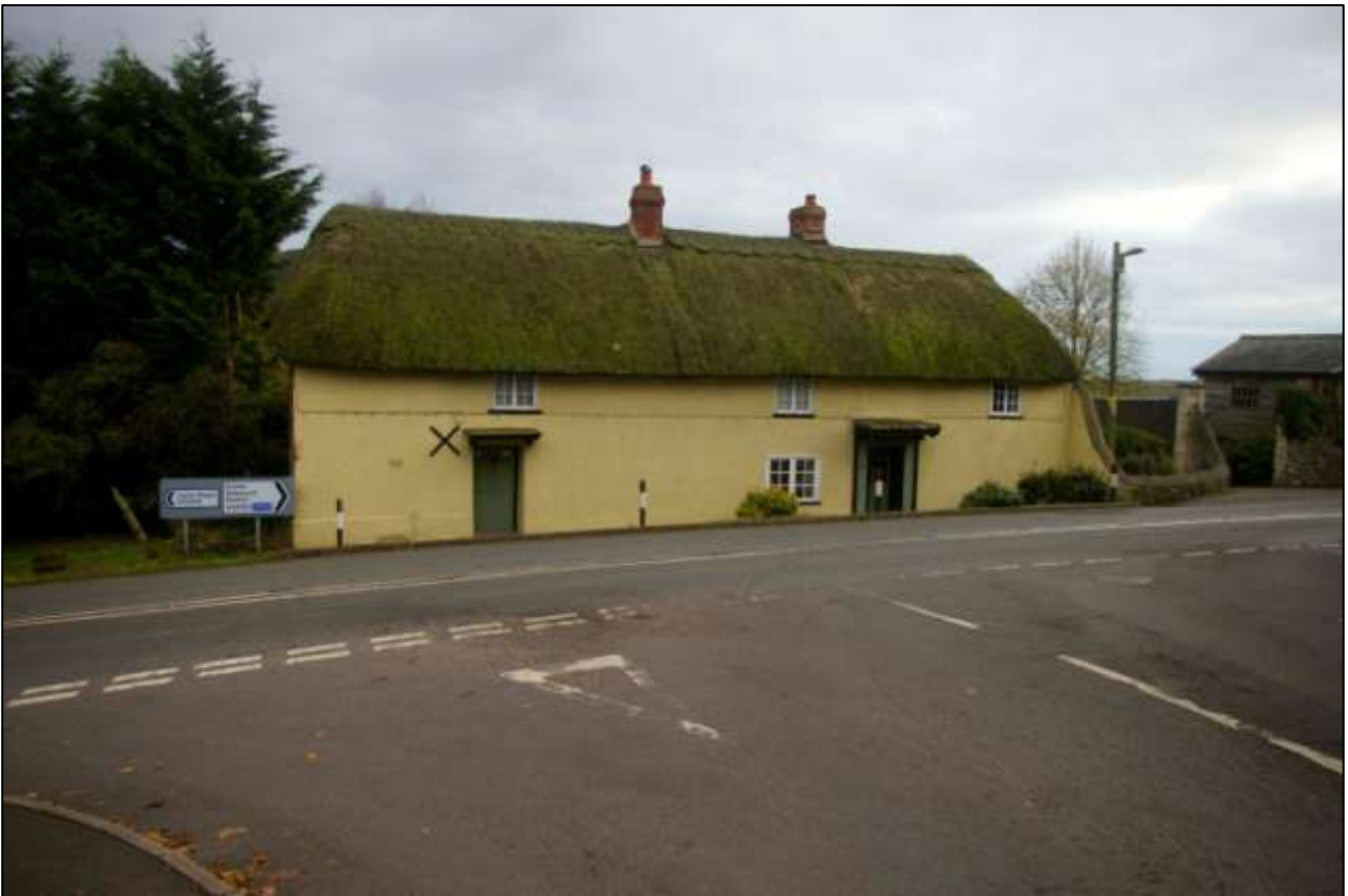
SHIP HOUSE; VIEWED FROM THE NORTH.
