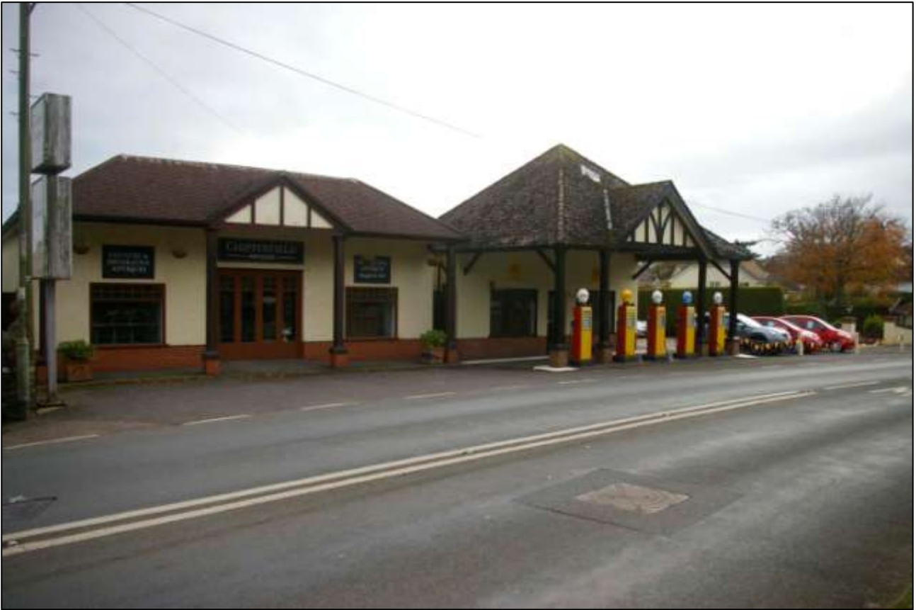
COLYFORD FILLING STATION; VIEWED FROM THE NORTH-EAST.
