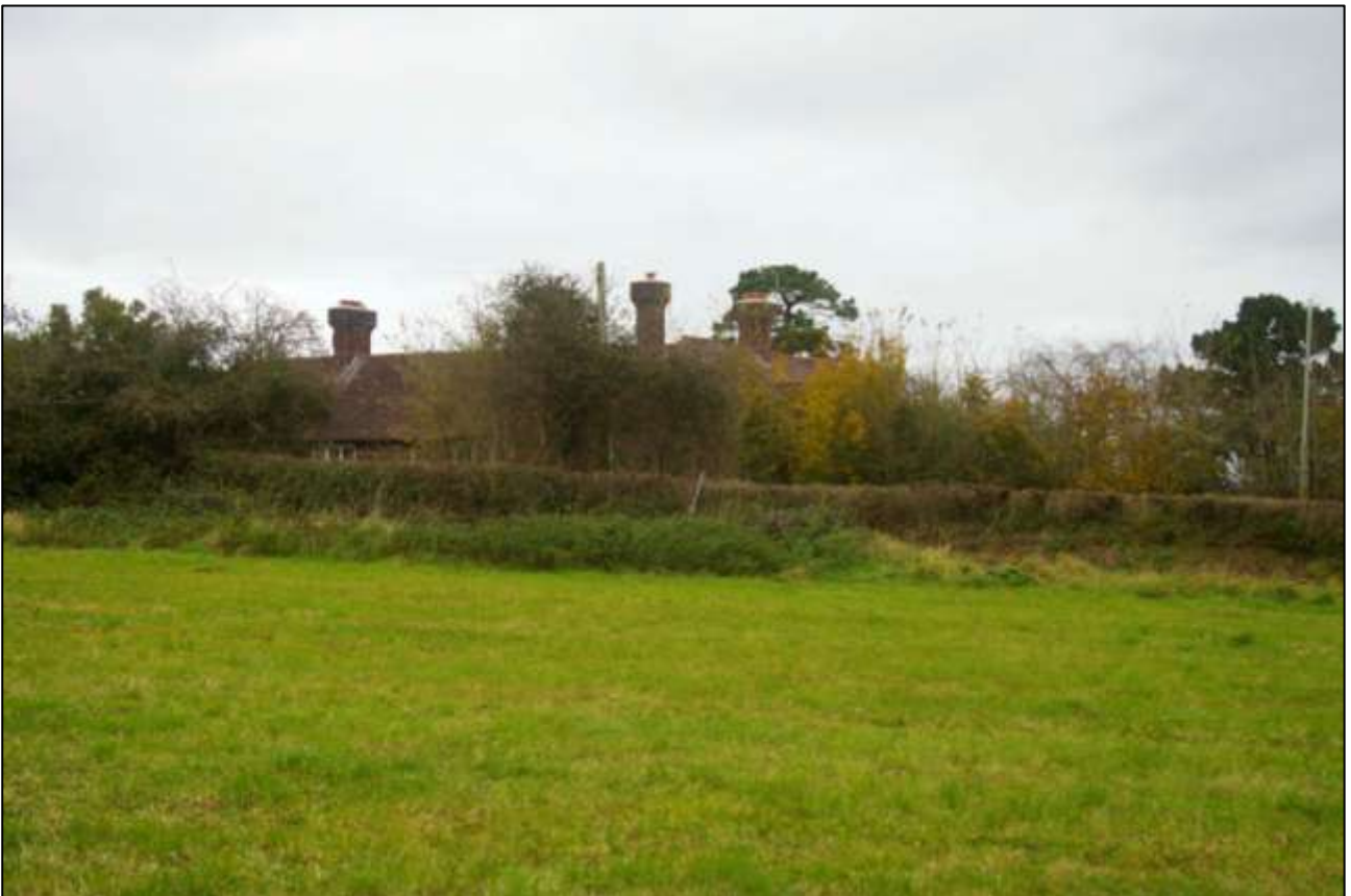
DEBRIS AND OVERGROWN AREA AT THE CENTRE OF THE NORTH-EASTERN EDGE OF THE SITE; VIEWED FROM THE SOUTH-WEST.
