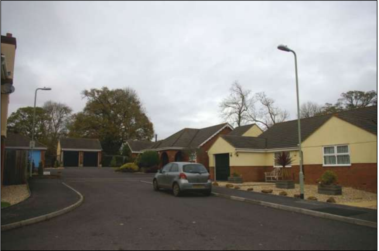
VIEW AT THE END OF OLD MANOR GARDENS LOOKING TOWARDS THE SITE; VIEWED FROM THE SOUTH-WEST.
