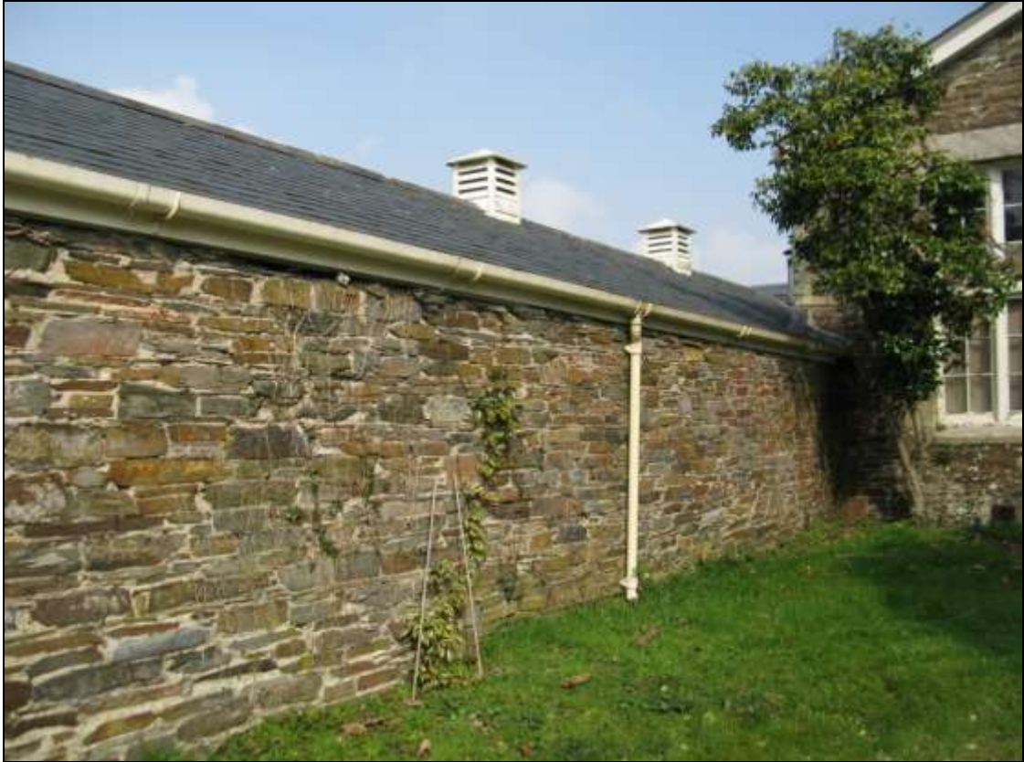
The east elevation of the east range; from the south-east
