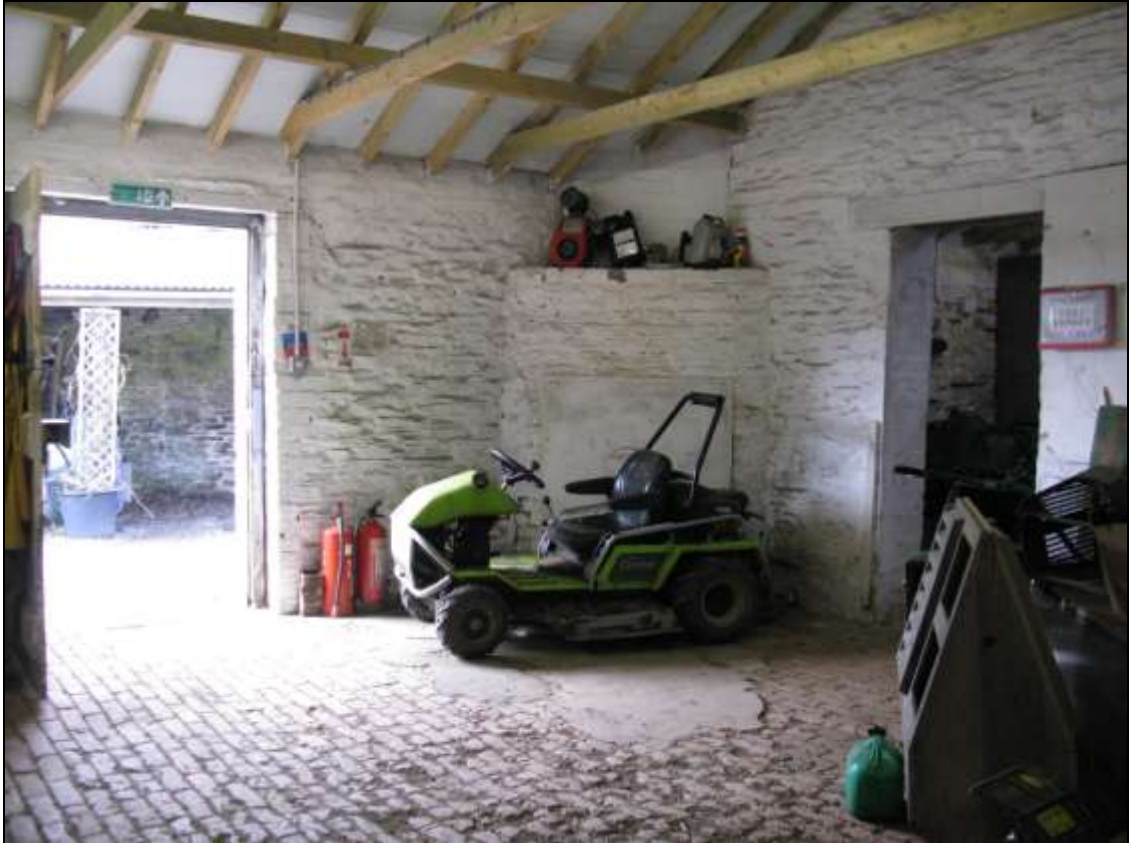
The brick-built hearth in the south-west corner of the east range; from the north-east
