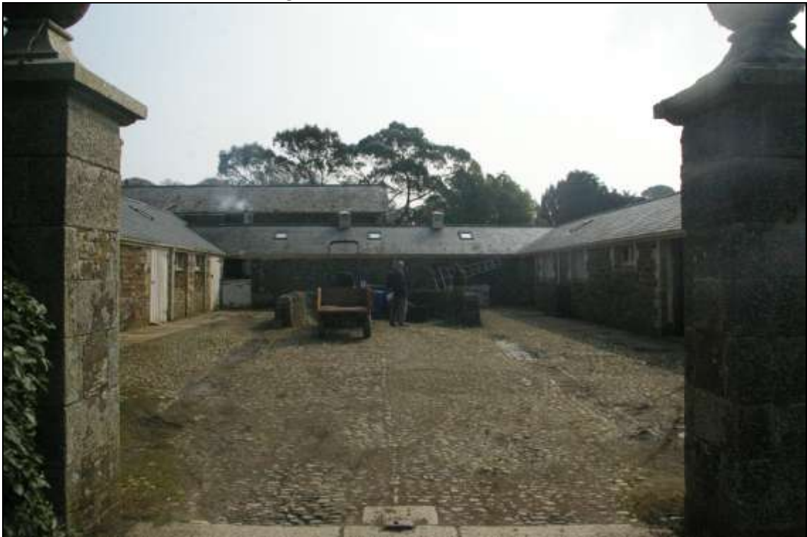
View of the former slaughter yard; from the west
