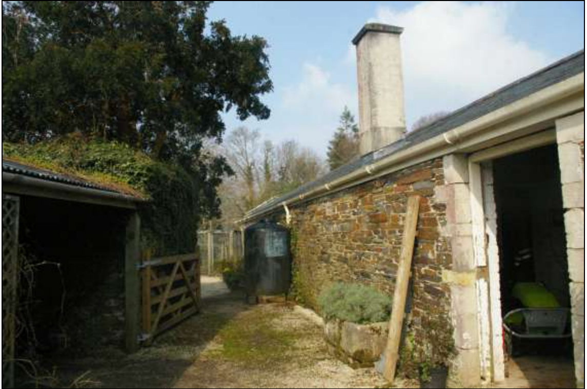
The south elevation of the south range; from the east.
