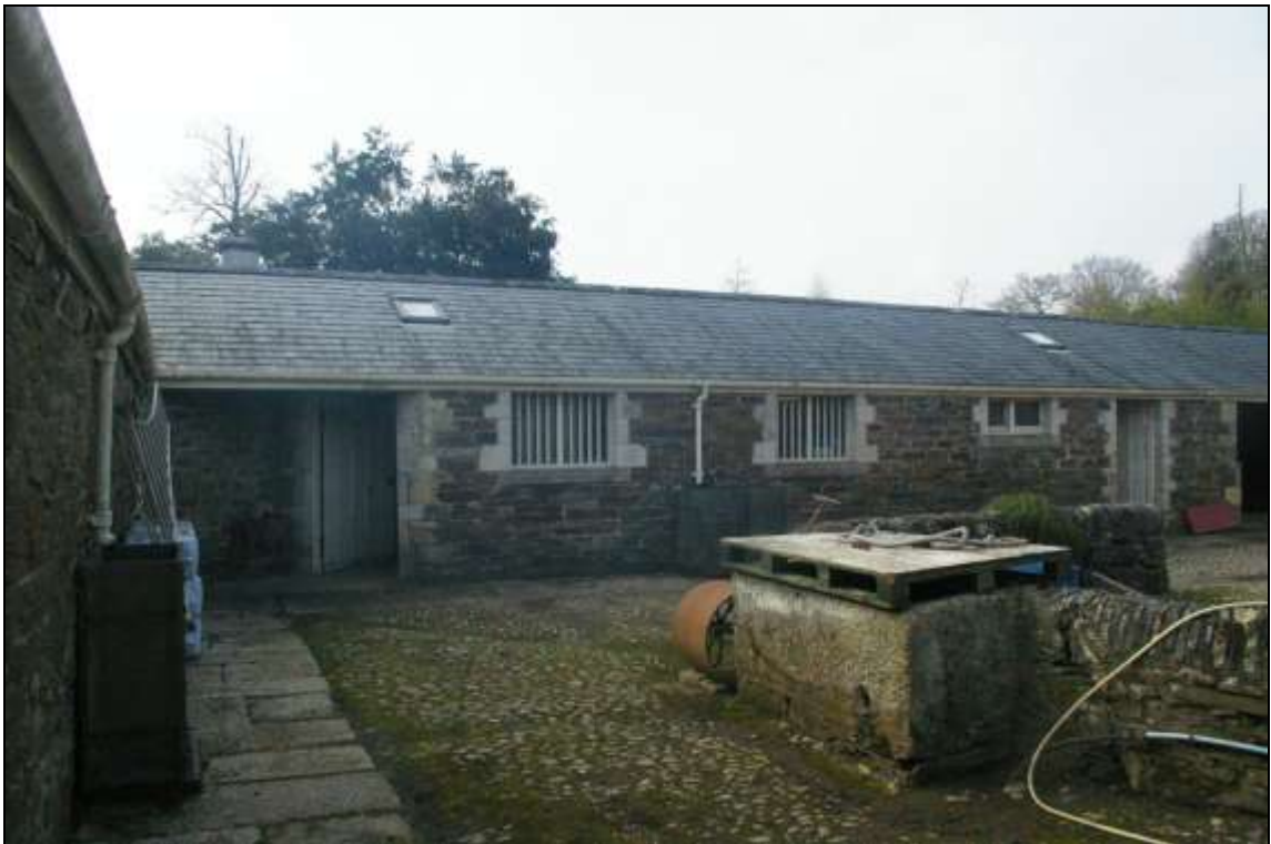
The north elevation of the south range, within the former slaughter yard, at the eastern end; from the north-east
