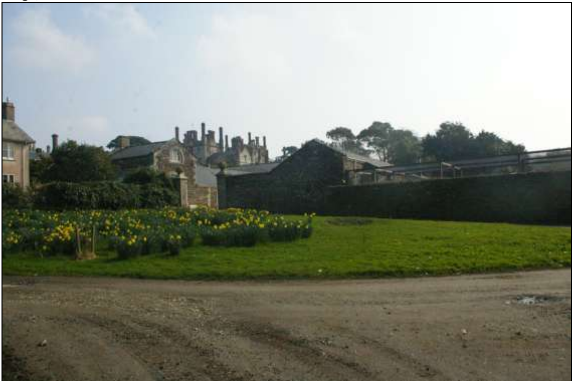
View to Tregothnan House, over the service yards; from the south-west
