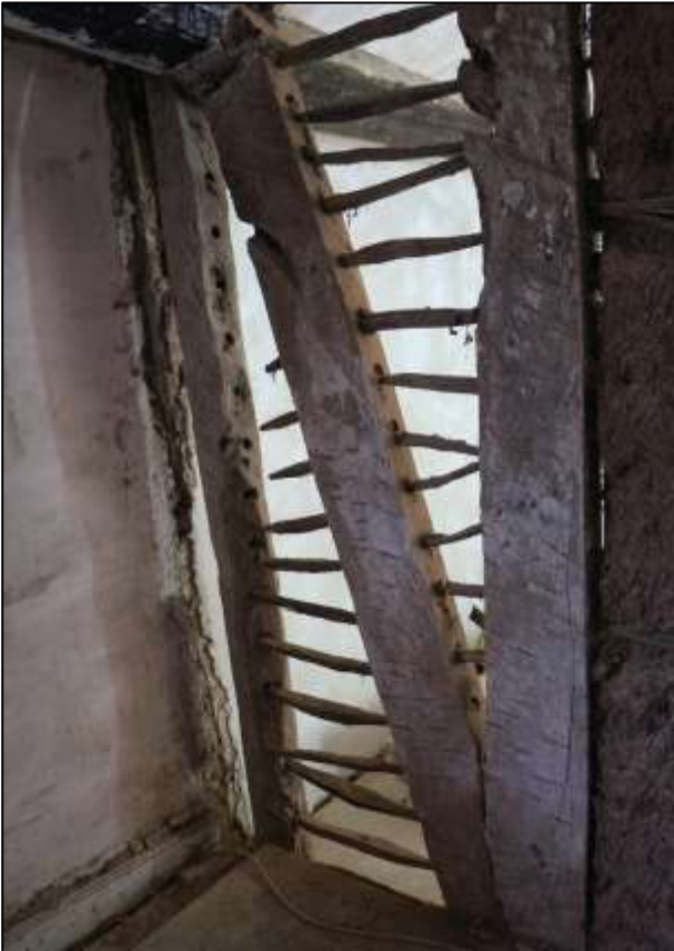
105. LEFT: AS ABOVE; DETAIL OF THE SHAPED PEGS.
