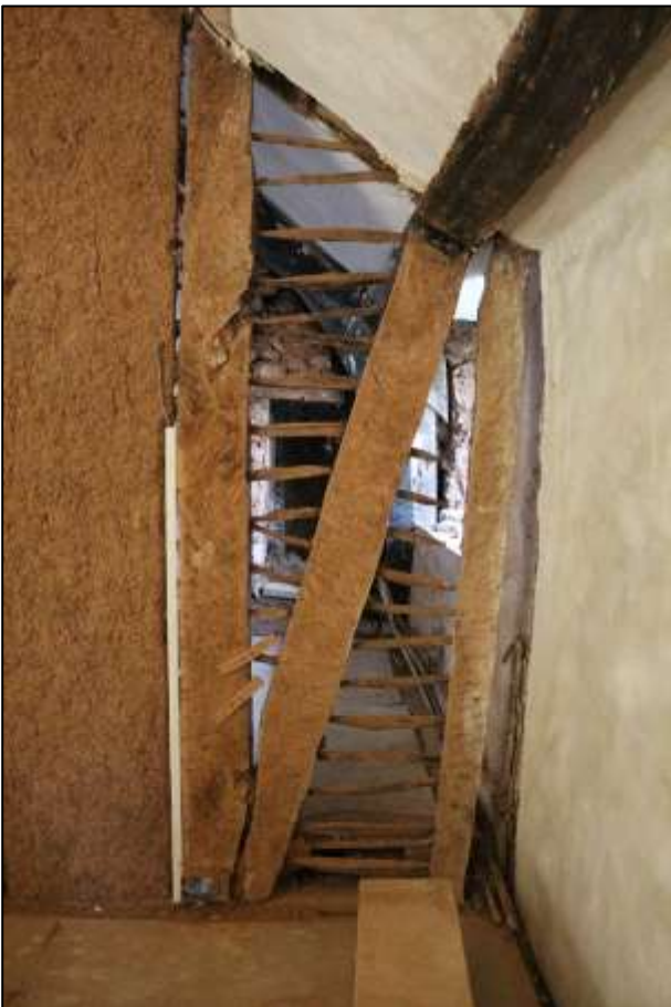
103. LEFT: AS ABOVE; DETAIL OF THE EXPOSED PEGS WITHIN THE COB PANELS. VIEWED FROM THE SOUTH-EAST.
