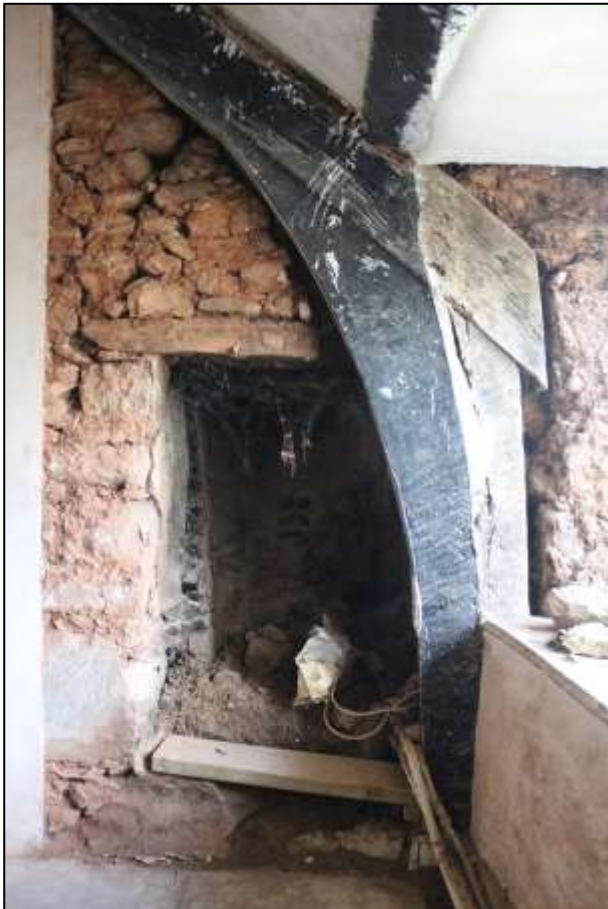
LEFT FIGURE 20: THE JOINTED CRUCK (CRUCK2) NEXT TO THE AXIAL STACK AND REVEALED ALCOVE; VIEWED FROM THE SOUTH-EAST. RIGHT FIGURE 21: THE STUD AND COB WALL SEPARATING R8 FROM R6, SHOWING THE LATH AND PLASTER INFILL; VIEWED FROM THE ENE.
