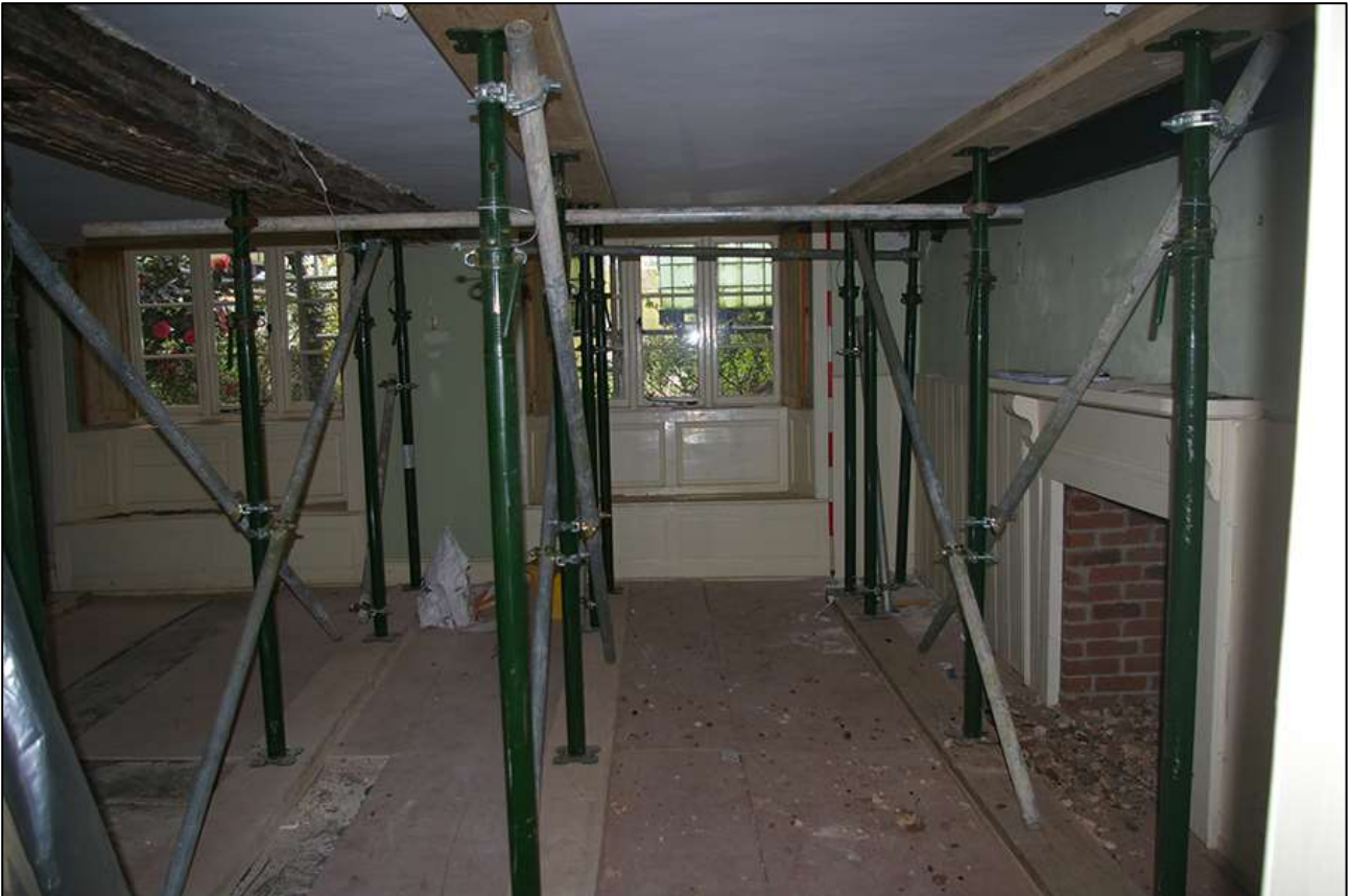
33. R2; VIEWED FROM THE SOUTH-WEST. SHOWING W2 AND W3 (SCALE 2M).
