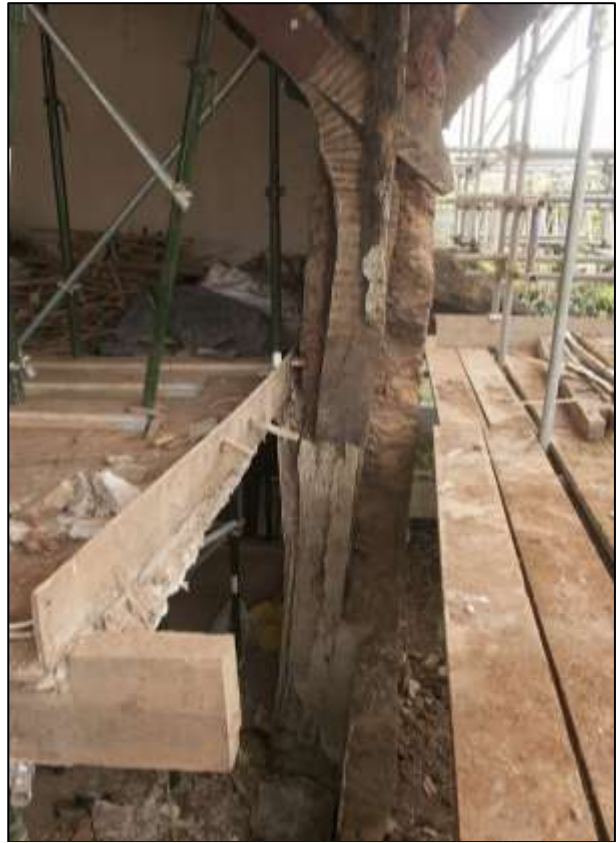
128. LEFT: R6; DETAIL OF THE FAILED JOINT IN THE RAISED CRUCK AND ITS CRUDE REPAIR. VIEWED FROM THE SSE.
