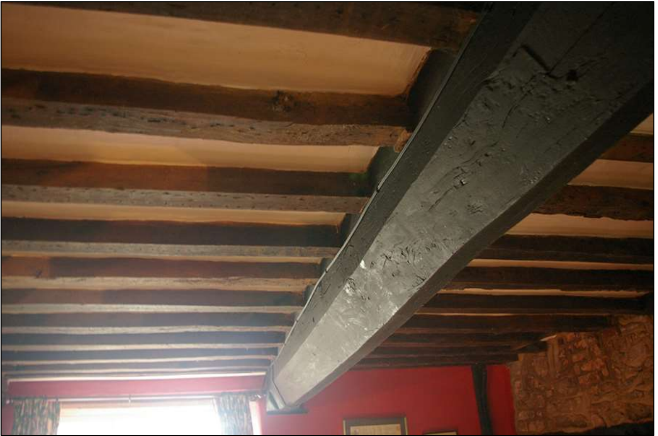
19. DETAIL OF THE CHAMFERED CEILING BEAM IN R10; VIEWED FROM THE SOUTH-WEST.
