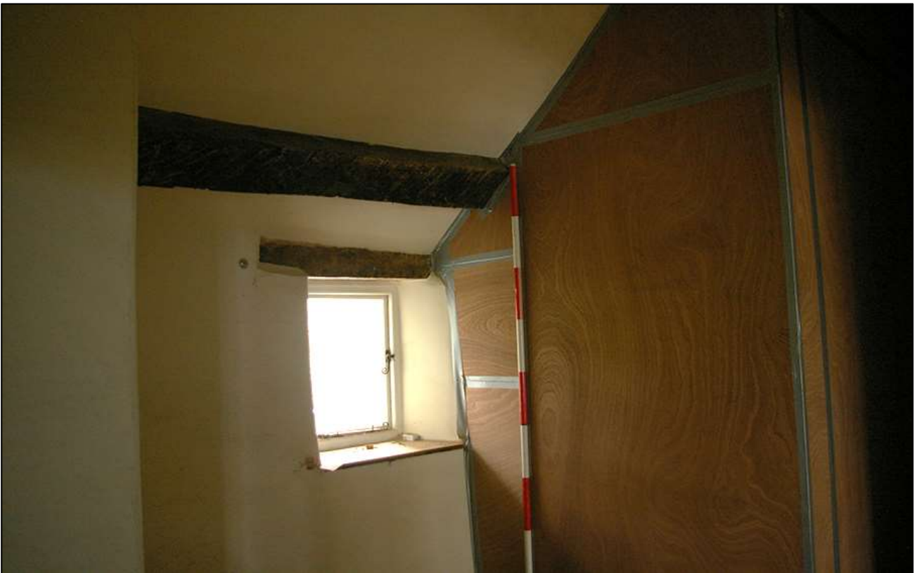
62. R7; SHOWING W9. VIEWED FROM THE EAST (SCALE 2M).
