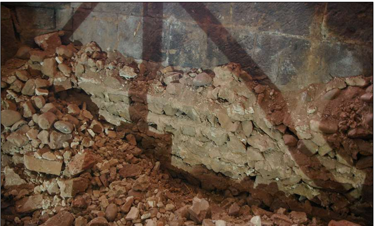
71. R2; DETAIL OF THE LOOSELY-MORTARED RIVER PEBBLES IN THE BACK OF THE 17 TH CENTURY HEARTH; VIEWED FROM THE WET-NORTH-WEST.
