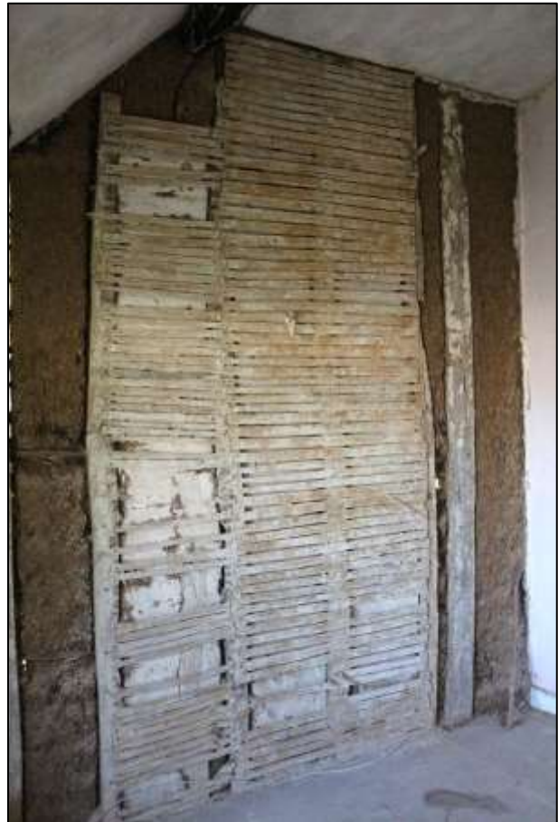
LEFT FIGURE 20: THE JOINTED CRUCK (CRUCK2) NEXT TO THE AXIAL STACK AND REVEALED ALCOVE; VIEWED FROM THE SOUTH-EAST. RIGHT FIGURE 21: THE STUD AND COB WALL SEPARATING R8 FROM R6, SHOWING THE LATH AND PLASTER INFILL; VIEWED FROM THE ENE.
