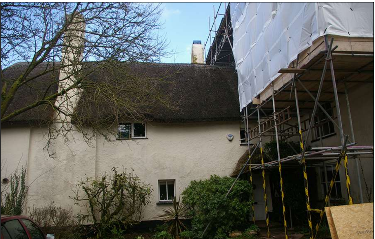
16. THE SOUTH-WEST ELEVATION OF THE MAIN RANGE; VIEWED FROM THE SOUTH-WEST.
