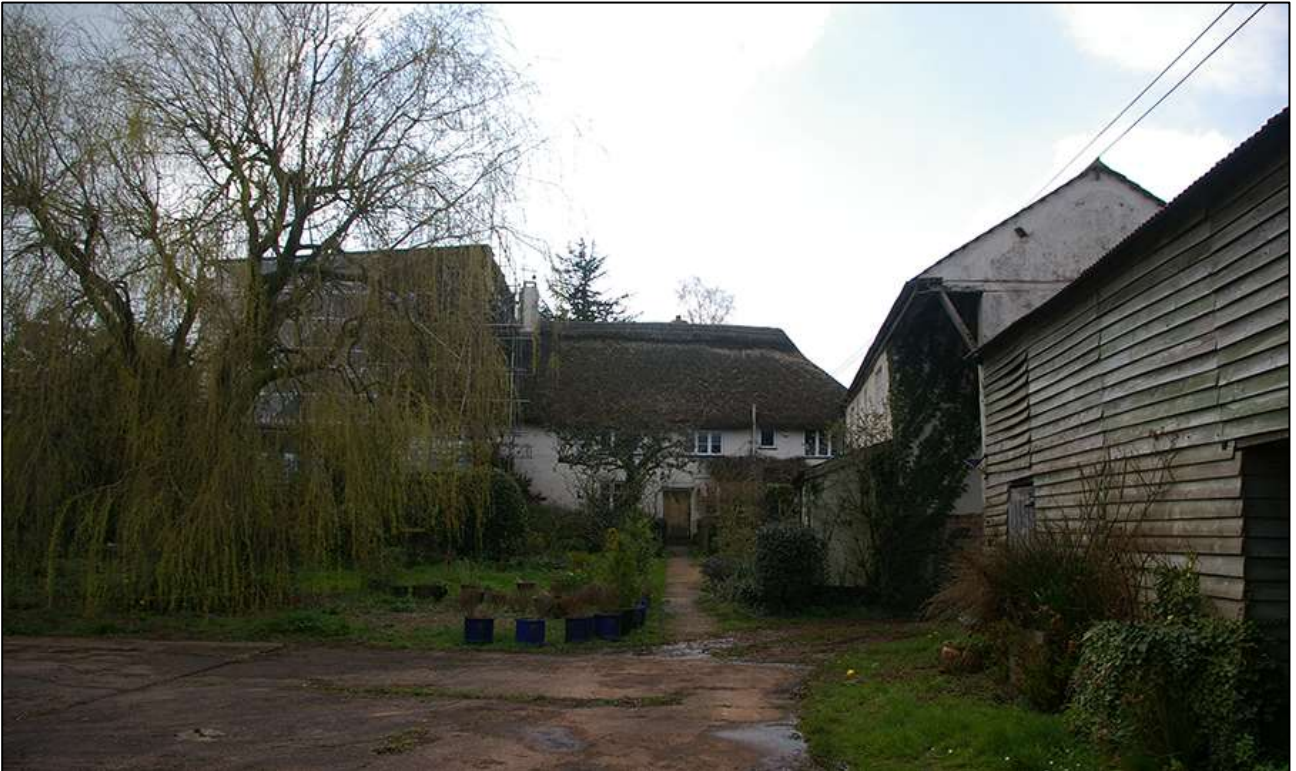
1. THE NORTH-EAST ELEVATION OF THE HOUSE; VIEWED FROM THE YARD.
