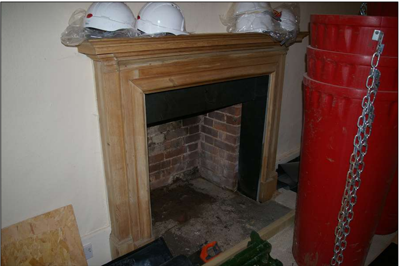
22. R1; DETAIL OF FP1. VIEWED FROM THE NORTH.
