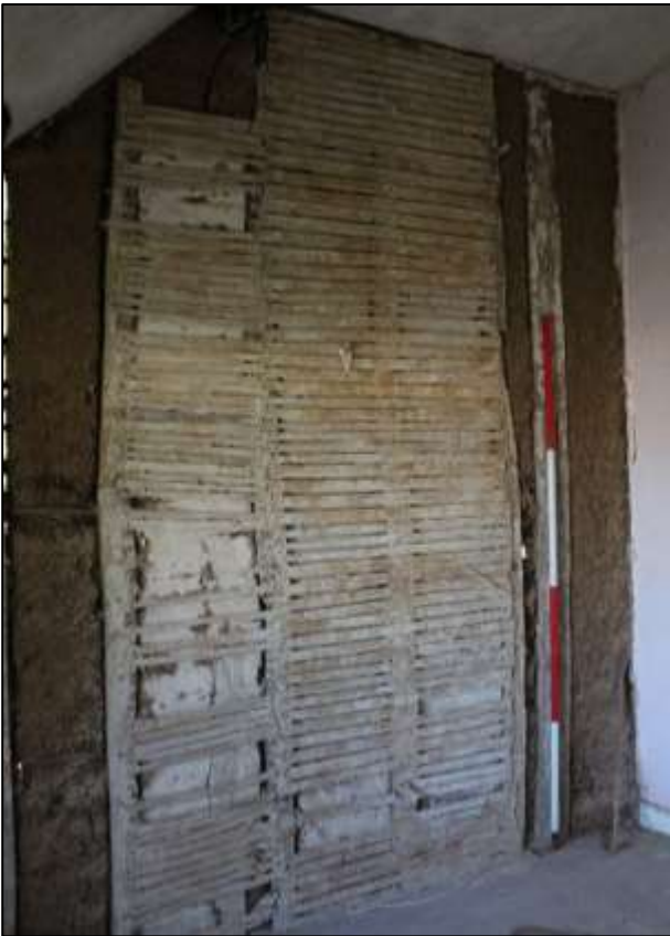
107. LEFT: R8; THE PARTY WALL WITH R6. DETAIL OF THE LATH AND PLASTER INFILL. VIEWED FROM THE NORTH (SCALE 2M).
