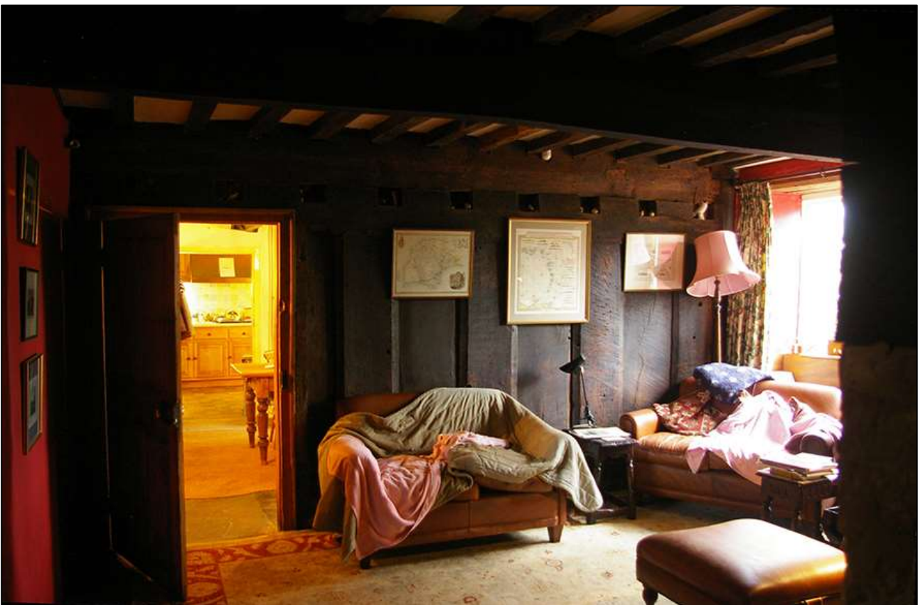
20. THE MEDIEVAL SCREEN IN R10; VIEWED FROM THE SOUTH. NOTE THE JOIST SOCKETS BELOW THE BEAM CARRYING THE JOISTS.
