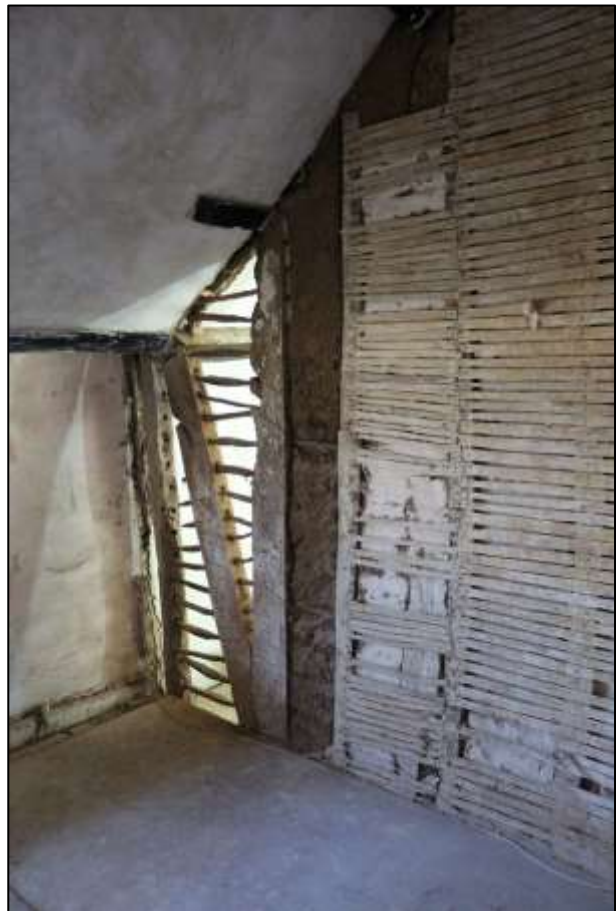
103. LEFT: AS ABOVE; DETAIL OF THE EXPOSED PEGS WITHIN THE COB PANELS. VIEWED FROM THE SOUTH-EAST.
