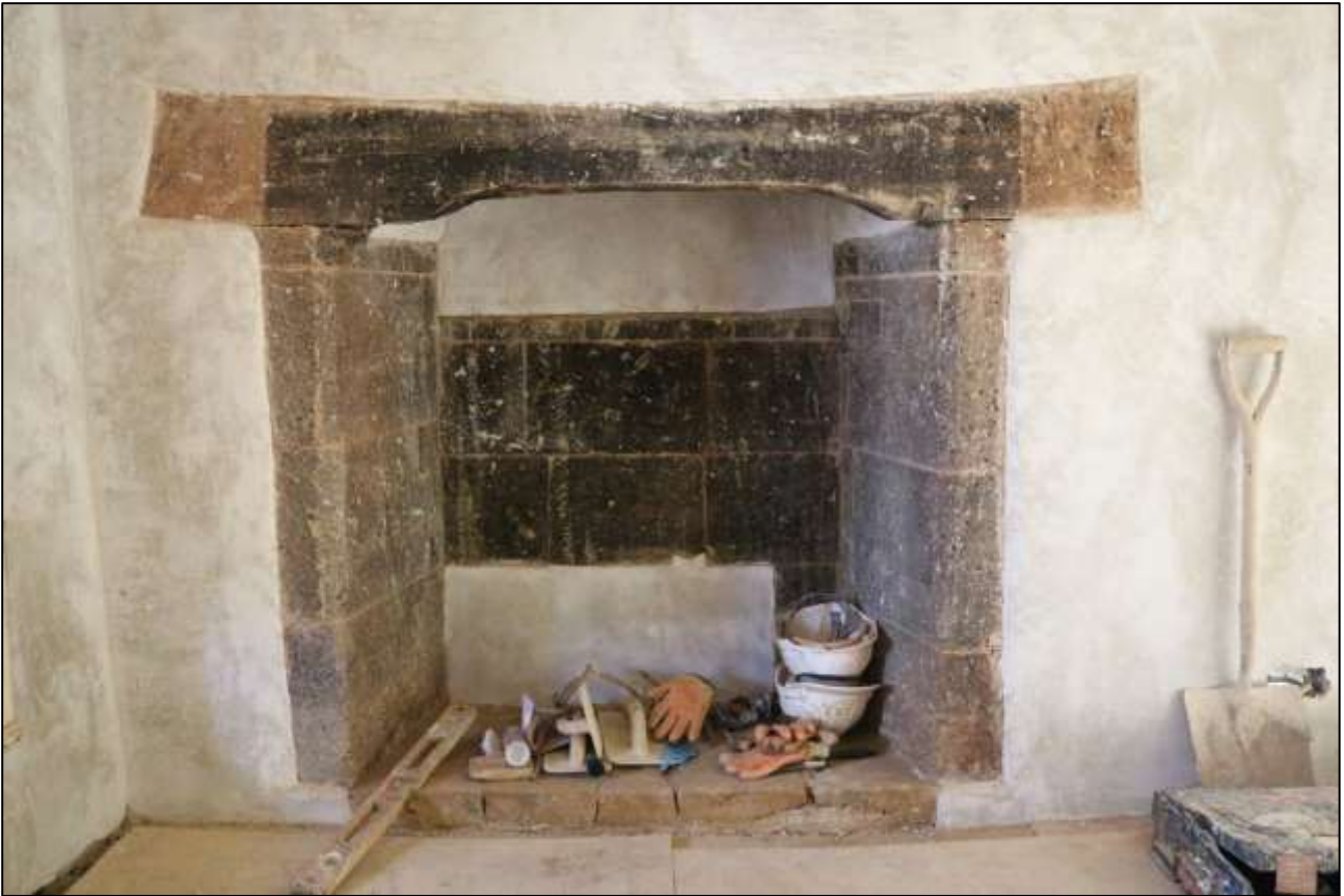
137. AS ABOVE; DETAIL OF THE RESTORED FP4.
