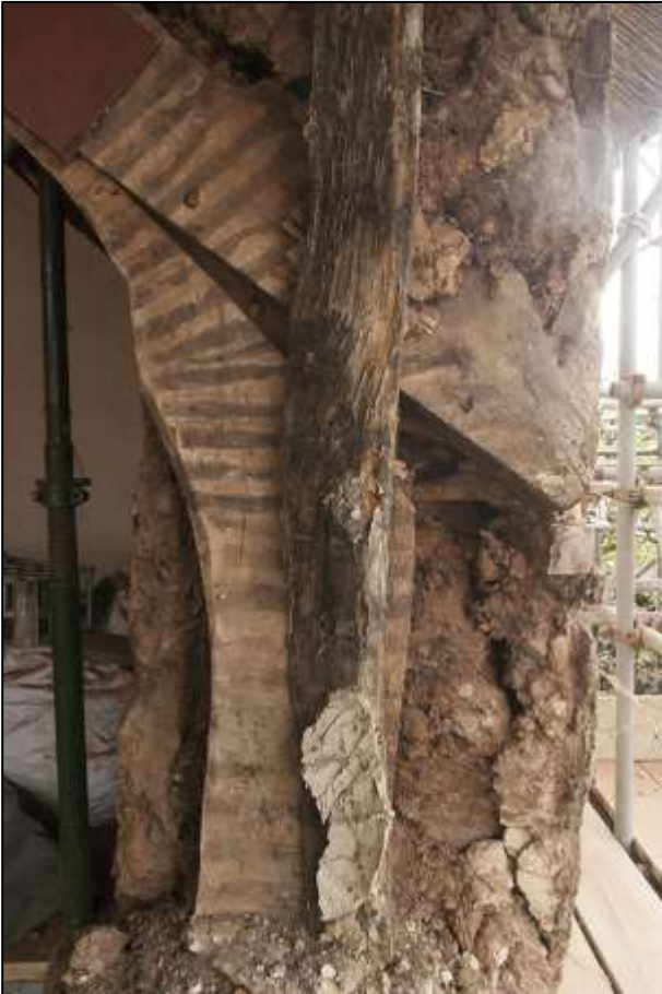
LEFT FIGURE 15: THE FAILED JOINT IN THE 17 TH CENTURY JOINTED CRUCK; VIEWED FROM THE SOUTH-EAST.
