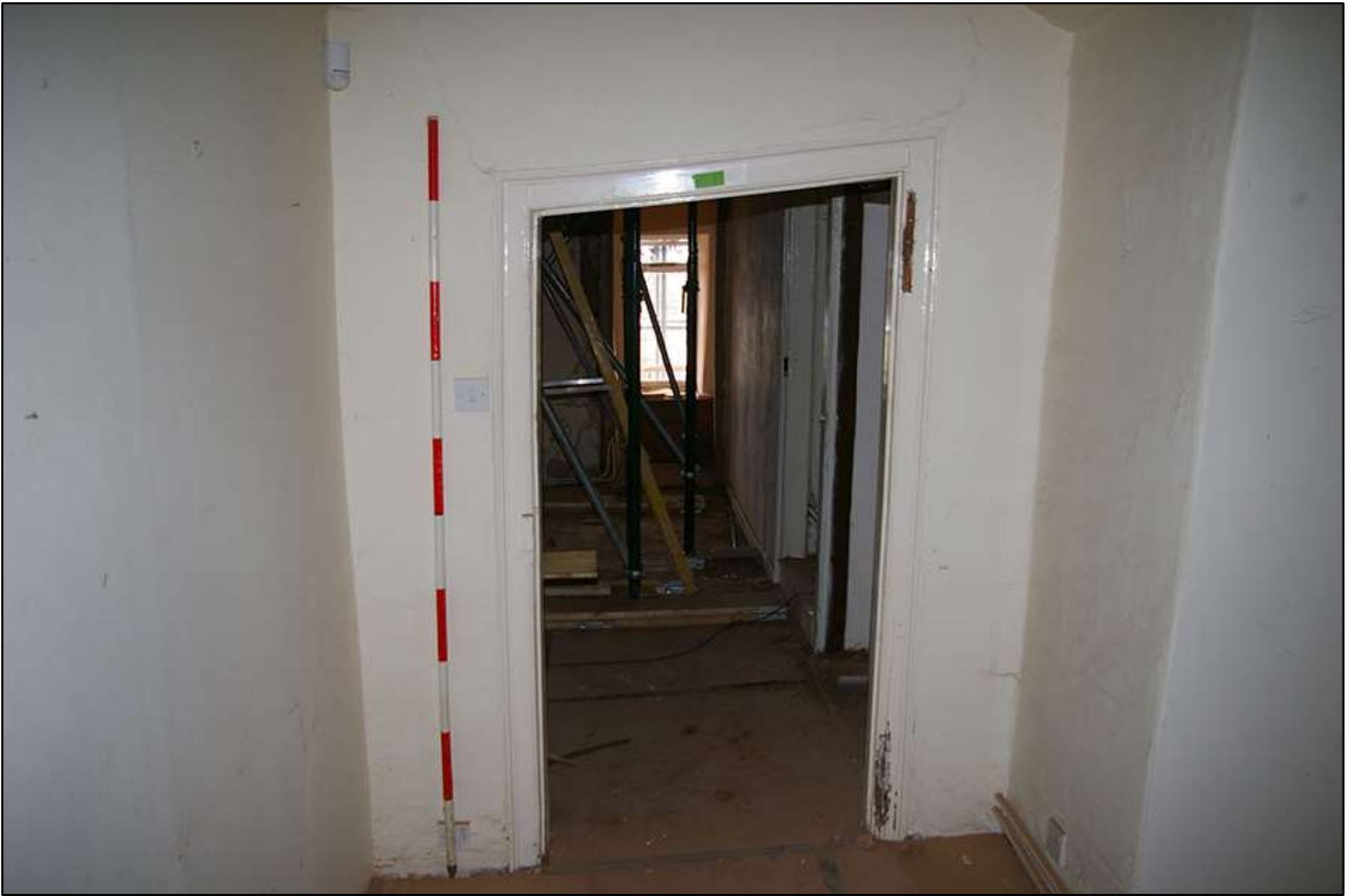
58. R7; SHOWING THE DISTORTED ANGLE OF D9. VIEWED FROM THE NORTHWEST (SCALE 2M).
