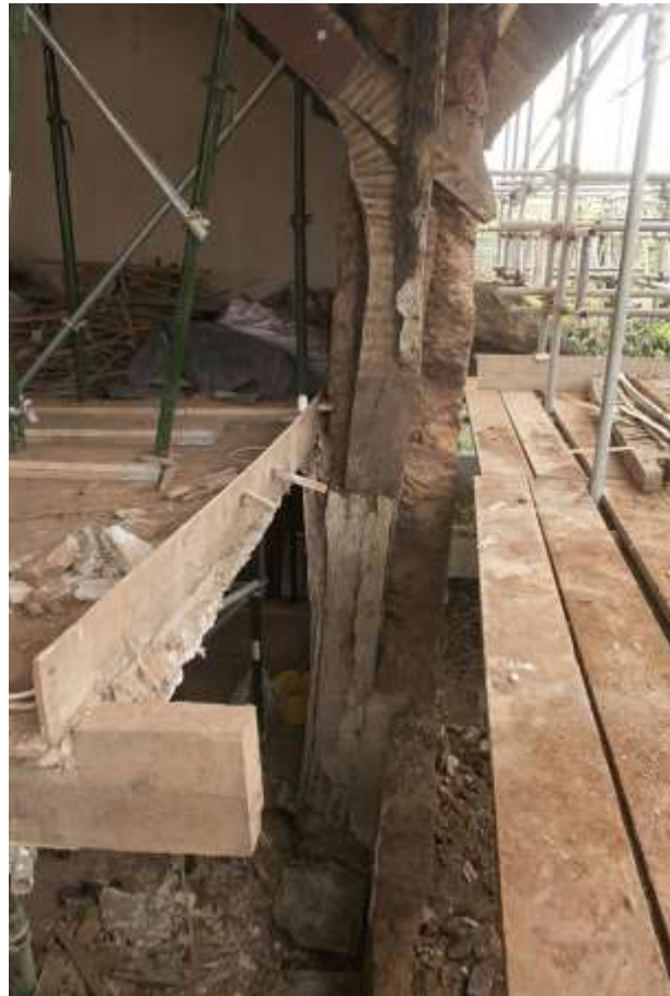
LEFT FIGURE 15: THE FAILED JOINT IN THE 17 TH CENTURY JOINTED CRUCK; VIEWED FROM THE SOUTH-EAST.
