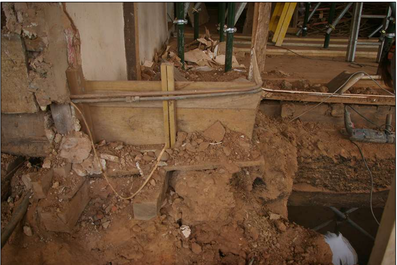
101. AS ABOVE; VIEWED FROM THE SOUTH-EAST.
