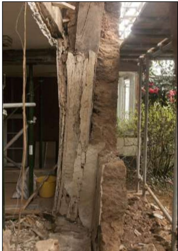
129. RIGHT: R2/R6; DETAIL OF THE CRUCK POST EMBEDDED IN THE EXTERNAL WALL. VIEWED FROM THE SOUTH-EAST.
