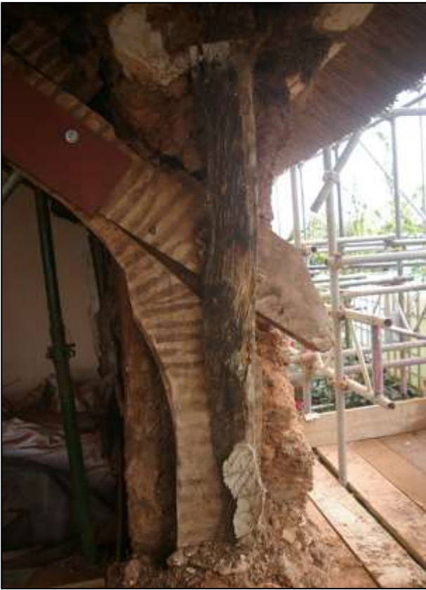
128. LEFT: R6; DETAIL OF THE FAILED JOINT IN THE RAISED CRUCK AND ITS CRUDE REPAIR. VIEWED FROM THE SSE.
