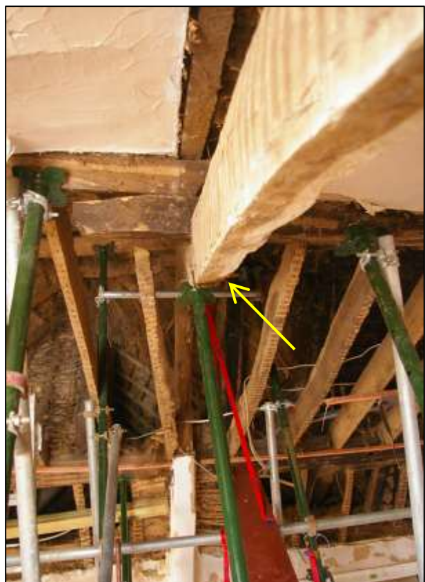
110. LEFT: R6; THE BROKEN JOINT IN THE RAISED CRUCK TRUSS NEXT TO W8; VIEWED FROM THE SOUTH-EAST.
