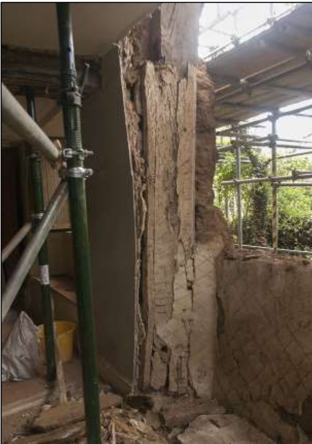
130. LEFT: R6; THE BASE OF THE CRUCK POST. VIEWED FROM THE SOUTH.
