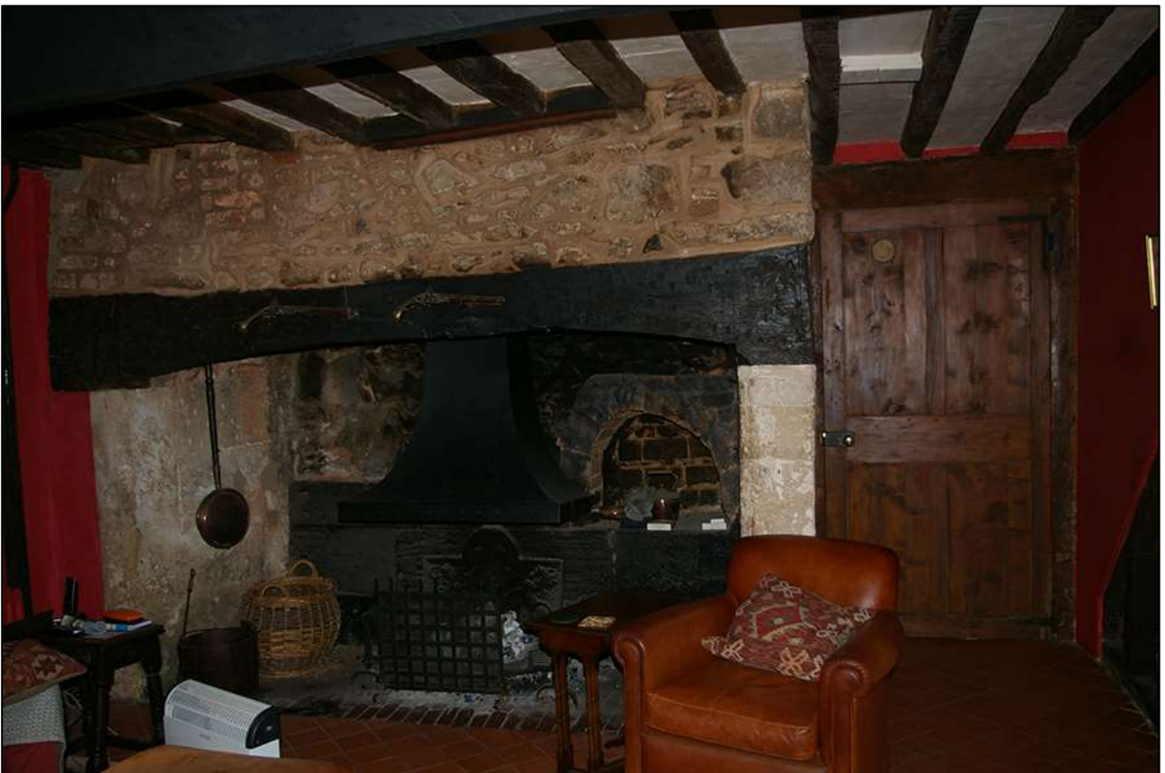
18. THE 17 TH CENTURY AXIAL STACK IN R10; VIEWED FROM THE NORTH-WEST.
