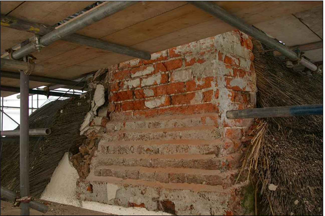
9. THE 18 TH CENTURY BRICK STACK ABOVE FP2/FP4; VIEWED FROM THE EAST-SOUTH-EAST.
