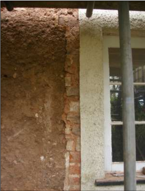
89. LEFT: THE NORTH-EAST ELEVATION, SHOWING THE BRICK INFILL AROUND W2; VIEWED FROM THE NORTH-EAST.
