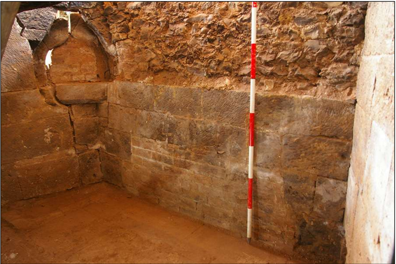
76. AS ABOVE; VIEWED FROM THE WEST-NORTH-WEST (SCALE 2M).
