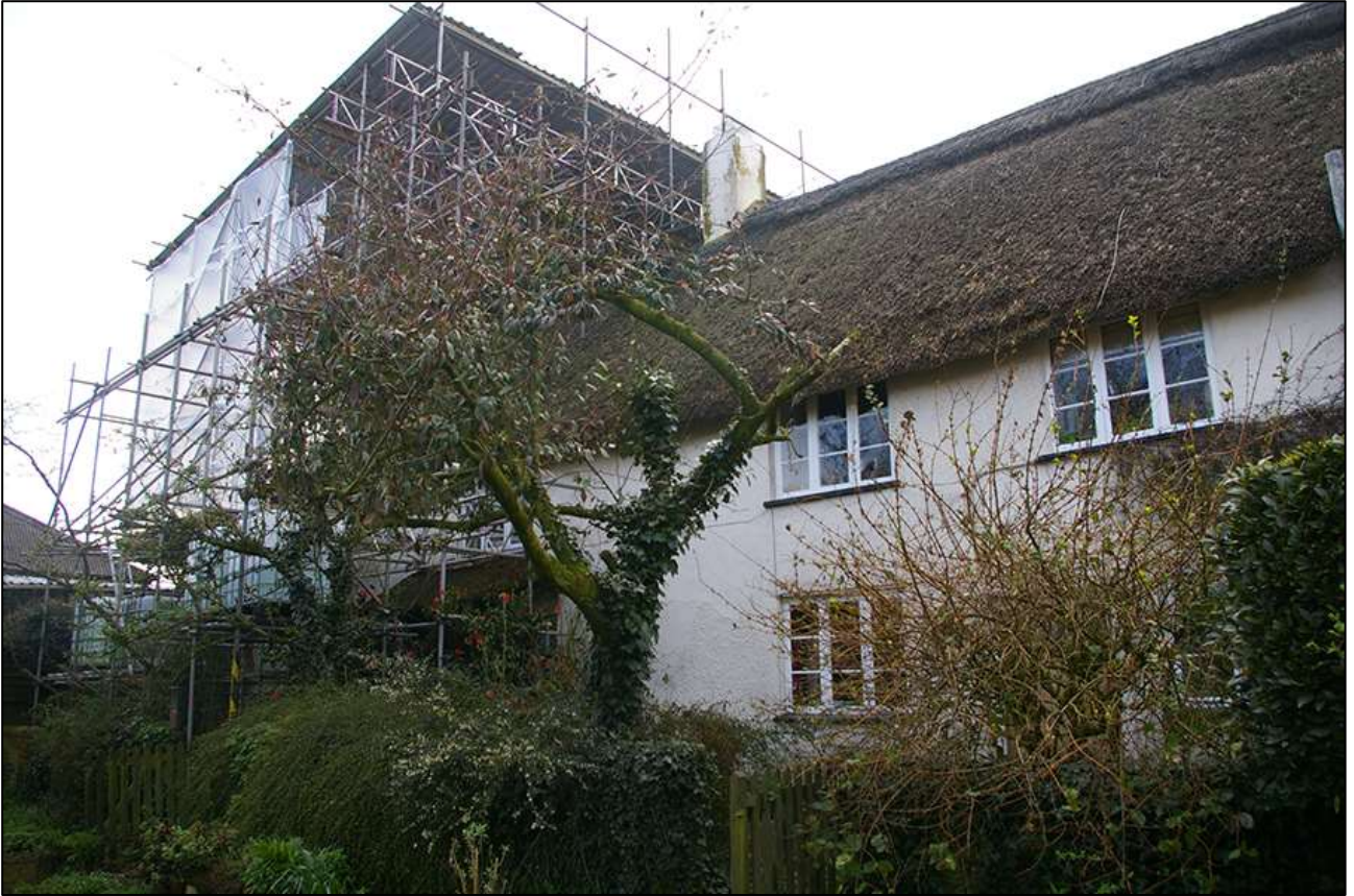
3. AS ABOVE; VIEWED FROM THE NORTH-NORTH-EAST.
