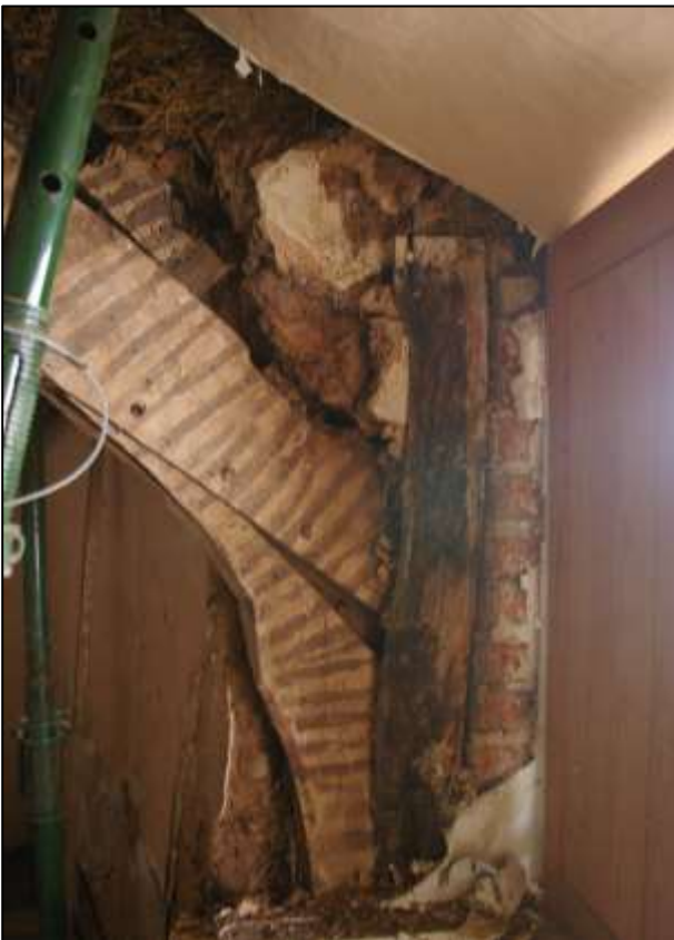
110. LEFT: R6; THE BROKEN JOINT IN THE RAISED CRUCK TRUSS NEXT TO W8; VIEWED FROM THE SOUTH-EAST.
