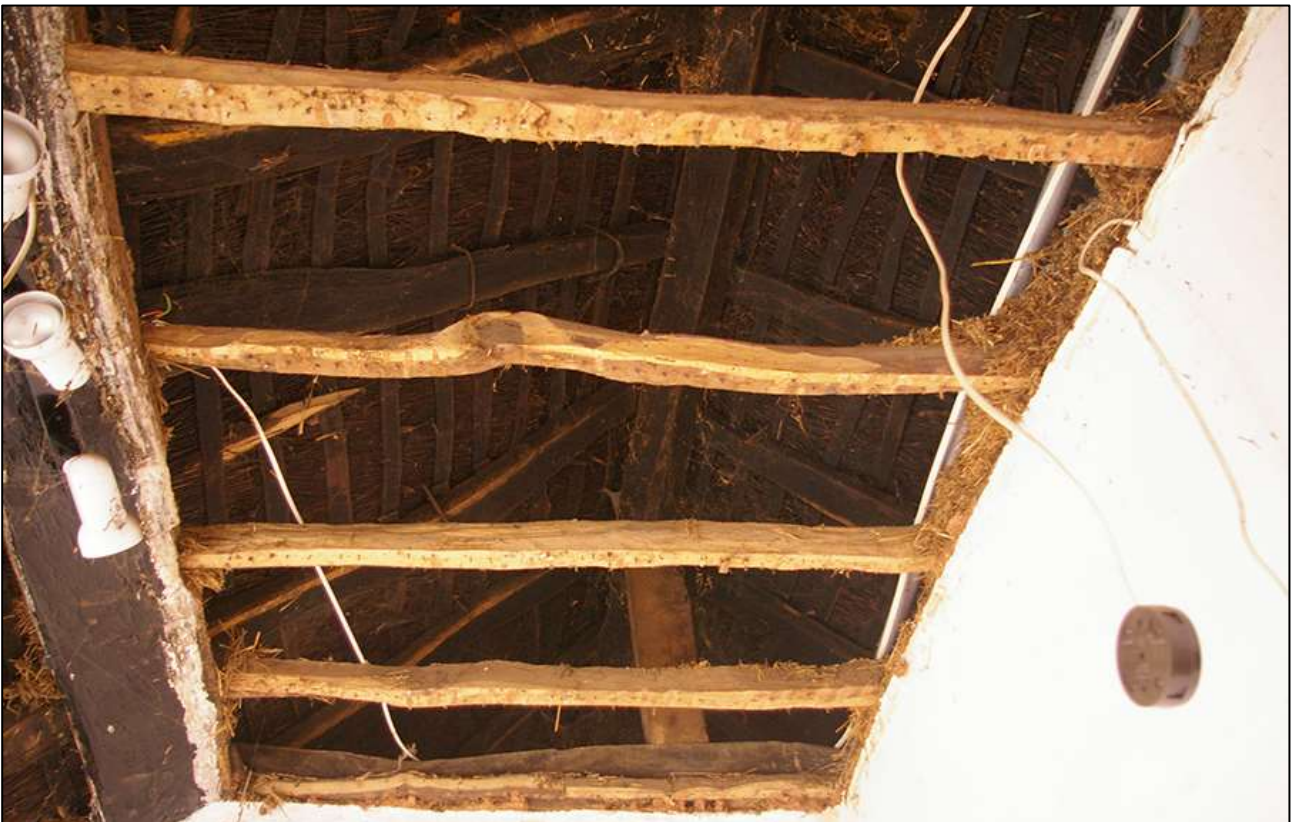
127. R8; THE MEDIEVAL ROOF ABOVE CEILING LEVEL. VIEWED FROM THE NORTH.
