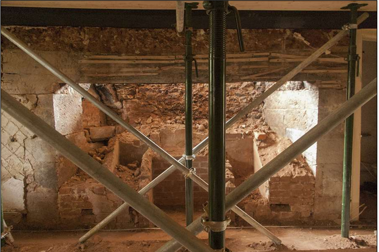
68. AS ABOVE; AS THE BLOCKING MATERIAL IS REMOVED.
