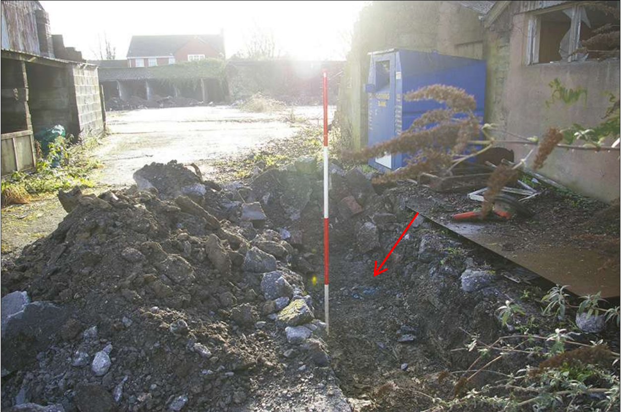
TRENCH 2, BLUE TAPE VISIBLE OVER ELECTRIC CABLE (INDICATED), SEALED FUEL TANK AT FAR EDGE; VIEWED FROM THE NORTH-EAST (2M SCALE).
