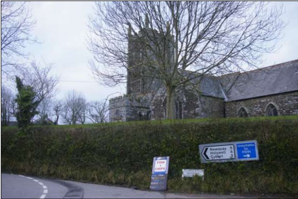
VIEW OF THE CHURCH OF ST. NEWLYNA; VIEWED FROM THE EAST-SOUTH-EAST.
