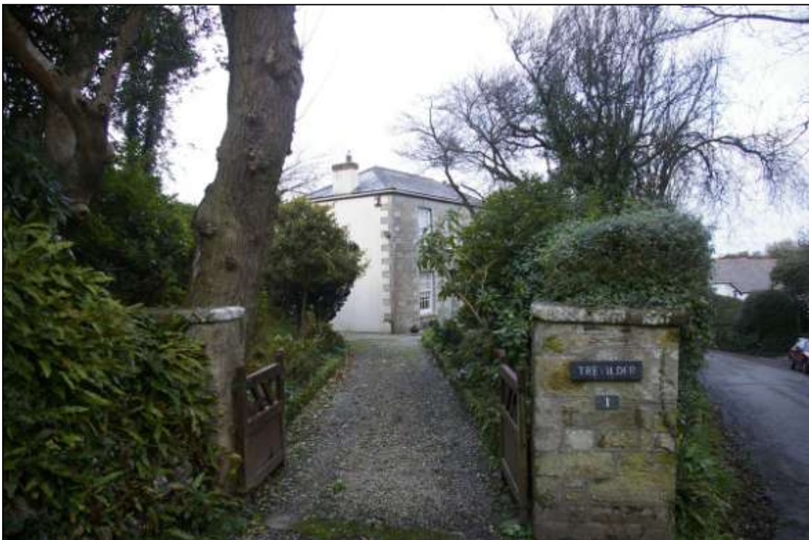
VIEW OF BUSHMEAD HOUSE; VIEWED FROM THE SOUTH.
