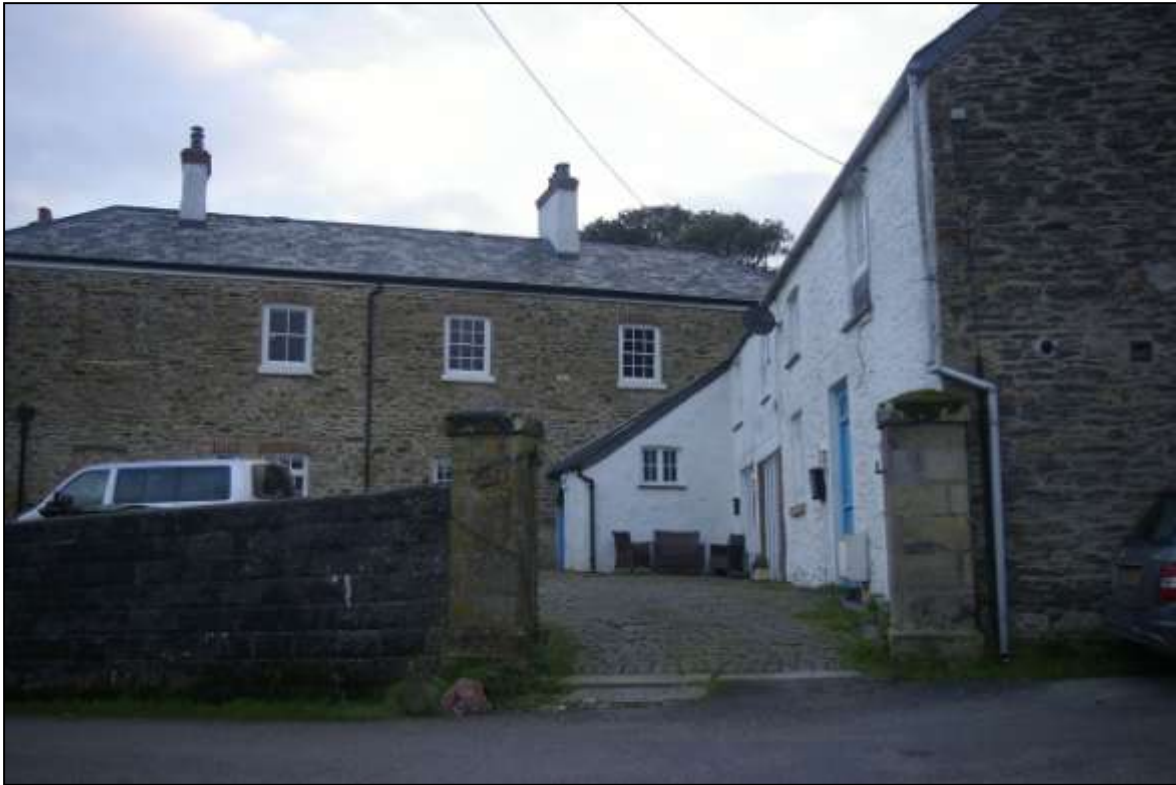
VIEW OF THE OLD VICARAGE; VIEWED FROM THE NORTH.
