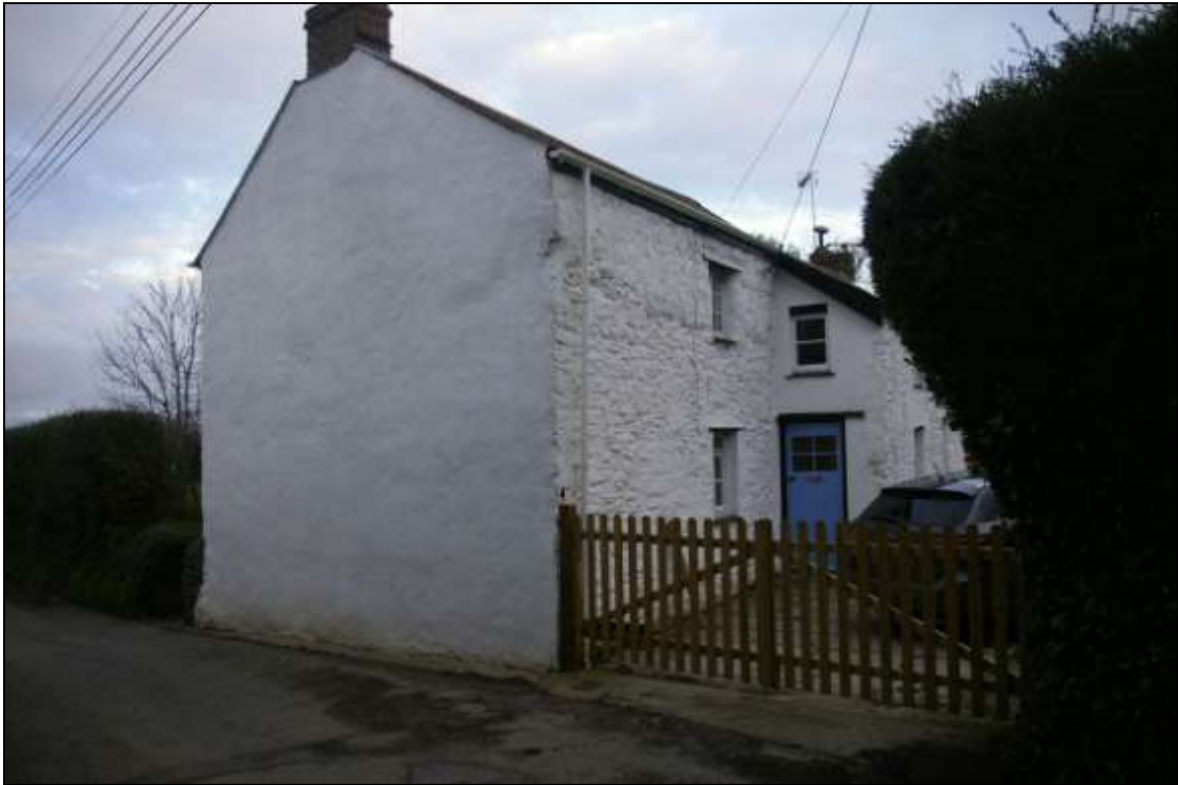
VIEW OF NO. 4 AND COTTAGE; VIEWED FROM THE WEST.
