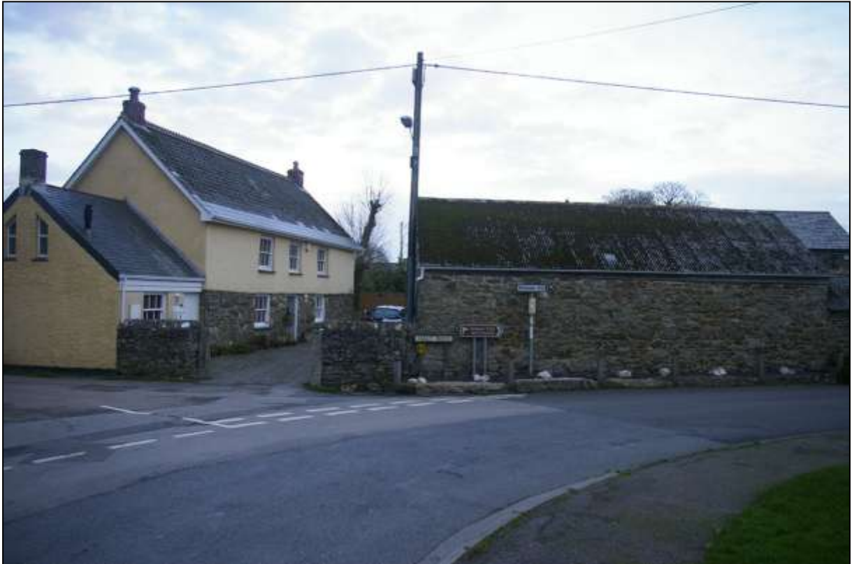
VIEW OF POPHAM FARMHOUSE, AND ASSOCIATED BUILDINGS; VIEWED FROM THE WEST.
