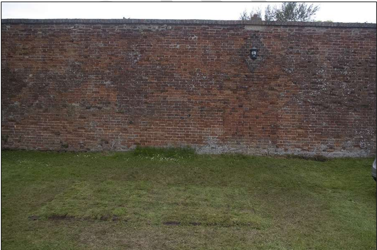
21. TEST PIT, POST-BACKFILLING, IN RELATION TO BLOCKED ENTRANCE IN ADJACENT WALL; VIEWED FROM THE EAST (NO SCALE).
