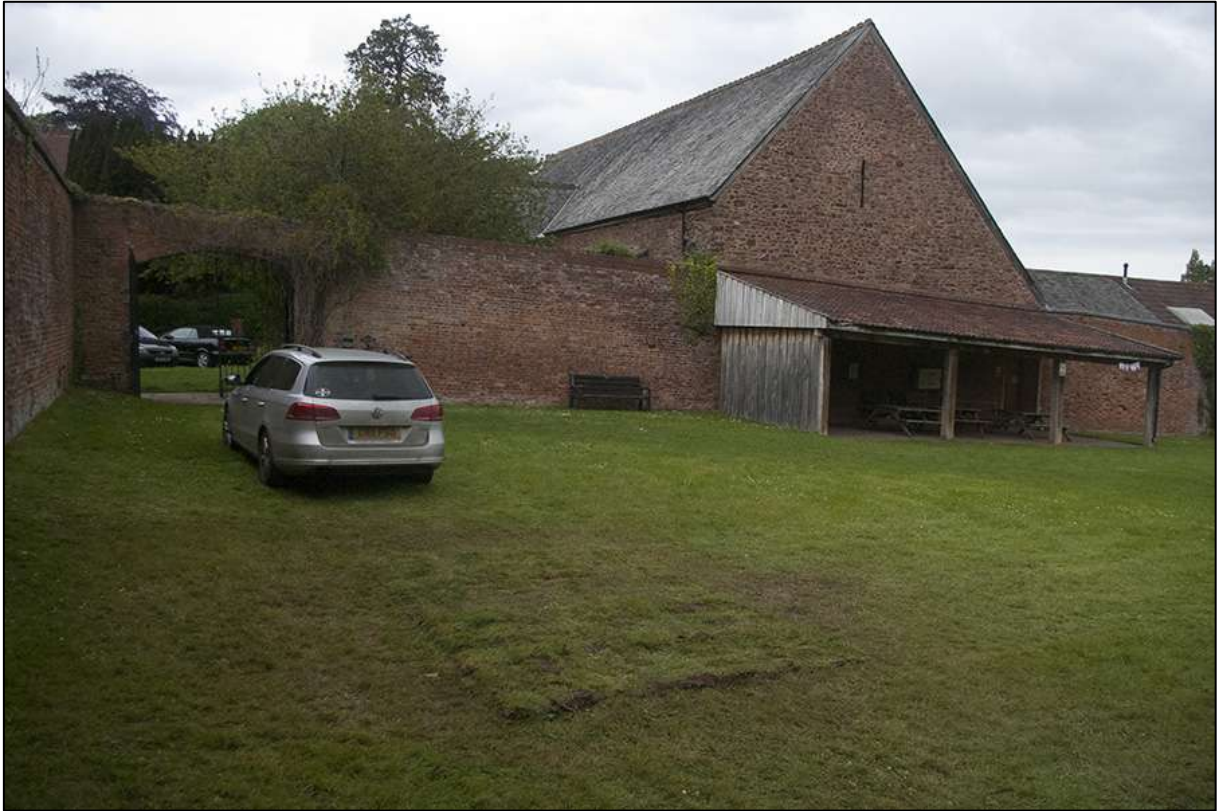
20. TEST PIT, POST-BACKFILLING, IN RELATION TO TITHE BARN; VIEWED FROM THE SOUTH-WEST (NO SCALE).
