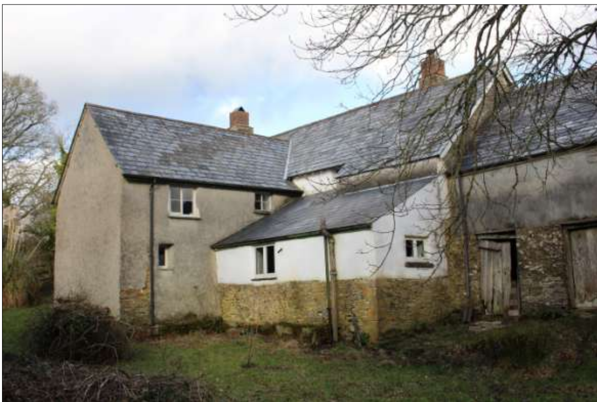
FIGURE 8: THE FARMHOUSE, VIEWED FROM THE SOUTH-WEST. THE CROSSWING IS TO THE LEFT, THE HALL WITH PROJECTION TO THE REAR, THE PUMP ROOM IN THE ANGLE BETWEEN THE TWO, AND THE SHIPPON ON THE RIGHT.
