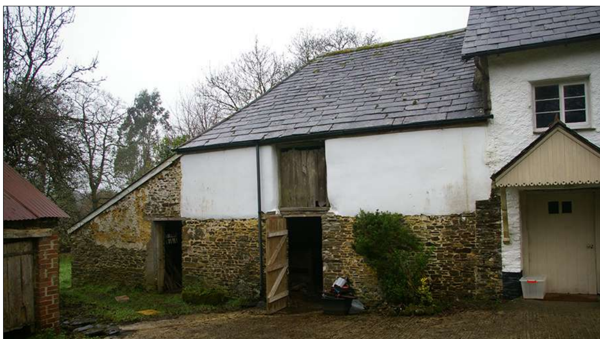
FIGURE 13: EAST ELEVATION OF BARN; VIEWED FROM THE EAST.
