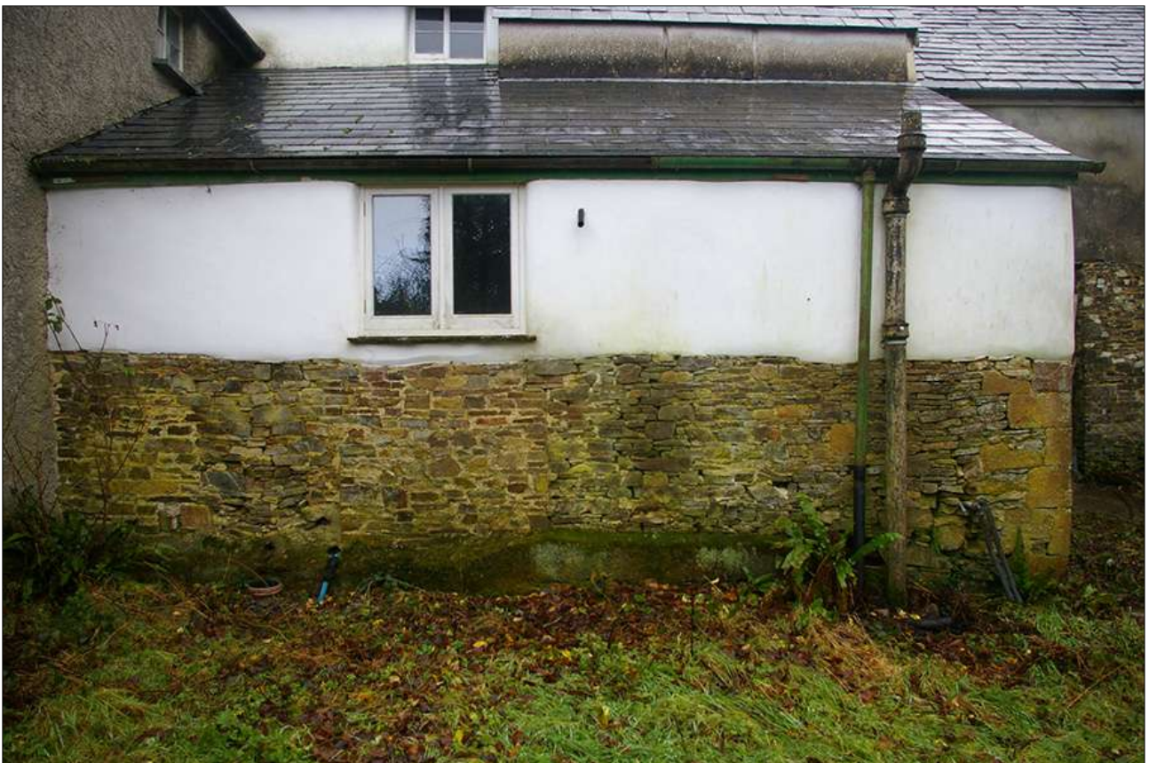
WEST ELEVATION OF THE PUMP ROOM; VIEWED FROM THE WEST.
