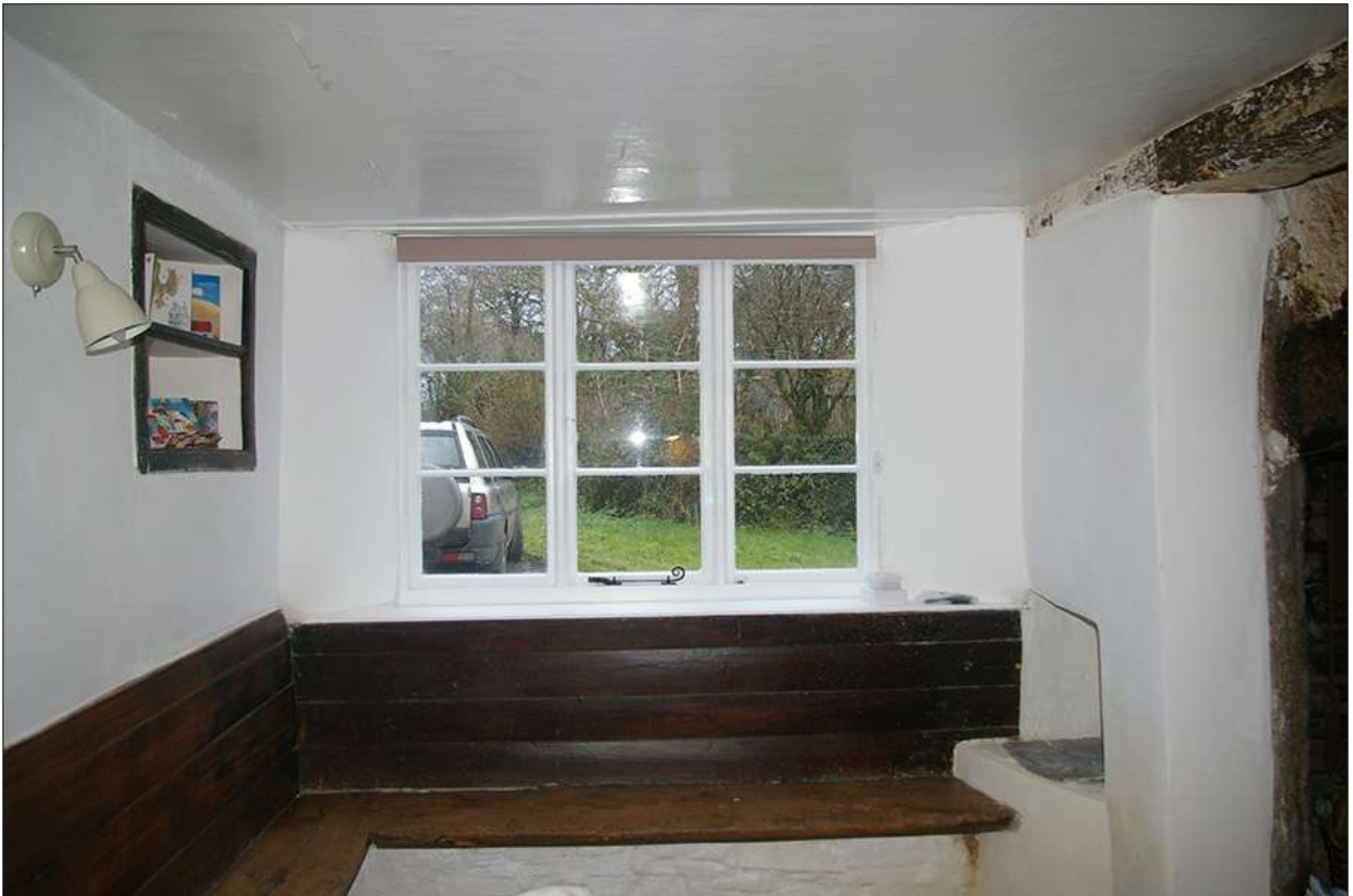
HALL, NORTH-EAST CORNER BENCH (S3) WITH WINDOW (W1) AND BOILER/COPPER (S2); VIEWED FROM THE WEST.
