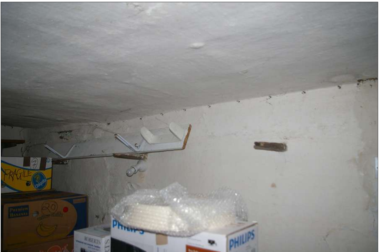
DAIRY, EAST WALL AND CEILING; VIEWED FROM THE SOUTH-WEST.
