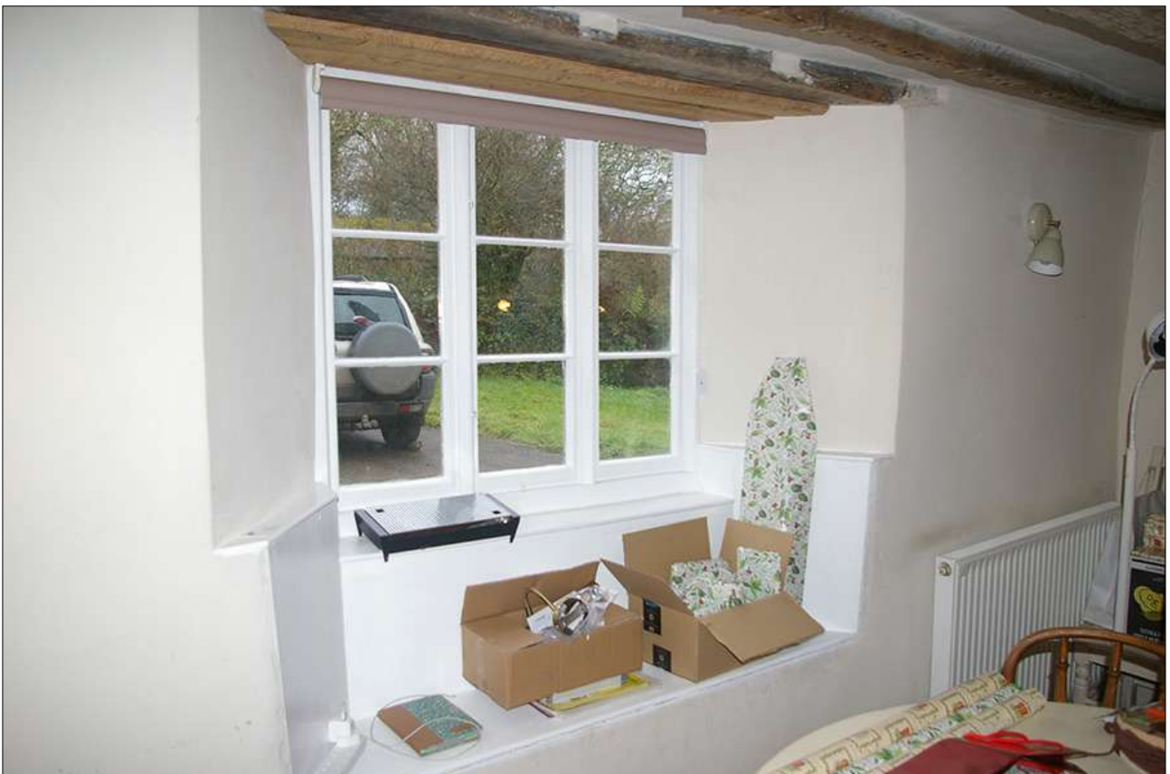
PARLOUR, EAST WINDOW (W2); VIEWED FROM THE NORTH-WEST.
