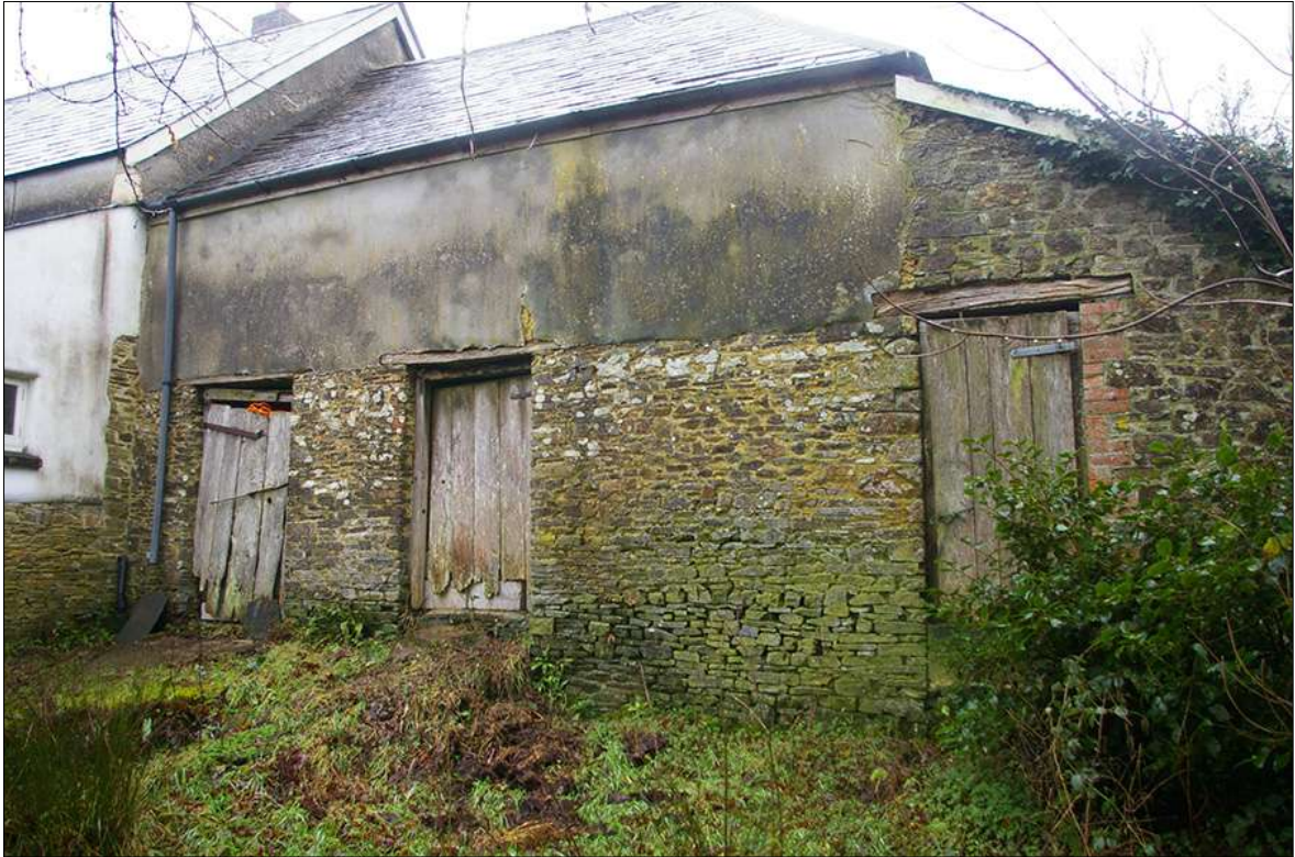
FIGURE 14: WEST ELEVATION OF SHIPPON; VIEWED FROM THE SOUTH-WEST.
