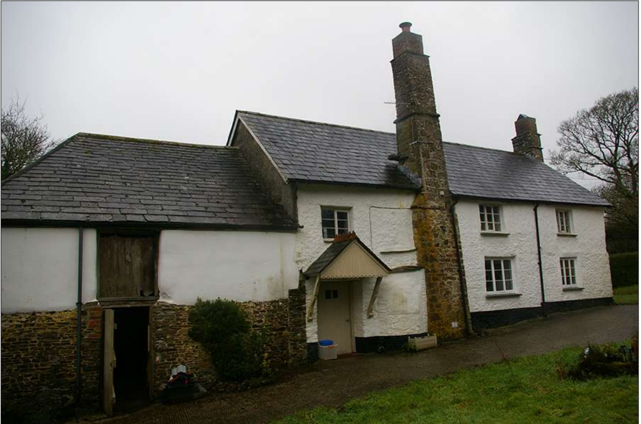
EAST ELEVATION; VIEWED FROM THE SOUTH-EAST.
