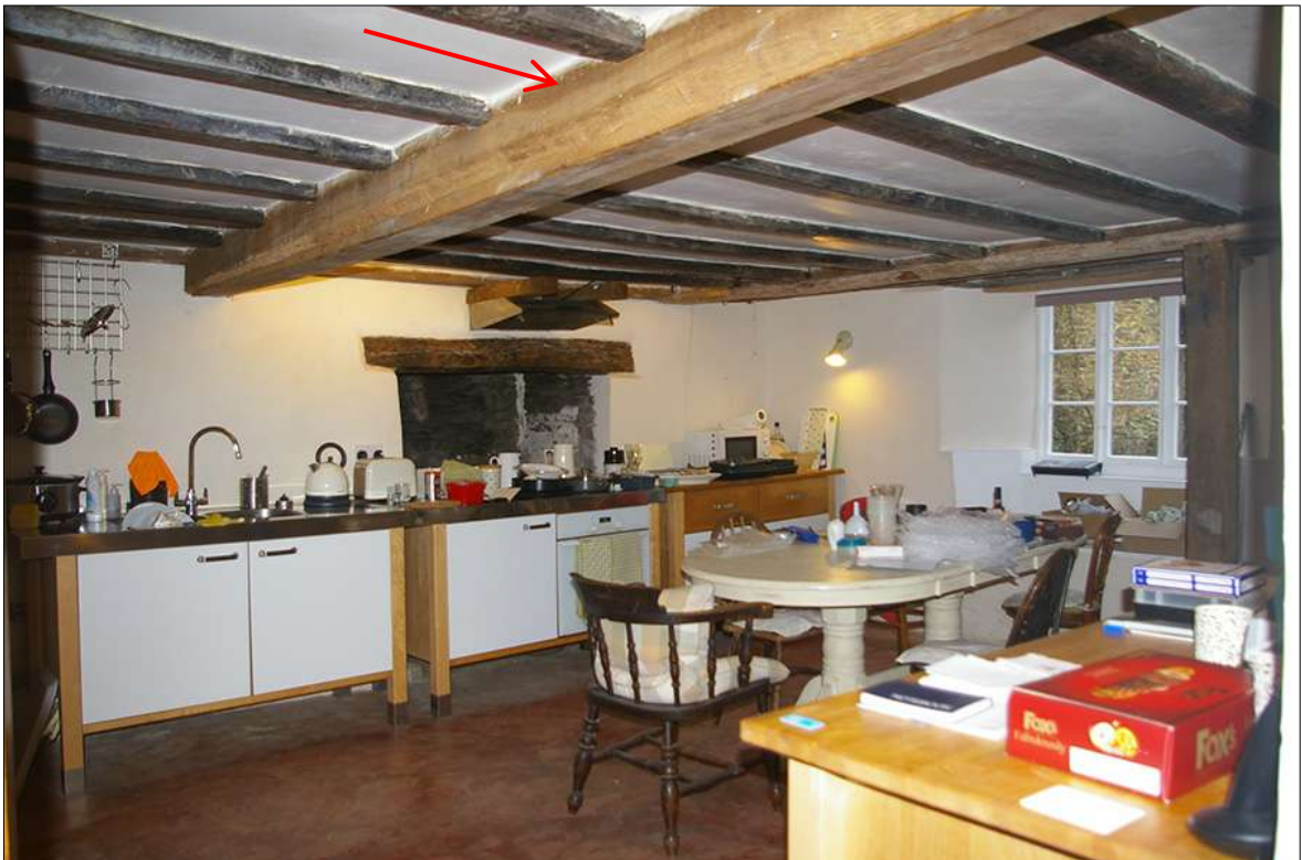
FIGURE 10: THE PARLOUR, VIEWED FROM THE SOUTH-WEST CORNER. THE REPLACED BEAM IS INDICATED.
