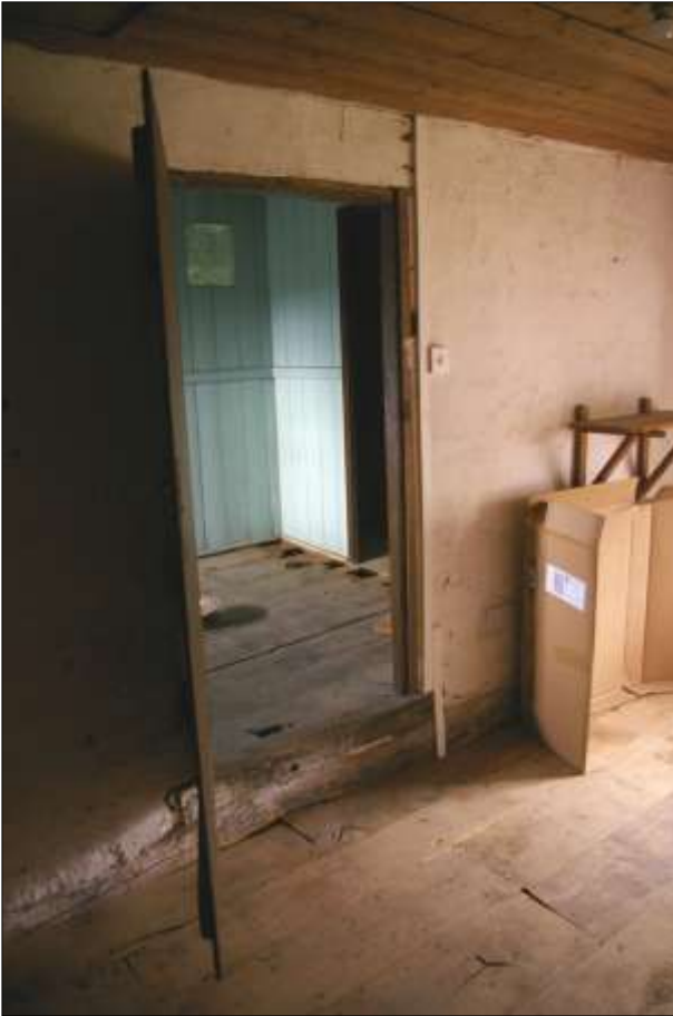
APPLE STORE, DOORWAY (D16) INTO BEDROOM 4; VIEWED FROM THE SOUTH-SOUTH-WEST.
