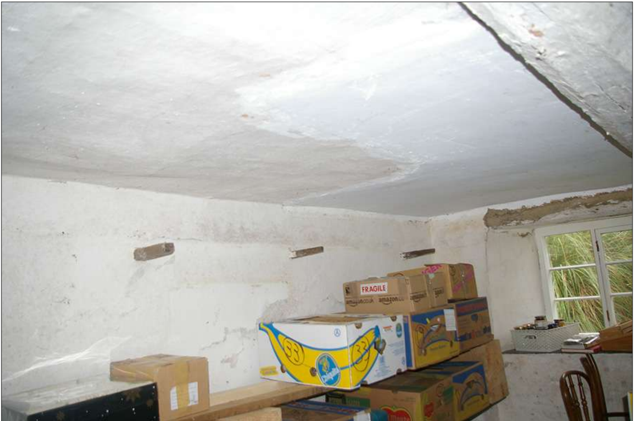
DAIRY, NORTH-WEST CORNER WITH NORTH WINDOW (W3); VIEWED FROM THE SOUTH-EAST.
