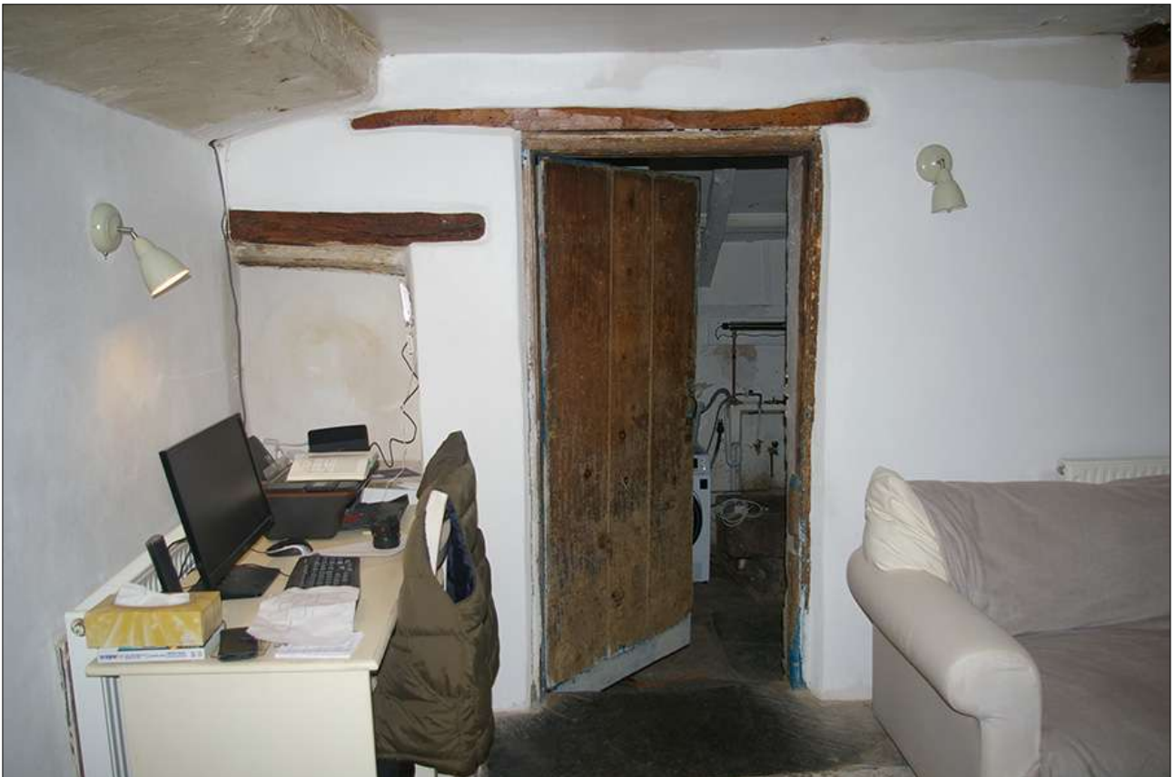
HALL, WEST WALL, SHOWING D5 INTO THE PUMP ROOM, AND THE ALCOVE BO4; VIEWED FROM THE EAST.
