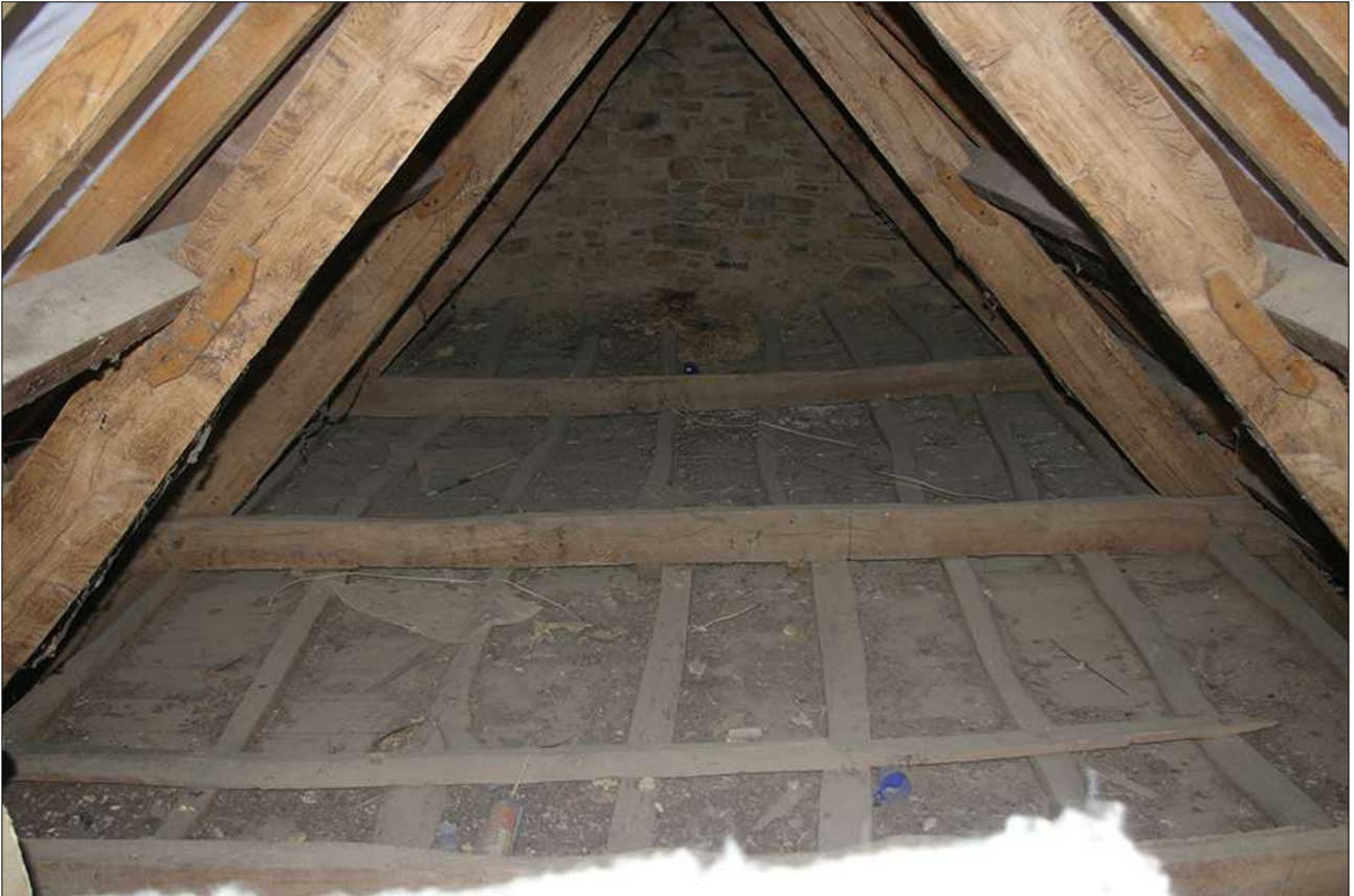
THE ROOF ABOVE THE CROSSWING; VIEWED FROM THE EAST.
