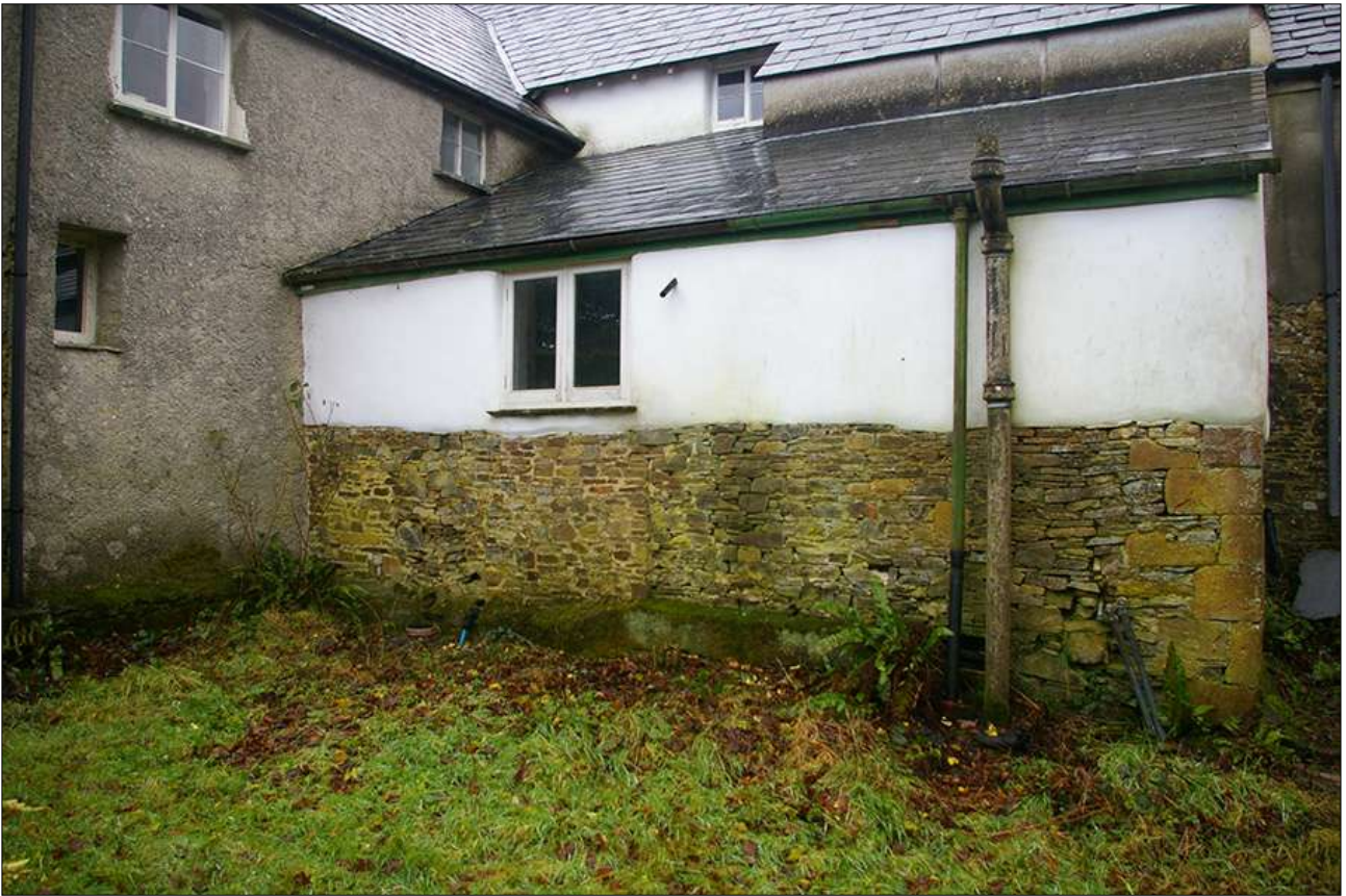
WEST ELEVATION OF THE PUMP ROOM; VIEWED FROM THE WEST-SOUTH-WEST.
