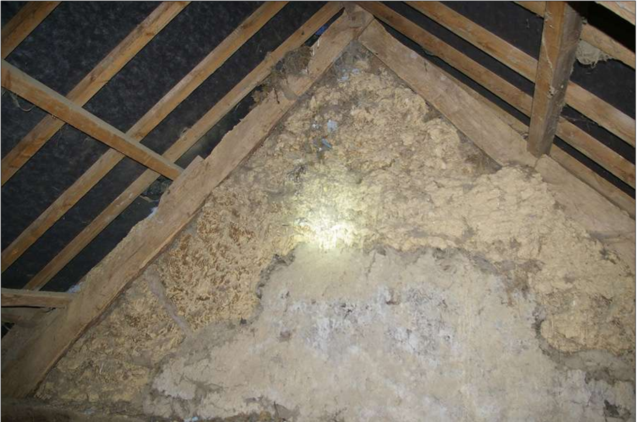
DETAIL OF THE SOUTH GABLE; VIEWED FROM THE NORTH.
