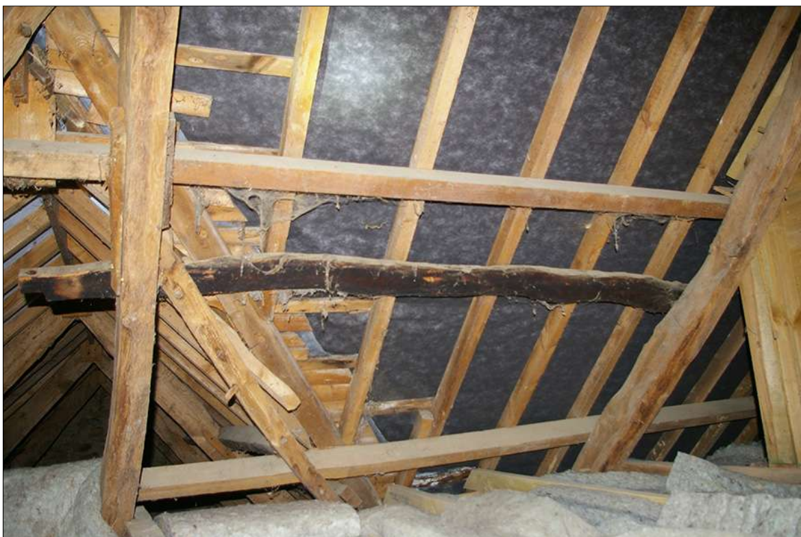
FIGURE 12: DETAIL OF THE ROOF STRUCTURE ABOVE THE PARLOUR BEDROOM, SHOWING A RE-USED SMOKE-BLACKENED RAFTER; VIEWED FROM THE SOUTH-EAST.
