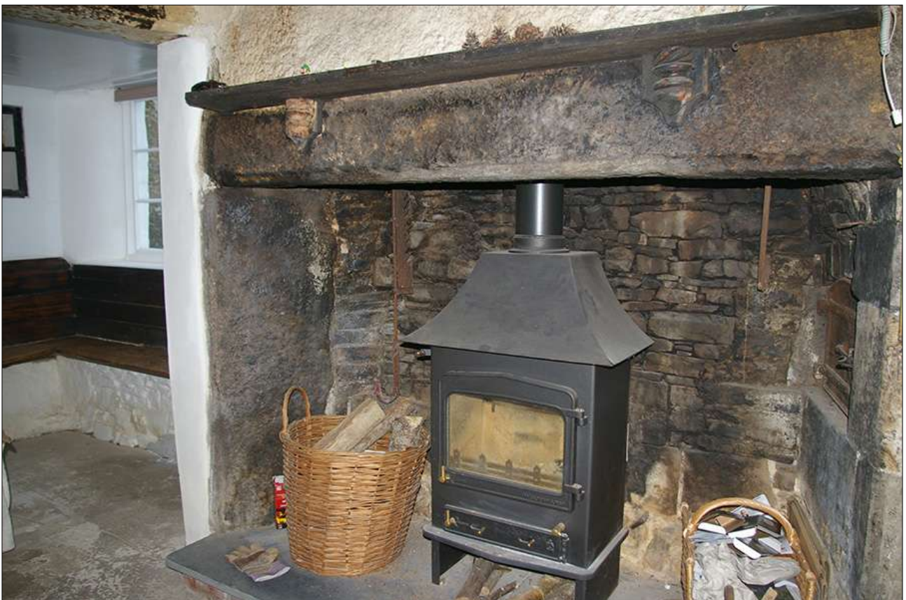
HALL, FP1 IN EAST WALL; VIEWED FROM THE SOUTH-WEST.
