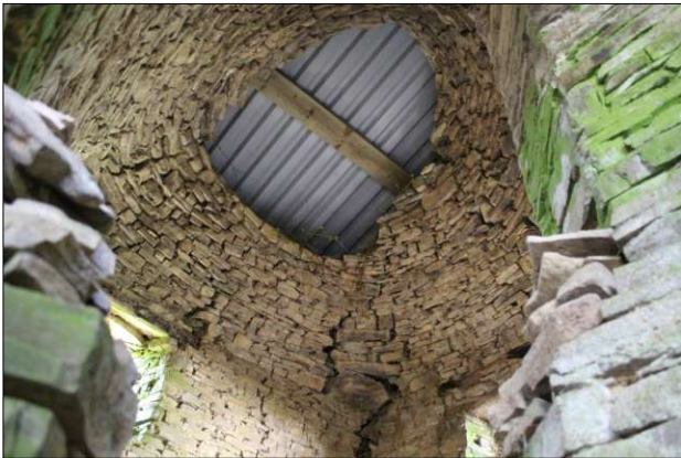
LEFT FIGURE 24: THE CEILING OF THE MALTING KILN; VIEWED FROM THE BELOW/SOUTH-EAST.
