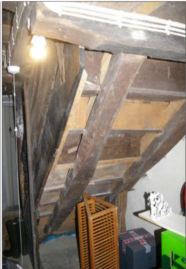
RIGHT: STAIRHALL, THE UNDERSIDE OF THE STAIRS WITH OBVIOUS REPAIRS; VIEWED FROM THE NORTH-EAST.
