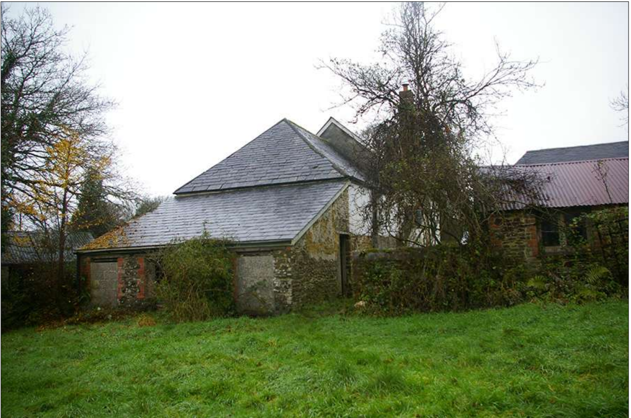
SOUTH AND EAST ELEVATIONS OF THE SHIPPON; VIEWED FROM THE SOUTH-EAST.
