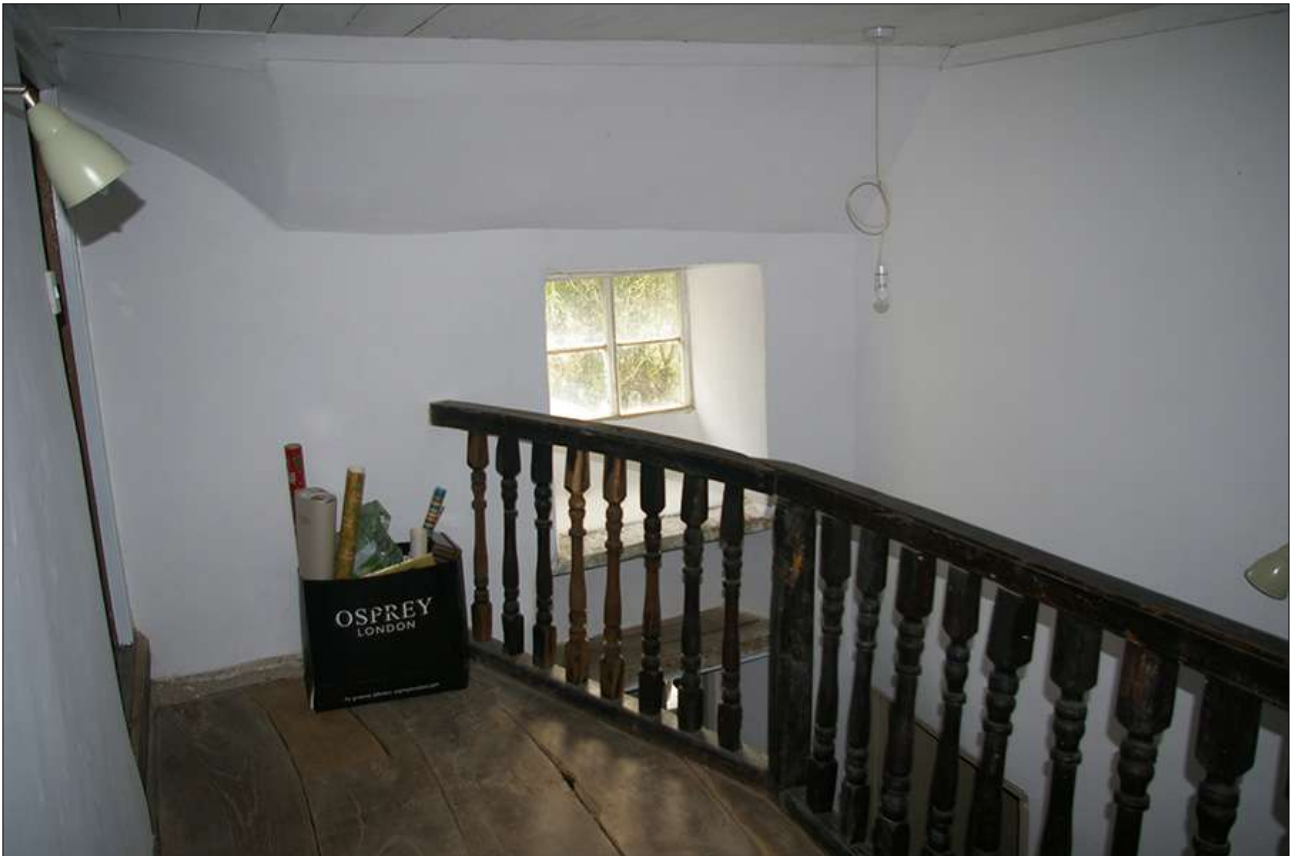
AS ABOVE; VIEWED FROM THE NORTH-NORTH-EAST.
