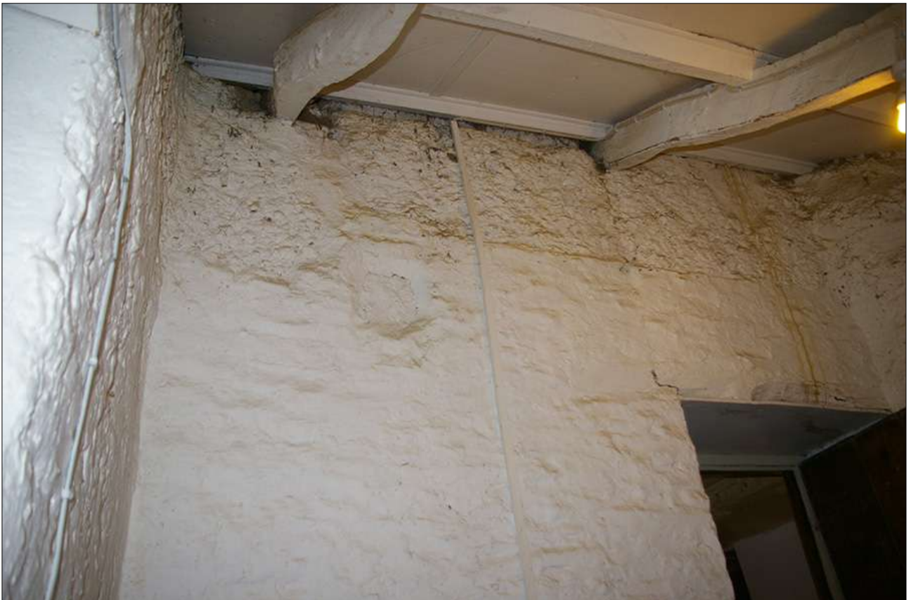
PUMP ROOM, EAST WALL SHOWING RAFTERS; VIEWED FROM THE WEST.
