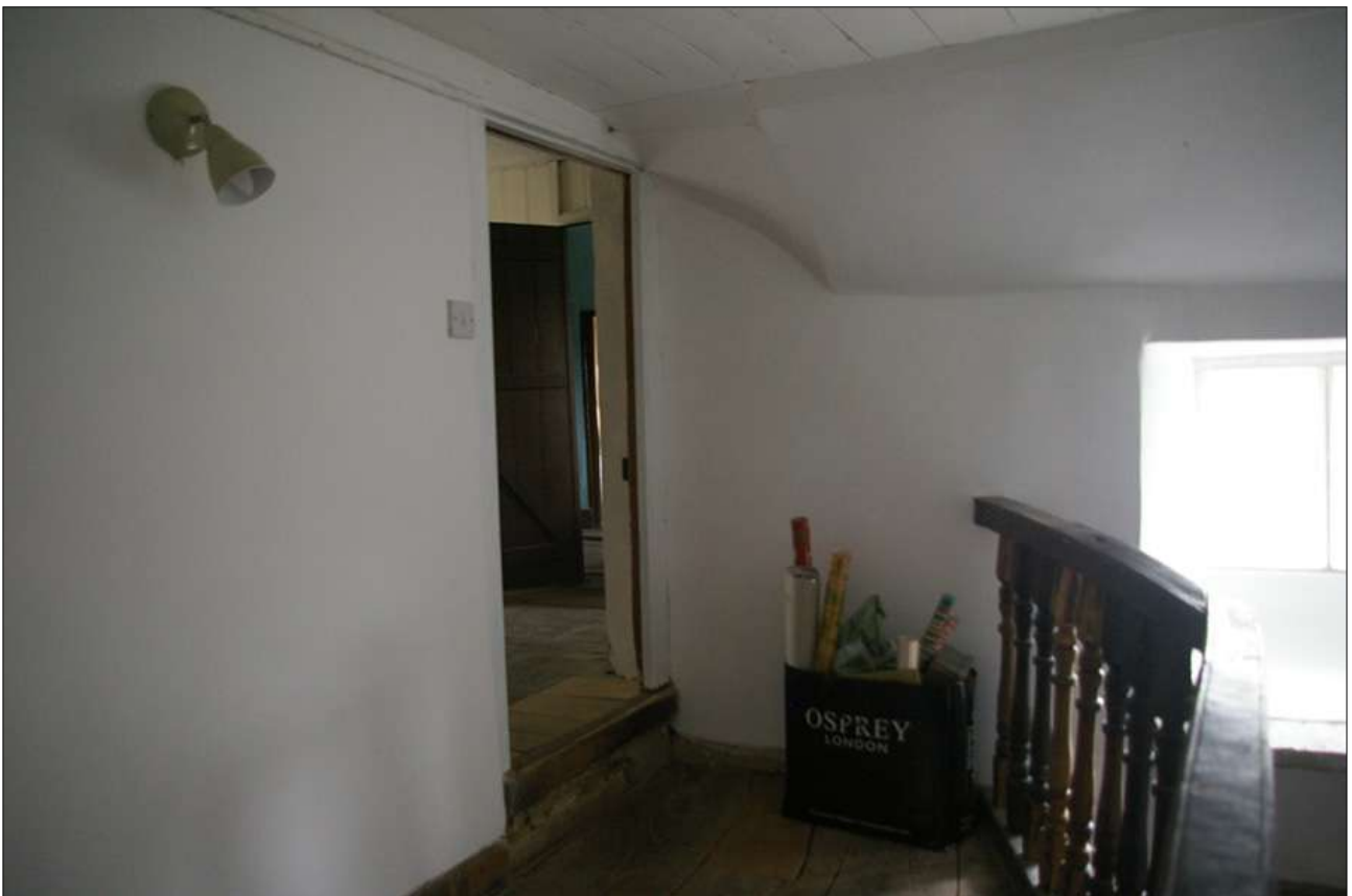
STAIRHALL FF, THE LANDING SHOWING THE DOORWAY (D13) INTO BEDROOM 3; VIEWED FROM THE NORTH.
