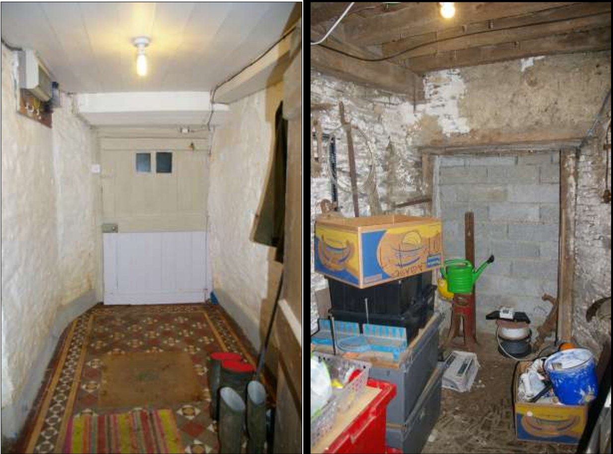
LEFT: THE CROSS PASSAGE, EAST END WITH THE FRONT DOOR D1; VIEWED FROM THE WEST
