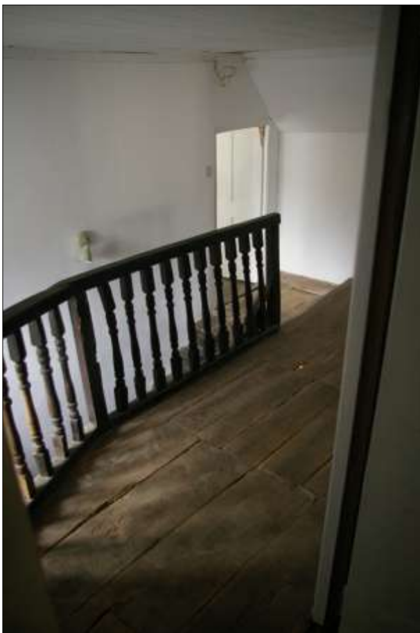
LEFT: STAIRHALL FF, THE LANDING AND RAIL; VIEWED FROM THE SOUTH-EAST.
