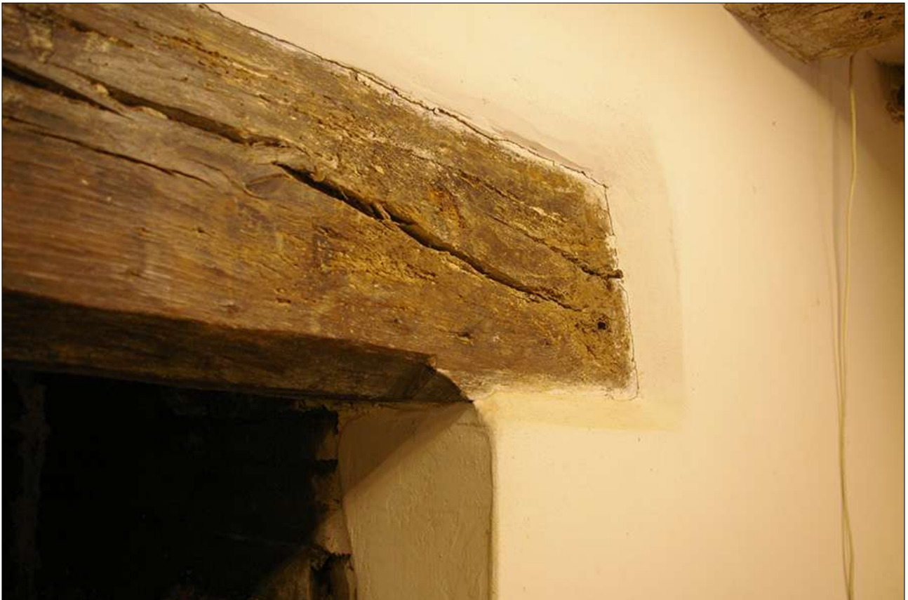
AS ABOVE, DETAIL OF THE CHAMFER ON THE LINTEL; VIEWED FROM THE SOUTH-WEST.
