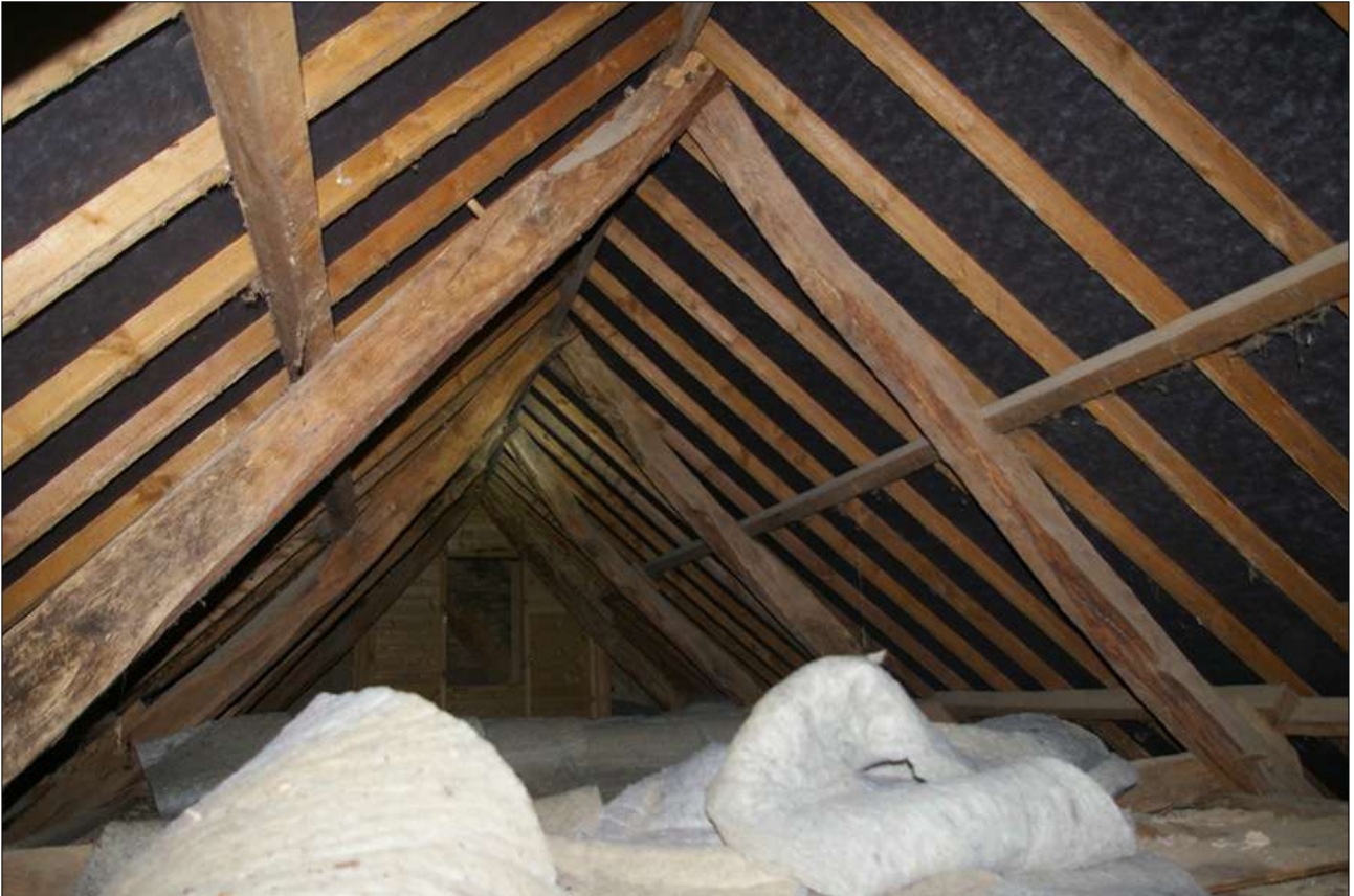
THE ROOF ABOVE BEDROOMS 2 AND 3; VIEWED FROM THE SOUTH.
