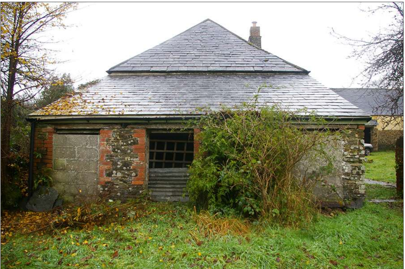
SOUTH ELEVATION OF THE PIGSTY; VIEWED FROM THE SOUTH.
