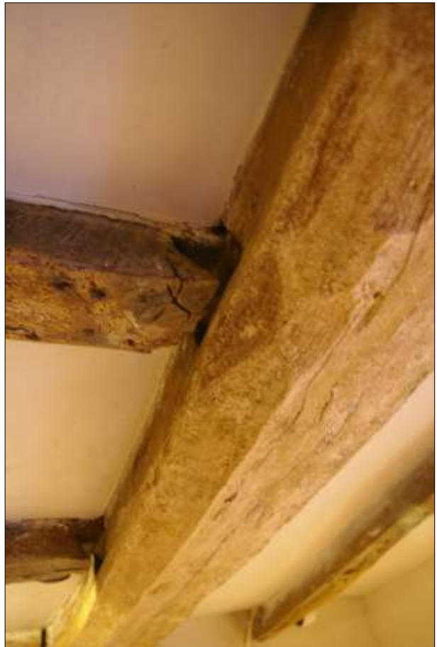
LEFT: PARLOUR, THE ORIGINAL BEAM (RIGHT) WITH ROUGH JOISTS IN THE GAP BETWEEN THE BEAM AND THE EAST WALL; VIEWED FROM THE NORTH. RIGHT: PARLOUR, THE ORIGINAL BEAM SHOWING THE JOISTS PULLING OUT; VIEWED FROM THE SOUTH.
