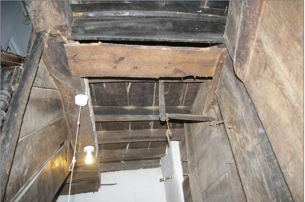
STAIRHALL, THE UNDERSIDE OF THE LANDING; VIEWED FROM THE SOUTH.
