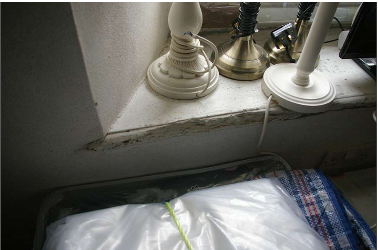
AS ABOVE, DETAIL OF THE WINDOW SILL; VIEWED FROM THE WEST.
