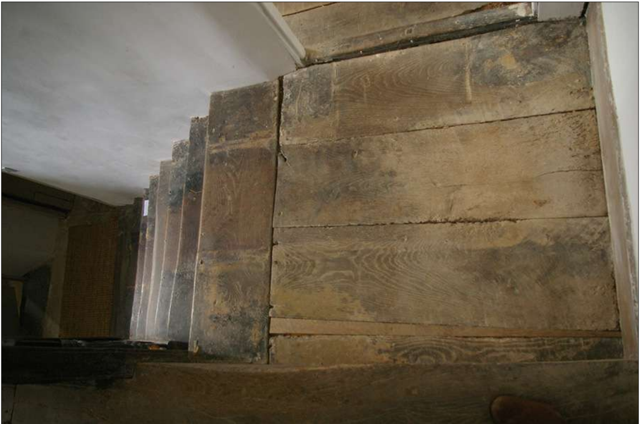
STAIRHALL FF, SHOWING THE FLOORBOARDS; VIEWED FROM THE EAST.
