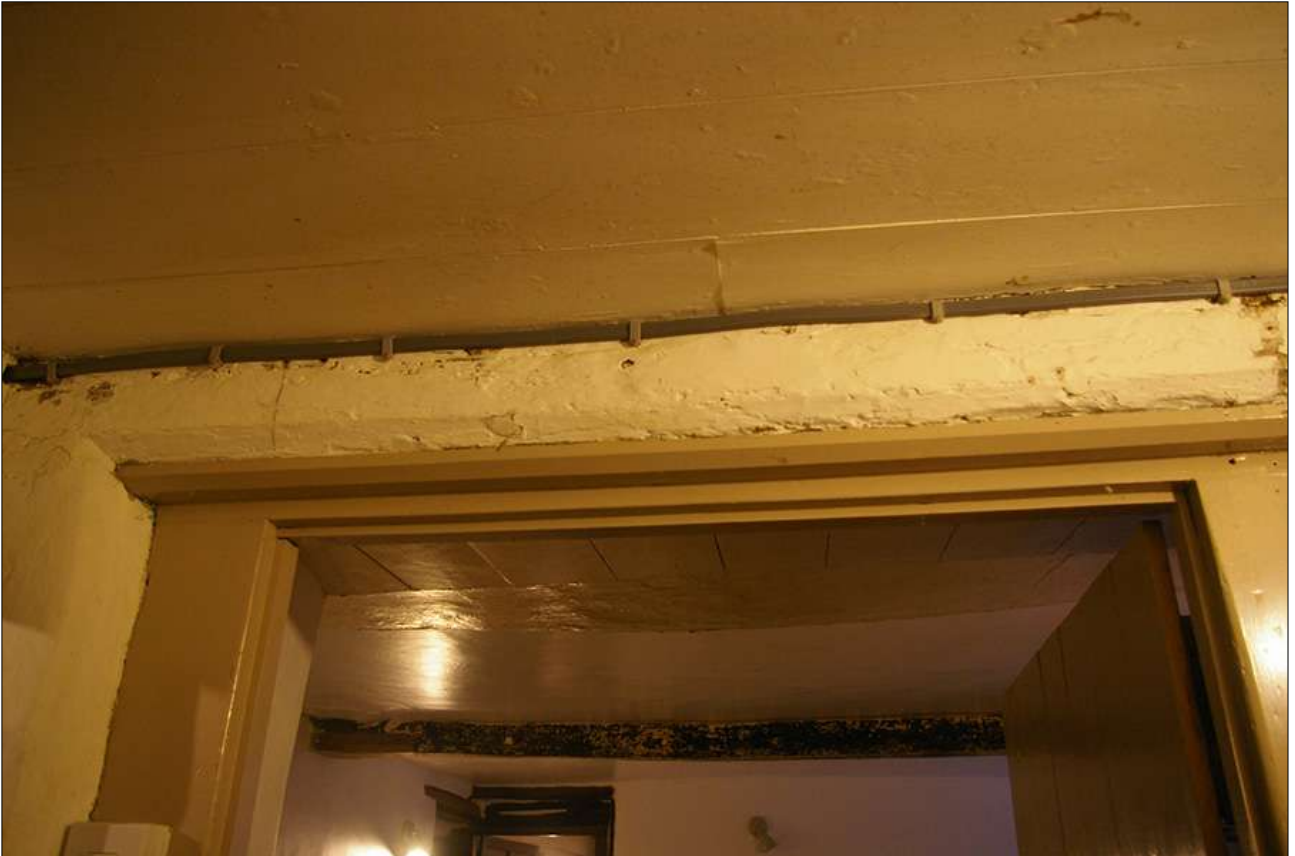
CROSS PASSAGE NORTH WALL WITH DOORWAY D2; VIEWED FROM THE SOUTH.
