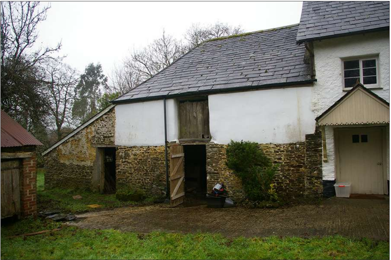
EAST ELEVATION OF THE SHIPPON; VIEWED FROM THE NORTH-EAST.
