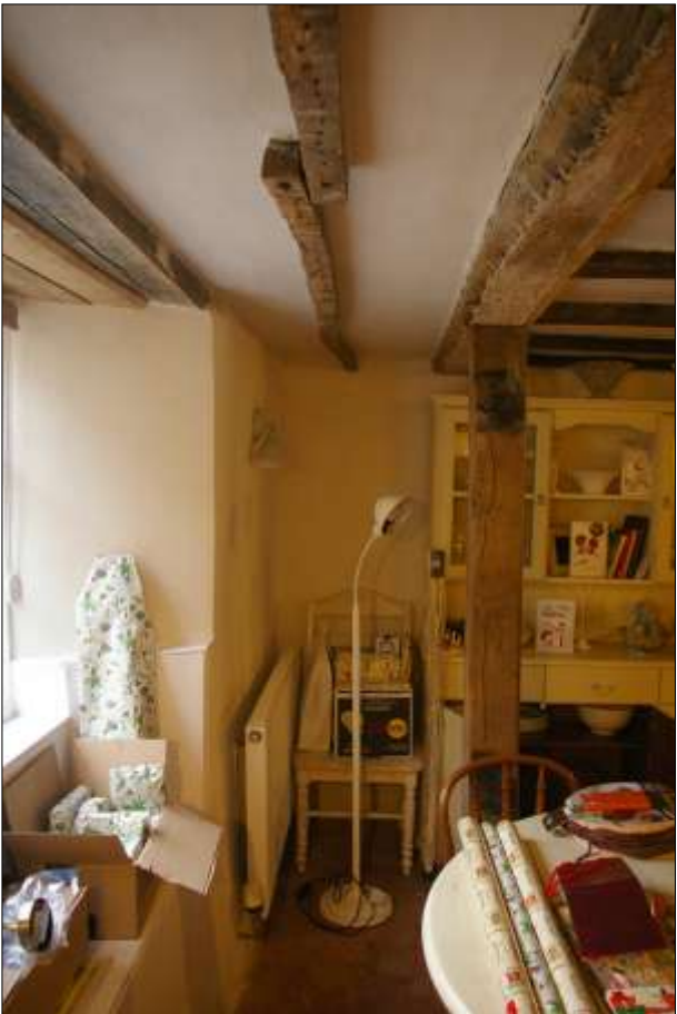
LEFT: PARLOUR, THE ORIGINAL BEAM (RIGHT) WITH ROUGH JOISTS IN THE GAP BETWEEN THE BEAM AND THE EAST WALL; VIEWED FROM THE NORTH. RIGHT: PARLOUR, THE ORIGINAL BEAM SHOWING THE JOISTS PULLING OUT; VIEWED FROM THE SOUTH.
