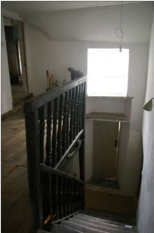
LEFT: STAIRHALL FF, STAIRCASE; VIEWED FROM THE NORTH.
