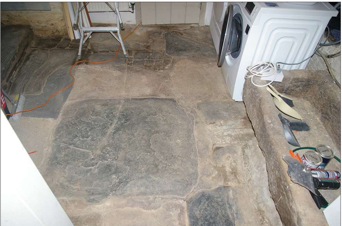
PUMP ROOM, DETAIL OF THE FLOOR; VIEWED FROM THE NORTH.
