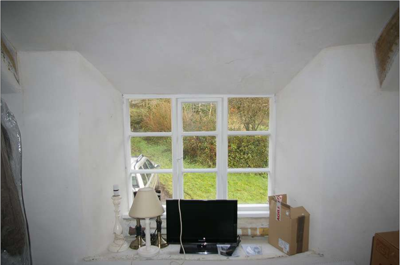
BEDROOM 3, THE WINDOW (W8) IN THE EAST WALL; VIEWED FROM THE WEST.
