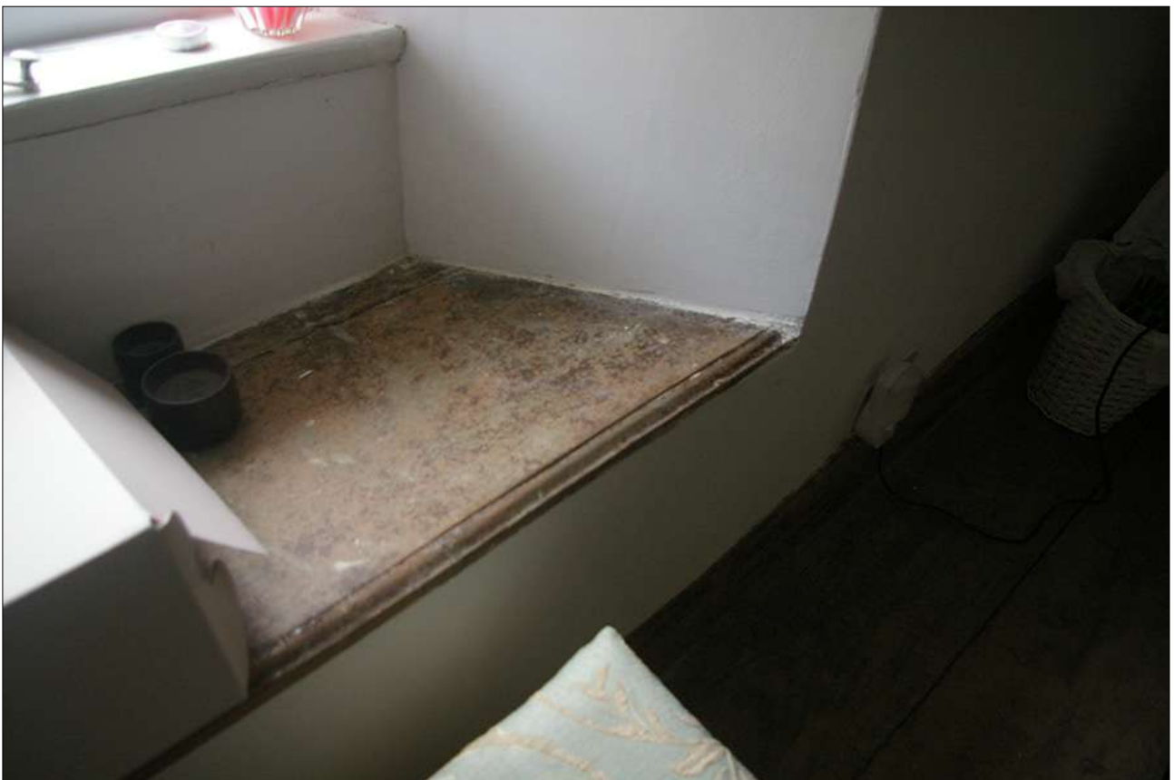
AS ABOVE, DETAIL OF THE WINDOW SEAT; VIEWED FROM THE NORTH-WEST.
