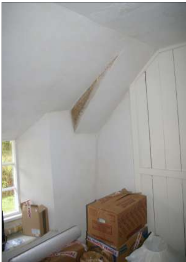
AS ABOVE, SHOWING THE FOOT OF THE TRUSS SOUTH OF W8, AND THE SIDE OF THE STACK; VIEWED FROM THE NORTH-WEST.
