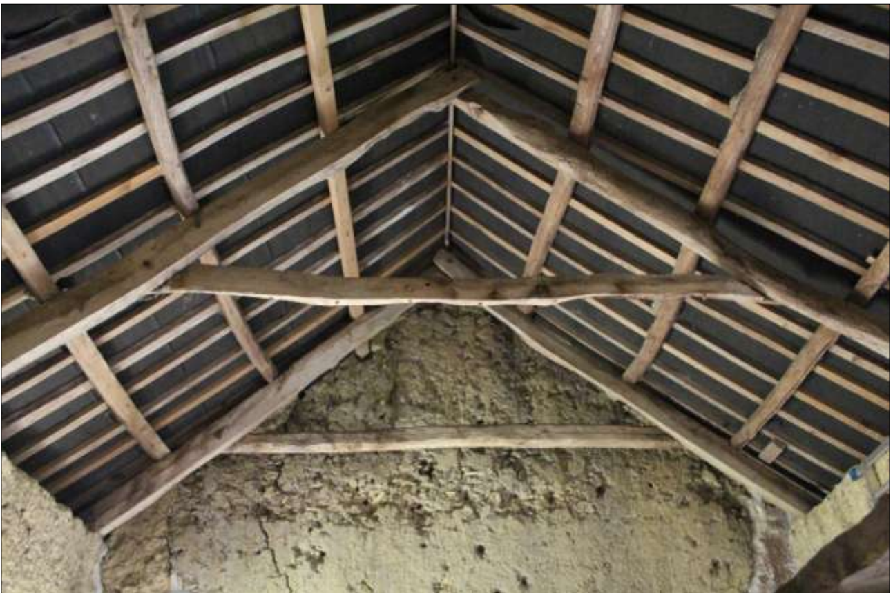
THE ROOF STRUCTURE; VIEWED FROM THE SOUTH.
