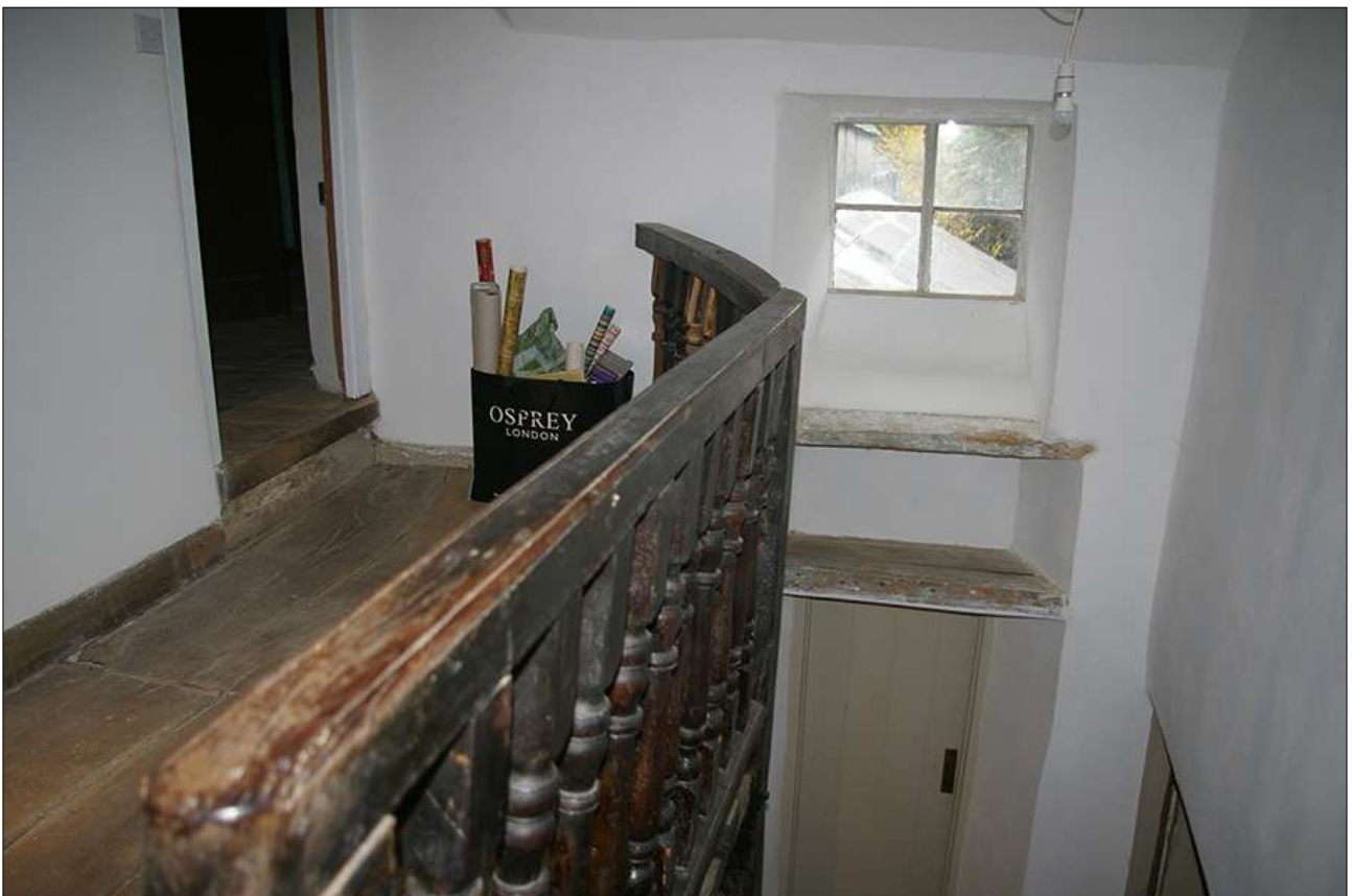
STAIRHALL FF, SHOWING THE BEADED HAND RAIL AND, BEYOND, THE WINDOW INSERTED INTO AN EARLIER DOORWAY (W11); VIEWED FROM THE NORTH.
