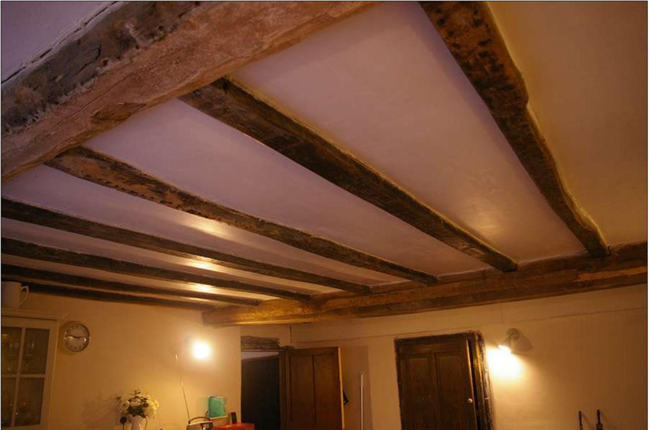
PARLOUR, CEILING JOISTS; VIEWED FROM THE NORTH-EAST.
