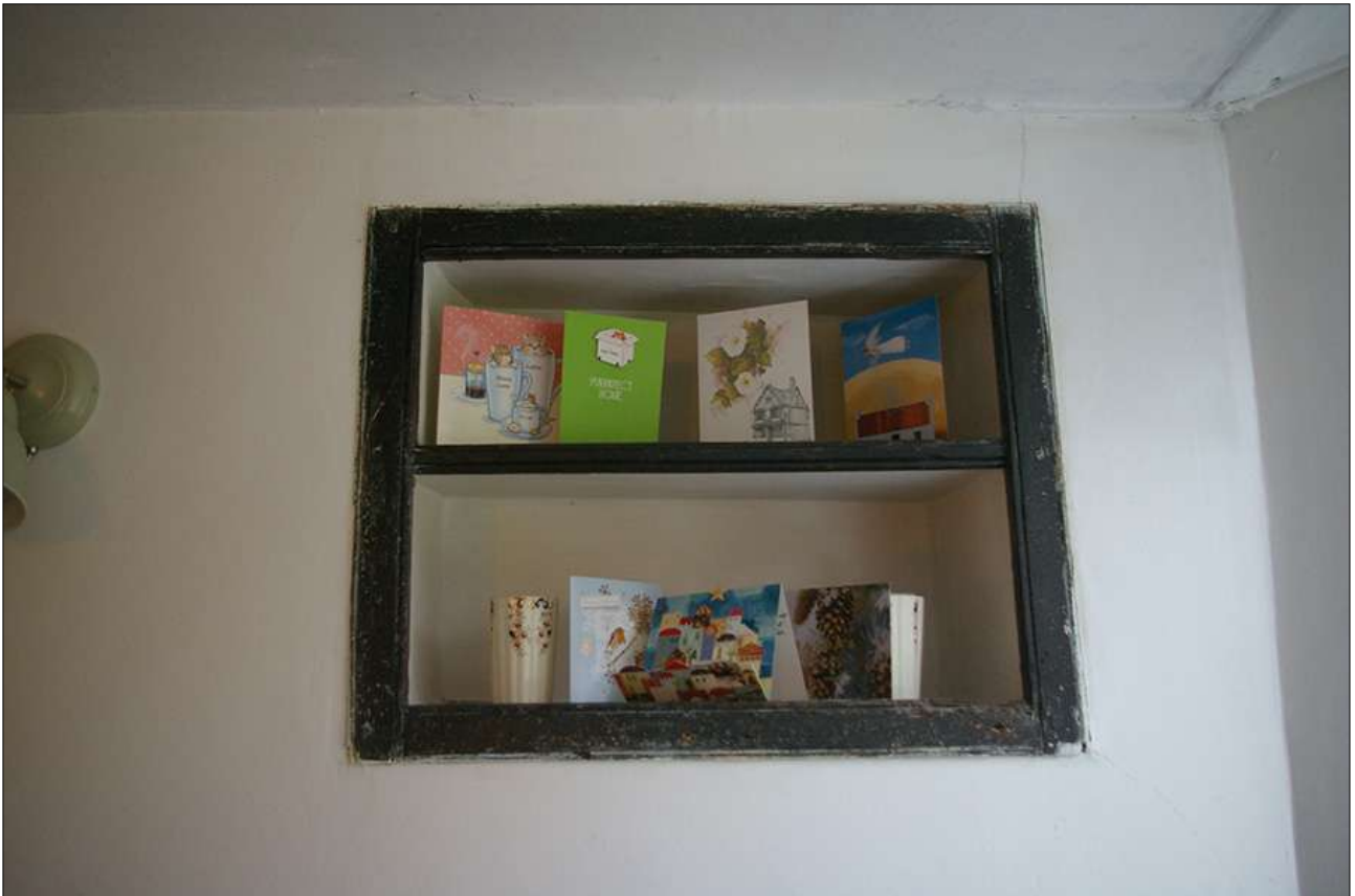
HALL, KEEPING PLACE IN THE NORTH WALL (S4); VIEWED FROM THE SOUTH.
