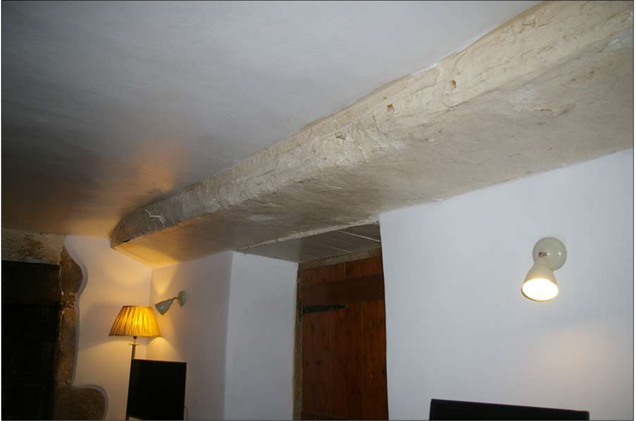
HALL, SOUTH WALL, SHOWING THE PLASTERED JETTY; VIEWED FROM THE NORTH-WEST.
