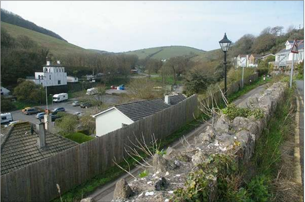
AS ABOVE, LOOKING BACK TO THE VILLAGE CAR PARK AND PENLEE LODGE; VIEWED FROM THE NORTH-EAST.
