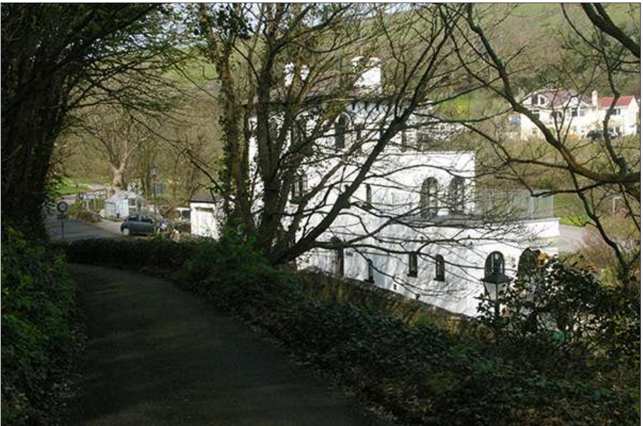
PENLEE LODGE, VIEWED FROM THE EARL'S DRIVE; VIEWED FROM THE SOUTH-EAST.
