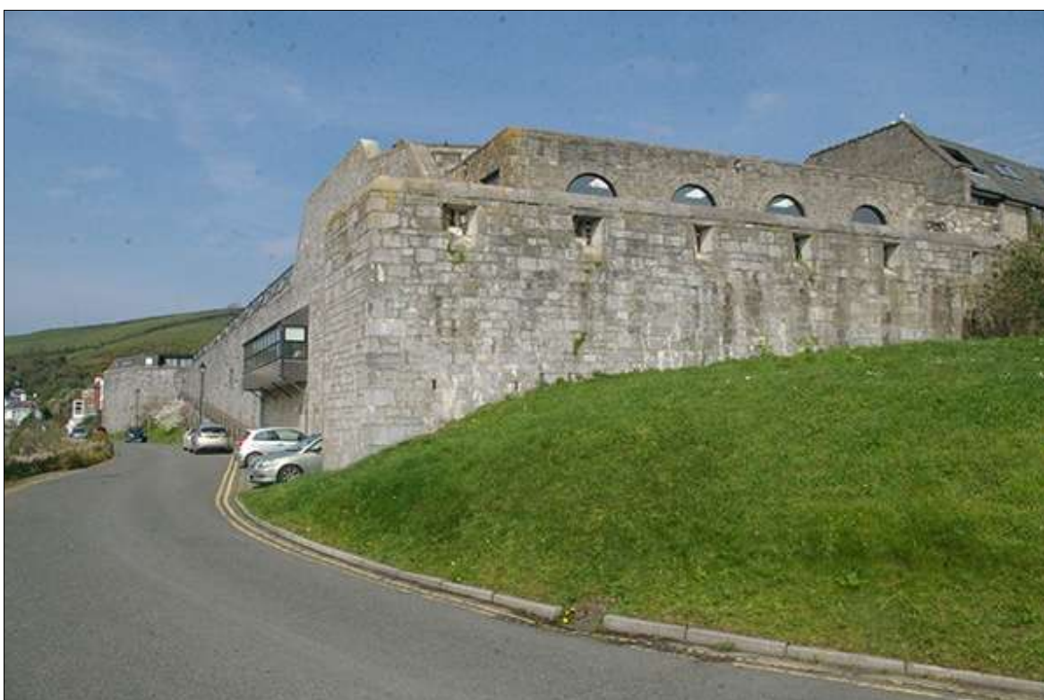
FIGURE 16: THE SOUTH-EASTERN CORNER OF CAWSAND FORT; VIEWED FROM THE SOUTH-EAST.
