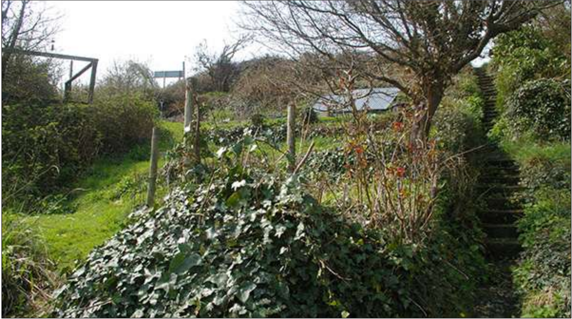
FIGURE 13: THE NORTHERN PART OF THE SITE, LOOKING UP ALONG THE STEPS FLANKING THE SITE TO THE NORTH; VIEWED FROM THE NORTH-EAST, LOOKING SOUTH-WEST.
