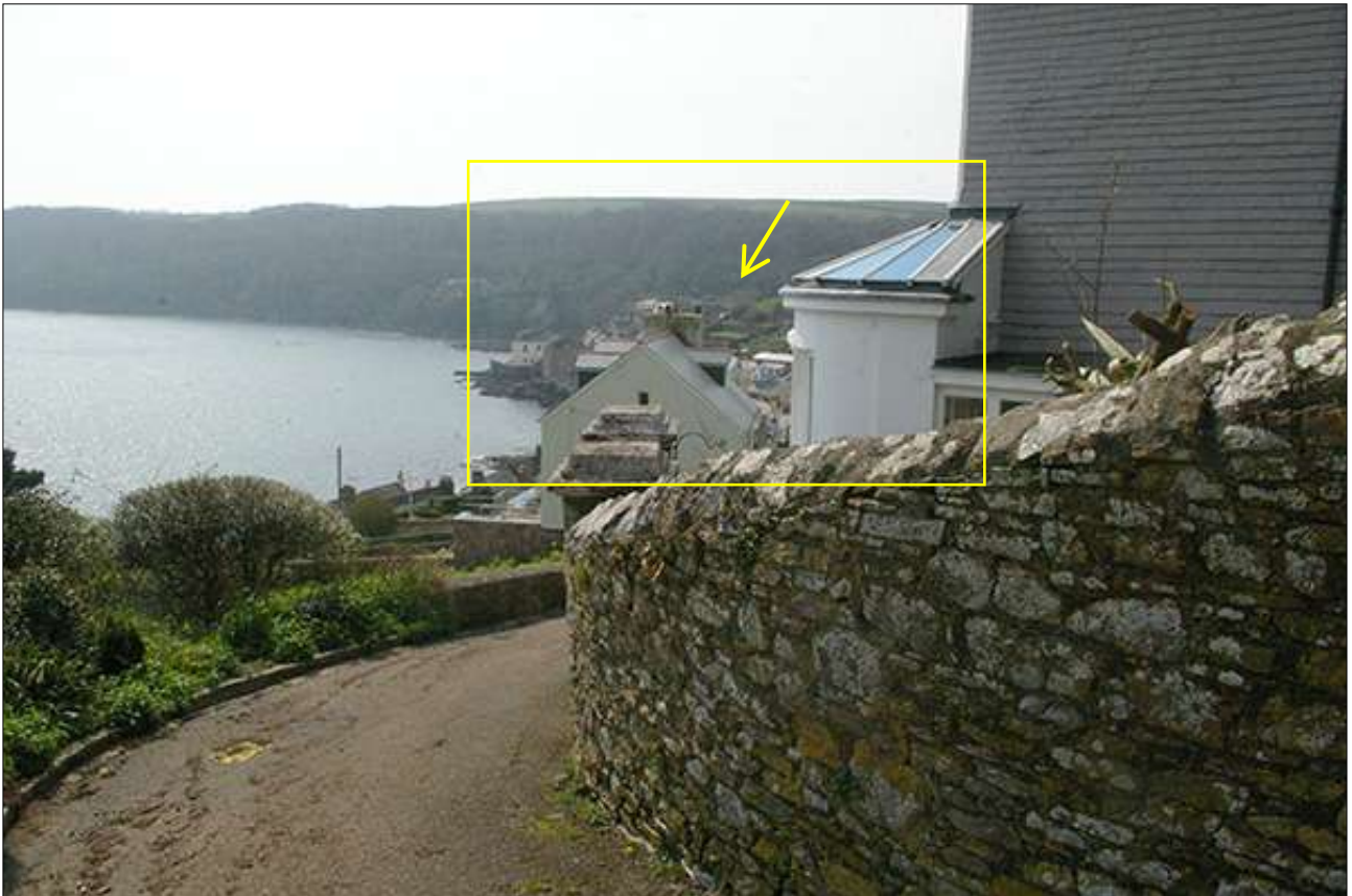
VIEW FROM PENLEY VILLA, LOOKING TOWARDS THE WAR MEMORIAL (INDICATED); VIEWED FROM THE NORTH.
