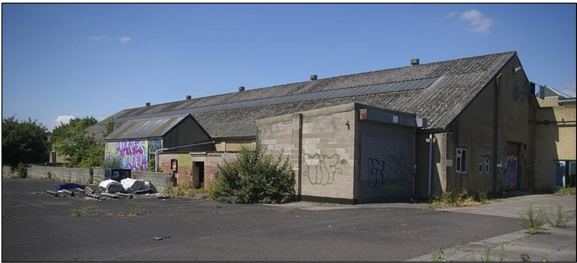
FIGURE 4: EXTERIOR OF BAY 10 (BUILDING 4); VIEWED FROM THE EAST.
