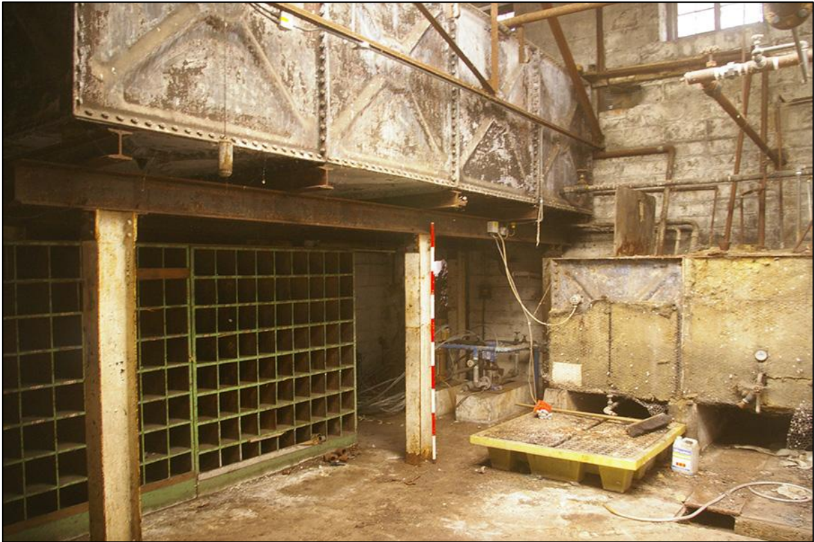
FIGURE 7: INTERIOR OF PLANT ROOM (BUILDING 8), NORTH-EAST ROOM; VIEWED FROM THE EAST (2M SCALE).
