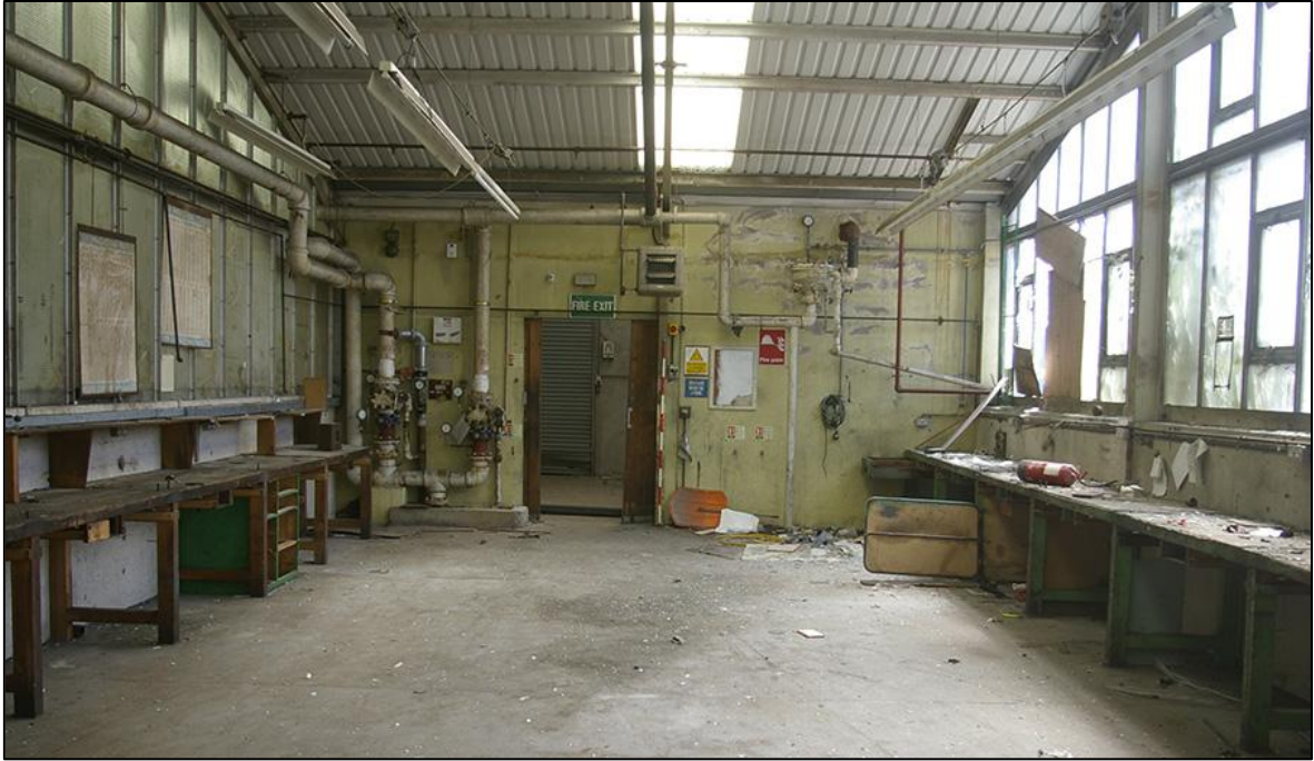
FIGURE 5: INTERIOR OF WORKSHOP (BUILDING 5), SOUTH-WEST ROOM; VIEWED FROM THE NORTH-WEST (2M SCALE).
