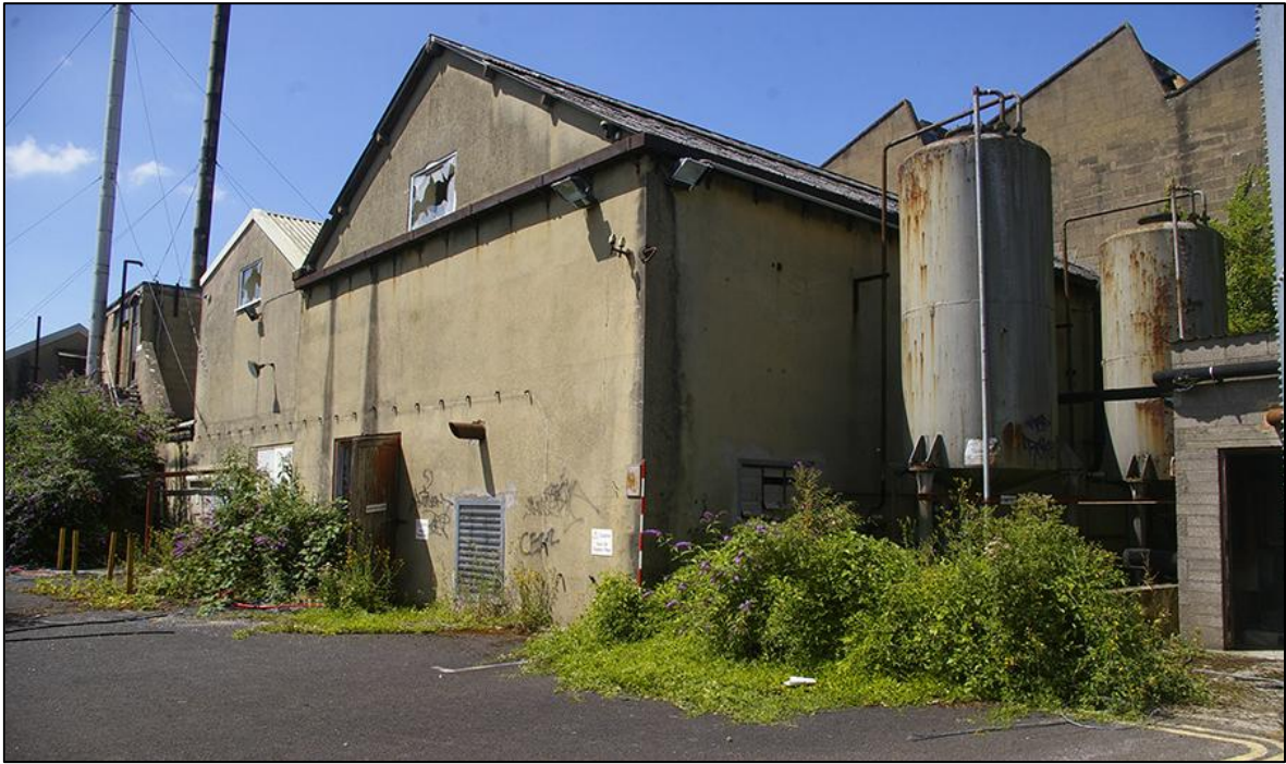
FIGURE 8: EXTERIOR OF MACHINERY SHED (BUILDING 9); VIEWED FROM THE EAST-NORTH-EAST (2M SCALE).
