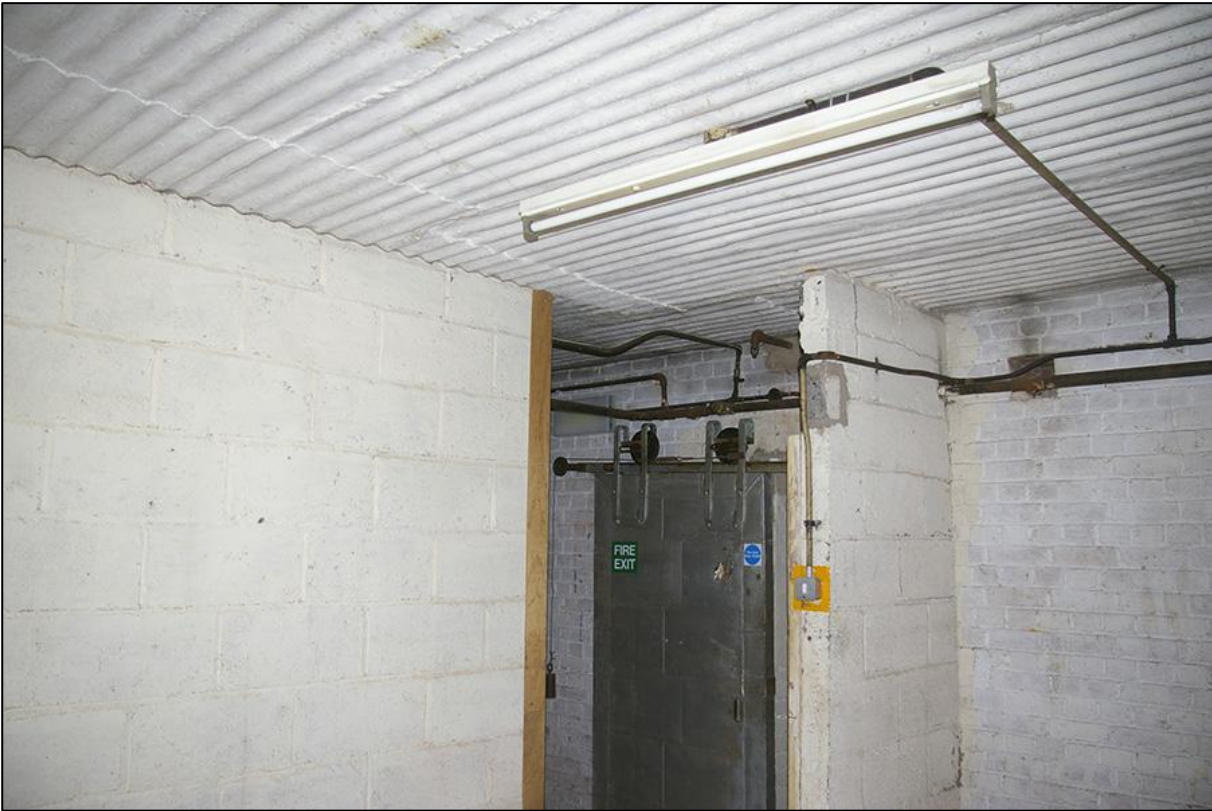
ENTRANCE TO CELLAR; VIEWED FROM INSIDE CELLAR.
