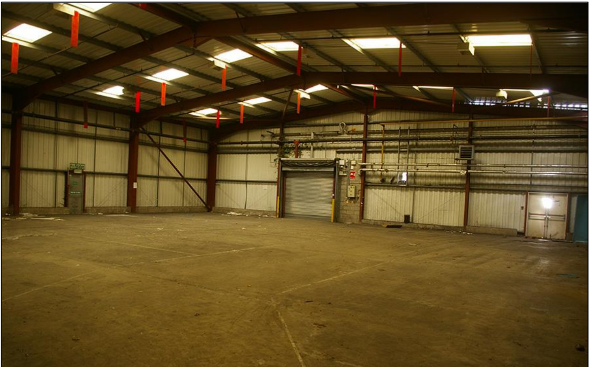
FIGURE 12: THE MOST RECENT WAREHOUSE (BUILDING 15); VIEWED FROM THE SOUTH.
