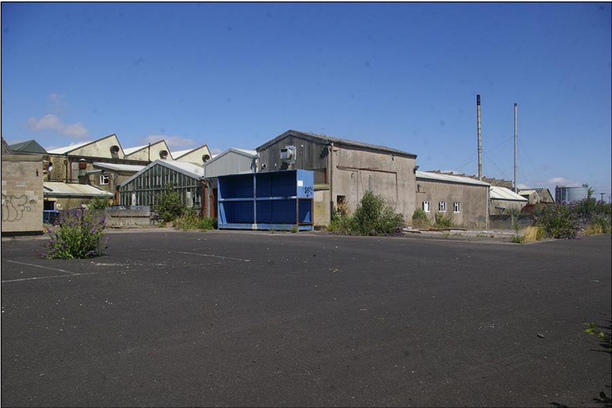
SITE SHOT SHOWING WORKSHOPS (BUILDING 5) AND ROOF OF MAIN FACTORY (BUILDING 1) BEHIND; VIEWED FROM THE SOUTH.
