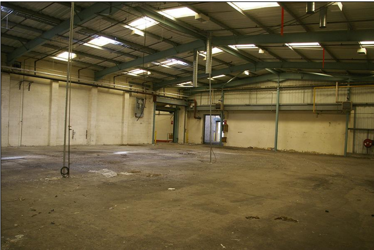
MIDDLE WAREHOUSE TO BUILDING 15; VIEWED FROM THE NORTH.
