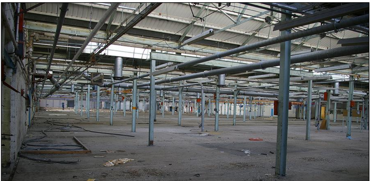
FIGURE 2: INTERIOR OF MAIN FACTORY (BUILDING 1); VIEWED FROM THE NORTH-EAST.
