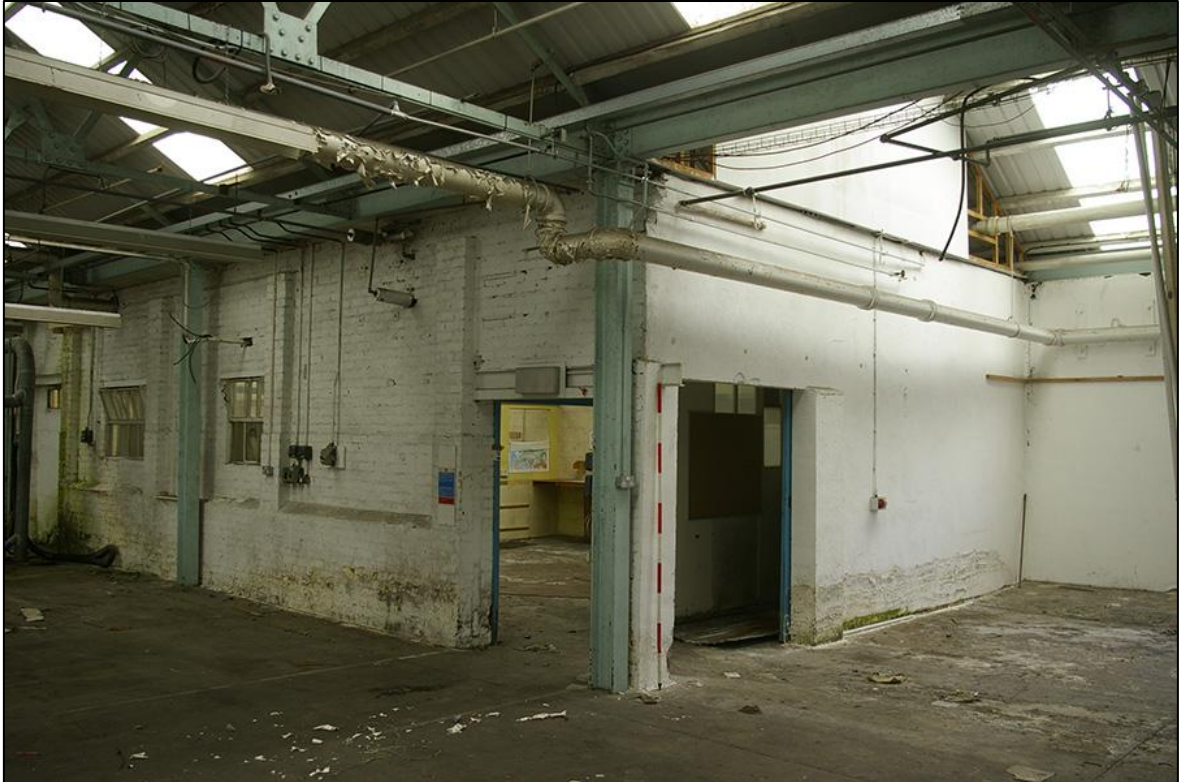
FIGURE 6: FORMER EXTERIOR OF BRICK SHED (BUILDING 7); VIEWED FROM THE WEST (2M SCALE).
