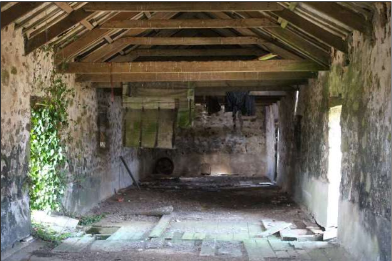
190. B9A FF INTERIOR; VIEWED FROM THE SOUTH-WEST.
