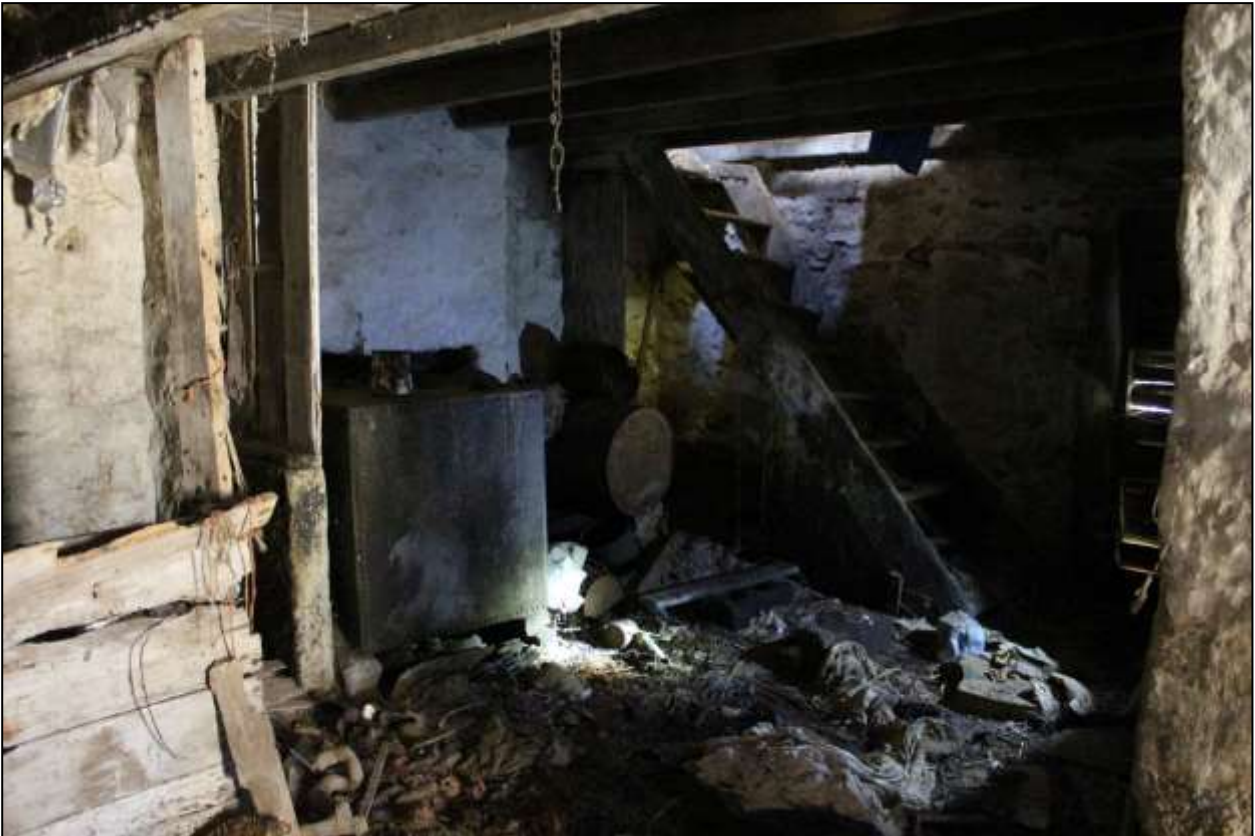
125. B3 GF INTERIOR; VIEWED FROM THE NORTH.
