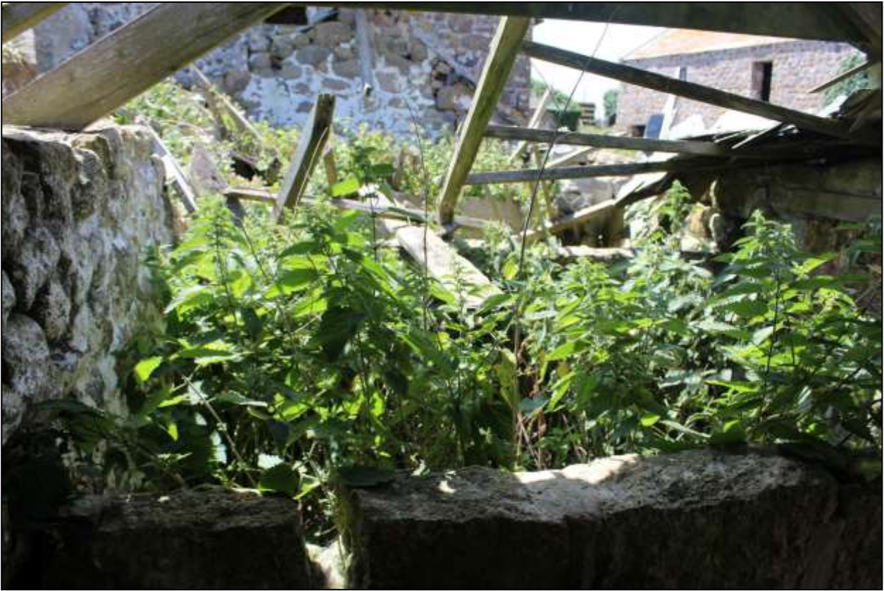
100. B1 INTERIOR, THE GRANITE SLAB PIGSTY WALLS; VIEWED FROM THE NORTH-EAST.
