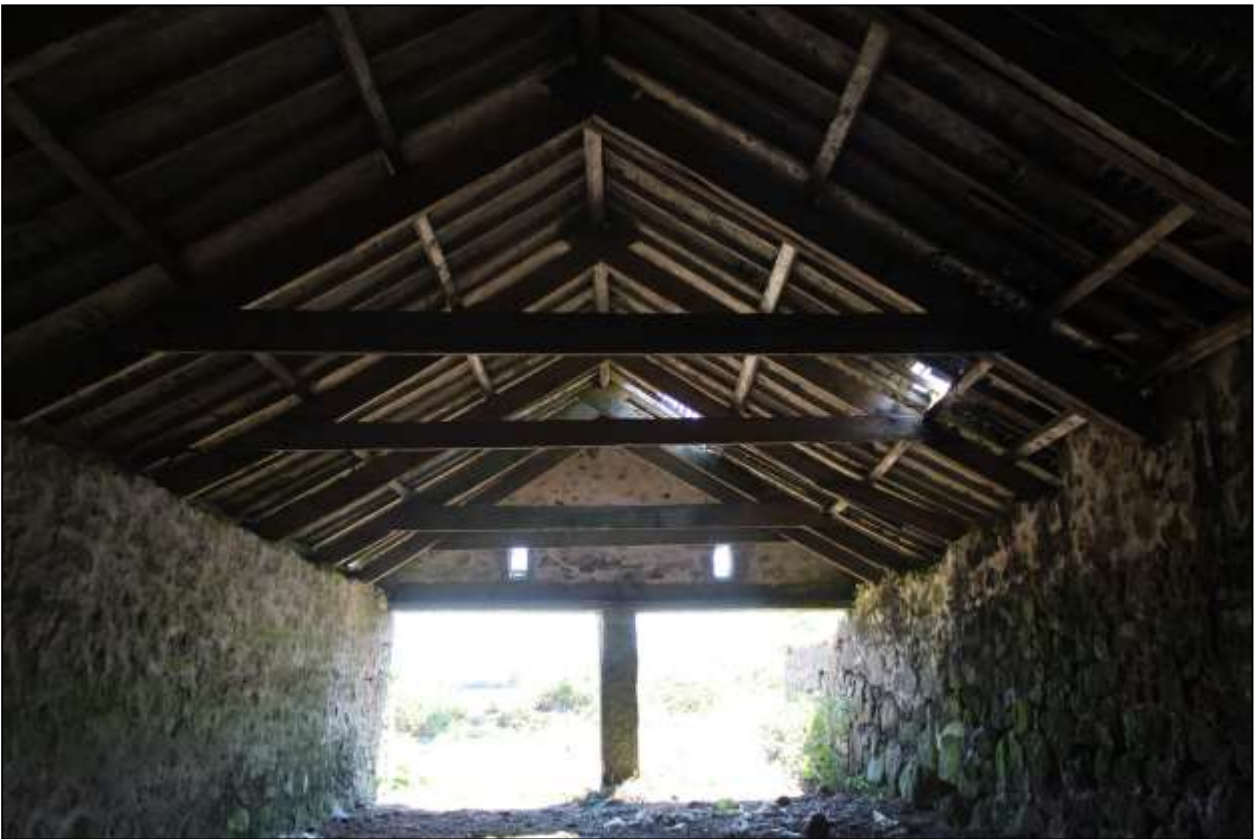
221. B11 INTERIOR; VIEWED FROM THE NORTH-WEST.
