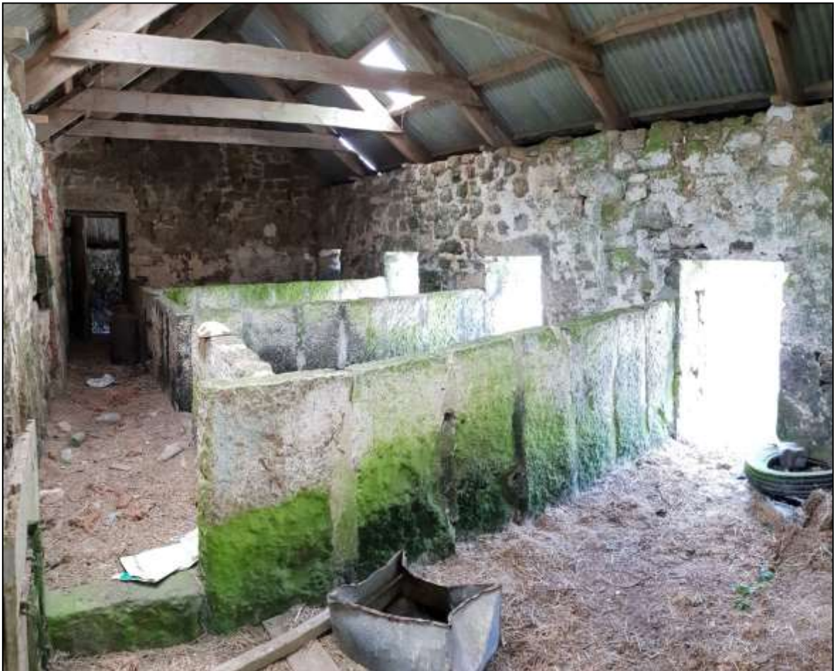
FIGURE 10: INTERIOR OF B2B FROM LARGER PEN AT NORTH-EAST END, WITH GRANITE SLAB PARTITIONS TO PENS AND FEED PASSAGE DOWN THE SOUTH-EAST SIDE (LEFT); VIEWED FROM THE EAST.
