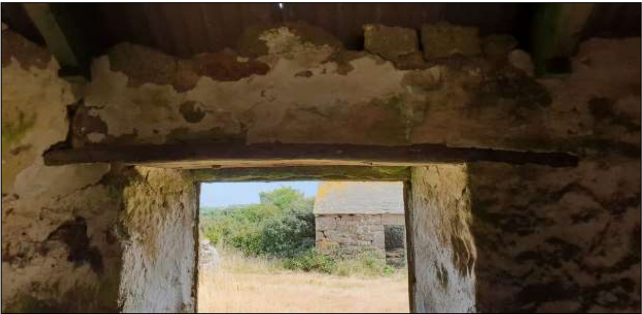
209. B10B INTERIOR, DETAIL OF LINTEL OVER GW17; VIEWED FROM THE NORTH-WEST.
