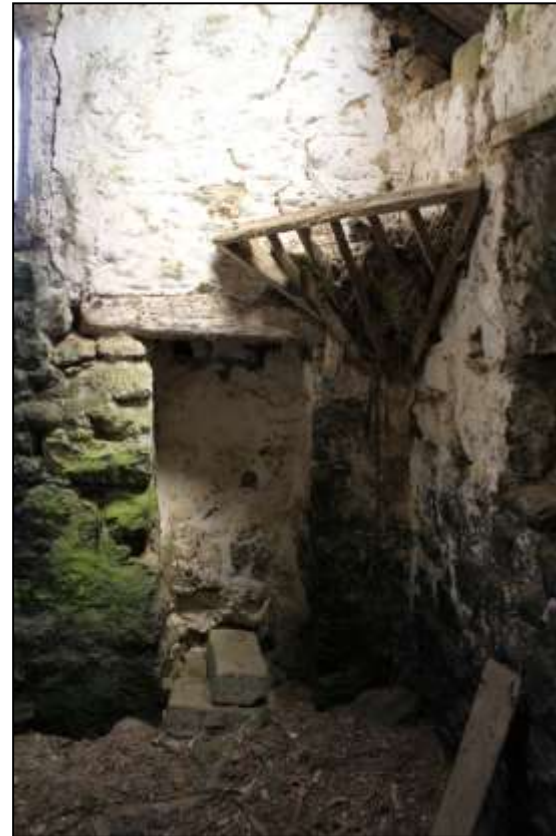
104. LEFT: B1A INTERIOR, THE NORTH-EAST GABLE WALL WITH FW1 WITH REUSED GRANITE FIREPLACE JAMBS; VIEWED FROM THE SOUTH.
