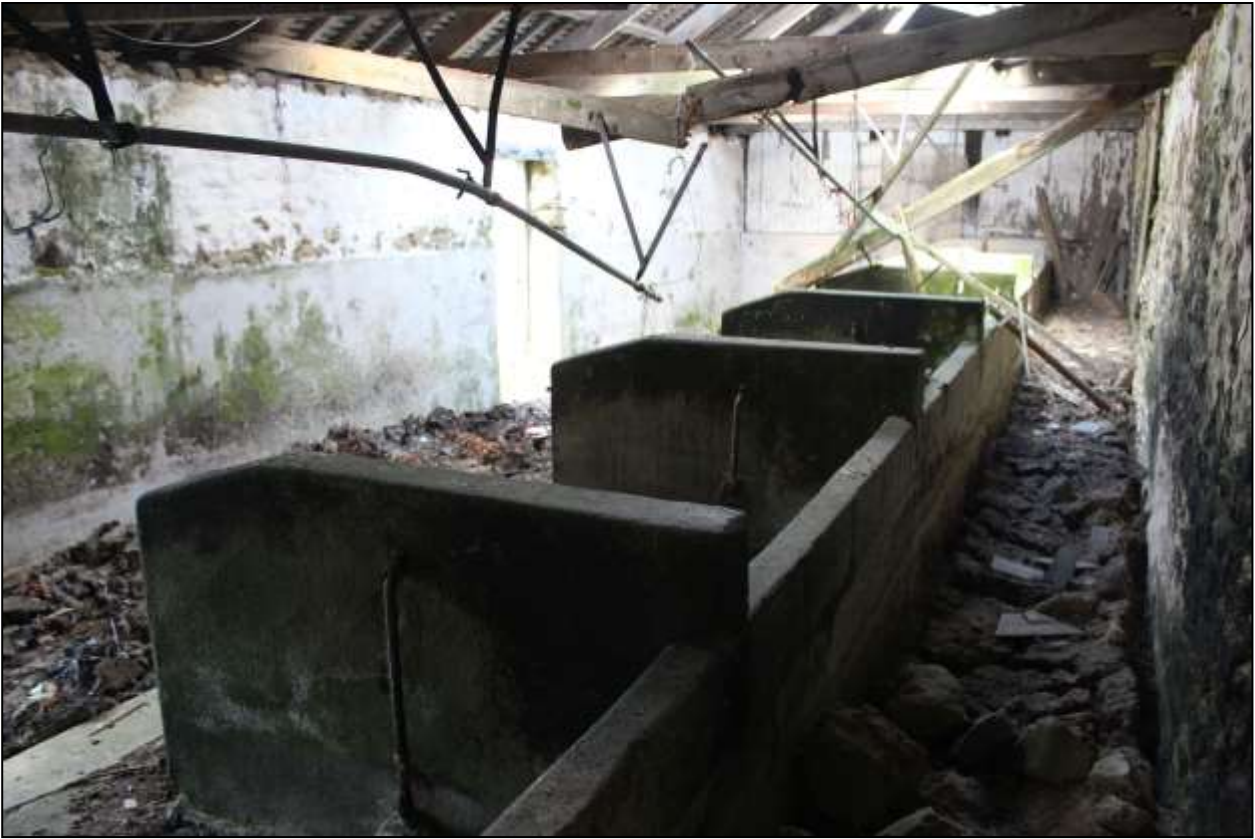
143. B4 INTERIOR, VIEWED FROM THE SSW (SCALE 2M).
