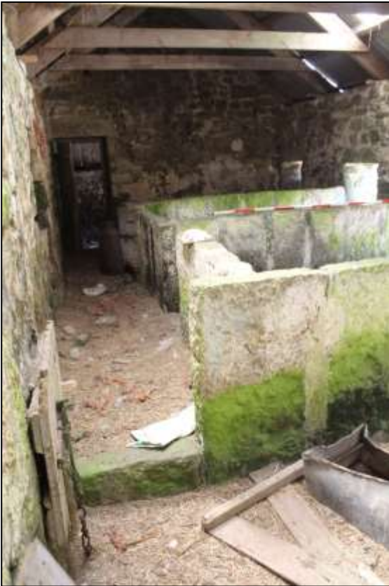
109. LEFT: B1B INTERIOR, THE GRANITE SLAB PIGSTY WALLS, VIEW ALONG THE FEED PASSAGE; VIEWED FROM THE NORTH-EAST (SCALE 2M).
