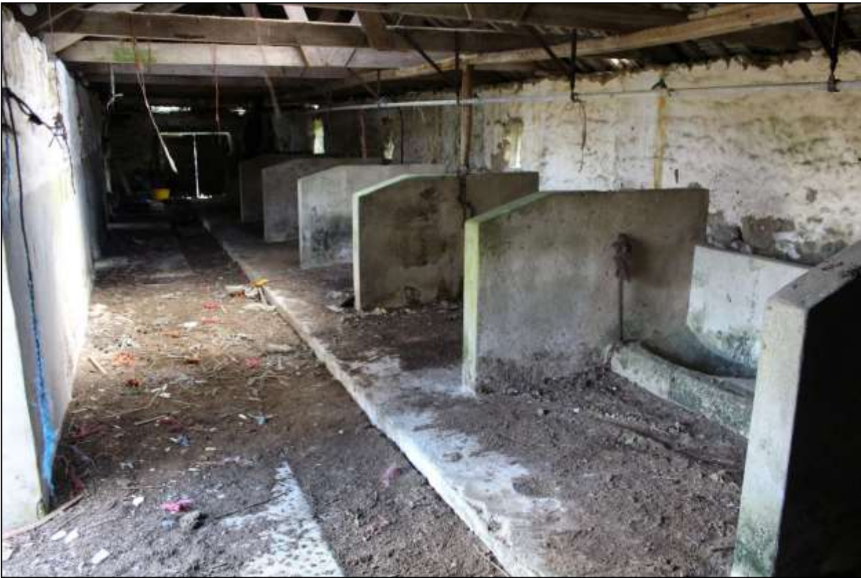
171. B7 INTERIOR; VIEWED FROM THE WEST.
