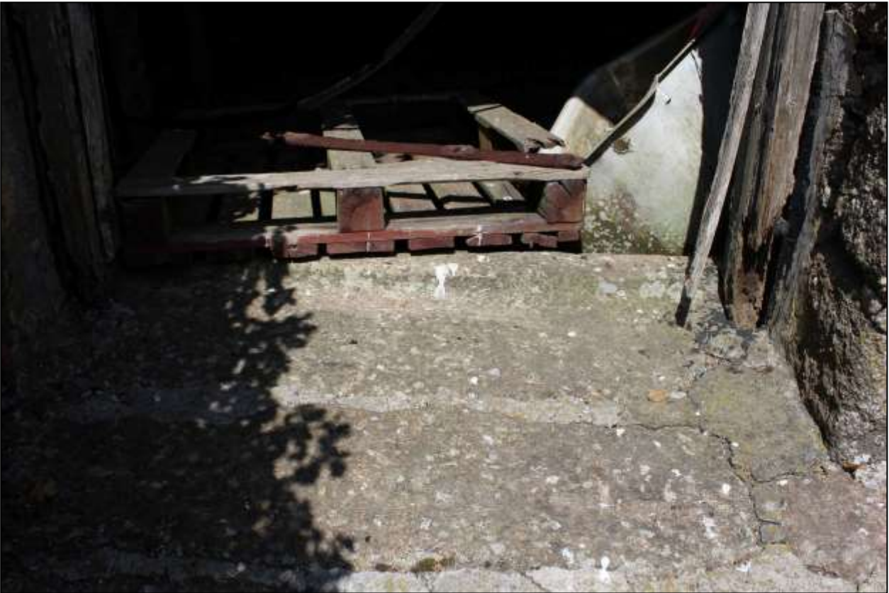
188. B9B FF INTERIOR, DETAIL OF SHAPED GRANITE SLAB REUSED AS THRESHOLD OF FD1; VIEWED FROM THE SOUTH-WEST.
