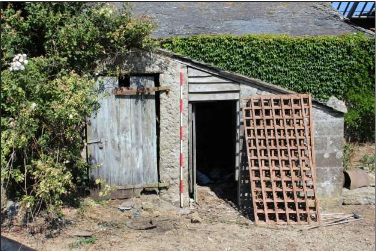
21. B5 AND B6, SOUTH-EAST ELEVATIONS; VIEWED FROM THE SOUTH-EAST (SCALE 2M).
