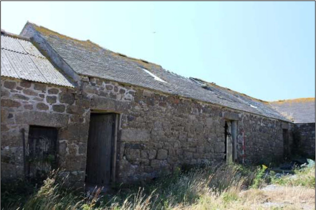
43. B4, NORTH-WEST ELEVATION; VIEWED FROM THE NORTH (SCALE 2M).
