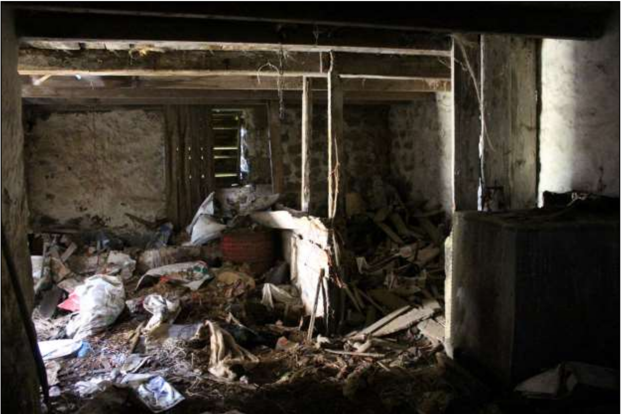
127. B3 GF INTERIOR, VIEWED FROM THE SOUTH-WEST.
