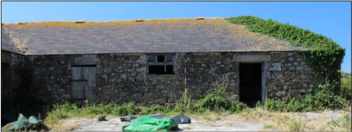
FIGURE 21: B7, NORTH-EAST ELEVATION; VIEWED FROM THE NORTH-EAST (SCALE 2M).
