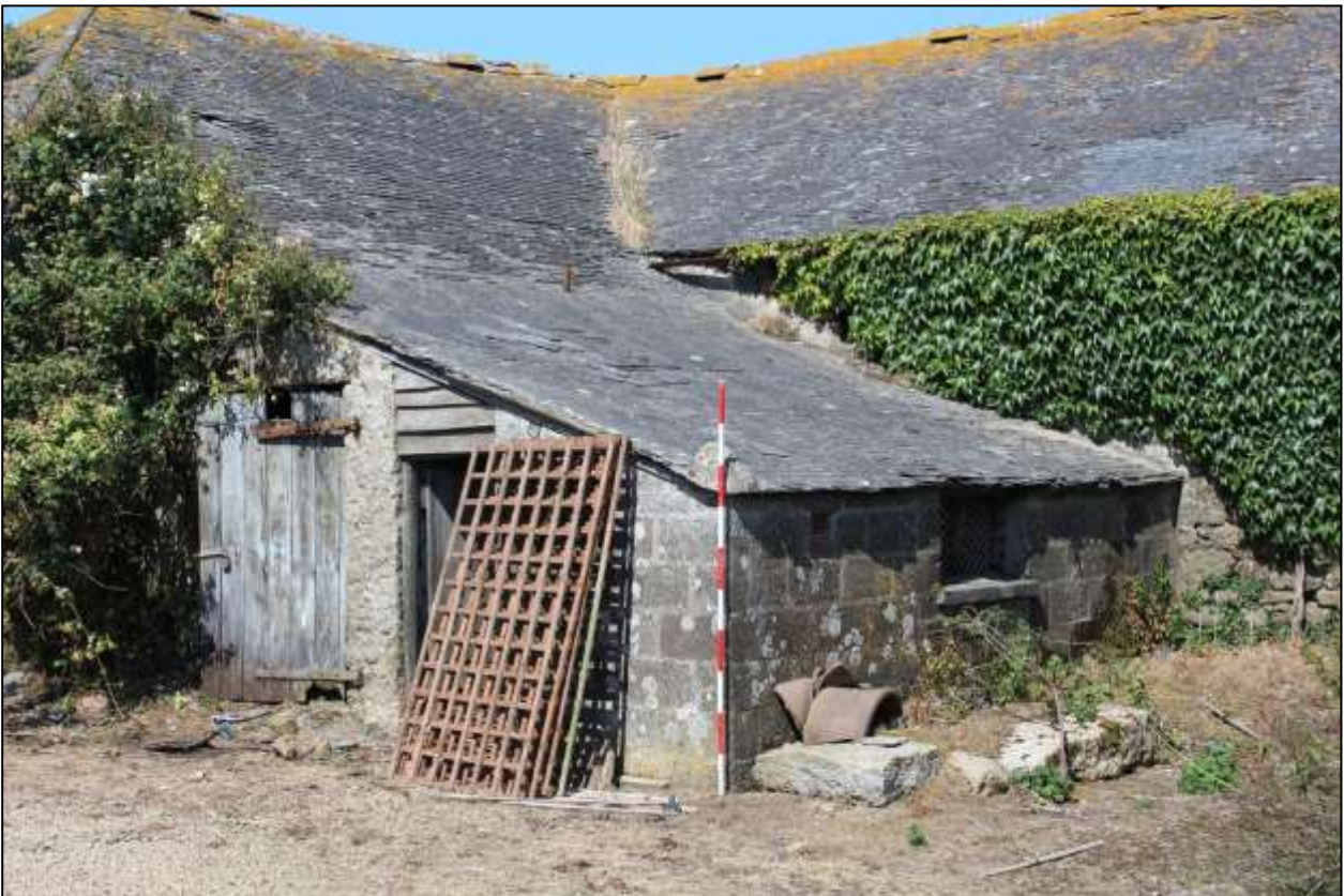
17. B5 AND B6, SOUTH-EAST ELEVATIONS; VIEWED FROM THE EAST (SCALE 2M).
