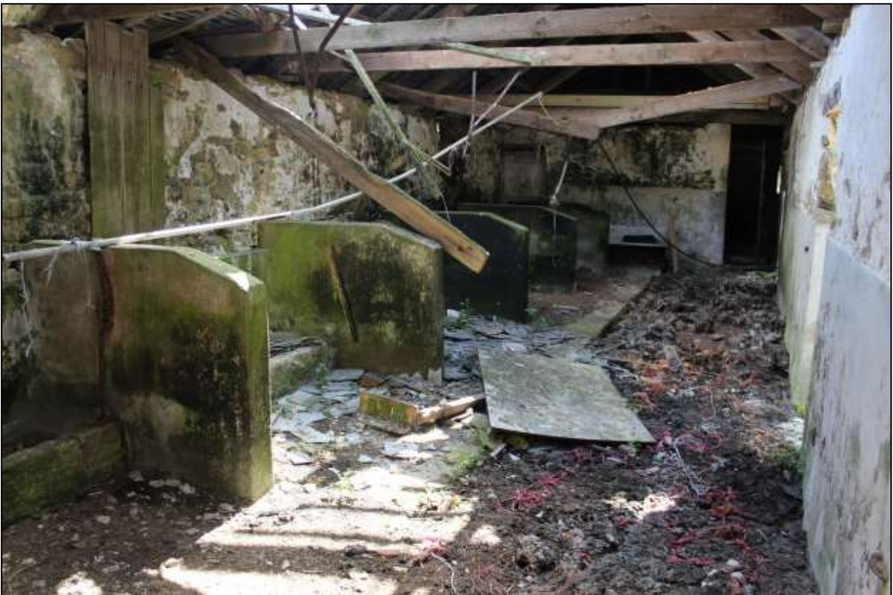
146. B4 INTERIOR, VIEWED FROM THE NNE.
