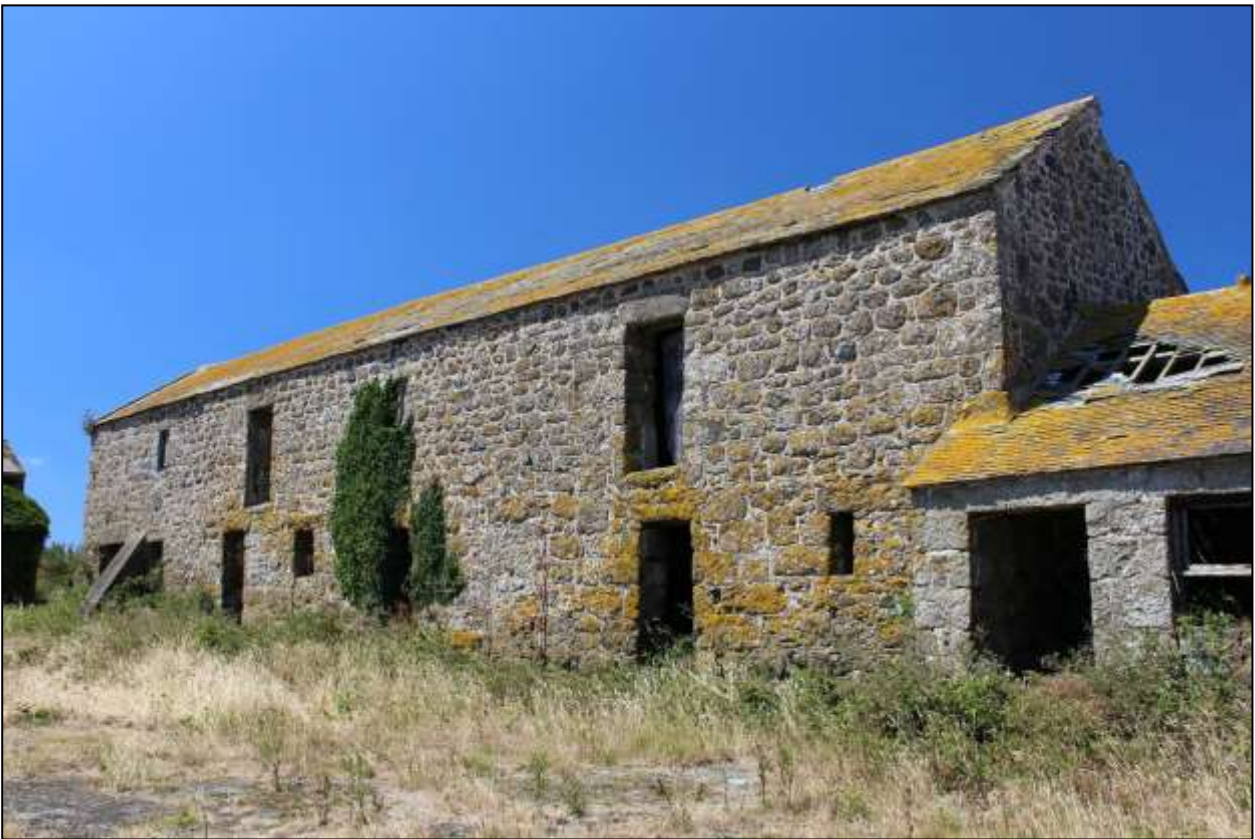
77. B9, SOUTH-EAST ELEVATION; VIEWED FROM THE NORTH-EAST (SCALE 2M).
