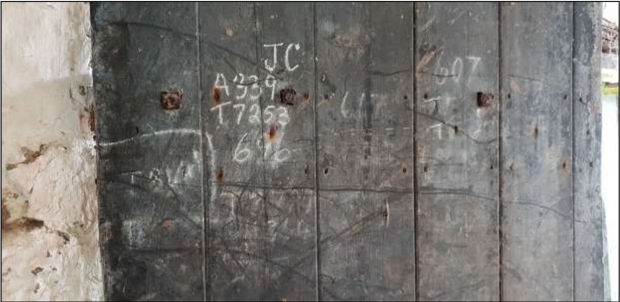
170. B7 INTERIOR, DETAIL OF THE TALLY MARKS ON GD9; VIEWED FROM THE SOUTH.
