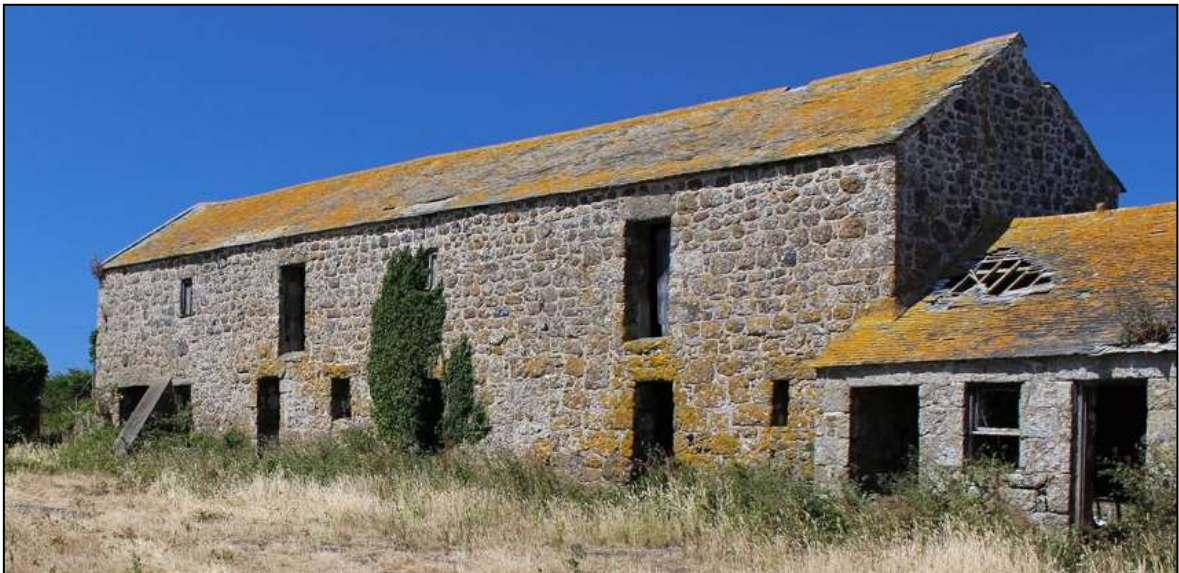
FIGURE 25: B9, SOUTH-EAST ELEVATION; VIEWED FROM THE EAST.
