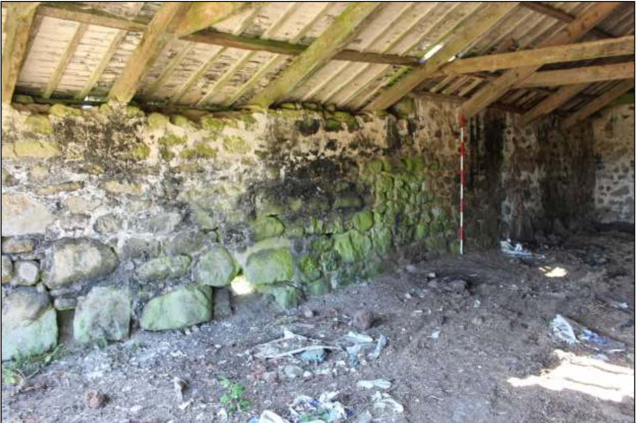
218. B11 INTERIOR; VIEWED FROM THE NNE (SCALE 2M).
