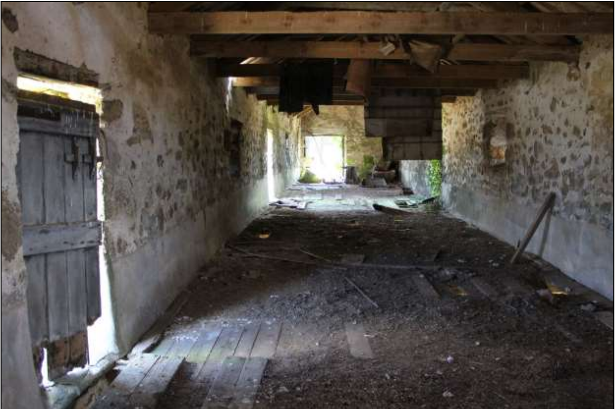
191. B9A AND B9B FF INTERIOR; VIEWED FROM THE NORTH-WEST.
