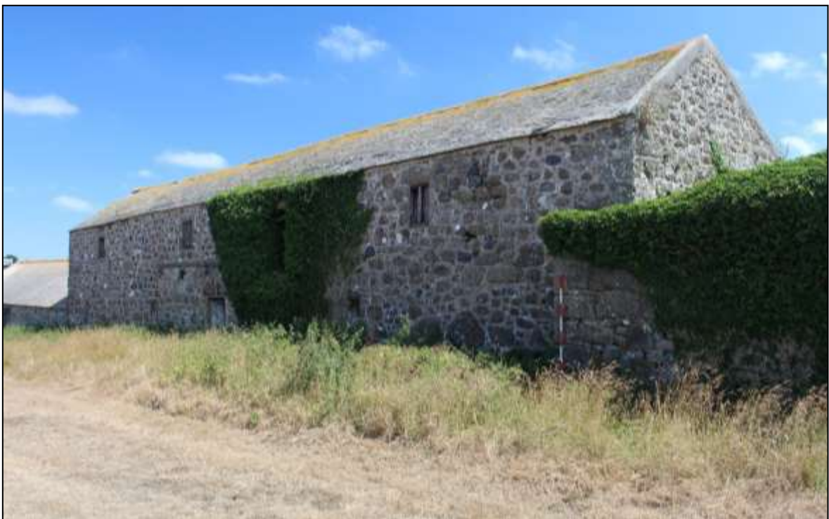
FIGURE 26: B9, NORTH-WEST ELEVATION; VIEWED FROM THE WSW (SCALE 2M).
