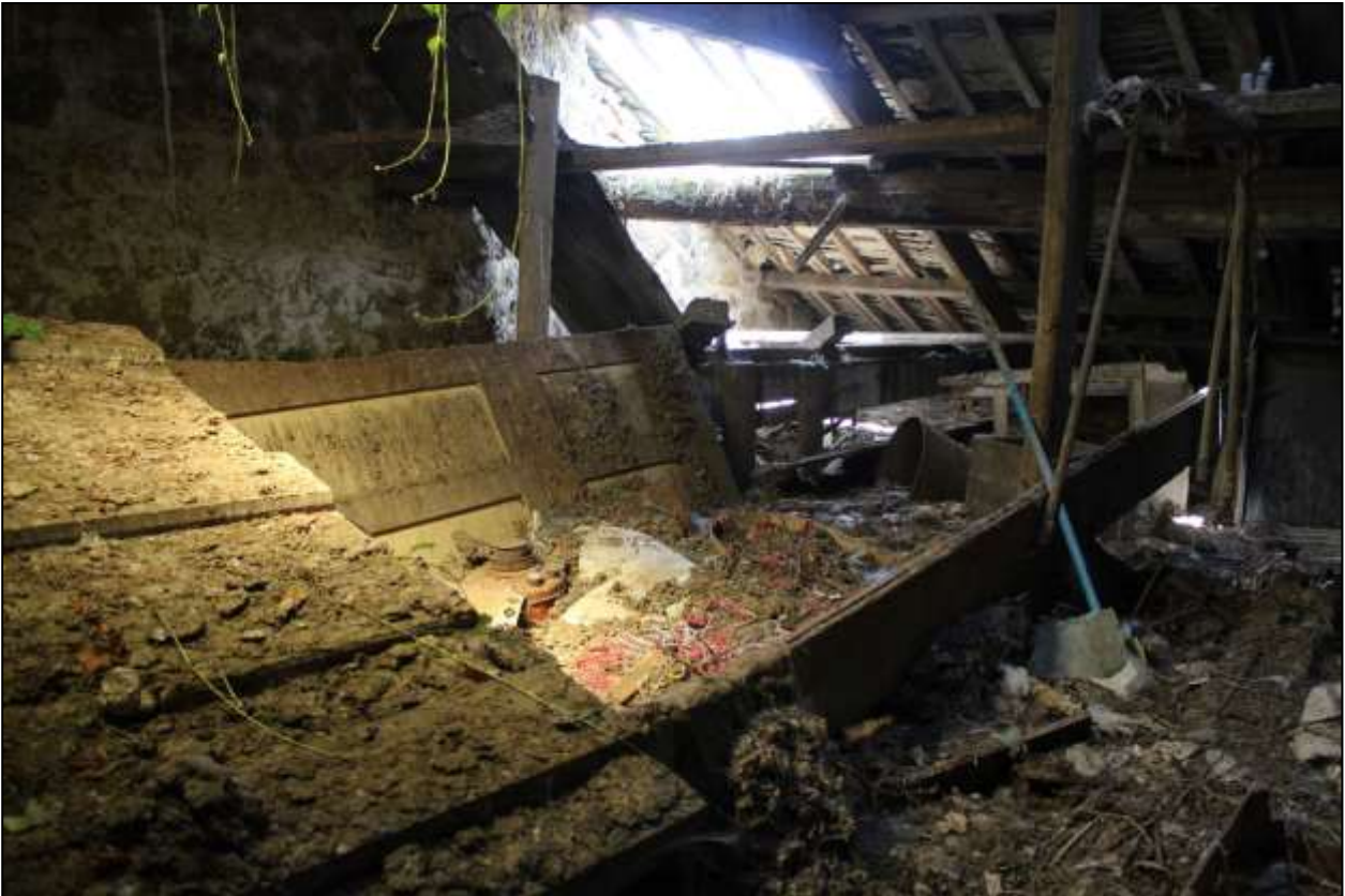
131. B3 FF INTERIOR, VIEWED FROM THE SOUTH.
