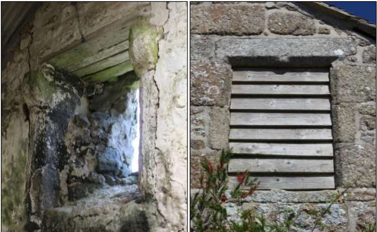
LEFT FIGURE 11: INTERIOR OF B2A; WINDOW IN NORTH-EAST GABLE RE-USING PARTS FROM A 17 TH CENTURY GRANITE FIREPLACE; VIEWED FROM THE SOUTH.
