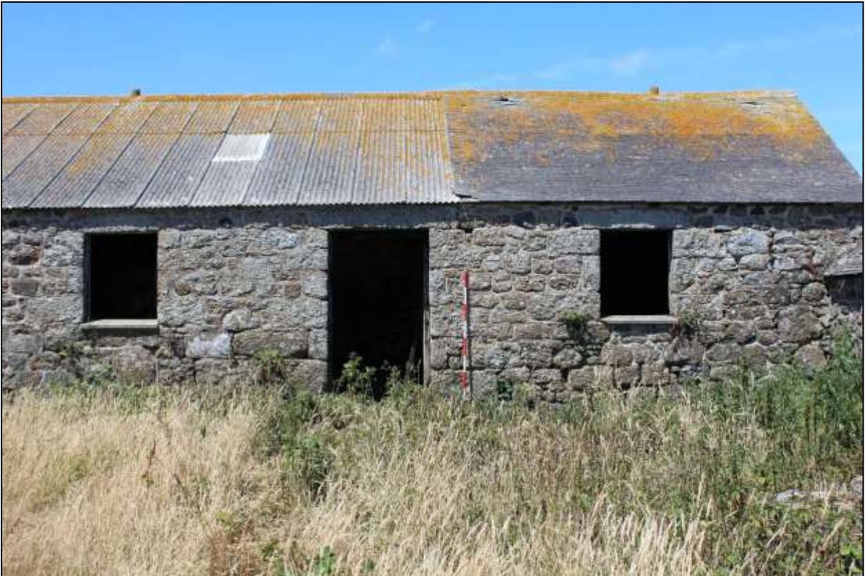
80. B10b, SOUTH-EAST ELEVATION; VIEWED FROM THE SOUTH-EAST (SCALE 2M).
