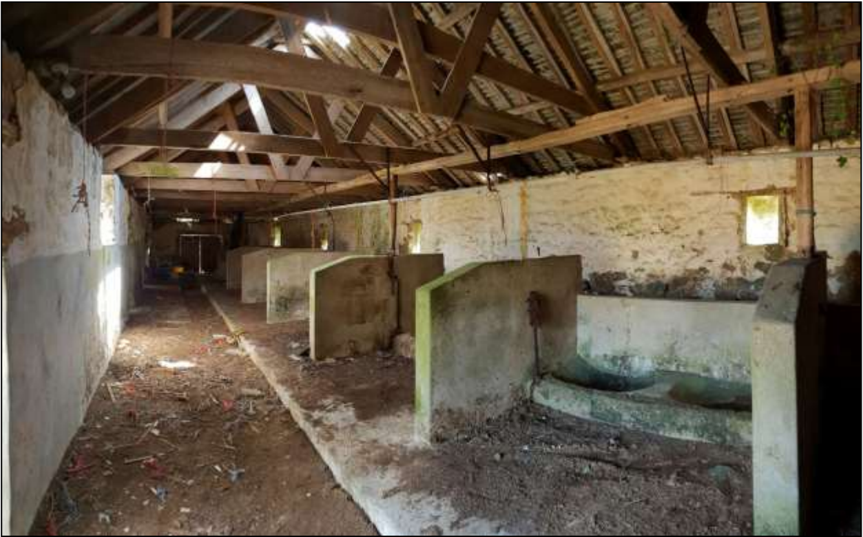
172. B7 INTERIOR; VIEWED FROM THE WEST.
