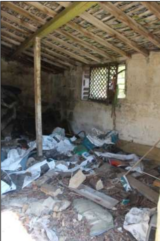
150. B5 INTERIOR; VIEWED FROM THE SSE.
