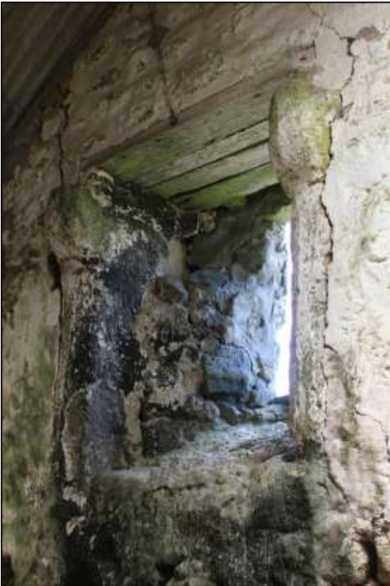
104. LEFT: B1A INTERIOR, THE NORTH-EAST GABLE WALL WITH FW1 WITH REUSED GRANITE FIREPLACE JAMBS; VIEWED FROM THE SOUTH.
