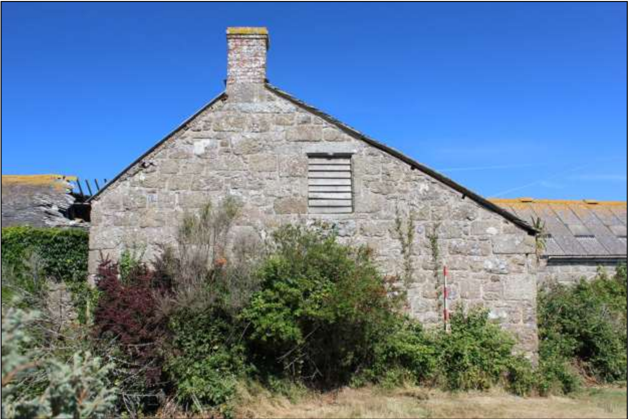
7. B3, SOUTH-EAST ELEVATION; VIEWED FROM THE SOUTH-EAST (SCALE 2M).
