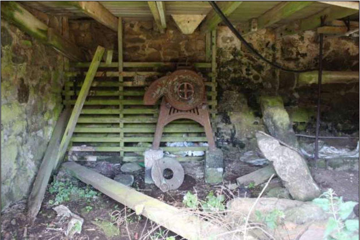
176. B9B GF INTERIOR, DETAIL OF BELT-DRIVEN ROLLER MILL; VIEWED FROM THE SOUTH-EAST.
