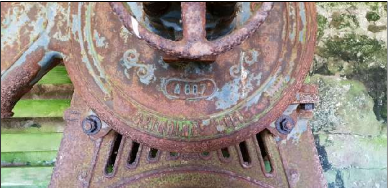
179. B9B GF INTERIOR, DETAIL OF BELT-DRIVEN ROLLER MILL; VIEWED FROM THE SOUTH-EAST.
