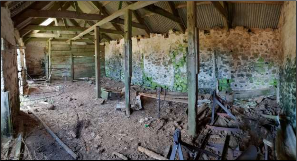
200. B10B INTERIOR; VIEWED FROM THE ENE.
