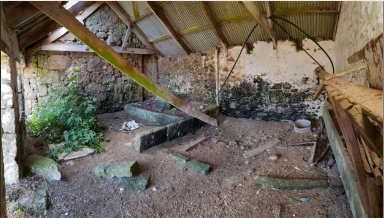
198. B10A INTERIOR; VIEWED FROM THE NORTH.
