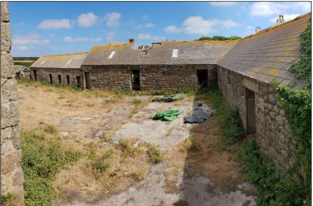
32. B7 AND B4, NORTH-EAST AND NORTH-WEST ELEVATIONS; VIEWED FROM THE WEST (SCALE 2M).
