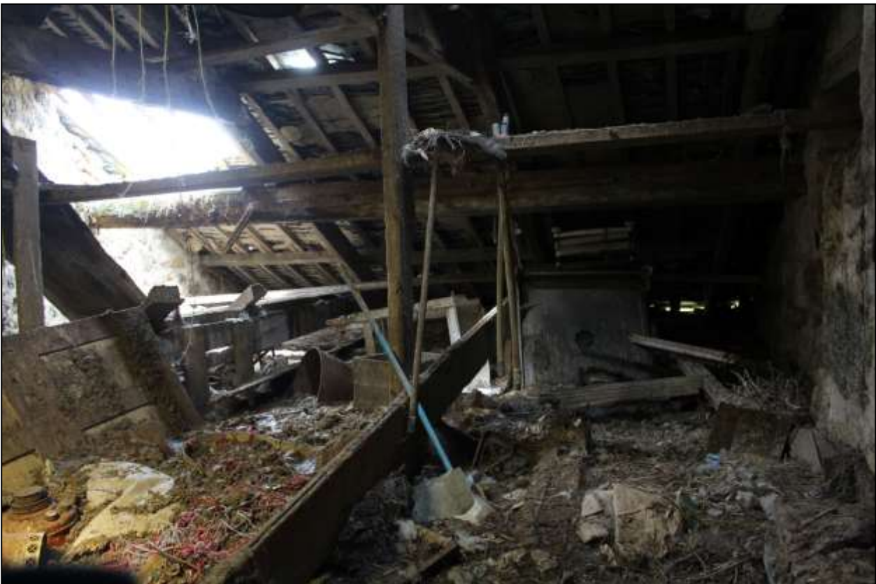
130. B3 FF INTERIOR, VIEWED FROM THE SSW.
