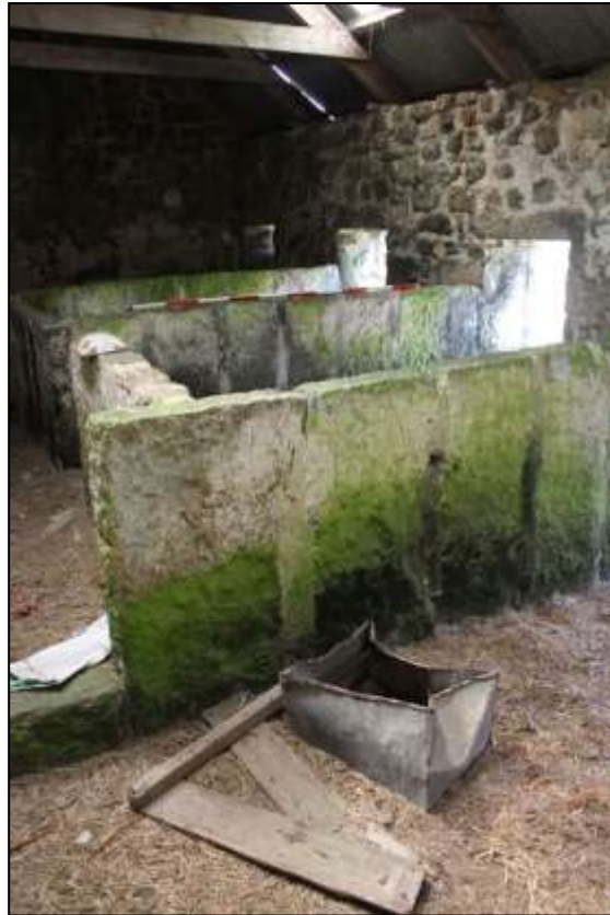
109. LEFT: B1B INTERIOR, THE GRANITE SLAB PIGSTY WALLS, VIEW ALONG THE FEED PASSAGE; VIEWED FROM THE NORTH-EAST (SCALE 2M).
