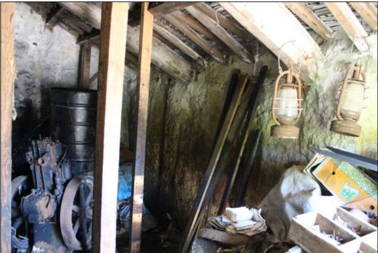
159. B6 INTERIOR, THE NORTH-EAST WALL COMPRISED OF GRANITE ORTHOSTATS; VIEWED FROM THE SSE.
