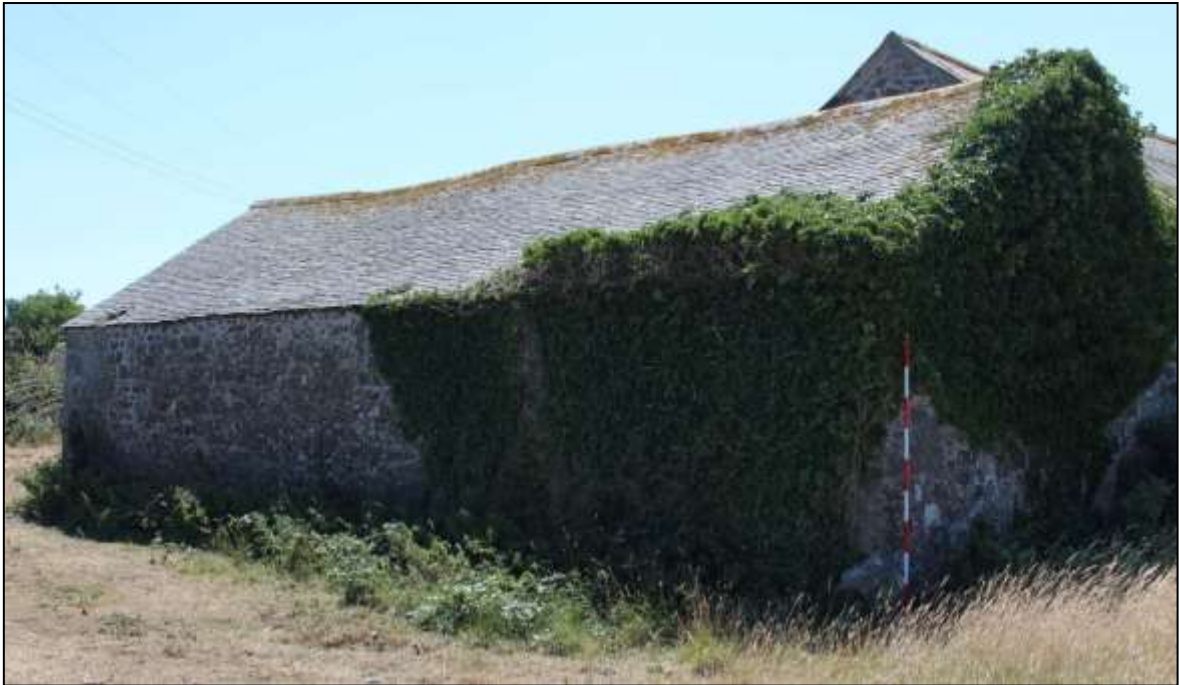
FIGURE 34: B11, NORTH-EAST AND NORTH-WEST ELEVATIONS; VIEWED FROM THE NORTH (SCALE 2M).
