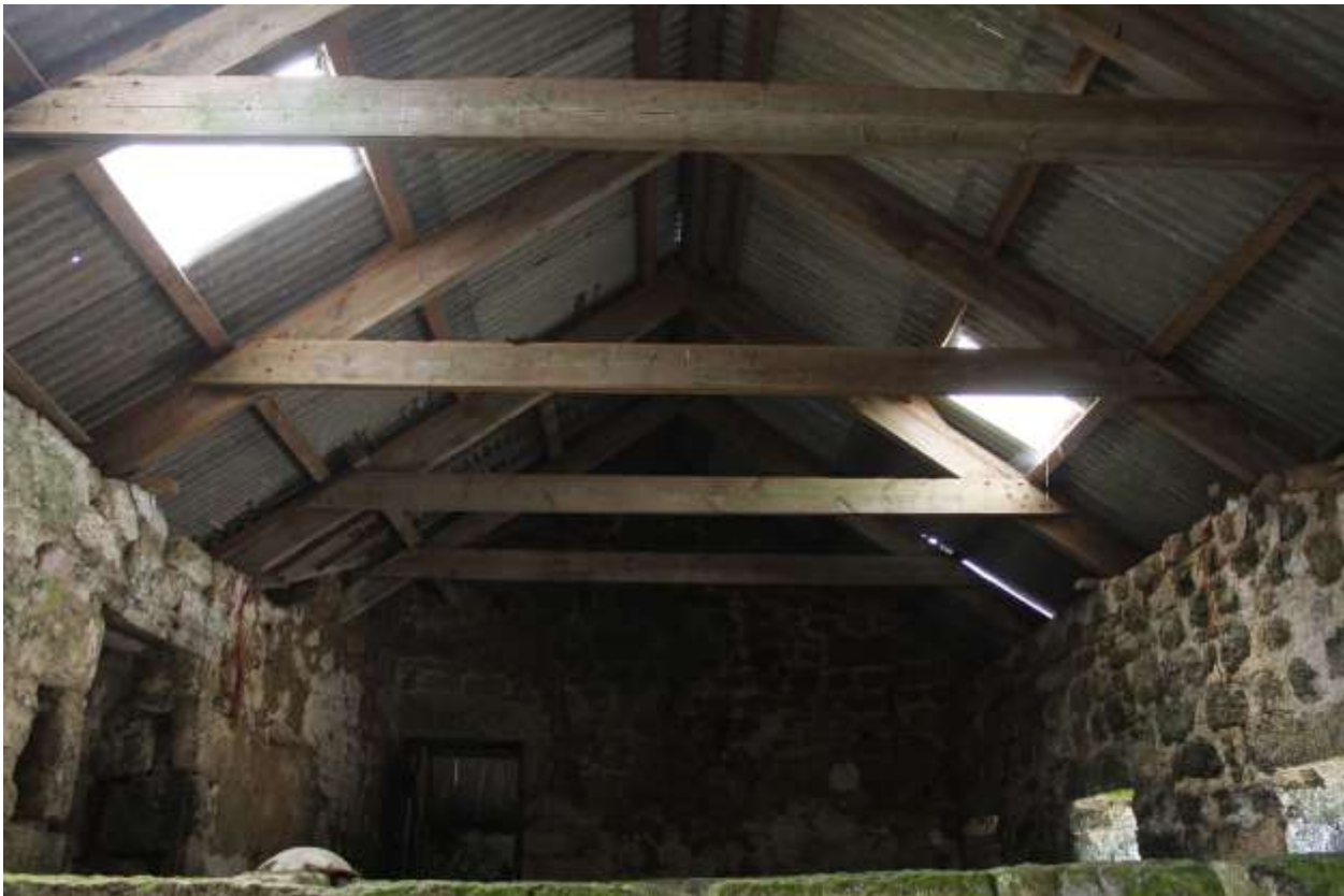
118. B1B INTERIOR, DETAIL OF THE ROOF STRUCTURE; VIEWED FROM THE NORTH-EAST.
