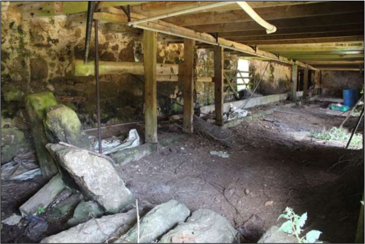
183. B9A GF INTERIOR; VIEWED FROM THE SOUTH.
