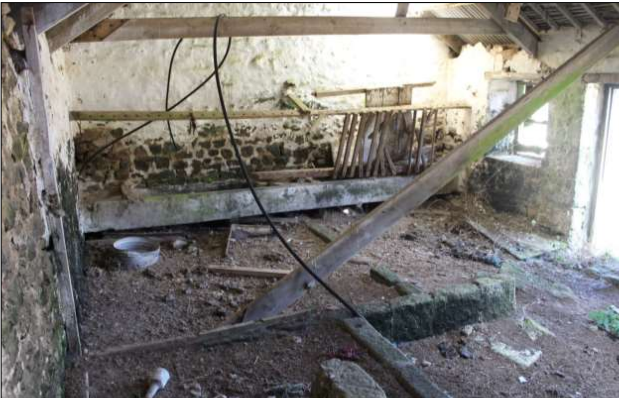
195. B10A INTERIOR; VIEWED FROM THE SOUTH.
