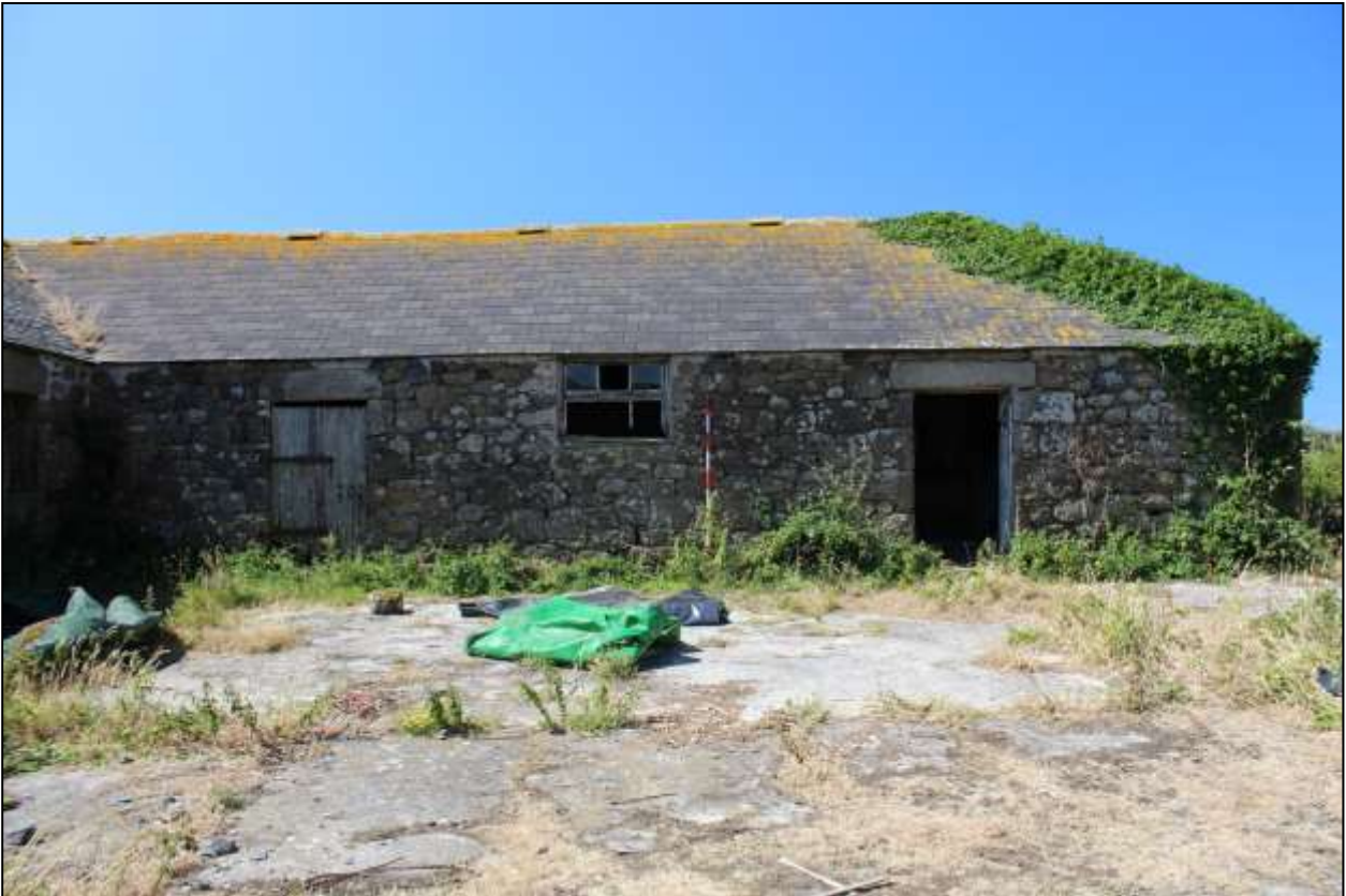
33. B7, NORTH-EAST ELEVATION; VIEWED FROM THE NORTH-EAST (SCALE 2M).
