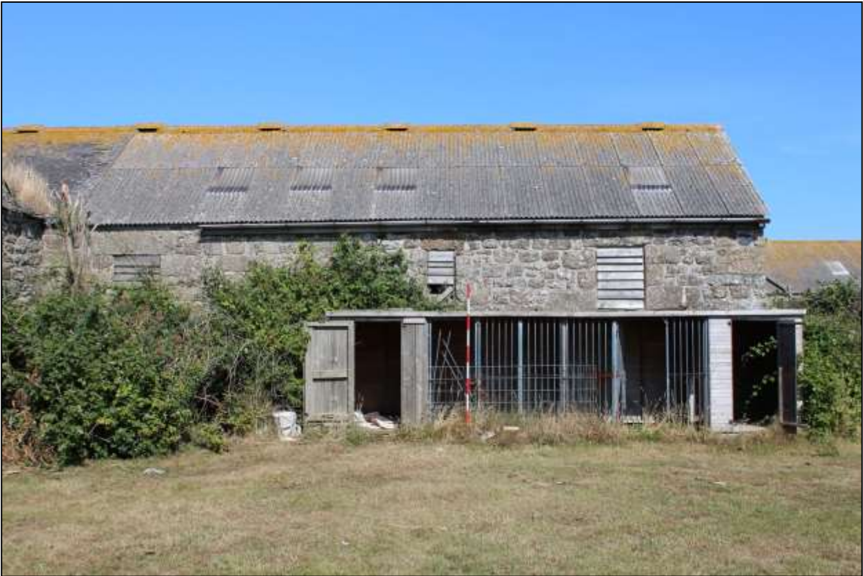
3. B2, SOUTH-EAST ELEVATION; VIEWED FROM THE SOUTH-EAST (SCALE 2M).
