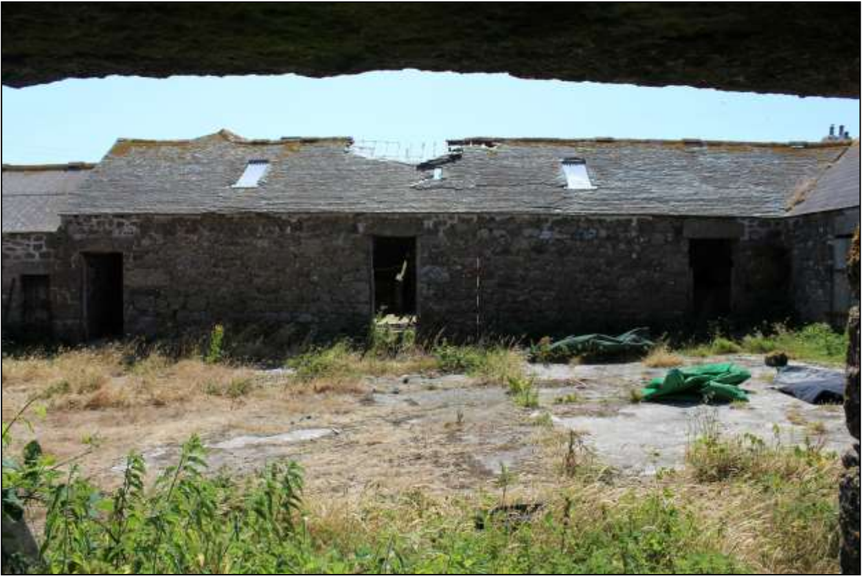
37. B4, NORTH-WEST ELEVATION; VIEWED FROM THE NORTH-WEST (SCALE 2M).
