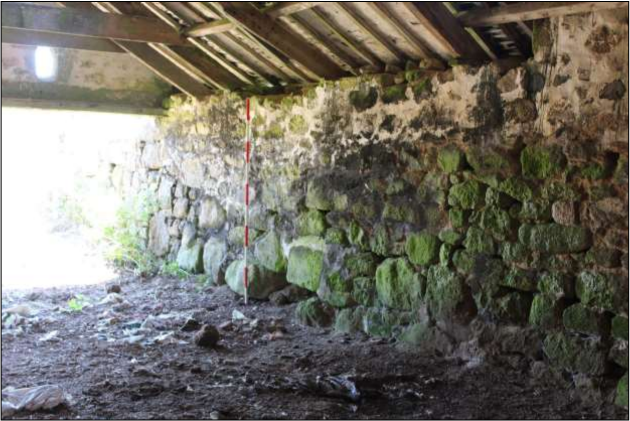
220. B11 INTERIOR, THE SOUTH-WEST WALL; VIEWED FROM THE NORTH (SCALE 2M).
