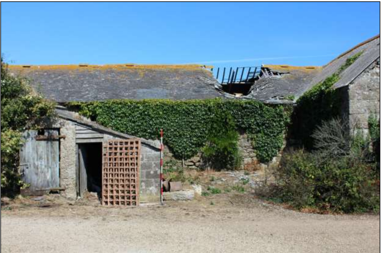
15. B4, SOUTH-EAST ELEVATION; VIEWED FROM THE SOUTH-EAST (SCALE 2M).
