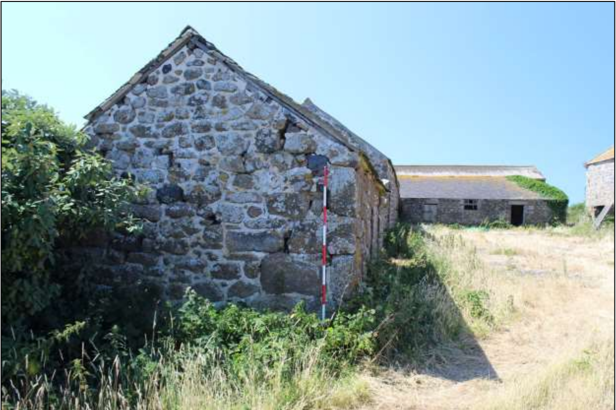
59. B1, NORTH-EAST GABLE ELEVATION; VIEWED FROM THE NORTH-EAST (SCALE 2M).
