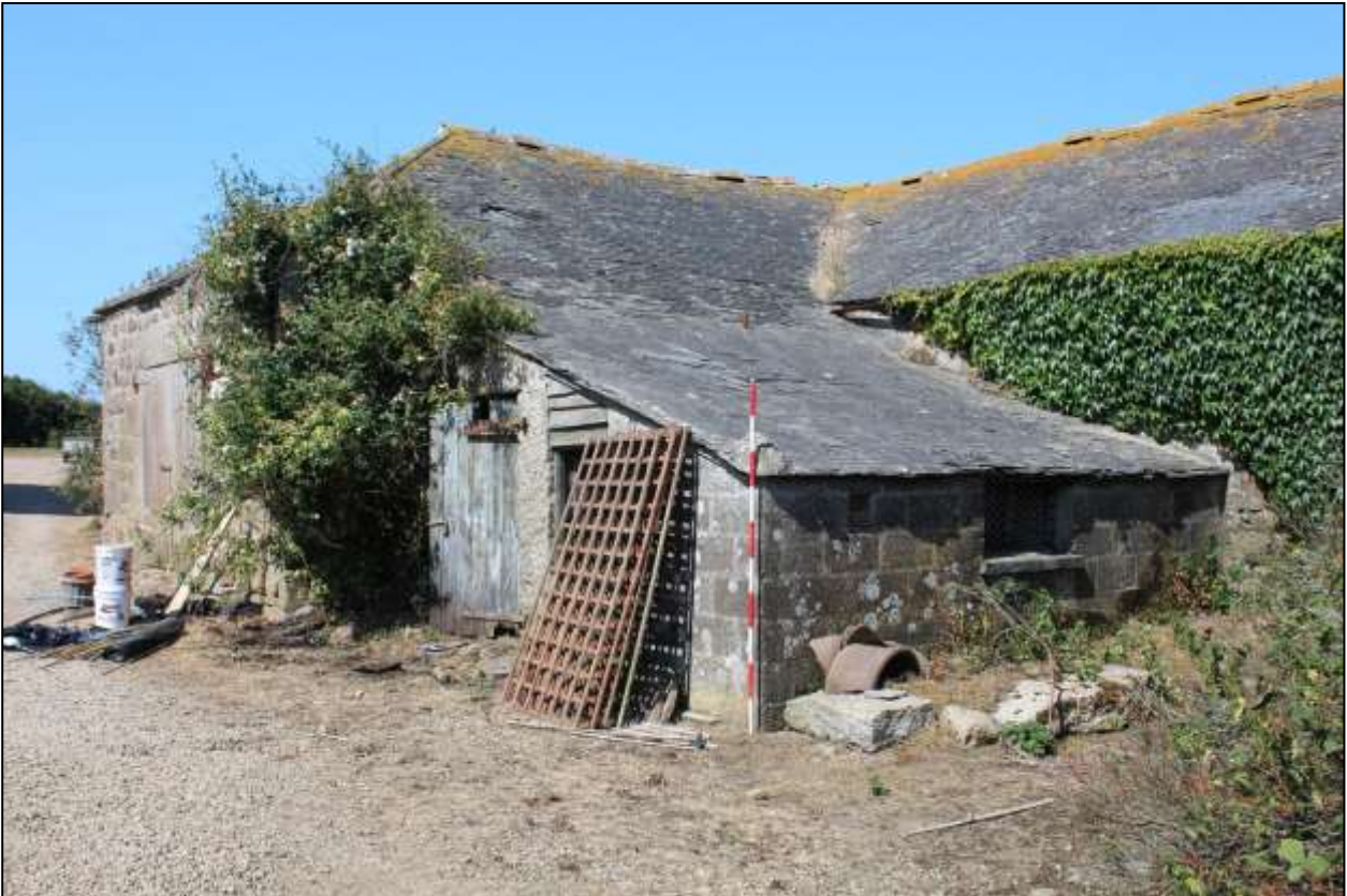
18. B5 AND B6, SOUTH-EAST ELEVATIONS; VIEWED FROM THE EAST (SCALE 2M).
