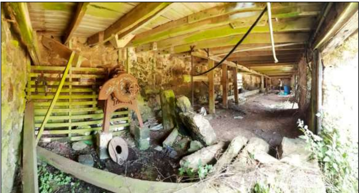
FIGURE 28: B9, GROUND FLOOR INTERIOR. NOTE THE 20 TH CENTURY GRAIN MILL, BELT-DRIVEN FROM TRACTOR OR ENGINE IN B8 TO LEFT OF IMAGE. VIEWED FROM THE SOUTH.
