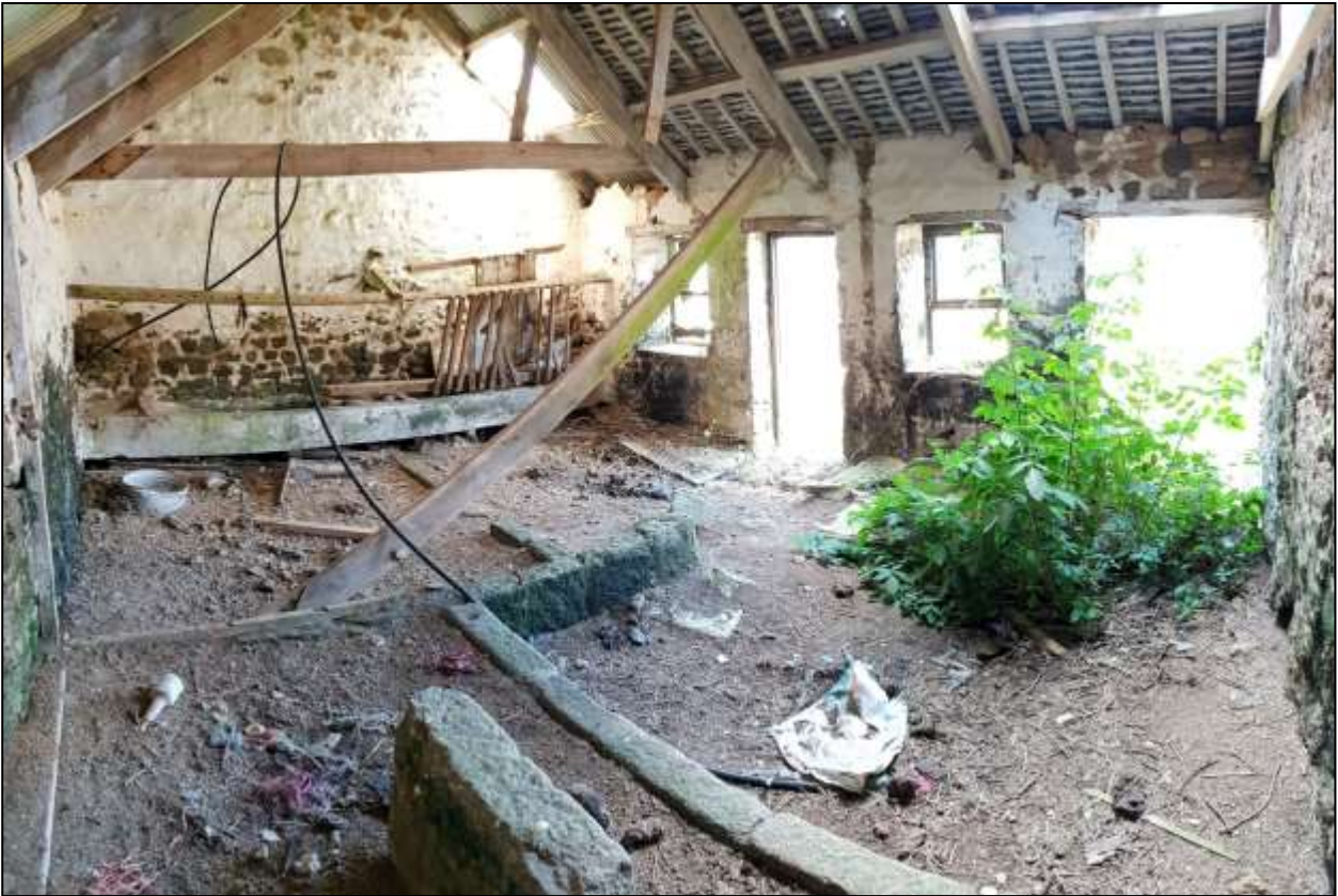
196. B10A INTERIOR; VIEWED FROM THE SOUTH.
