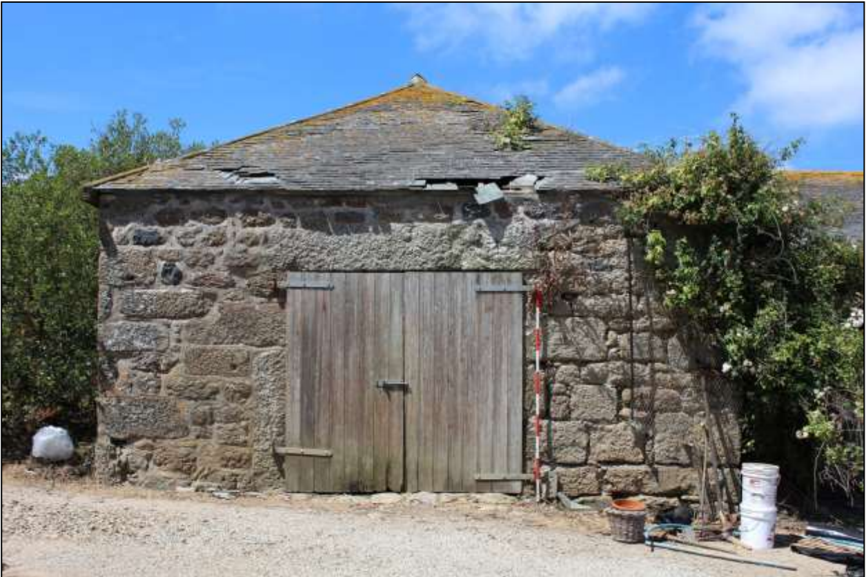
22. B7, SOUTH-EAST ELEVATION; VIEWED FROM THE SOUTH-EAST (SCALE 2M).
