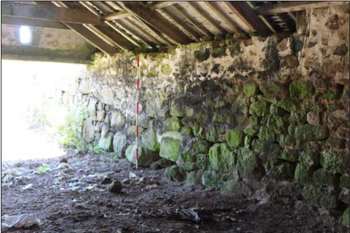
FIGURE 36: B11, INTERIOR, SHOWING THE MORTARED RUBBLE WALL SITTING ON AN OLDER YARD WALL OF MASSIVE BOULDERS; VIEWED FROM THE NORTH (SCALE 2M).
