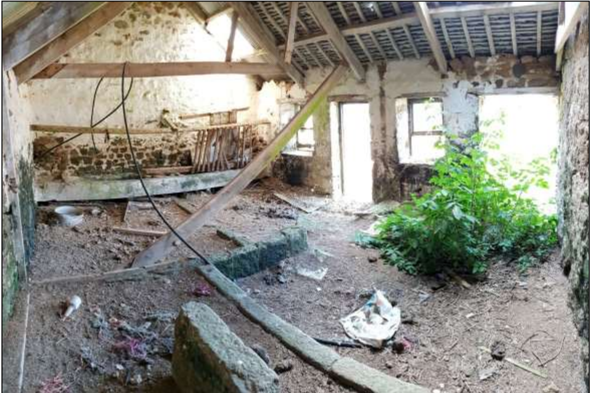
FIGURE 31: B10A, INTERIOR, THE REMAINS OF LOOSEBOXES FOR HORSES AS INDICATED BY THE GRANITE KERBS. VIEWED FROM THE WEST.
