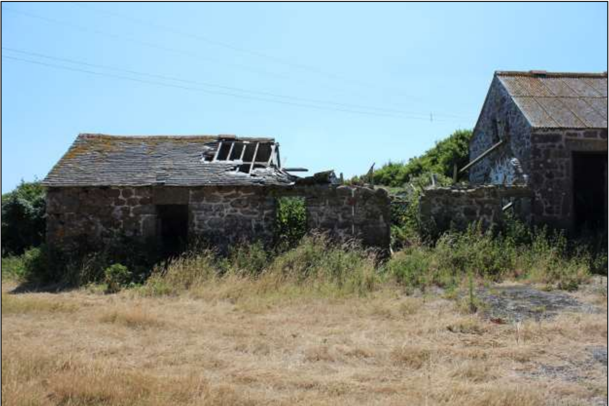
53. B1, NORTH-WEST ELEVATION; VIEWED FROM THE NORTH-WEST (SCALE 2M).
