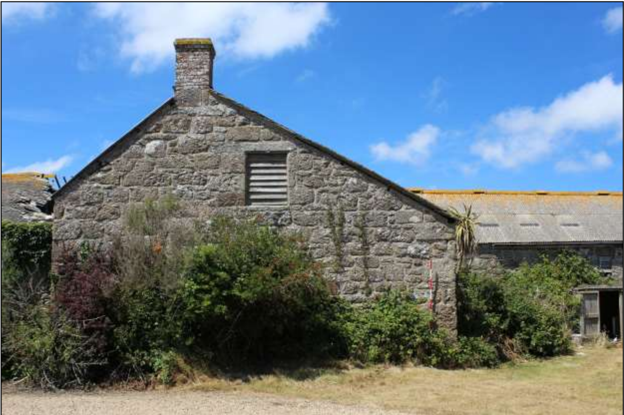
8. B3, SOUTH-EAST ELEVATION; VIEWED FROM THE SOUTH-EAST (SCALE 2M).
