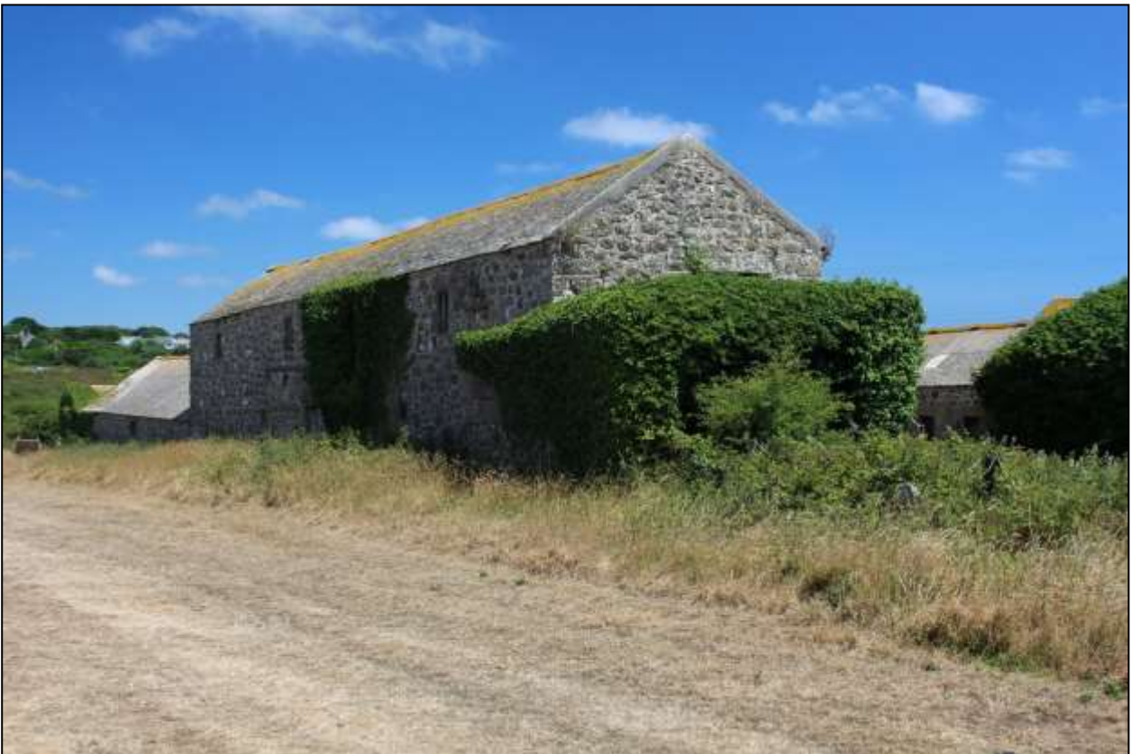
95. B9 AND B8, NORTH-WEST AND SOUTH-WEST ELEVATIONS; VIEWED FROM THE WEST.
