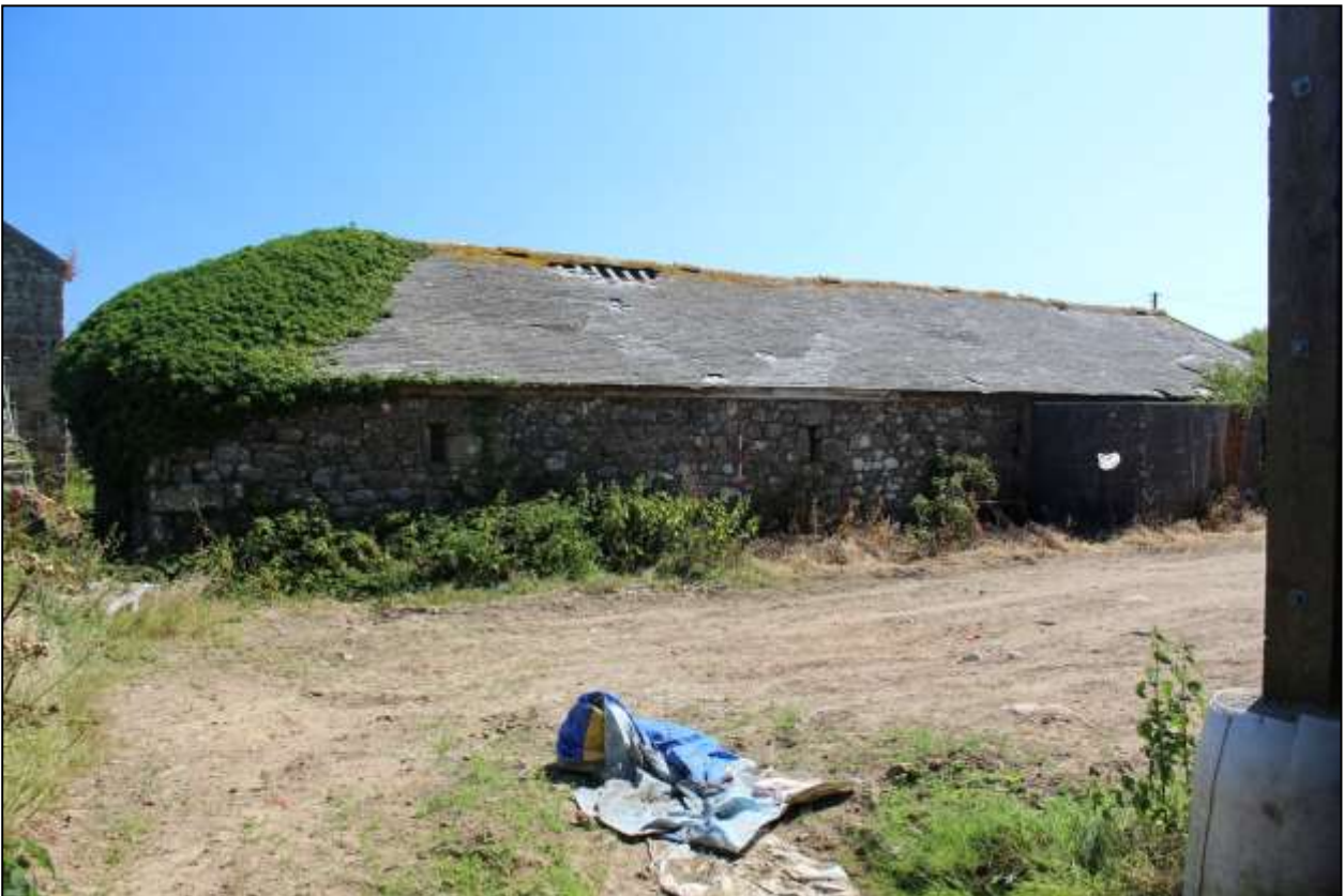
27. B7, THE WEST END OF THE SOUTH-WEST ELEVATION; VIEWED FROM THE WSW (SCALE 2M).
