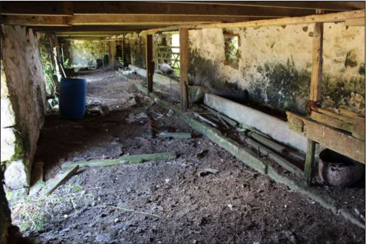
186. B9A GF INTERIOR; VIEWED FROM THE NNE.
