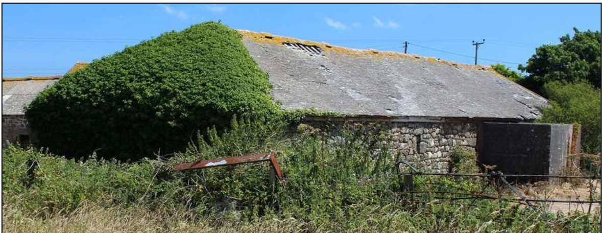
FIGURE 20: B7, NORTH-WEST AND SOUTH-WEST ELEVATIONS; VIEWED FROM THE WEST.
