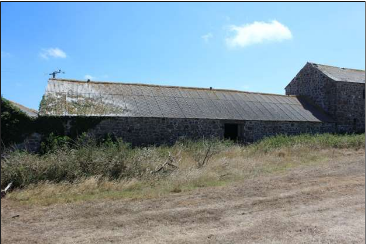
89. B10, NORTH-WEST ELEVATION; VIEWED FROM THE NNW (SCALE 2M).
