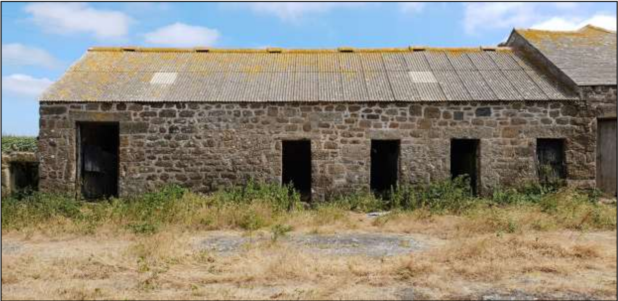
45. B2, NORTH-WEST ELEVATION; VIEWED FROM THE NORTH-WEST (SCALE 2M).
