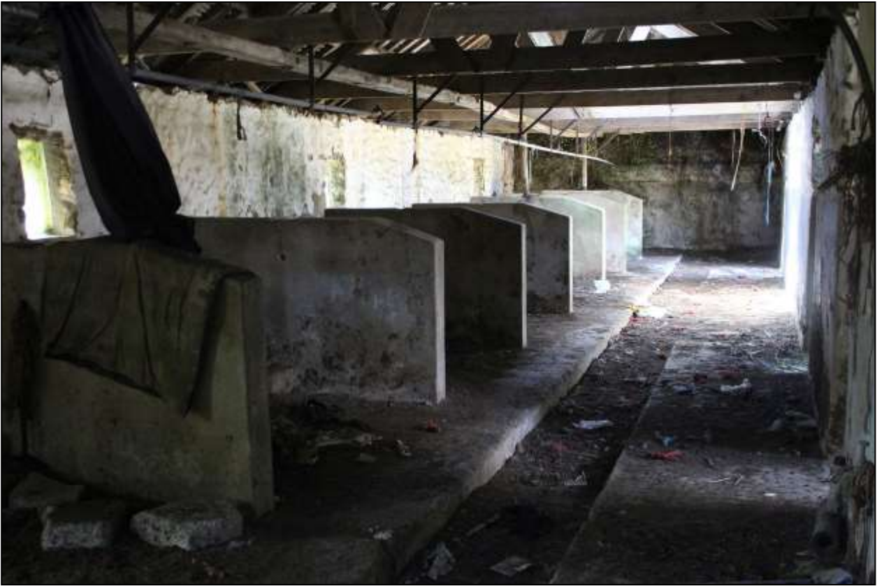
166. B7 INTERIOR; VIEWED FROM THE SOUTH-EAST.
