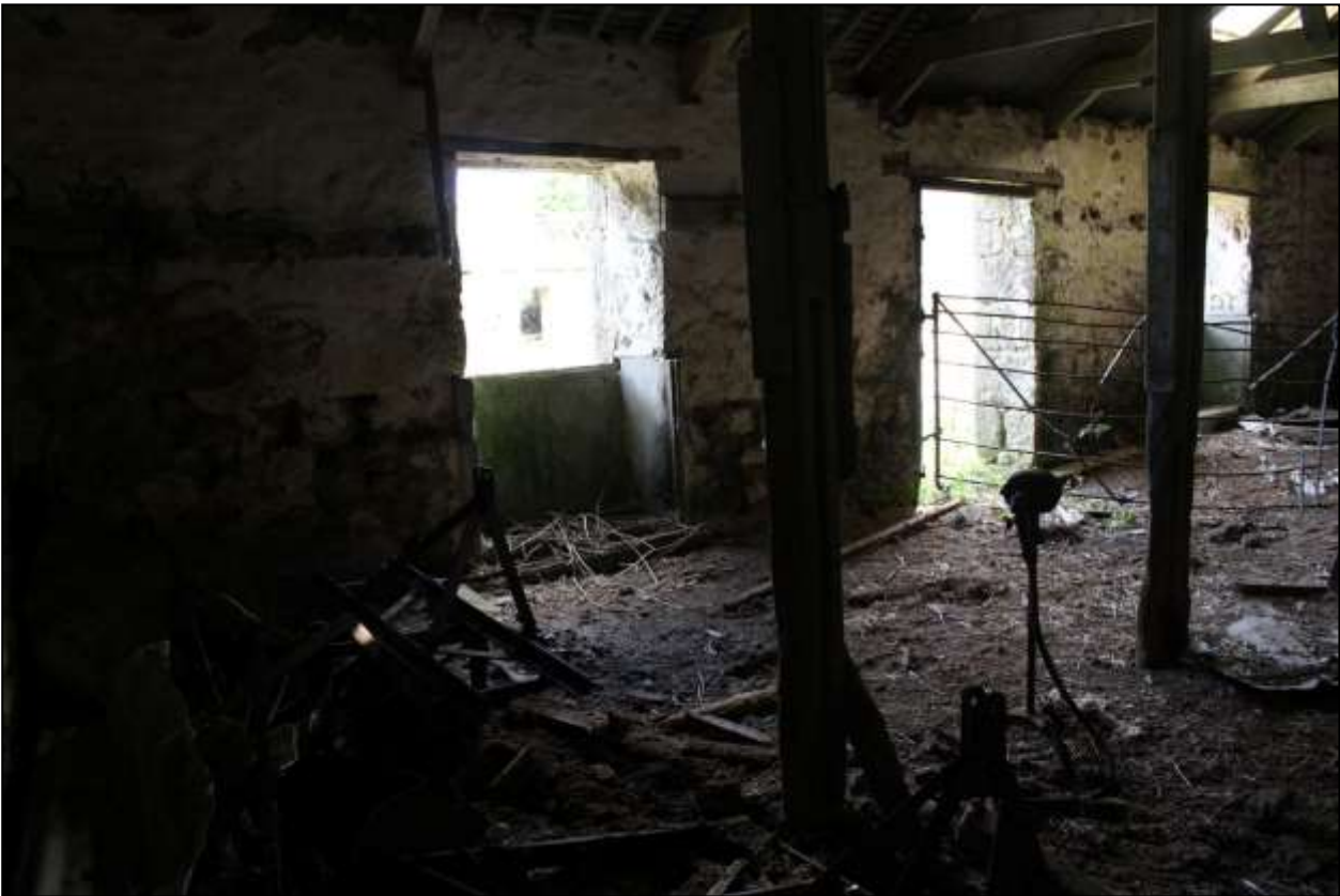
201. B10B INTERIOR; VIEWED FROM THE NORTH.
