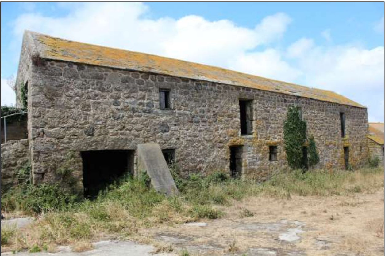
63. B9, SOUTH-EAST ELEVATION; VIEWED FROM THE SSE.
