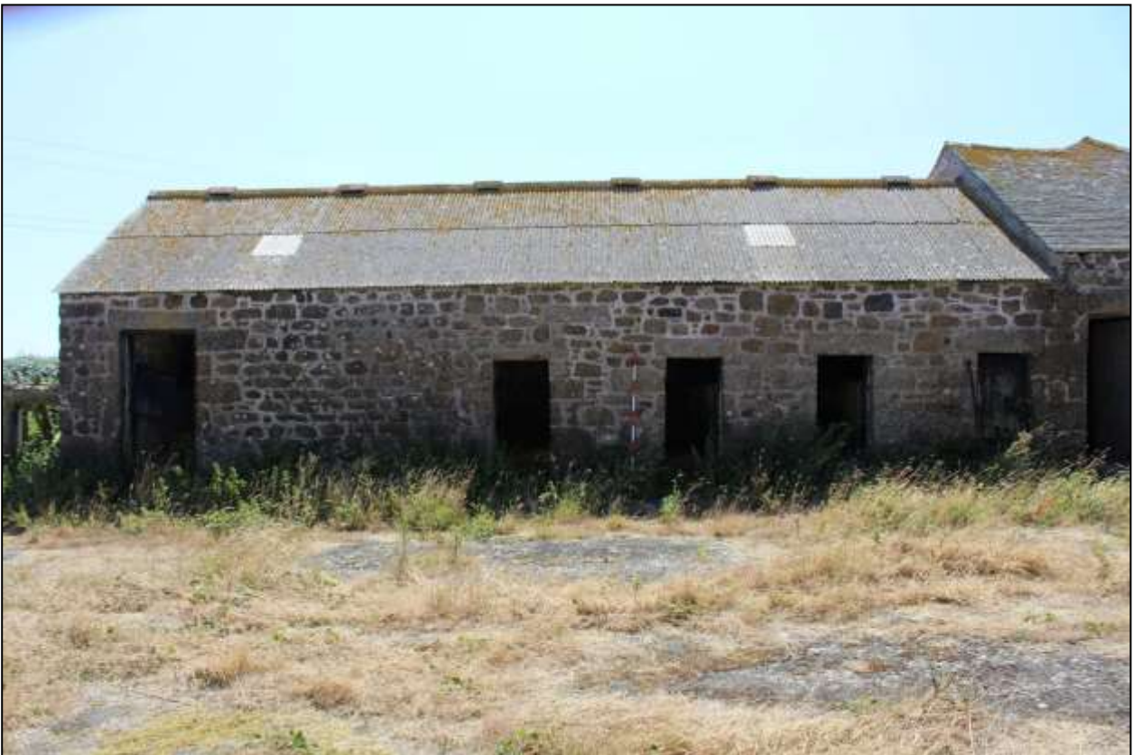
44. B2, NORTH-WEST ELEVATION; VIEWED FROM THE NORTH-WEST (SCALE 2M).
