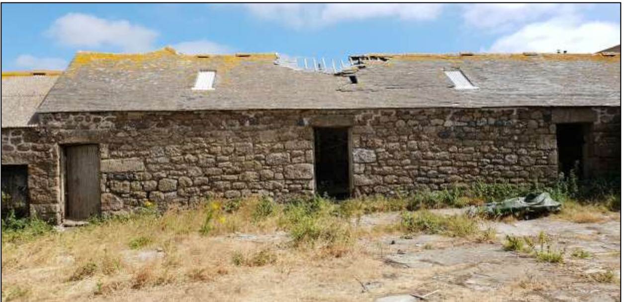
38. B4, NORTH-WEST ELEVATION; VIEWED FROM THE NORTH-WEST.
