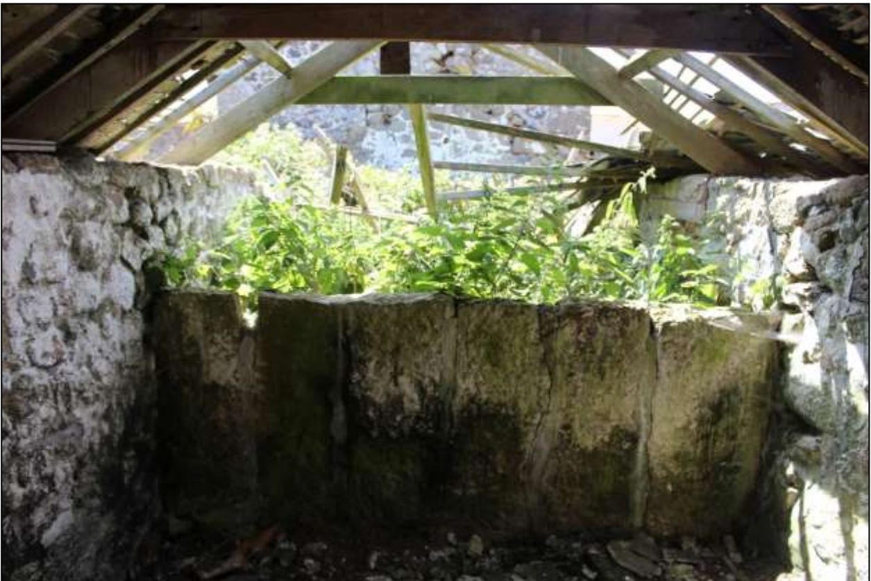
99. B1 INTERIOR, THE GRANITE SLAB PIGSTY WALLS; VIEWED FROM THE NORTH-EAST.
