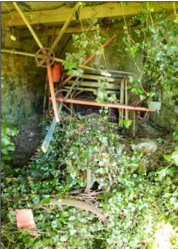
175. B8 INTERIOR, SHOWING OLD REPEAT/BINDER; VIEWED FROM THE SOUTH-WEST.
