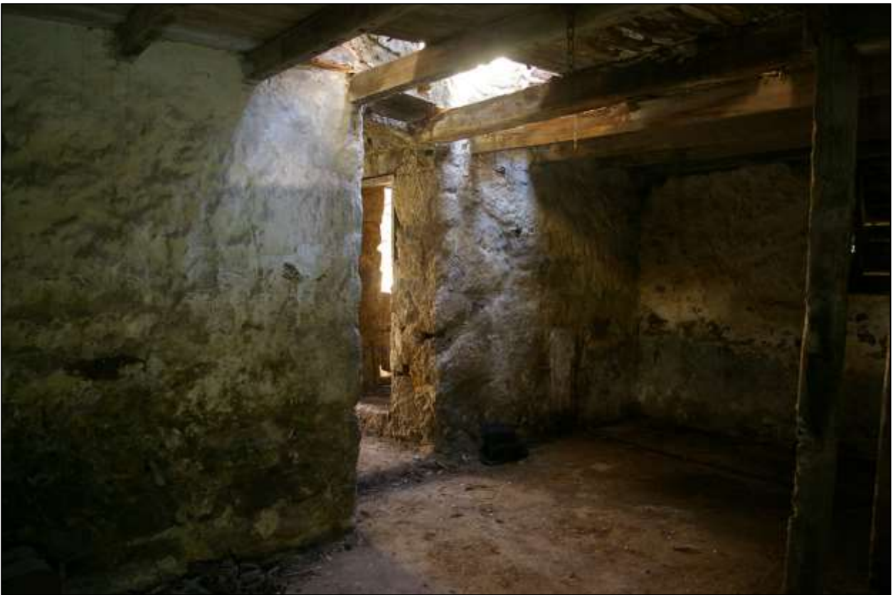
123. B3 GF INTERIOR, CLEARED OF RUBBISH; VIEWED FROM THE SOUTH.
