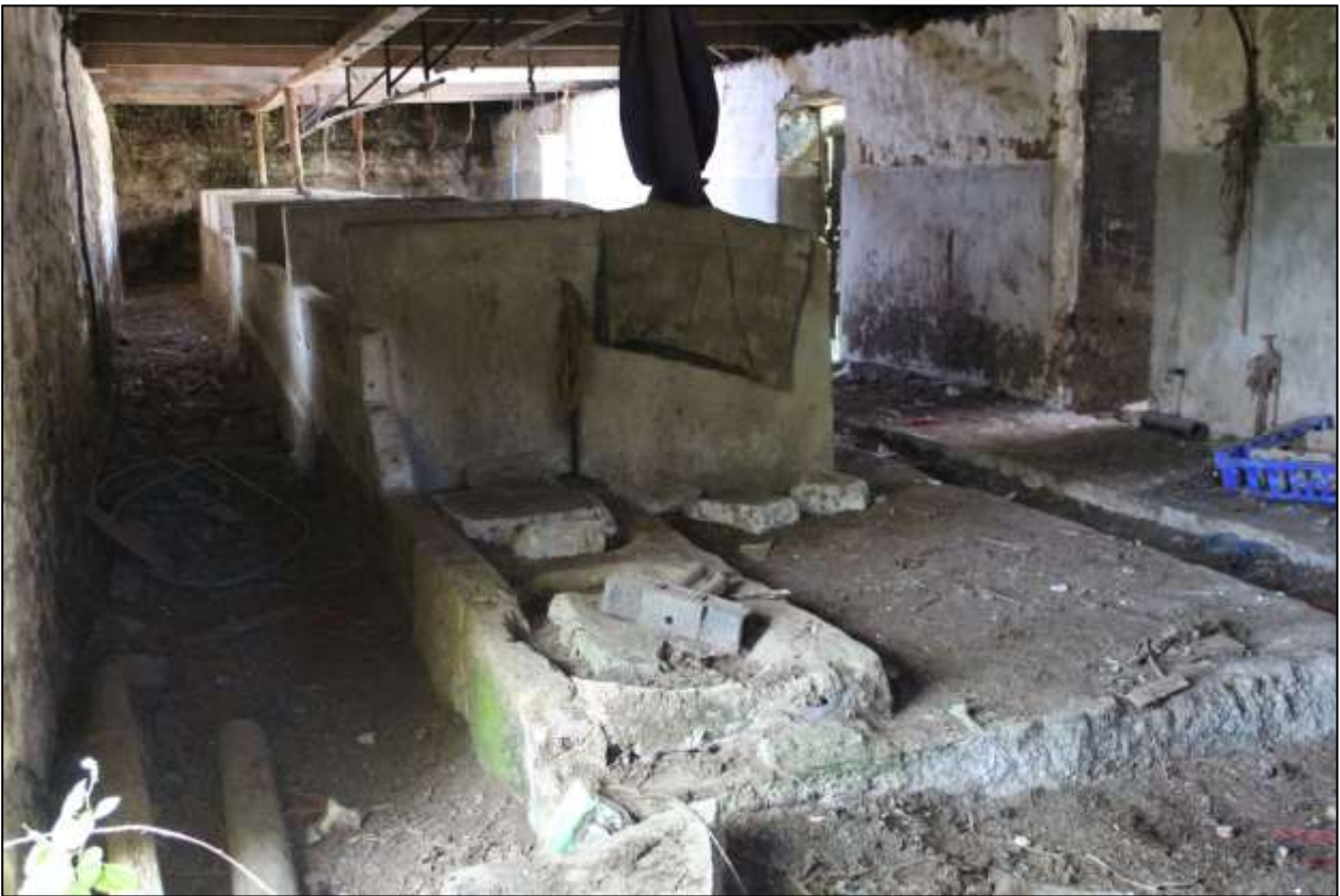
165. B7 INTERIOR; VIEWED FROM THE SSE.
