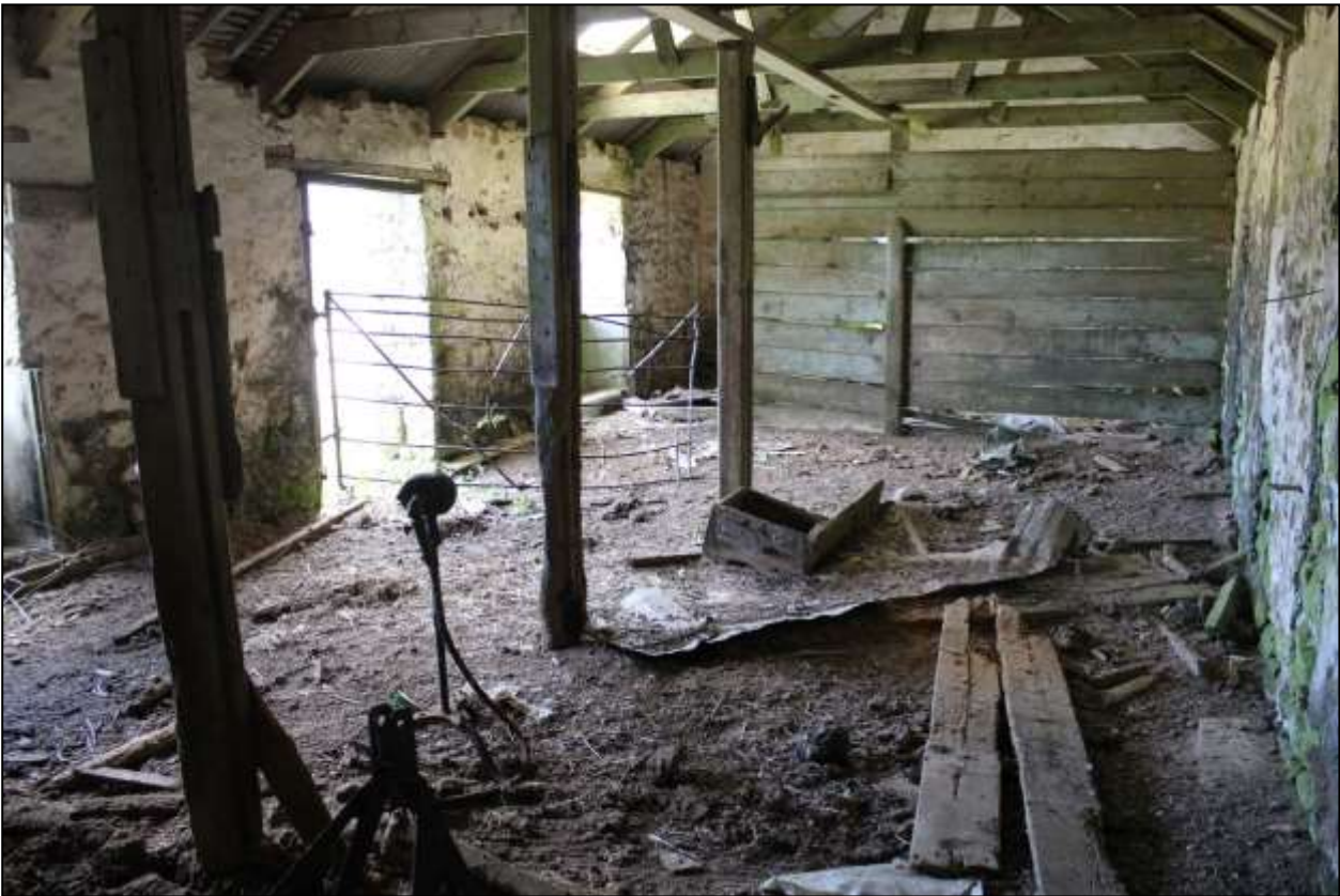
199. B10B INTERIOR; VIEWED FROM THE NNE.
