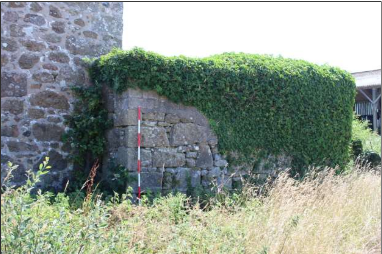
93. B8, NORTH-WEST ELEVATION; VIEWED FROM THE NNW (SCALE 2M).
