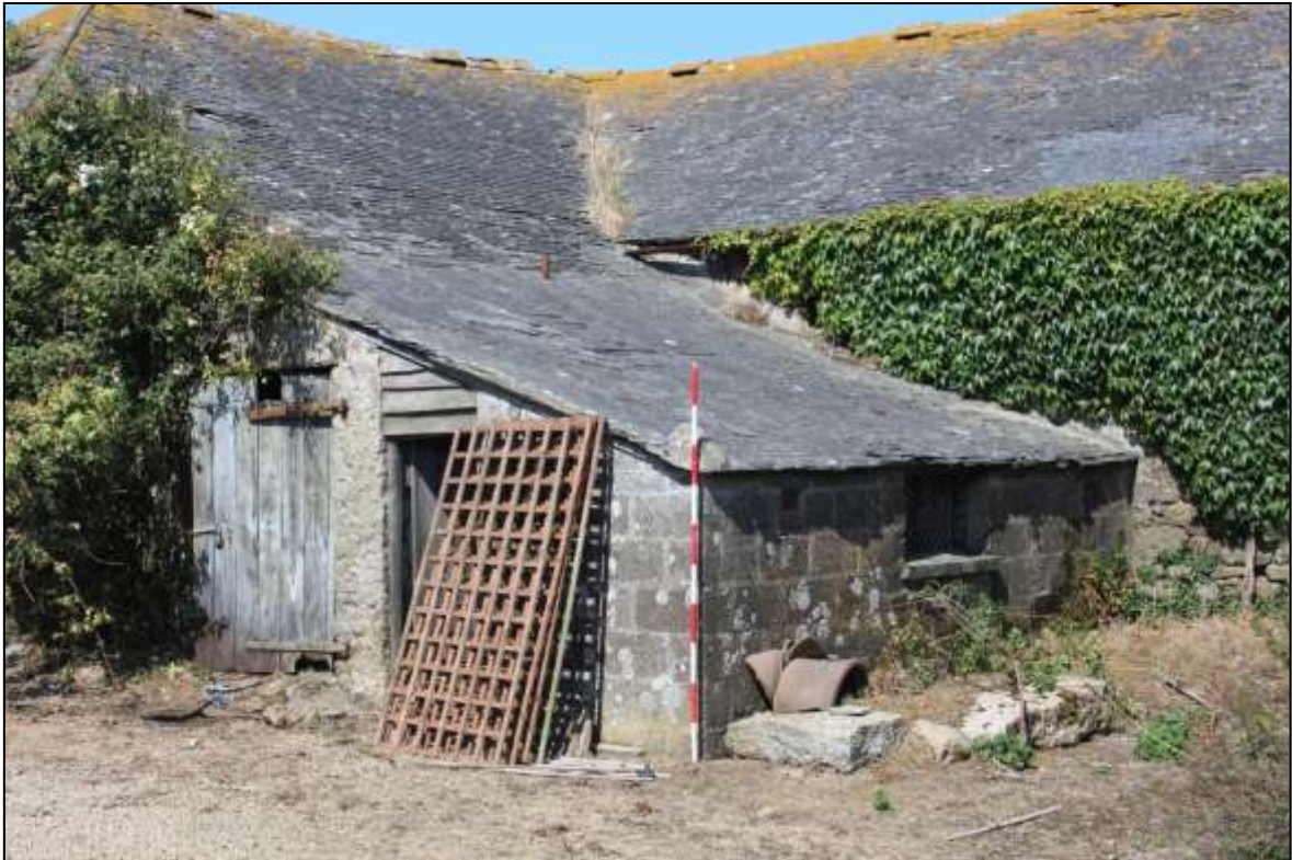
FIGURE 17: B5 AND B6; VIEWED FROM THE SOUTH (SCALE 2M).
