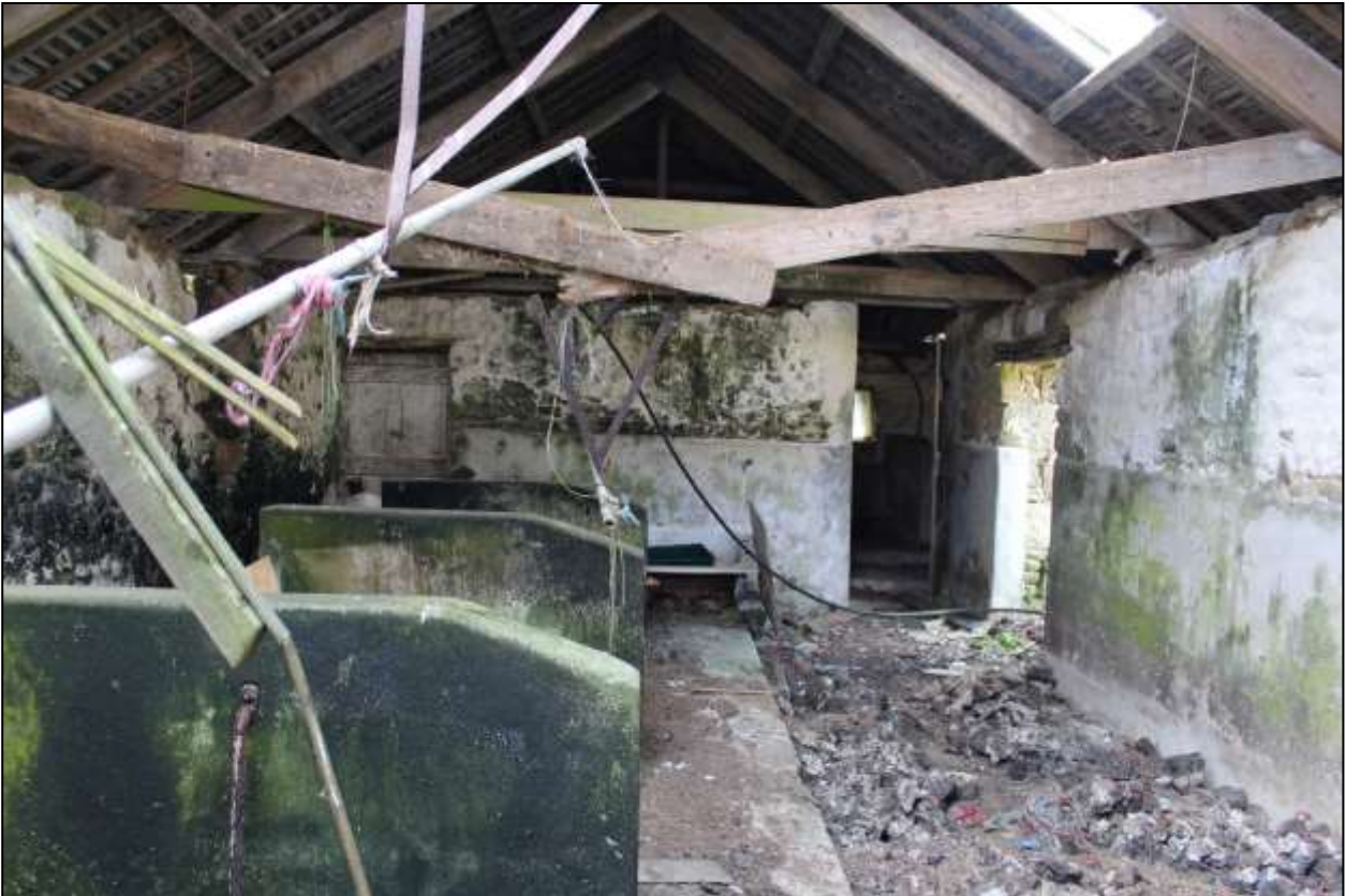
145. B4 INTERIOR, VIEWED FROM THE NORTH-EAST.
