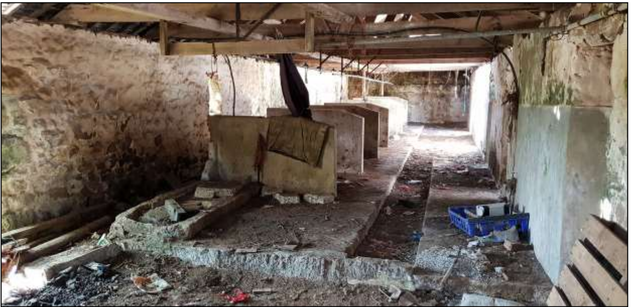
167. B7 INTERIOR; VIEWED FROM THE SOUTH-EAST.
