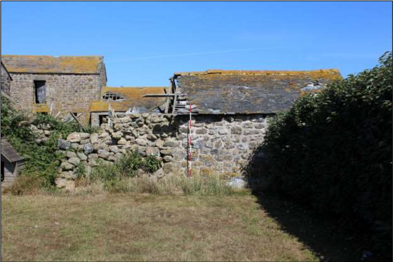
1. B1, SOUTH-EAST ELEVATION; VIEWED FROM THE SOUTH-EAST (SCALE 2M).
