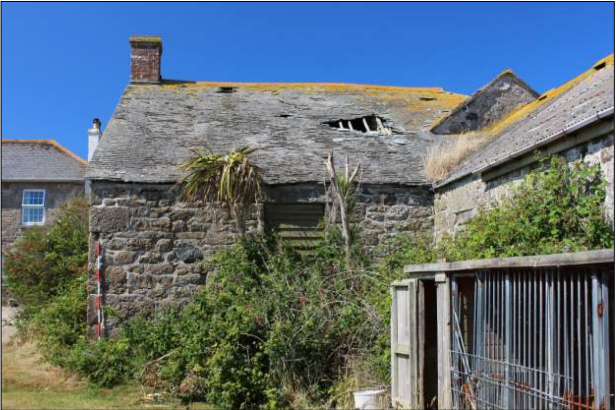
5. B3, NORTH-EAST ELEVATION; VIEWED FROM THE NORTH-EAST (SCALE 2M).
