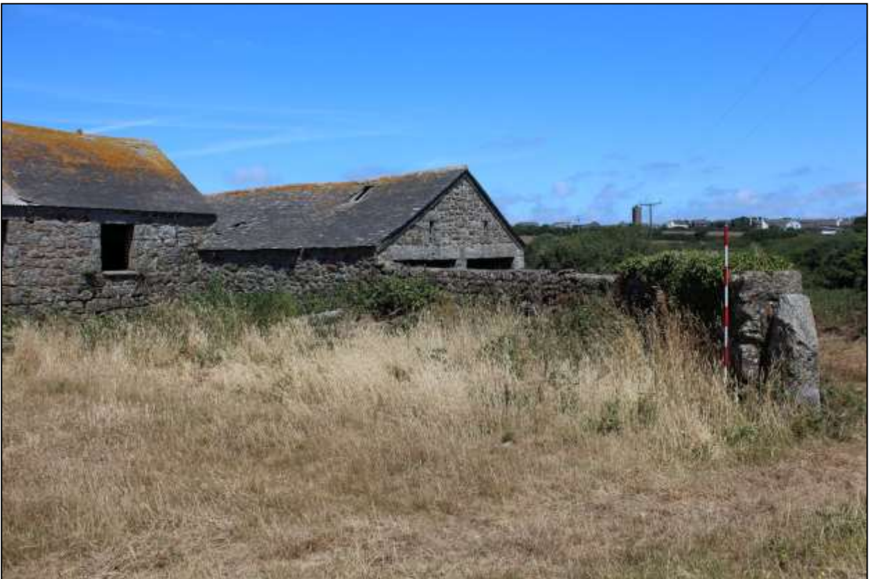
81. THE NORTH YARD WALL WITH B11 BEYOND; VIEWED FROM THE SOUTH (SCALE 2M).
