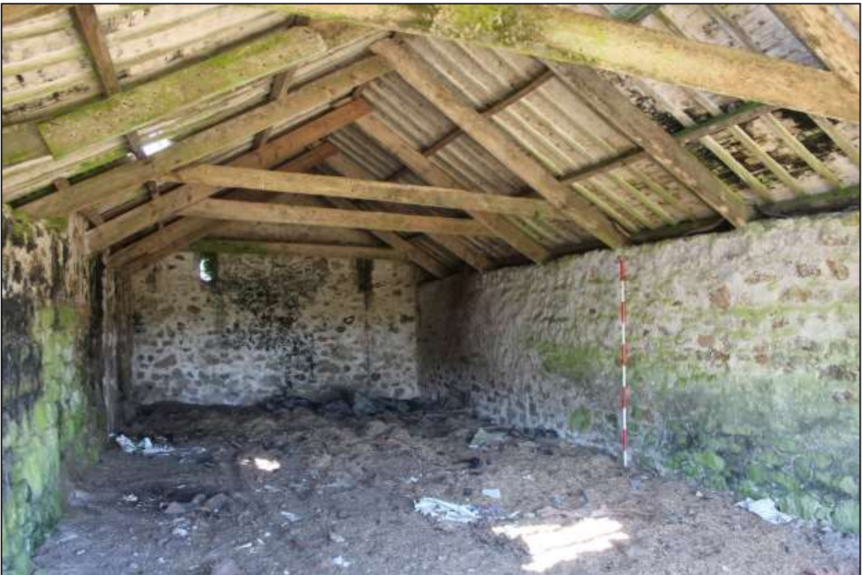
217. B11 INTERIOR; VIEWED FROM THE SSE (SCALE 2M).
