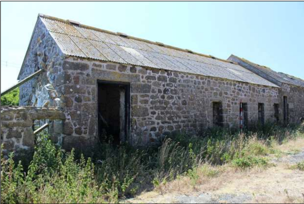
46. B2, NORTH-WEST ELEVATION; VIEWED FROM THE NORTH (SCALE 2M).
