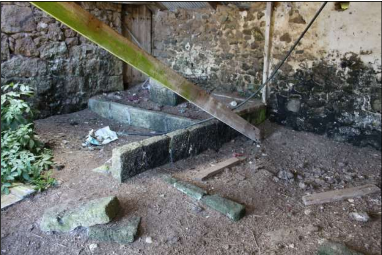
197. B10A INTERIOR; VIEWED FROM THE NORTH.
