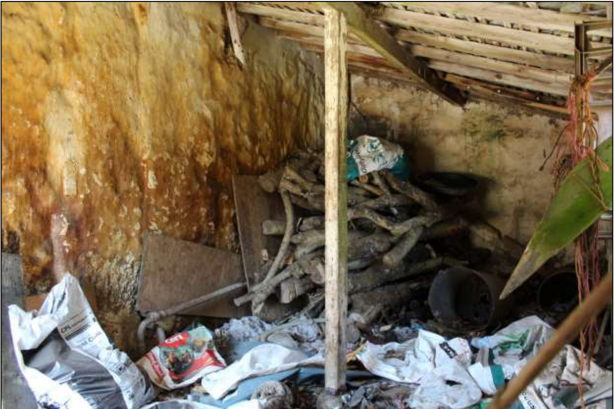
151. B5 INTERIOR, THE SOUTH-WEST WALL WITH BO5; VIEWED FROM THE NORTH-EAST.
