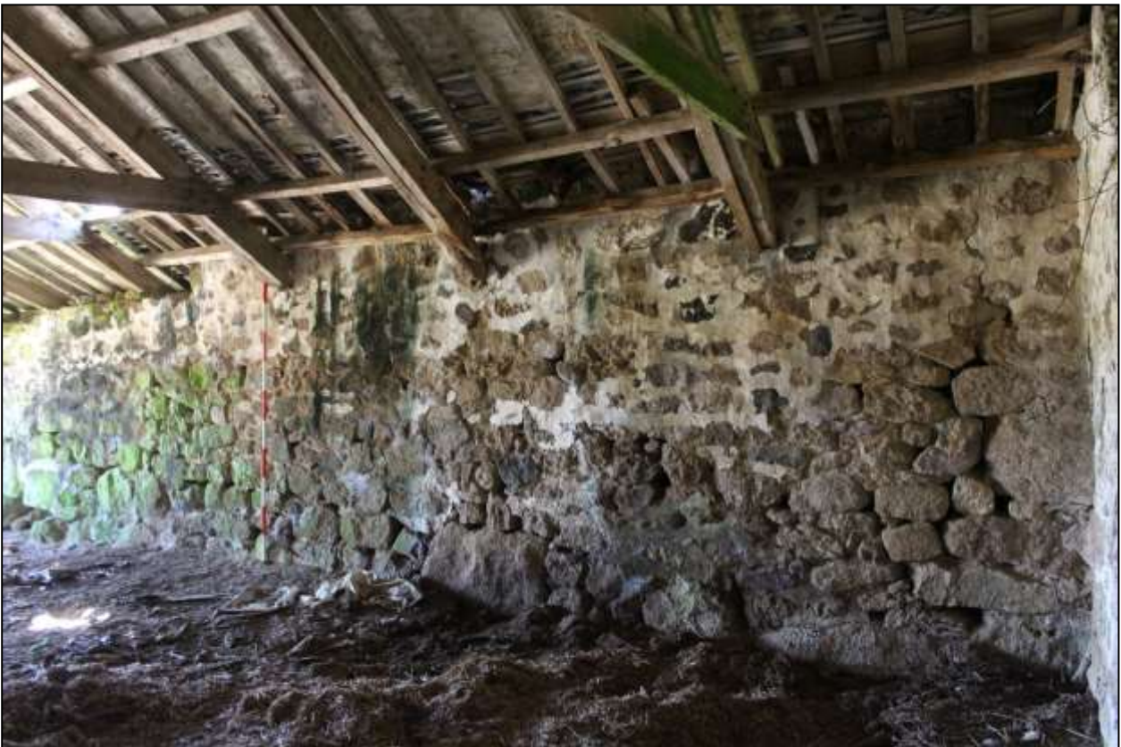
219. B11 INTERIOR, THE SOUTH-WEST WALL; VIEWED FROM THE NORTH (SCALE 2M).
