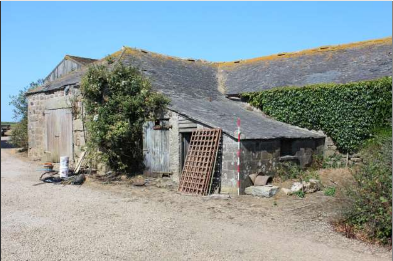
16. B5 AND B6, SOUTH-EAST ELEVATIONS; VIEWED FROM THE EAST (SCALE 2M).
