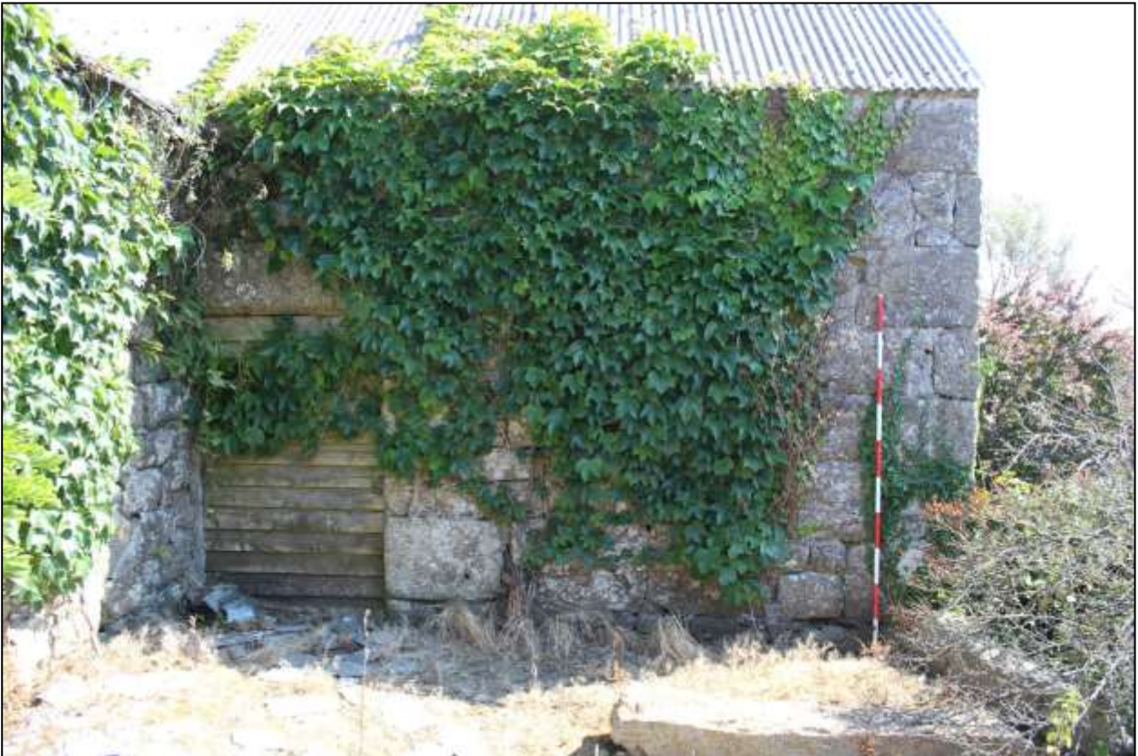
10. B3, SOUTH-EAST ELEVATION; VIEWED FROM THE SOUTH-EAST (SCALE 2M).
