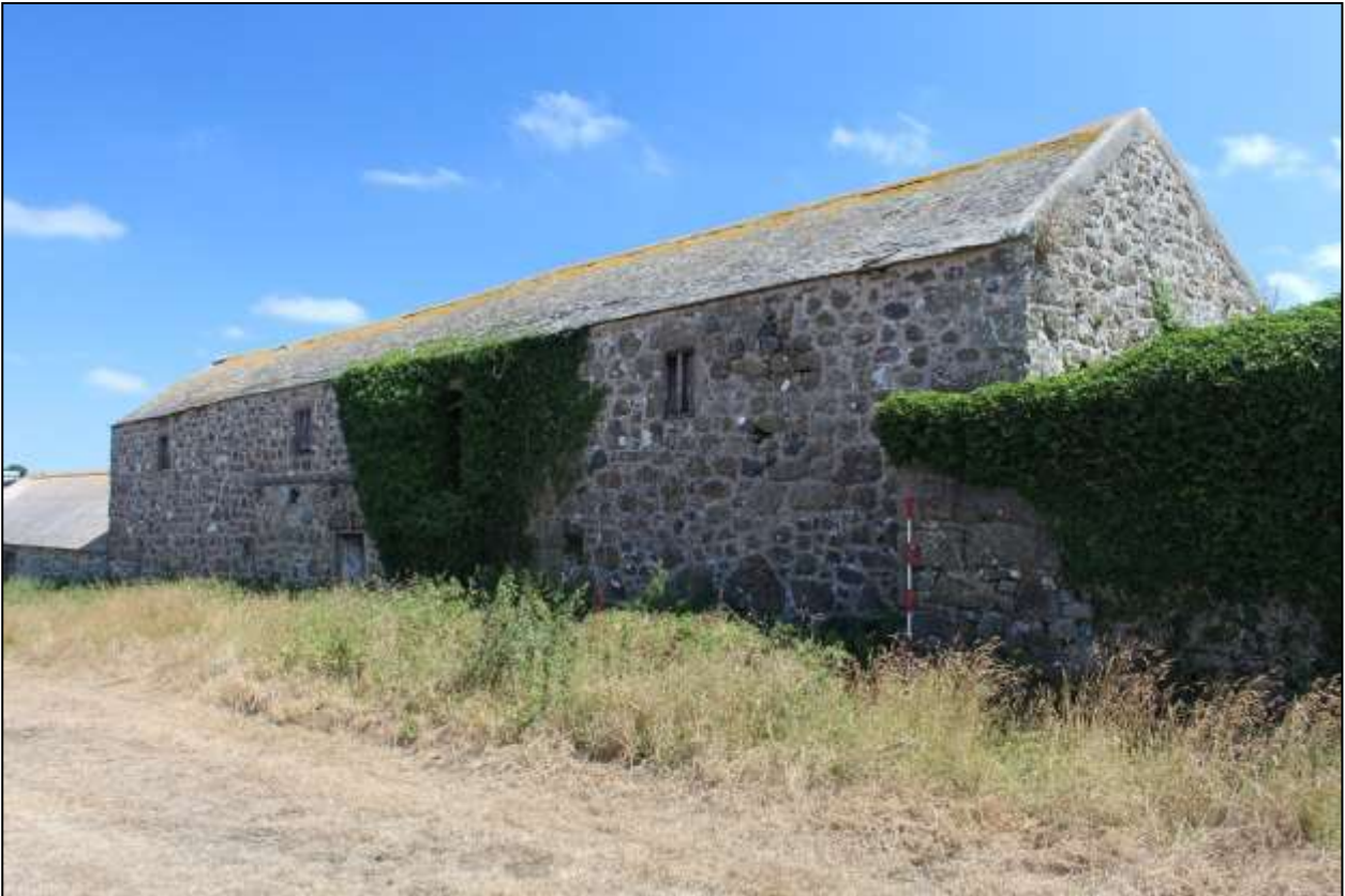
94. B9, NORTH-WEST ELEVATION; VIEWED FROM THE WSW (SCALE 2M).
