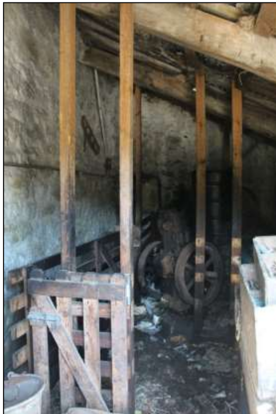
152. LEFT: B5 INTERIOR, THE SOUTH-WEST WALL COMPRISED OF GRANITE ORTHOSTATS; VIEWED FROM THE EAST.
