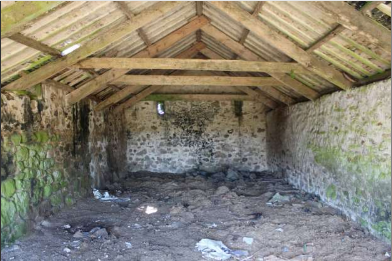
216. B11 INTERIOR; VIEWED FROM THE SOUTH-EAST.
