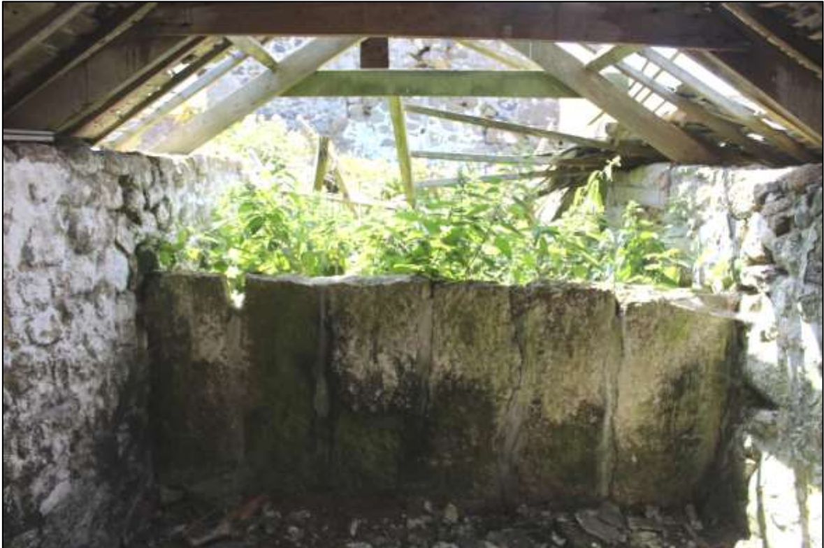
FIGURE 8: B1, GRANITE SLAB DIVIDERS; VIEWED FROM THE NORTH-EAST.
