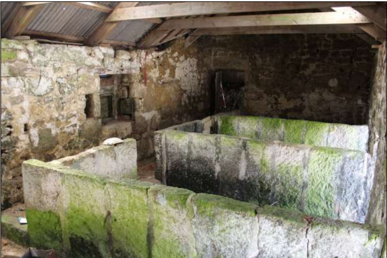
108. B1B INTERIOR, THE GRANITE SLAB PIGSTY WALLS; VIEWED FROM THE NORTH.
