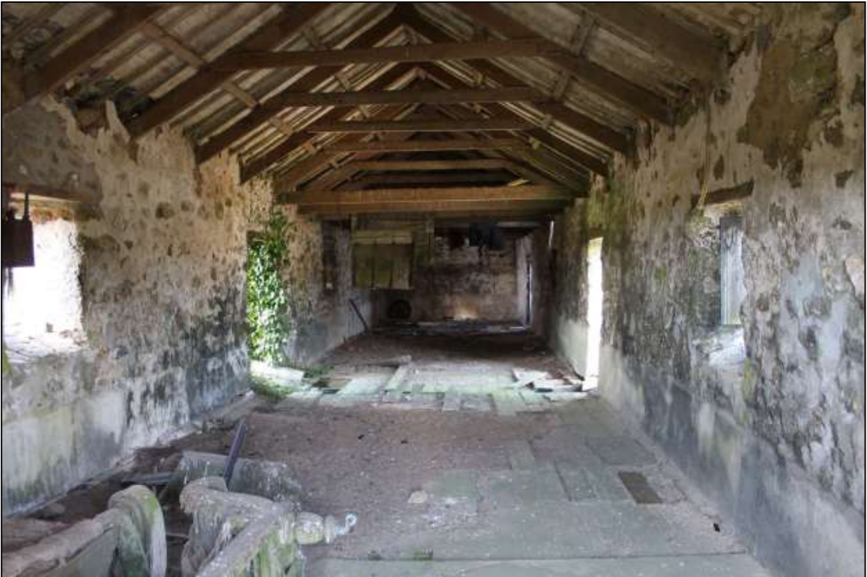
189. B9A FF INTERIOR; VIEWED FROM THE SOUTH-WEST.
