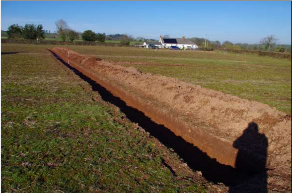
FIGURE 10: THE WEST-FACING SECTION OF TRENCH #4; VIEWED FROM THE SOUTH-WEST.
