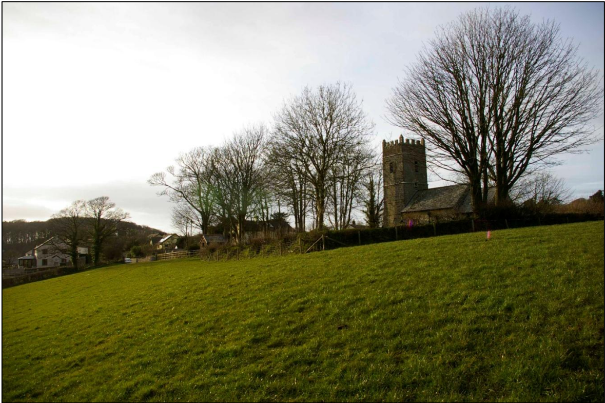
FIGURE 8: VIEW ALONG THE SOUTHERN EXTENT OF THE PLANNING AREA; VIEWED FROM THE SOUTH EAST.
