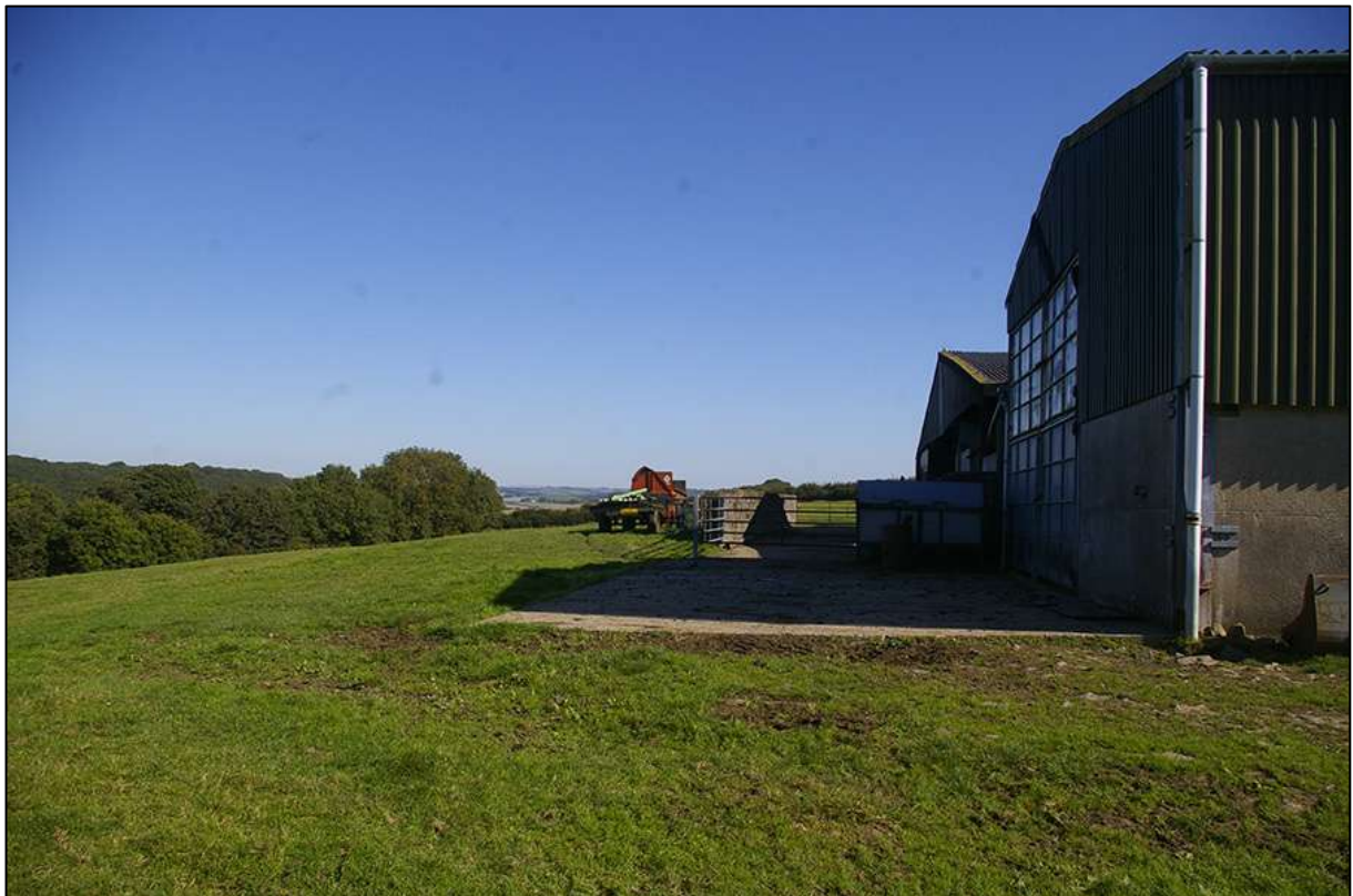
FIGURE 29: HARD STANDING ON THE NORTH-WEST SIDE OF THE NORTH AGRICULTURAL BUILDING; VIEWED FROM THE SOUTH-WEST (NO SCALE).
