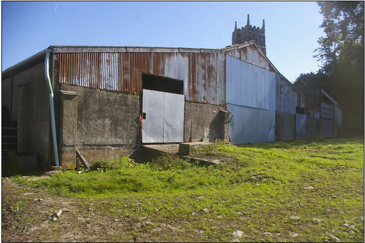
FIGURE 18: SOUTH AGRICULTURAL BUILDING; VIEWED FROM THE NORTH-WEST (NO SCALE).
