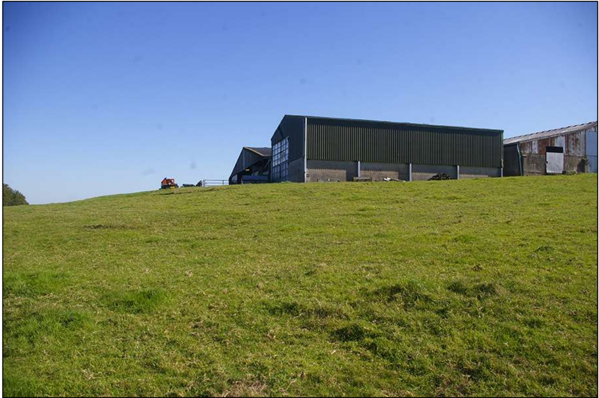
FIGURE 28: SITE SHOT SHOWING THE NORTH AGRICULTURAL BUILDING AND MADE-GROUND EARTHWORK RIDGE; VIEWED FROM THE WEST-NORTH-WEST (NO SCALE).
