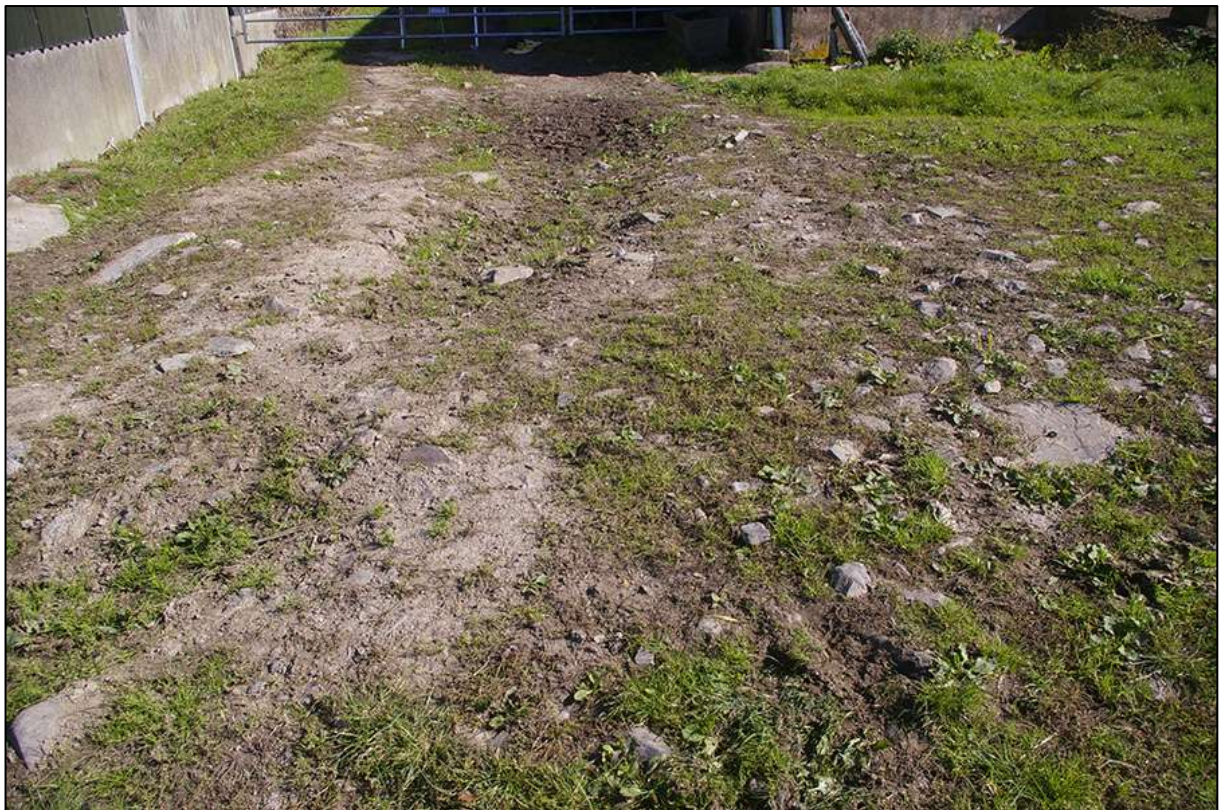
FIGURE 31: HARD-CORE STONE AND CONCRETE RUBBLE DEBRIS IN TRACK AT THE GATE/ENTRANCE BETWEEN THE TWO MODERN AGRICULTURAL BUILDINGS; VIEWED FROM THE SOUTH-WEST ((NO SCALE).
