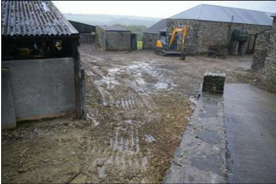
FIGURE 2: YARD AREA POST REDUCTION; VIEWED FROM THE SOUTH-WEST (NO SCALE).
