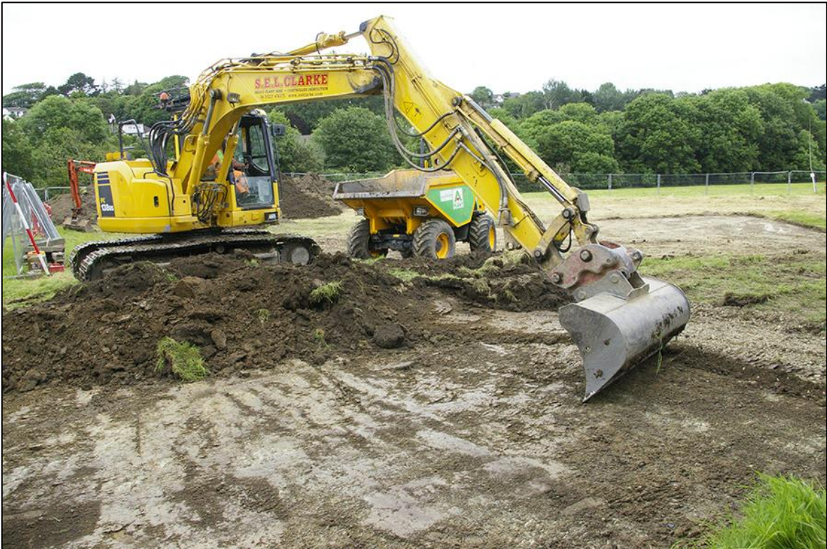
6. WORKING SHOT, SITE STRIP; VIEWED FROM THE SOUTH-WEST (NO SCALE).
