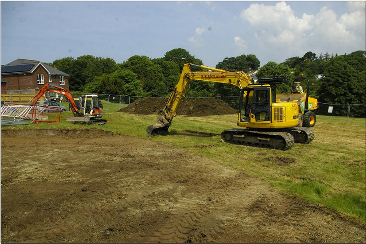
5. WORKING SHOT, SITE STRIP; VIEWED FROM THE SOUTH-EAST (NO SCALE).
