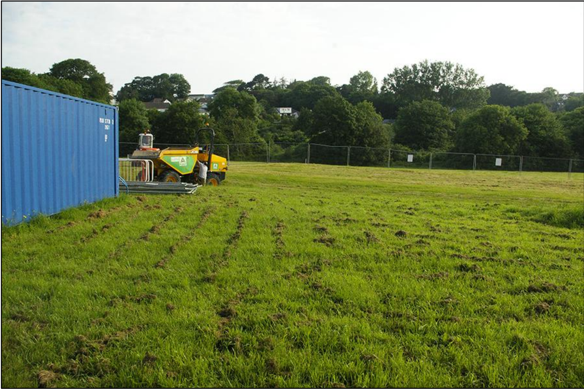
1. SITE VIEW PRE-EXCAVATION; VIEWED FROM THE SOUTH (NO SCALE).
