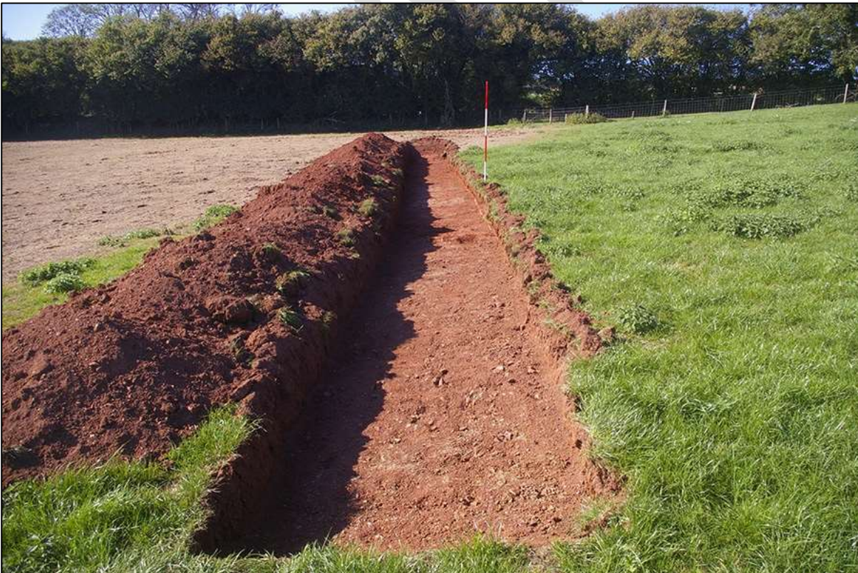
63. TRENCH 10, POST-EXCAVATION; VIEWED FROM THE SOUTH-EAST (92M SCALE).
