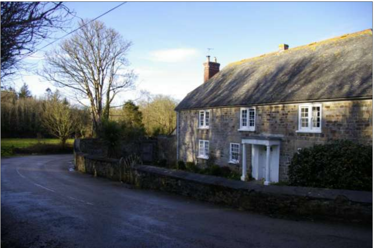
12. VIEW OF TRELOWETH; FARMHOUSE; VIEWED FROM THE SOUTH.
