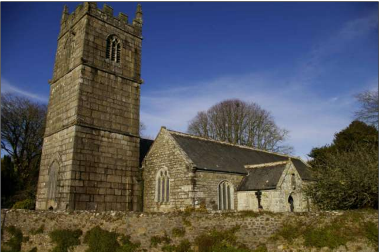
14. VIEW OF THE CHURCH; VIEWED FROM THE SOUTH-WEST.
