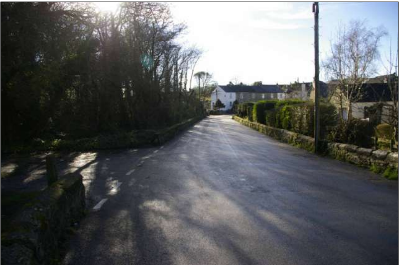
16. VIEW ALONG THE WESTERN SECTION OF ST ERTH BRIDGE; VIEWED FROM THE SOUTH-EAST.
