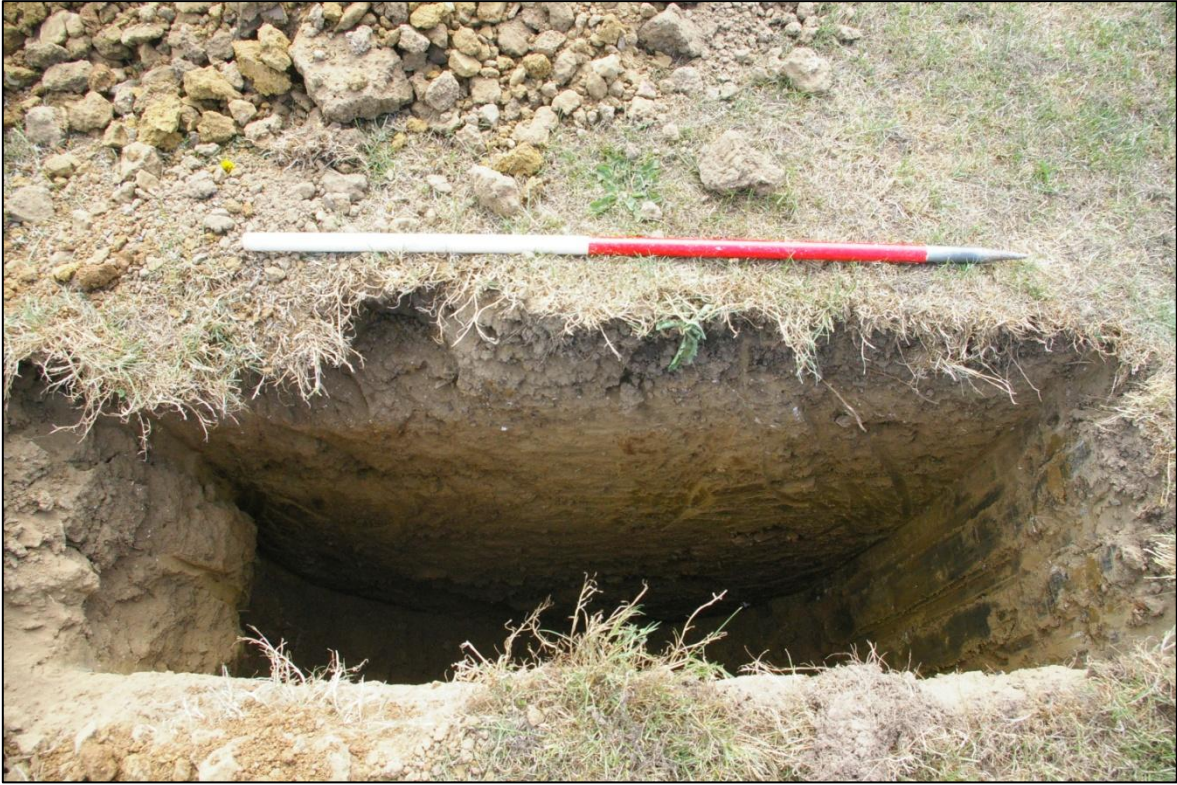
5. TRIAL-PIT 04, NORTH-WEST FACING SECTION; VIEWED FROM THE NORTH-WEST (1M SCALE).
