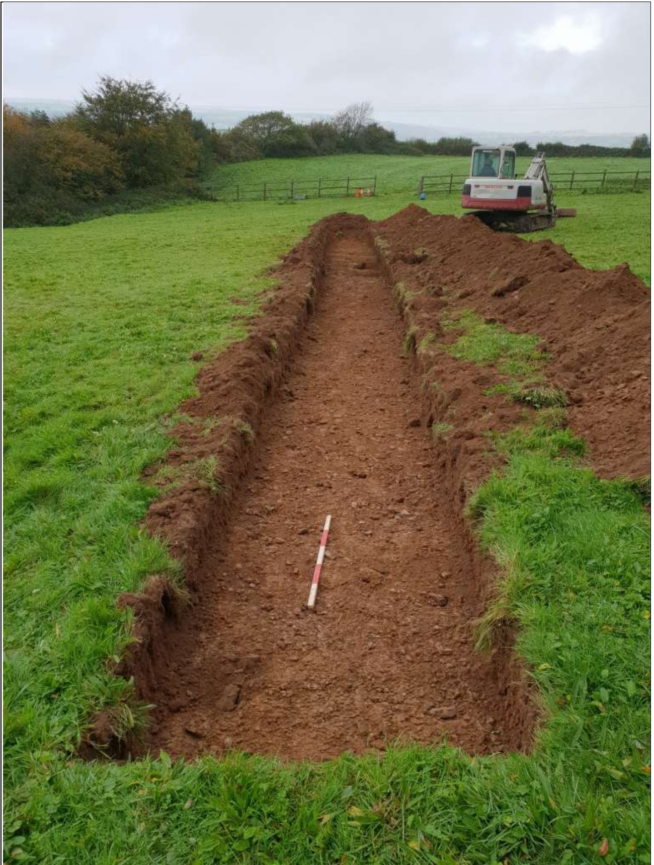
19. TRENCH 3, POST-EX, VIEWED FROM THE SOUTH-EAST (1M SCALE).
