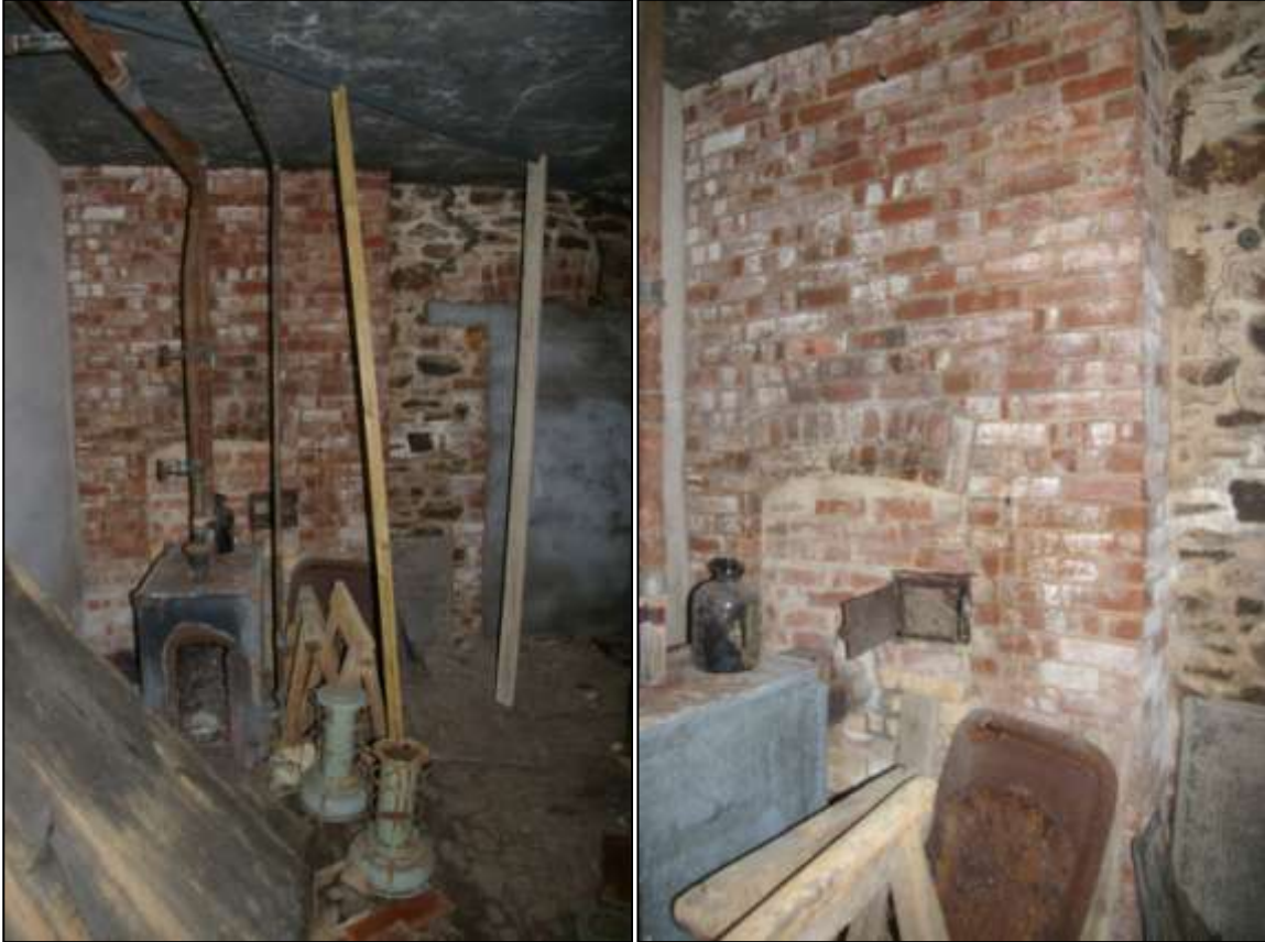
29. LEFT: THE BOILER WITH ITS BRICK FLUE; FROM THE NORTH.
