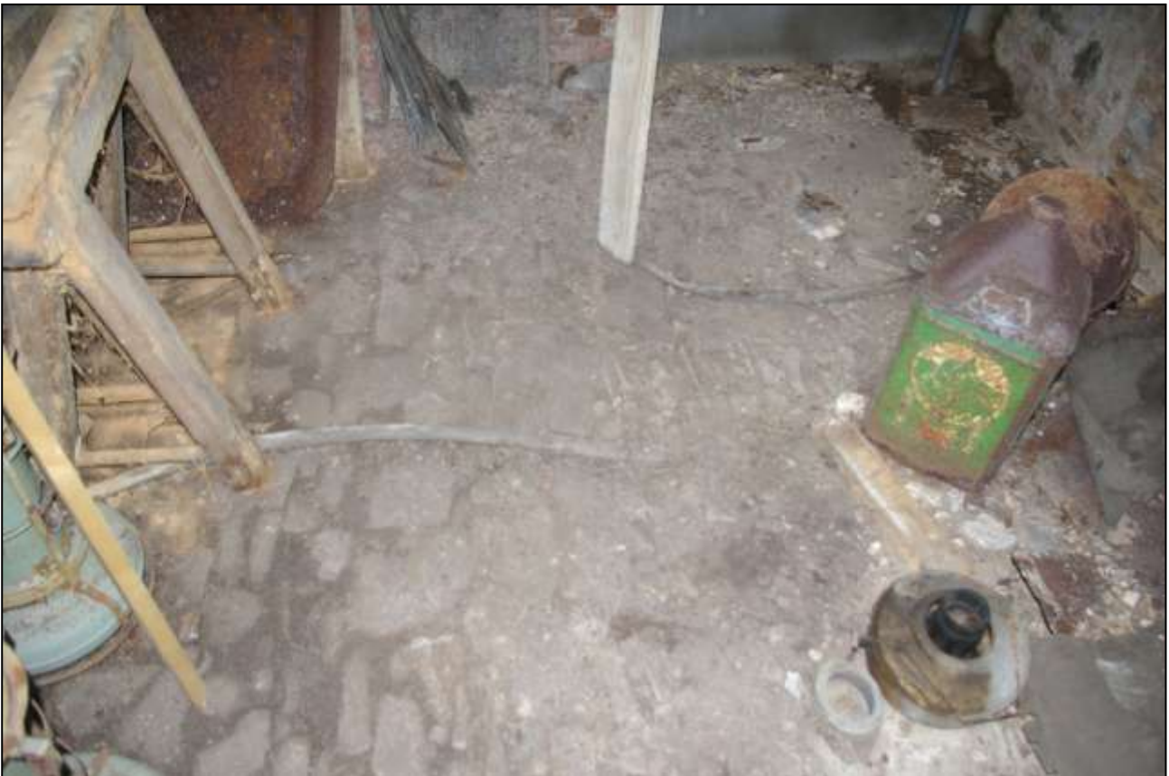
31. THE SLATESTONE COBBLED FLOOR OF THE BOILER ROOM; FROM THE NORTH.
