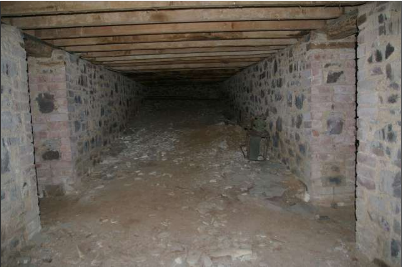
37. THE CENTRAL UNDERCROFT COMPARTMENT; FROM THE SOUTH.
