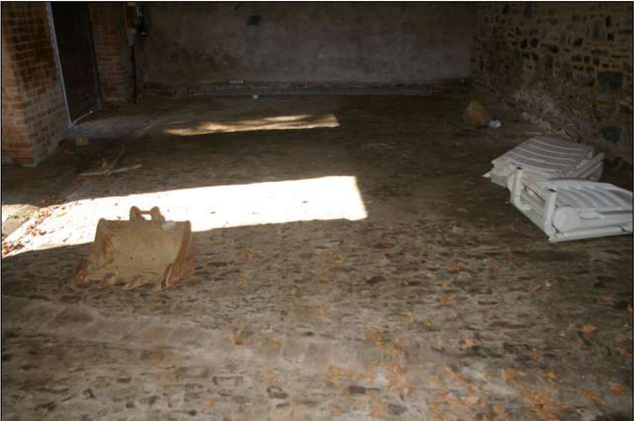
47. THE SLATESTONE COBBLED FLOOR OF THE CARRIAGE HOUSE, FROM THE EAST.
