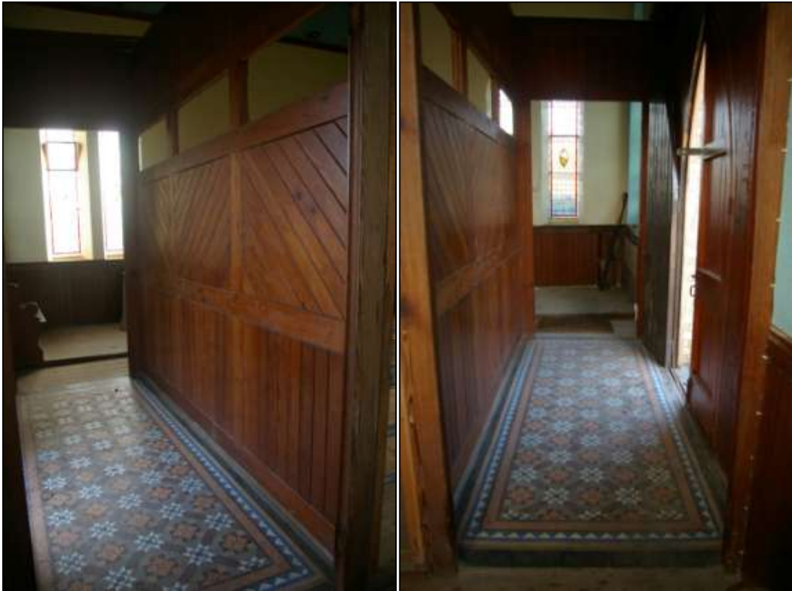
58. LEFT: THE FINE DIAGONAL BOARDING OF THE PORCH SCREEN; FROM THE WEST-NORTH-WEST.
