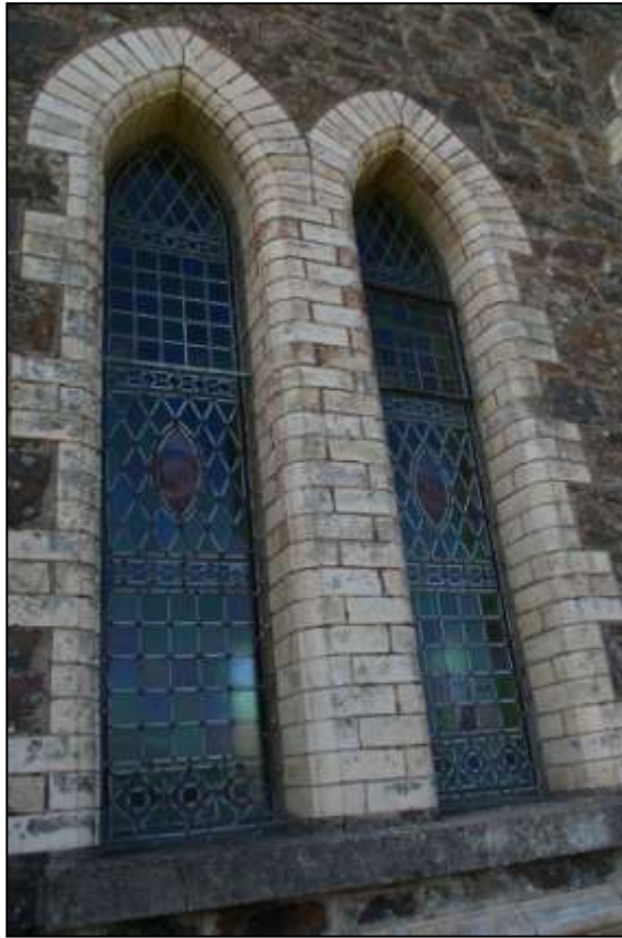
17. WINDOW 6 ON THE EAST WALL, AN EXAMPLE OF THE SIDE ELEVATION WINDOW DESIGN; FROM THE EAST.
