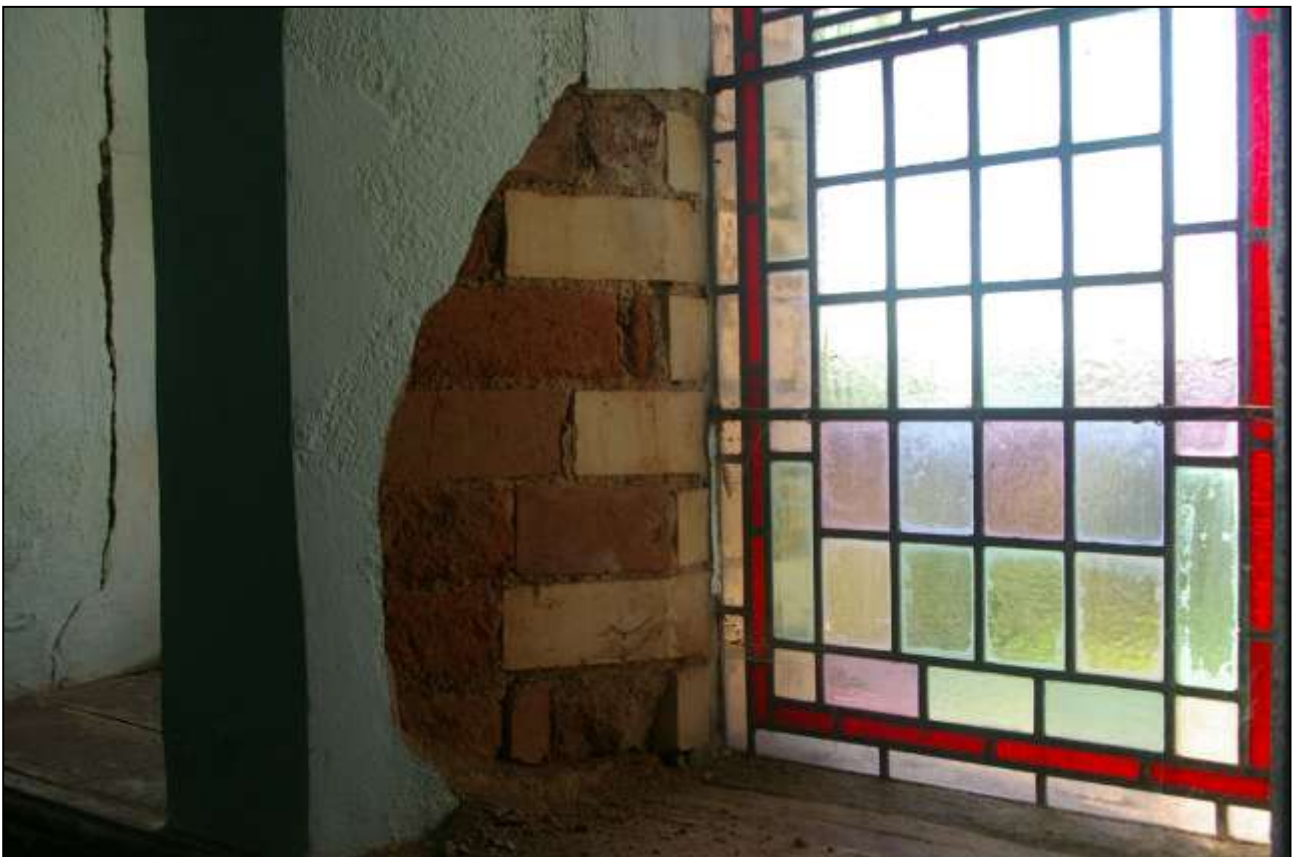
111. DETAIL OF REMOVED PLASTER AT WEST WINDOW, W18; SHOWING EXTERNAL CREAM CERAMIC BRICK, INTERNAL RED ENGINEERING BRICK; FROM THE EAST-NORTH-EAST.
