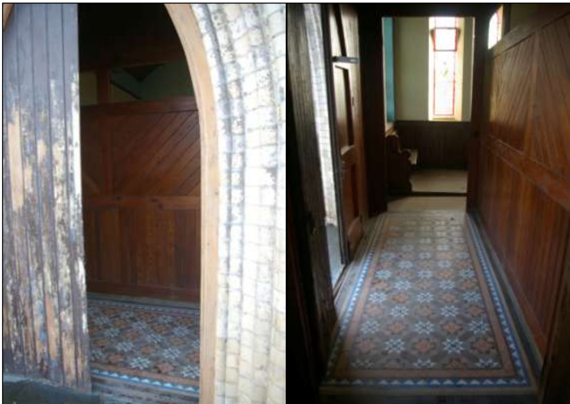
56. LEFT: THROUGH THE FRONT DOOR TO THE WEATHER PORCH, SHOWING TILED FLOOR; FROM THE NORTH-NORTH-WEST.
