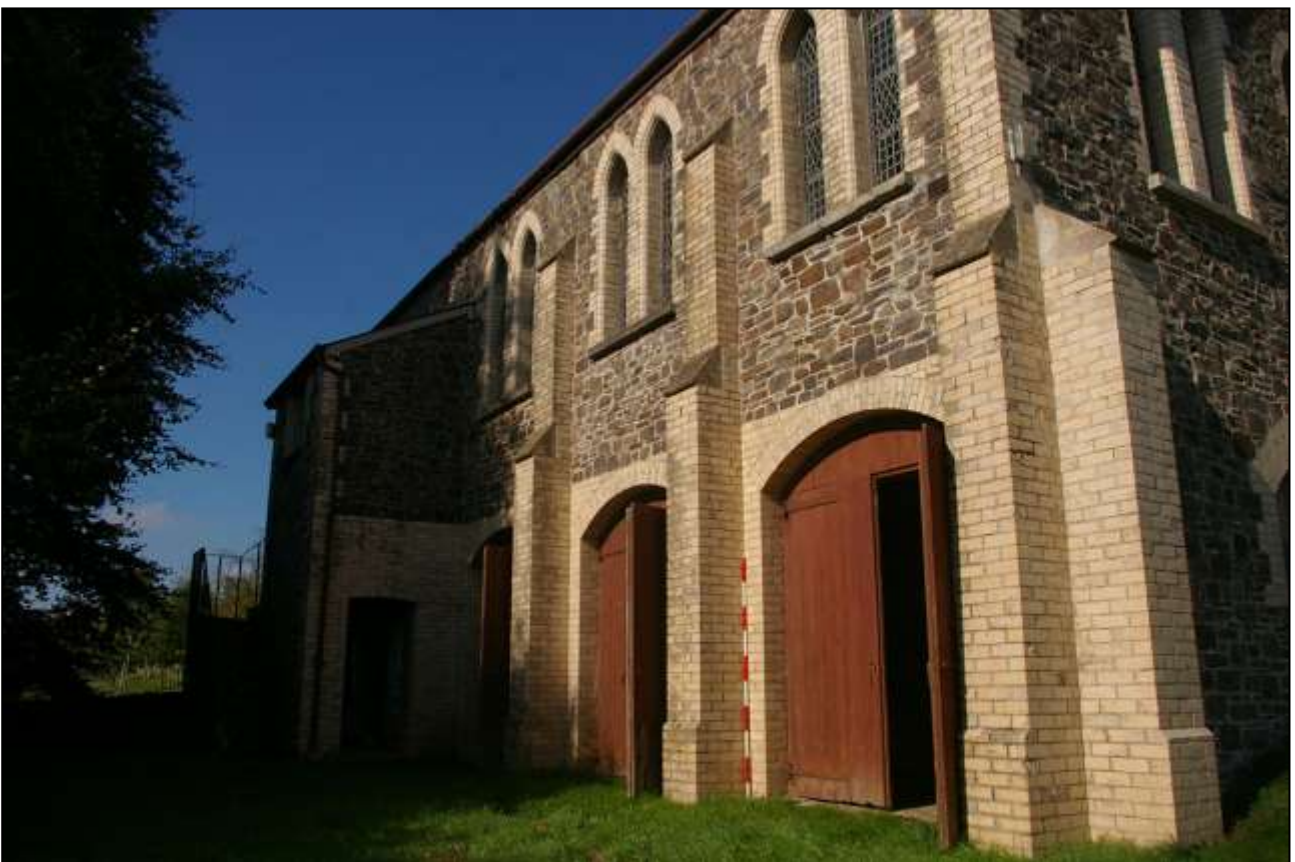
22. THE SOUTH ELEVATION OF THE CROSSWING, SHOWING SUBTLE DIFFERENCES IN BUILD, SUCH AS BRICK BUTTRESSES AND LOWER GROUND FLOOR; FROM THE SOUTH-EAST.
