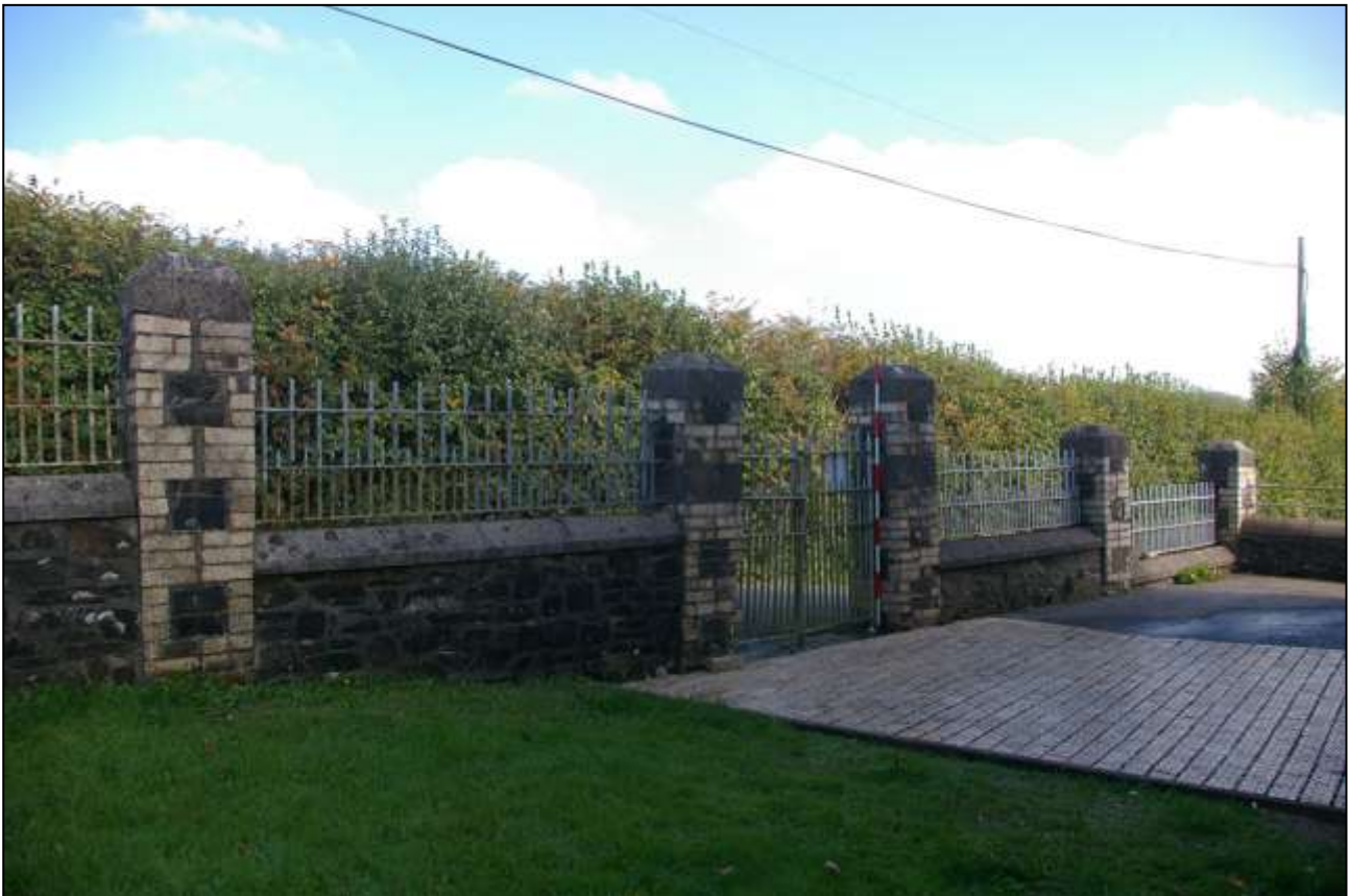
6. THE CERAMIC BRICK AND STONE RUBBLE DECORATIVE PIERS AND RAILINGS TO THE FRONT OF THE CHAPEL; FROM THE SOUTH-WEST.
