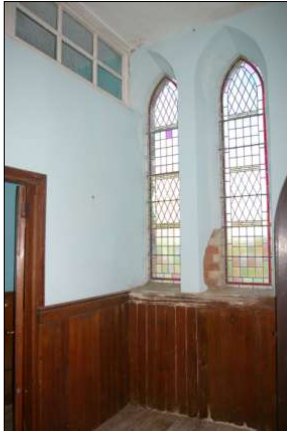
110. THE CURRENT WEST CLOAKROOM AND GENTS TOILETS, WITH INSERTED PARTITION; FROM THE EAST-NORTH-EAST.
