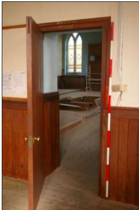
96. D3, FROM THE COMMUNITY HALL, LOOKING BACK INTO THE CHAPEL, WITH 2M SCALE; FROM THE SOUTH-EAST.
