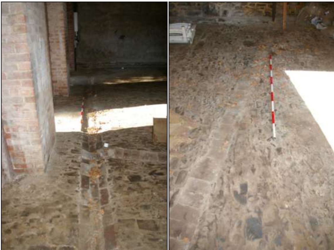
48. LEFT: THE BRICK DRAIN TO THE SOUTH SIDE OF THE COBBLED FLOOR IN THE CARRIAGE HOUSE, 2M SCALE; FROM THE EAST.
