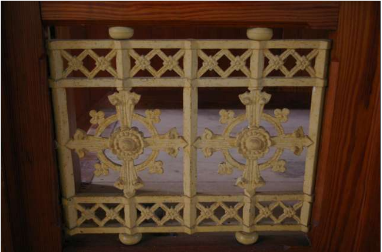
70. ONE OF THE IRONWORK FRETWORK PANELS INCLUDED IN THE PULPIT; FROM THE NORTH.
