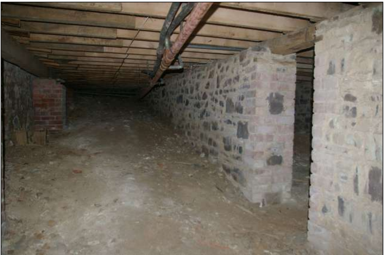
36. THE WESTERN COMPARTMENT WITHIN THE UNDERCROFT; FROM THE SOUTH.
