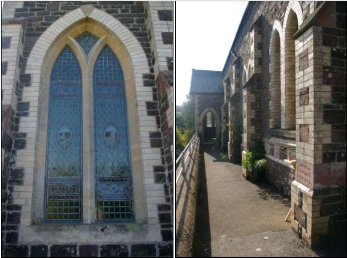
9. LEFT: WINDOW 2, AN EXAMPLE OF THE LARGER STONE WINDOWS IN THE PRESENTATION FRONT; FROM THE NORTH. 10. RIGHT: THE EAST ELEVATION OF THE CHAPEL, LOOKING TOWARDS THE SUNDAY SCHOOL ENTRANCE, WITH 2M SCALE; FROM THE NORTH-NORTH-EAST.
