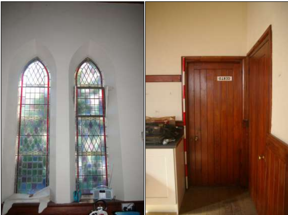
106. LEFT: WINDOW 16; FROM THE WEST. 107. RIGHT: ONE OF THE ORIGINAL BOARDED AND FRAMED DOORS, LEADING TO THE THE GENTS TOILETS; FROM THE EAST.
