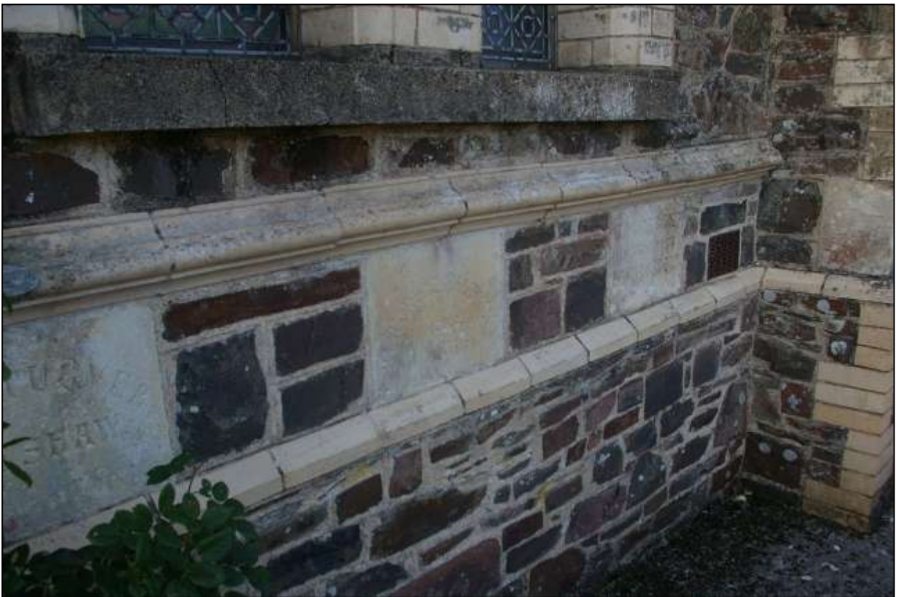
18. THE STRING COURSE AND DECORATIVE PLAQUES WITH THE NAMES OF THE CONTRIBUTORS; FROM THE SOUTH-EAST.
