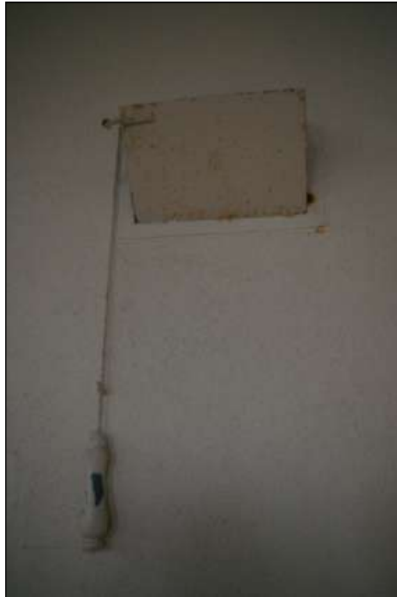
92. THE ELABORATE AIR VENTS IN THE EAST WALL; FROM THE SOUTH-WEST.
