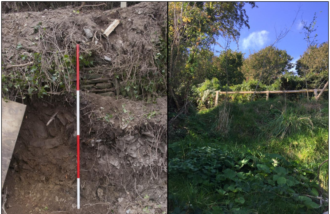
FIGURE 3: LEFT -SOUTH-EAST FACING ELEVATION OF WALL {104}, SHOWING ALTERNATING SECTIONS OF HORIZONTAL AND PITCHED SLATESTONE; VIEWED FROM THE SOUTH-EAST (2M SCALE). RIGHT – SITE RE-INSTATED IN OCTOBER 2018, FROM THE SOUTH (CLIENT).
