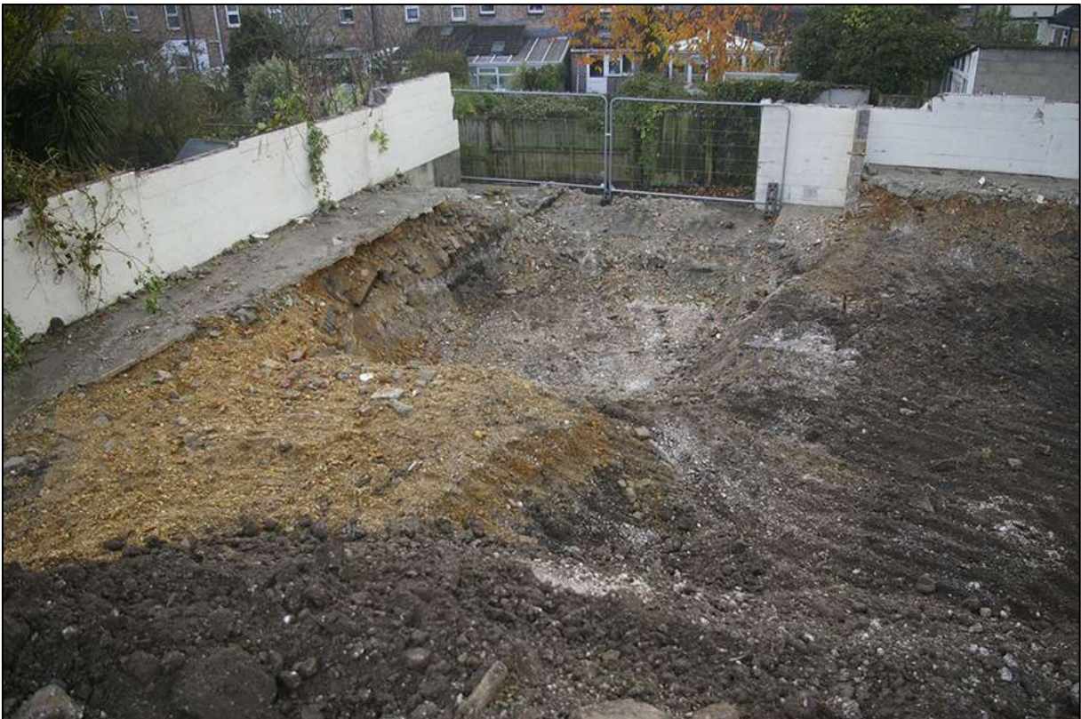
FIGURE 14: INSPECTION PIT; VIEWED FROM THE NORTH-NORTH-WEST (NO SCALE).
