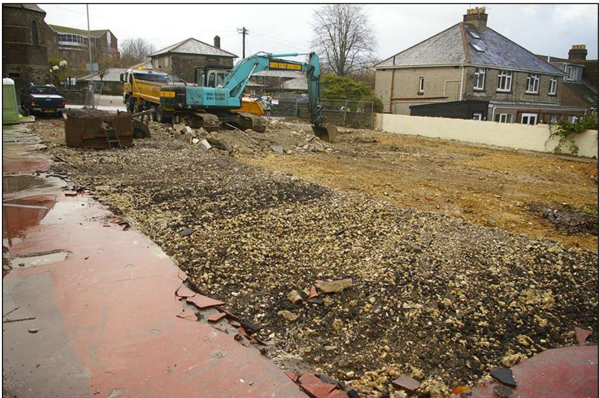
FIGURE 8: SITE SHOT POST-DEMOLITION OF STRUCTURE; VIEWED FROM THE SOUTH-WEST (NO SCALE).
