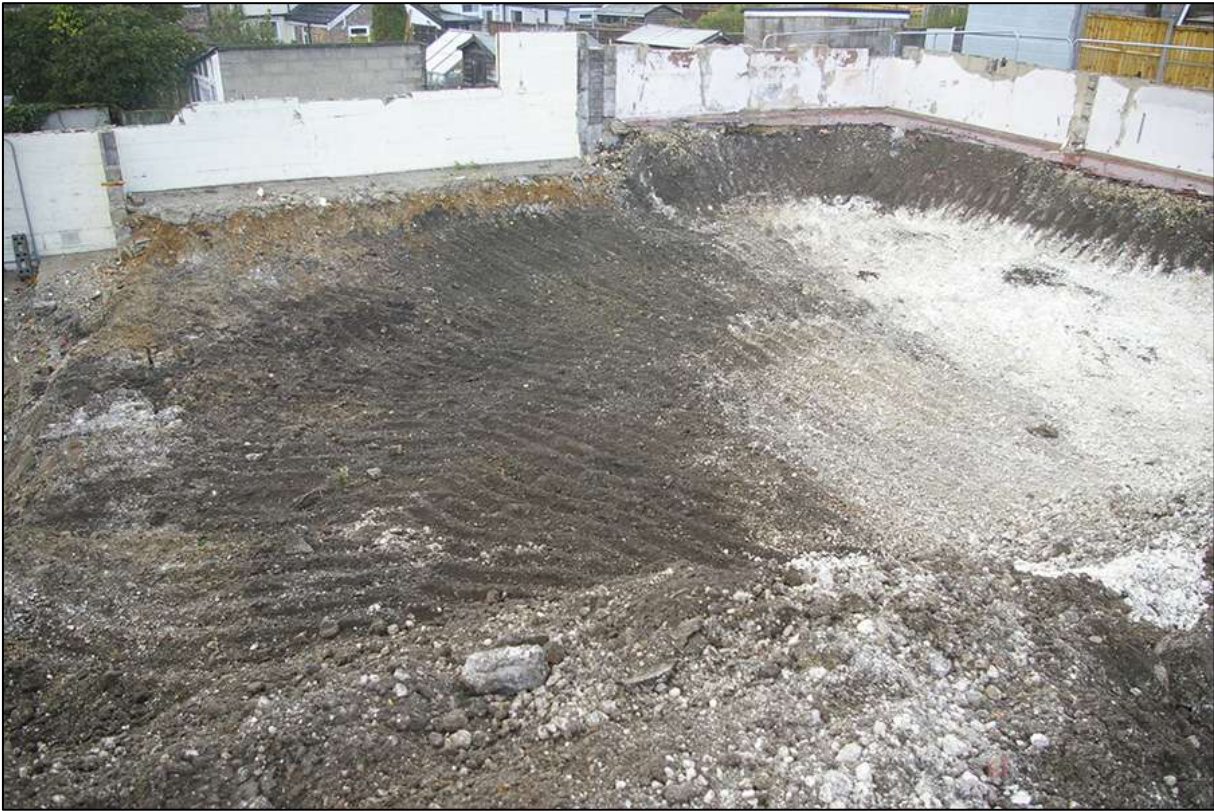
FIGURE 15: SITE SHOT MID-REDUCTION OF SOUTHERN HALF OF SITE; VIEWED FROM THE NORTH-EAST (NO SCALE).
