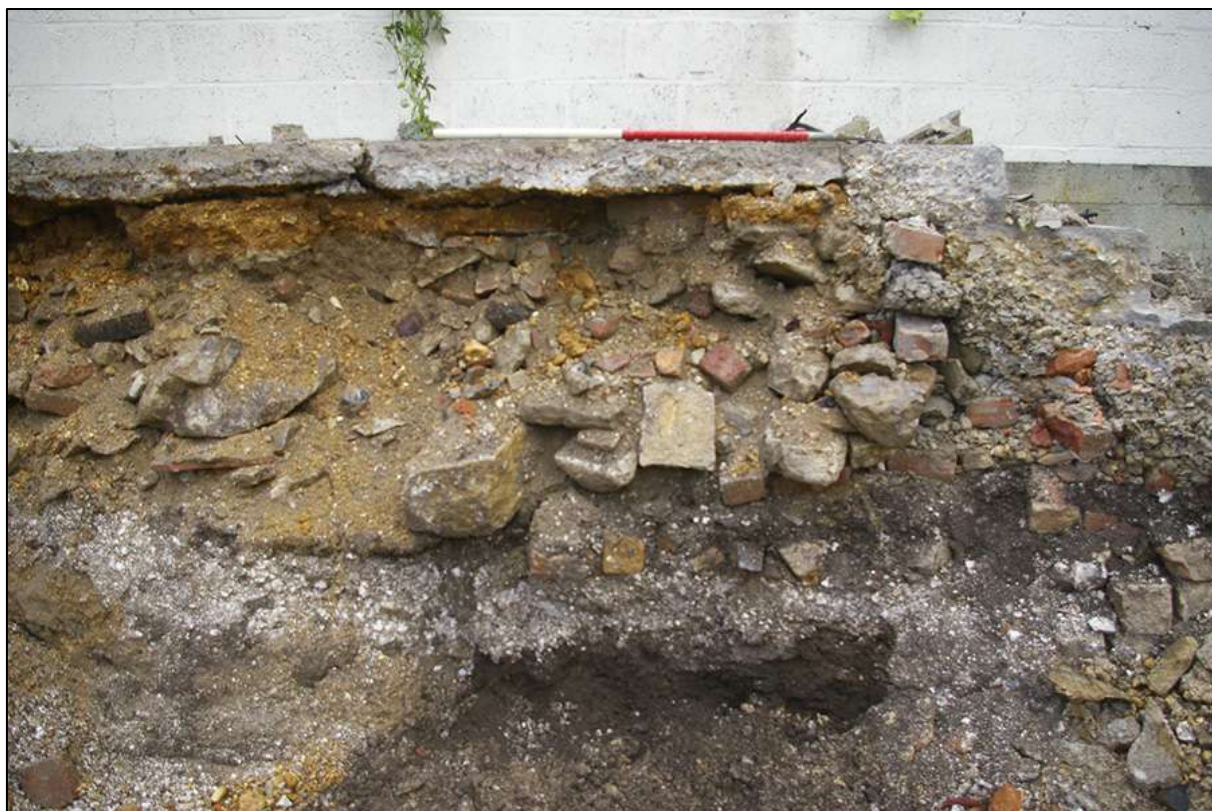
FIGURE 12: SAMPLE SECTION IN INSPECTION PIT; VIEWED FROM THE WEST (1M SCALE).
