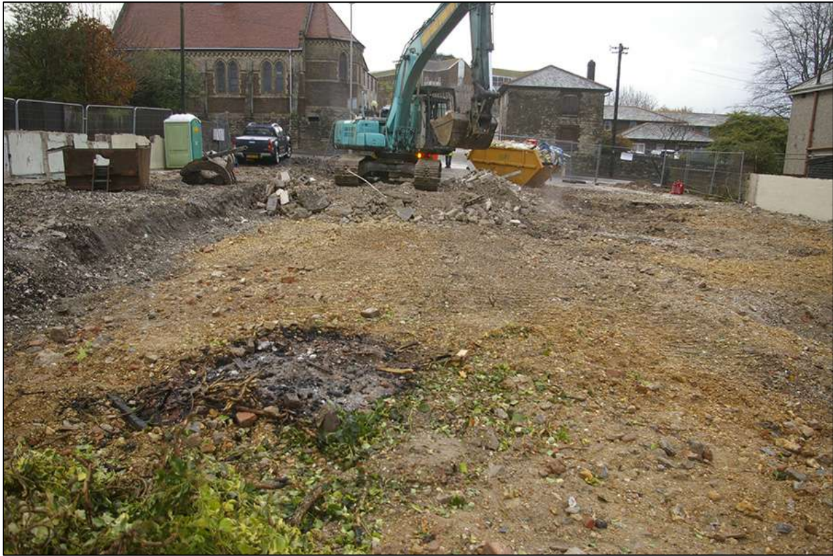
FIGURE 9: SITE SHOT POST-DEMOLITION OF STRUCTURE; VIEWED FROM THE SOUTH (NO SCALE).
