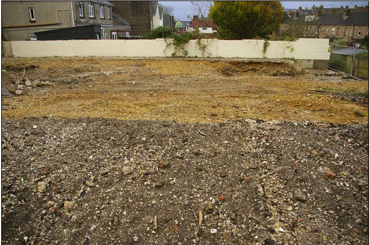
FIGURE 7: SITE SHOT POST-DEMOLITION OF STRUCTURE; VIEWED FROM THE WEST (NO SCALE).
