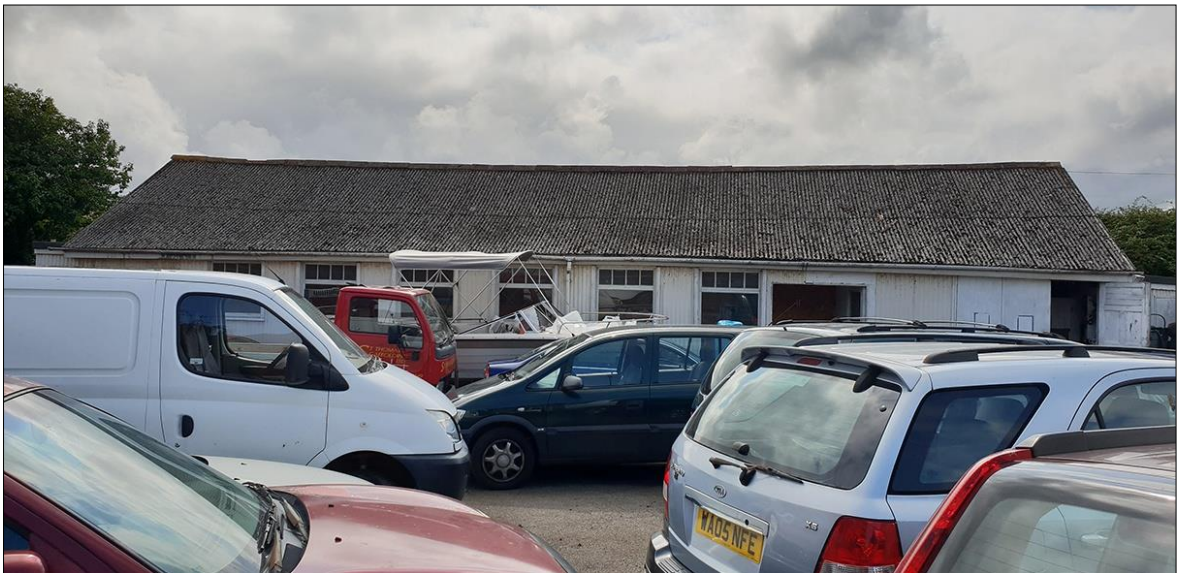
VIEW OF THE NORTH-EASTERN ELEVATION OF B1.1; VIEWED FROM THE NORTH-EAST.
