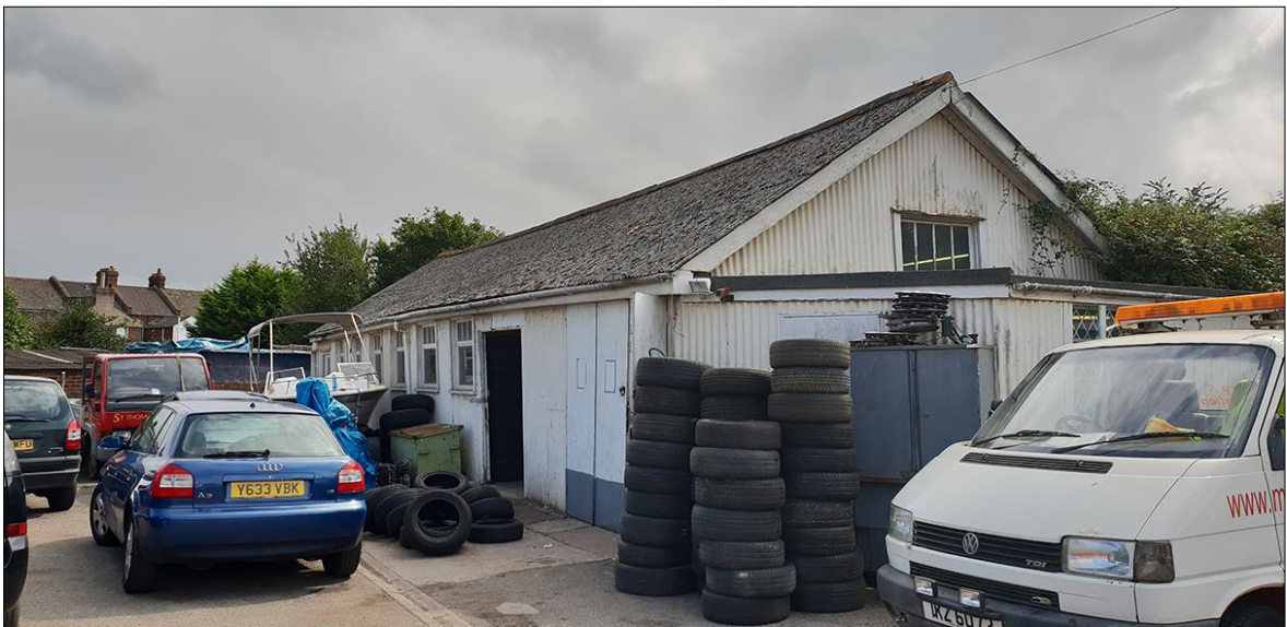
VIEW ALONG THE NORTH-EASTERN ELEVATION OF B1.1 (LEFT) AND B1.3 (RIGHT); VIEWED FROM THE NORTH-WEST.
