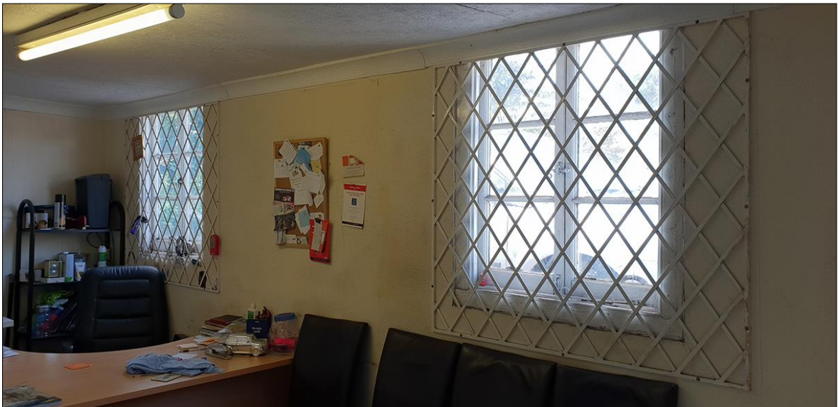
DETAIL OF THE INTERIOR OF B1.3 SHOWING THE WINDOWS IN THE NORTH-WEST ELEVATION; VIEWED FROM THE EAST.
