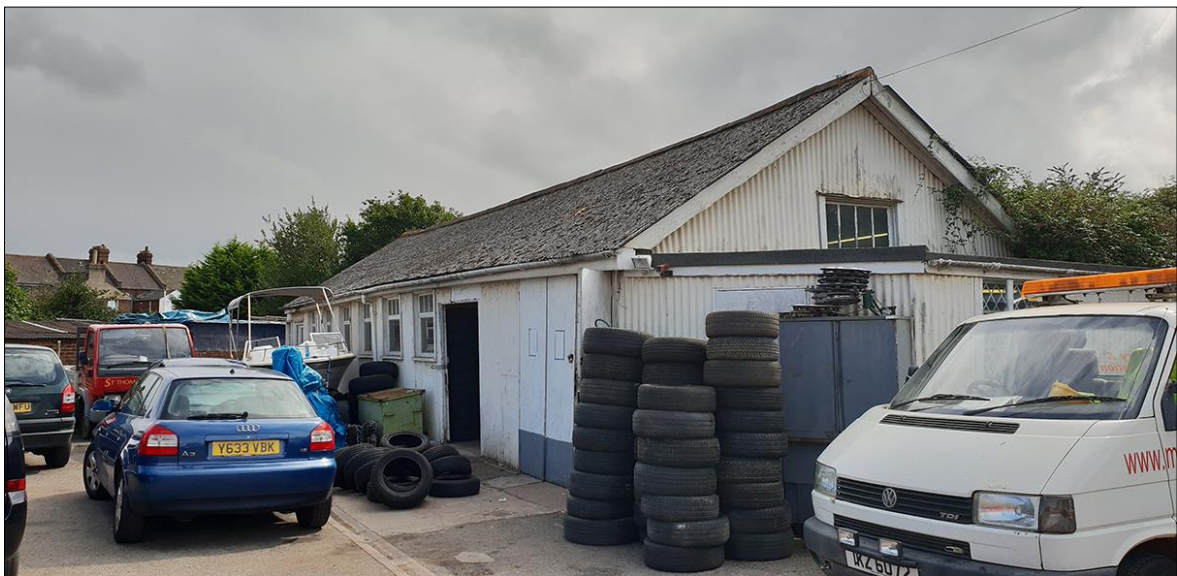
FIGURE 7: VIEW ALONG THE NORTH-EASTERN ELEVATION OF B1.1 (left) AND B1.2 (right); VIEWED FROM THE NORTH-WEST.
