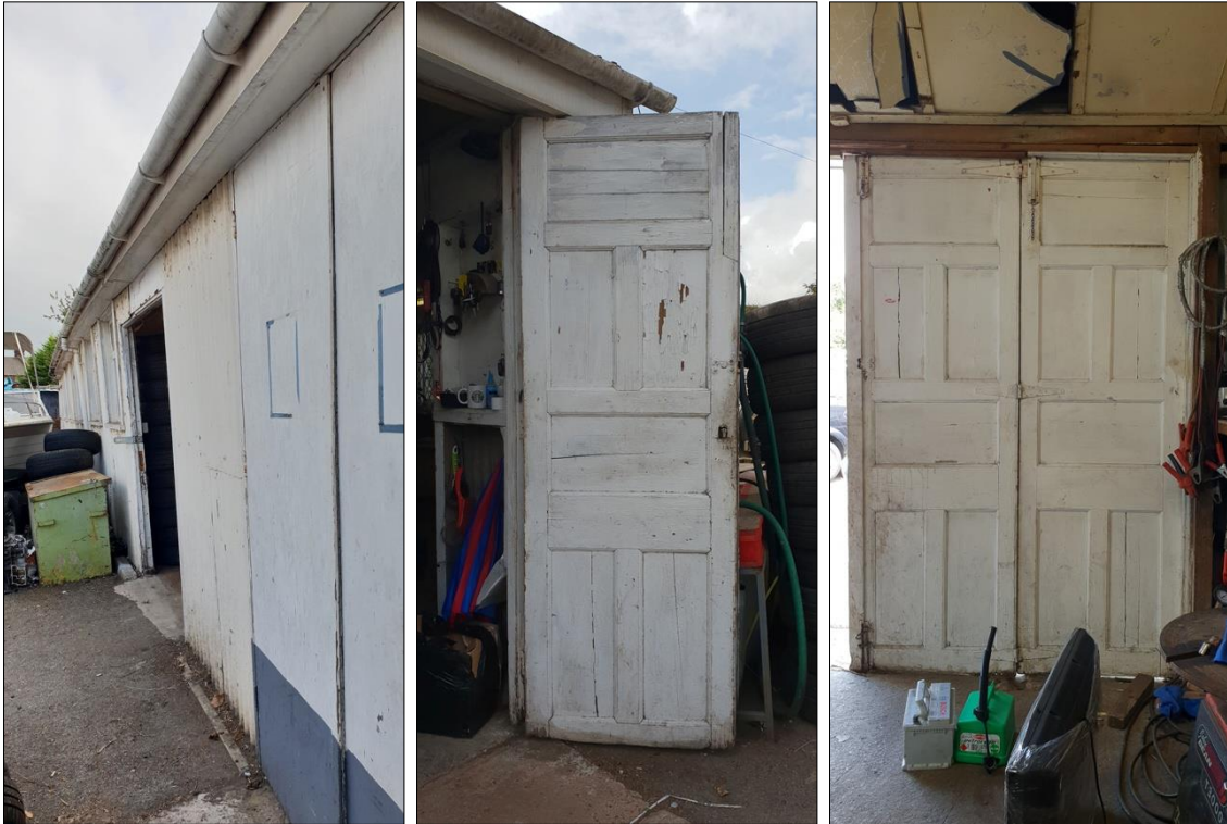
LEFT: DETAIL OF THE NORTH-EASTERN ELEVATION OF B1.1, SHOWING PANELLED LATE 19 TH CENTURY DOORS TO THE WESTERN END; VIEWED FROM THE WNW.
