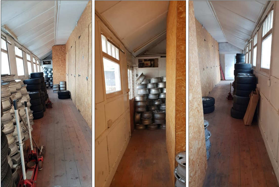
LEFT: DETAIL OF THE INTERIOR OF B1.1 SHOWING WINDOWS ALONG THE NORTH-EASTERN ELEVATION; THE TIMBER PLANK FLOOR; AND MODERN CHIPBOARD DIVISION OF THE MAIN ROOM; VIEWED FROM THE NORTH-WEST.
