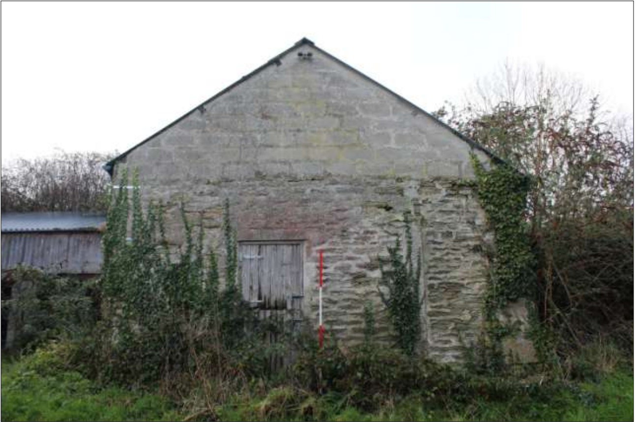
THE EAST ELEVATION OF FB3; VIEWED FROM THE EAST.
