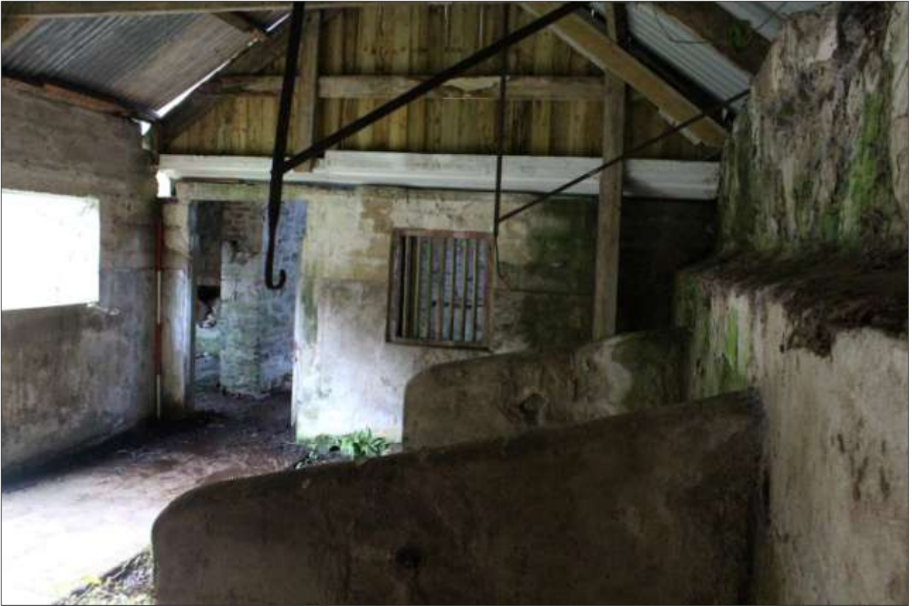
THE INTERIOR OF FB3; VIEWED FROM THE SOUTH.
