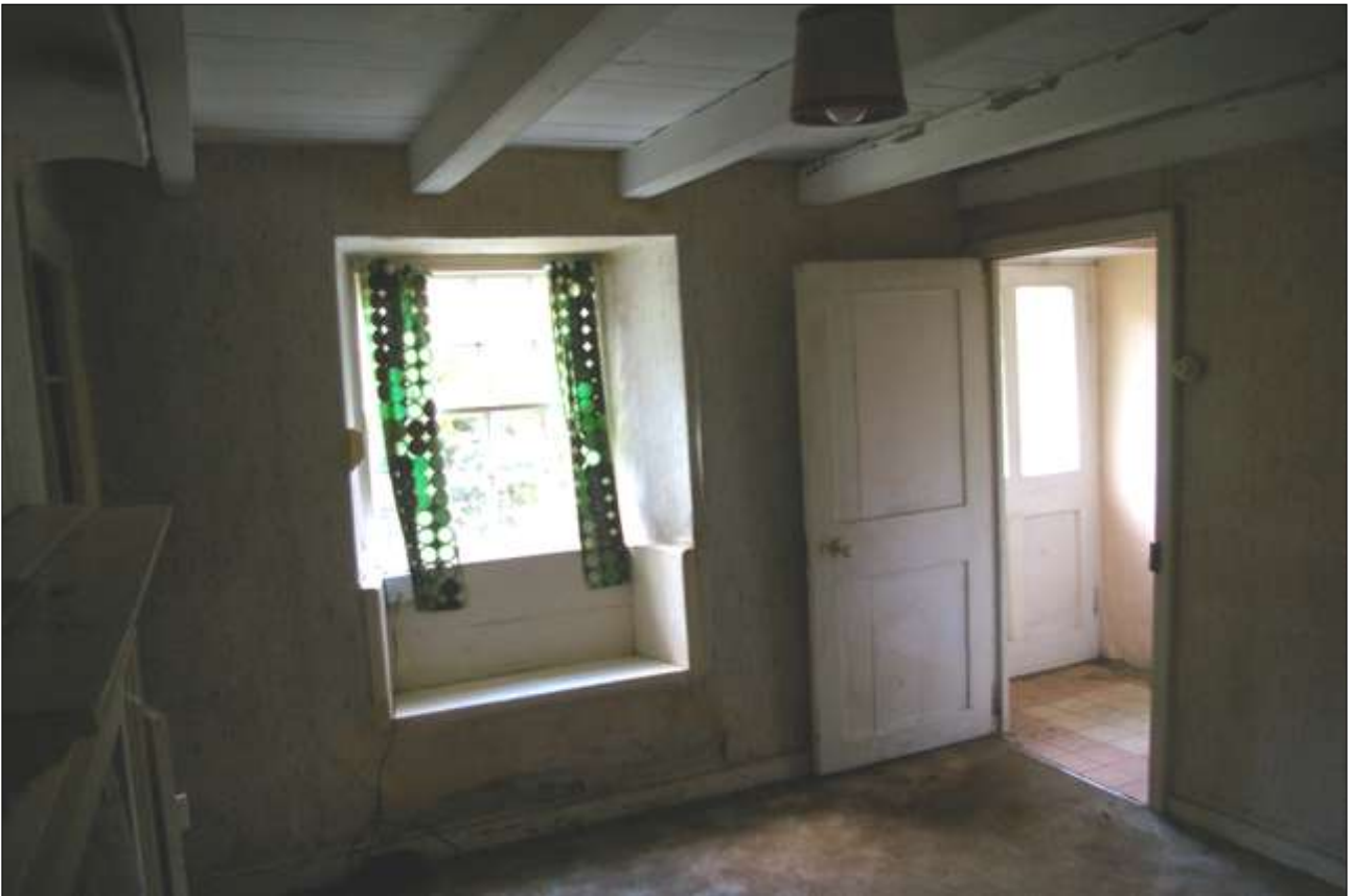
THE EAST WALL OF R2; VIEWED FROM THE ENE.
