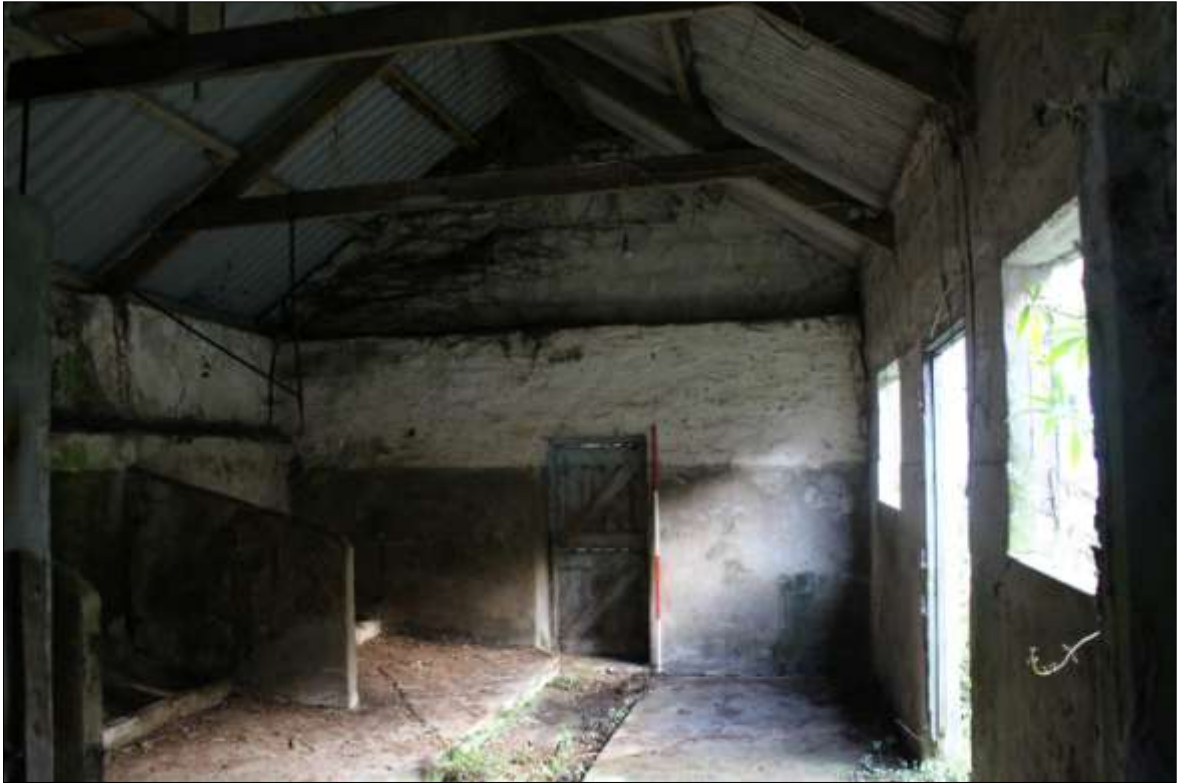
FIGURE 28: THE INTERIOR OF FB3; VIEWED FROM THE WEST (SCALE 2M).
