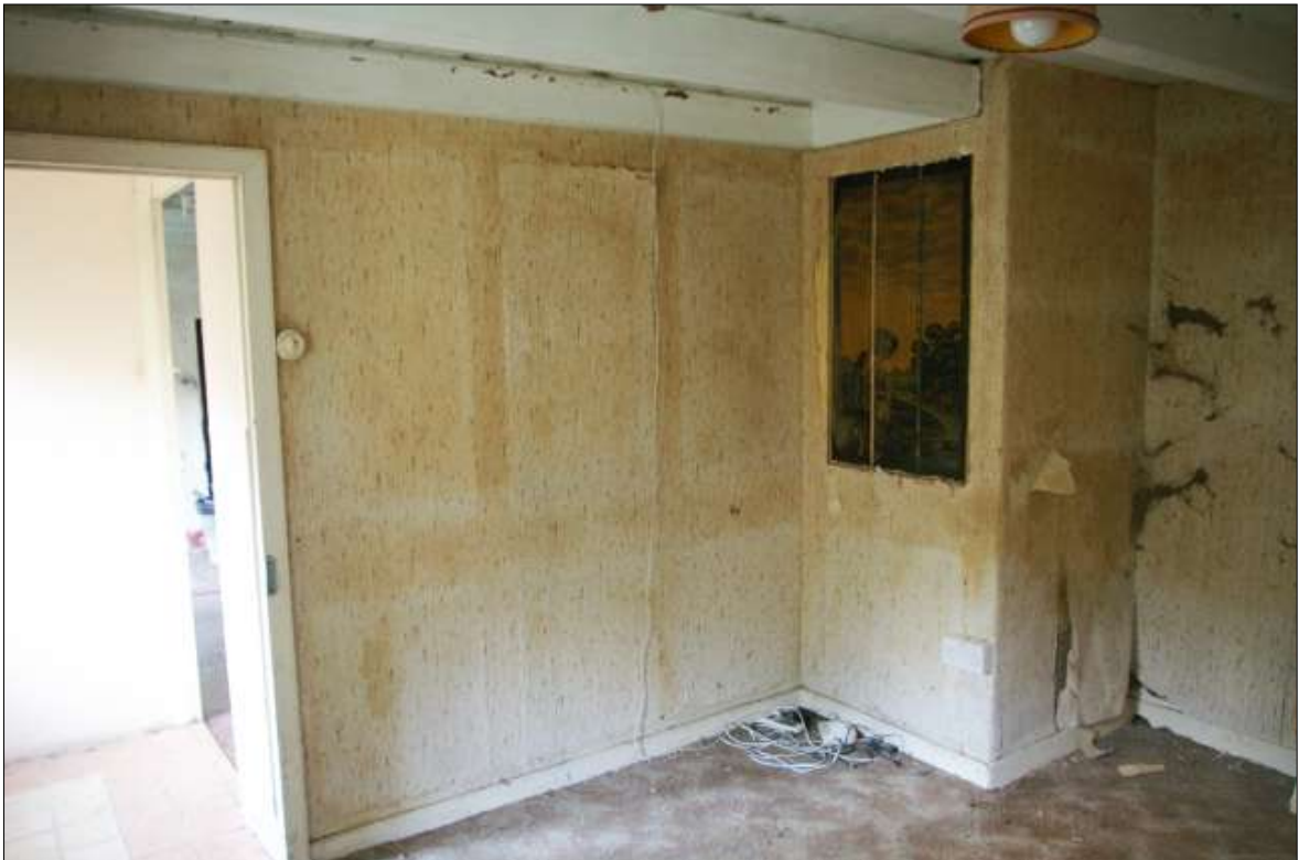
FIGURE 15: THE 18 TH CENTURY PARTITION WALL BETWEEN R1 AND R2, FROM R2; VIEWED FROM THE NORTH-EAST (NO SCALE). THE COVERED PANELS ARE VISIBLE, WITH THE EXPOSED PANEL TO THE RIGHT.
