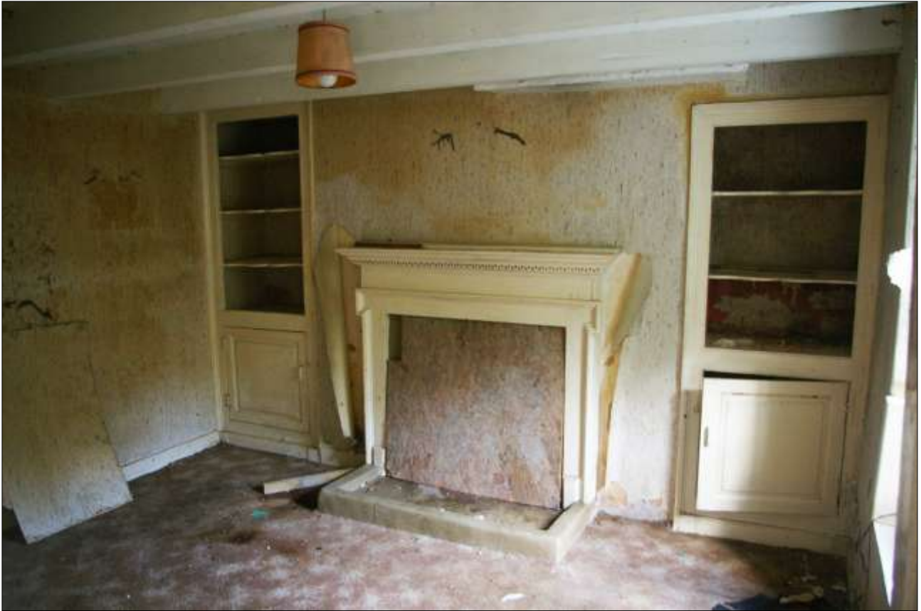
THE NORTH WALL OF R2, WITH RESET 18 TH CENTURY FIREPLACE AND 18 TH CENTURY ALCOVE SHELVES WITH CUPBOARDS; VIEWED FROM THE SOUTH-EAST (NO SCALE).
