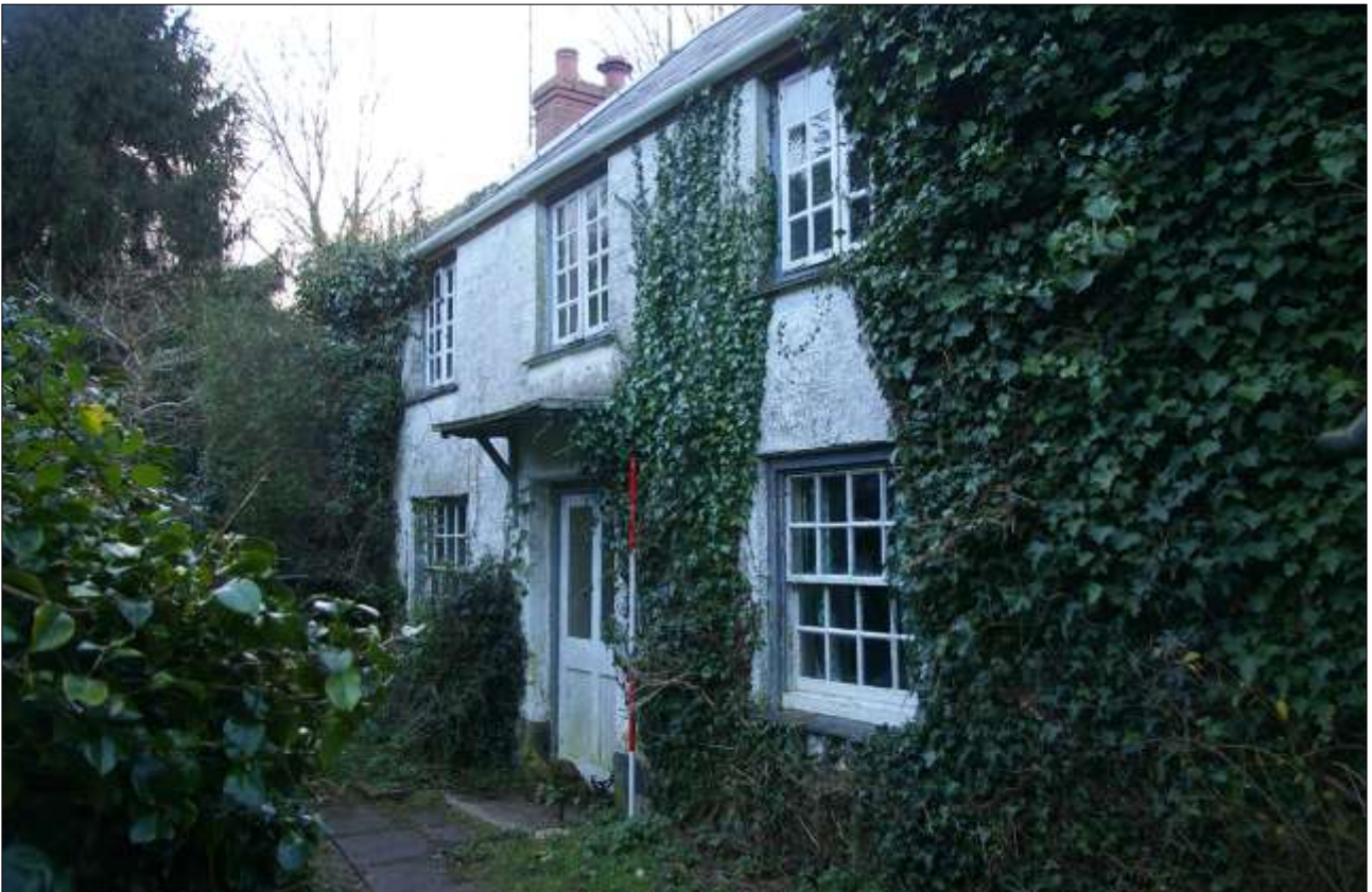
THE EAST ELEVATION, VIEWED FROM THE NORTH-EAST (SCALE 2M).
