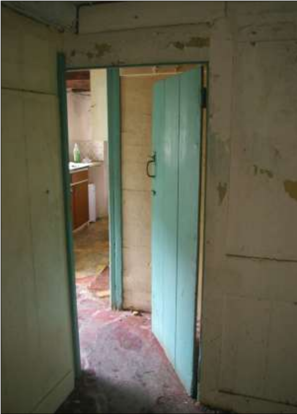
LEFT: DG8, FROM R1 TO R3; VIEWED FROM THE SOUTH.
