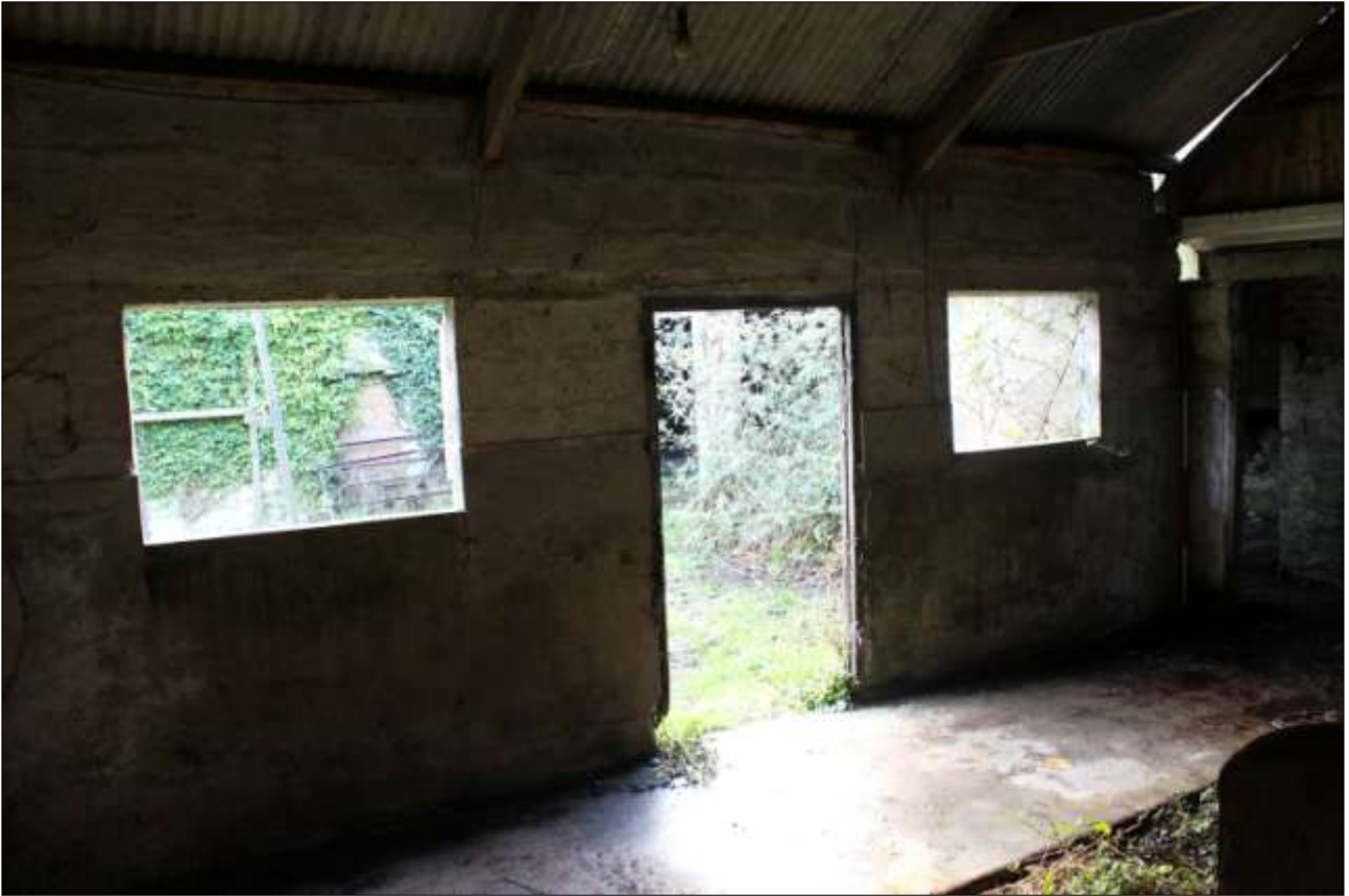
THE SOUTH WALL OF FB3; VIEWED FROM THE NORTH-EAST.
