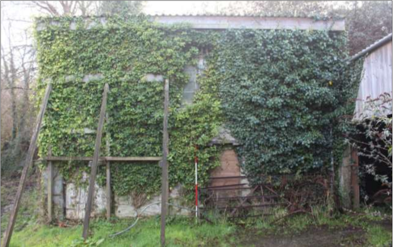
THE NORTH ELEVATION OF FB1; VIEWED FROM THE NORTH (SCALE 2M).
