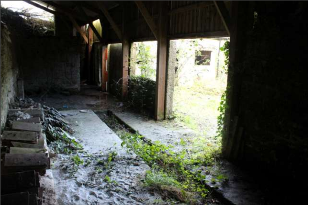
THE INTERIOR OF FB2A; VIEWED FROM THE SSW (SCALE 2M).
