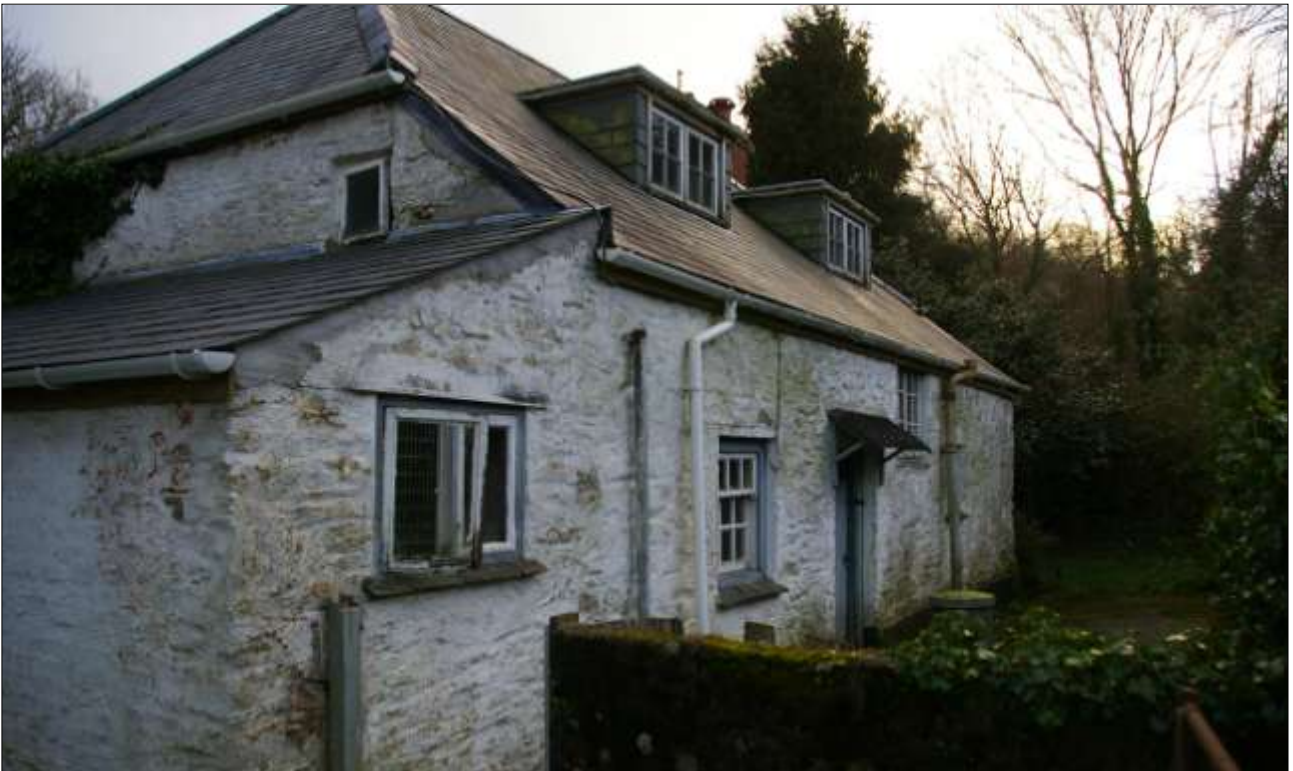
THE WEST ELEVATION OF THE COTTAGE; VIEWED FROM THE NORTH-WEST.
