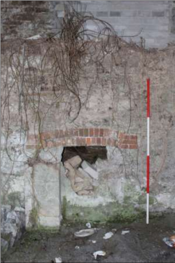
LEFT: BO4; VIEWED FROM THE EAST (SCALE 2M).
