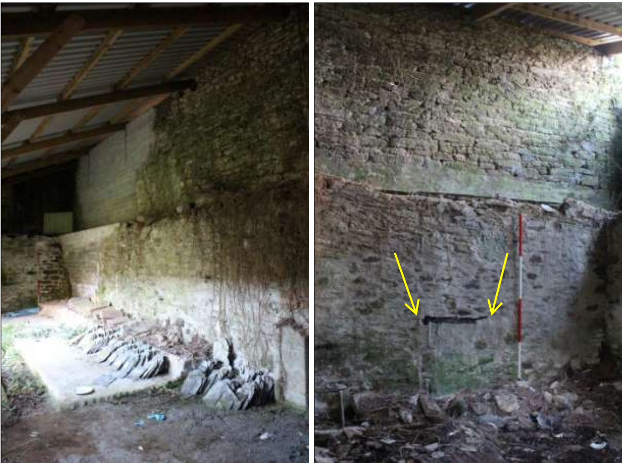
LEFT FIGURE 25: THE BACK (WEST) WALLS OF FB2A; VIEWED FROM THE NORTH-NORTH-EAST (NO SCALE). RIGHT FIGURE 26: THE BACK (WEST) WALLS OF FB2B, SHOWING THE BLOCKED FIREPLACE (INDICATED); VIEWED FROM THE EAST (SCALE 2M). NOTE THE QUALITY OF THE STONEMWORK IN THE UPPER WALL.
