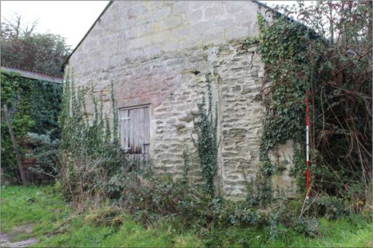
THE EAST ELEVATION OF FB3; VIEWED FROM THE NORTH-EAST (SCALE 2M).
