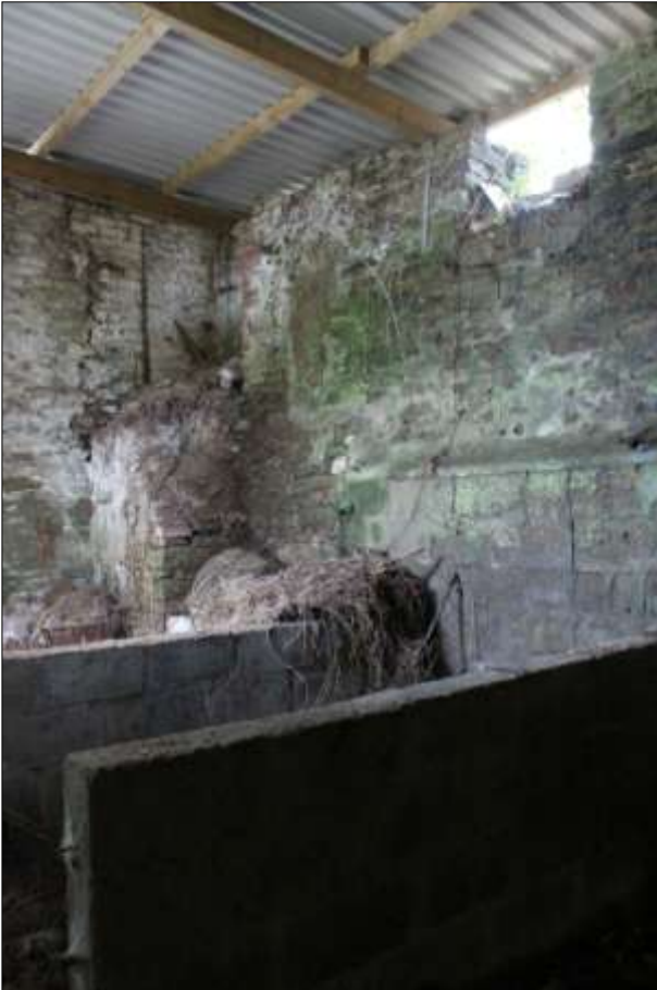
THE INTERIOR OF FB1; VIEWED FROM THE NORTH-WEST.
