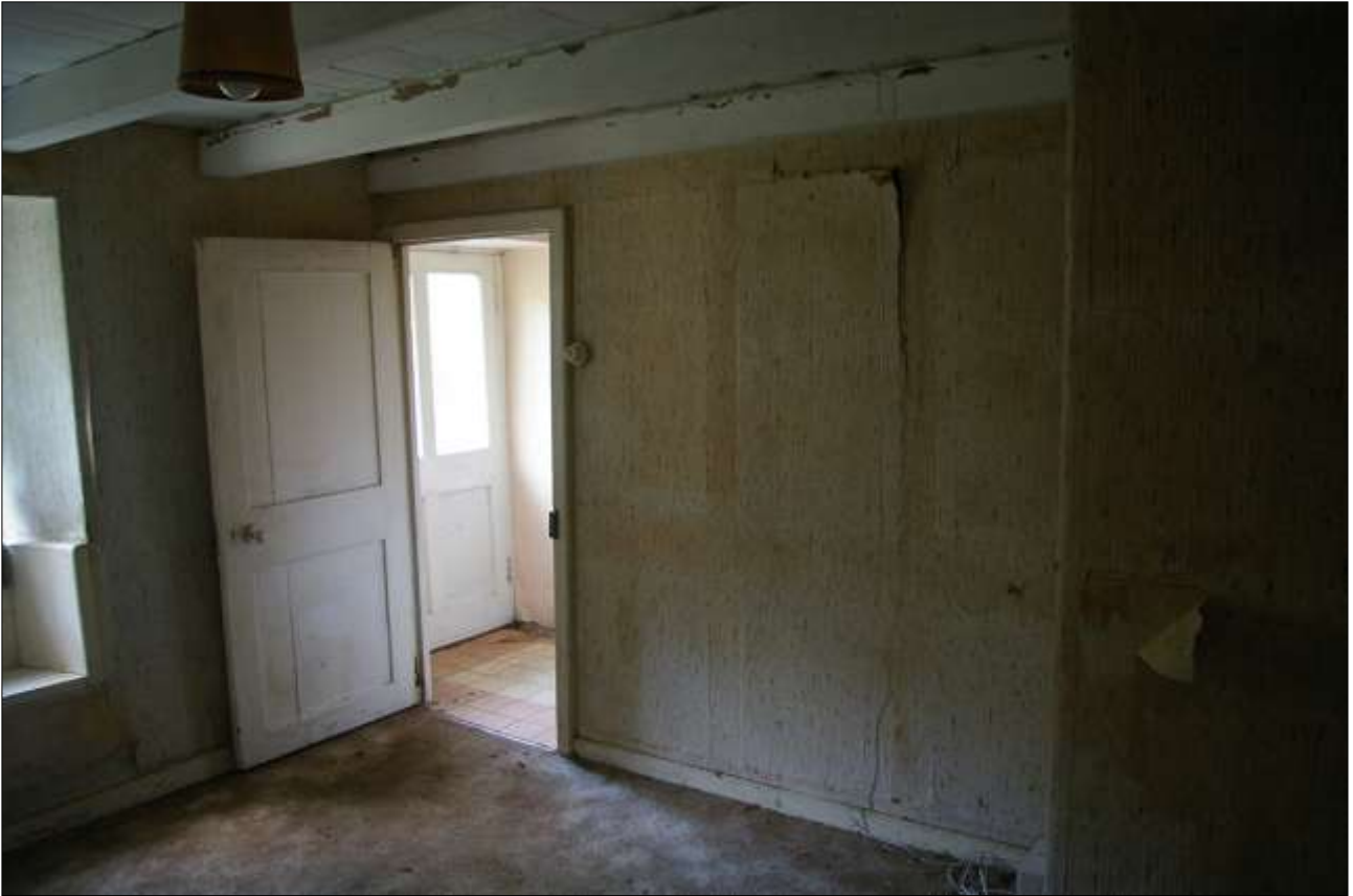
AS ABOVE; VIEWED FROM THE NORTH-WEST.
