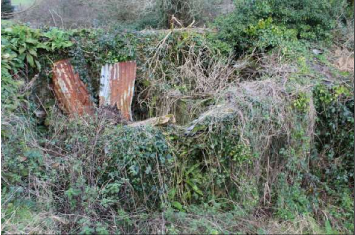
FIGURE 29: FB4A; VIEWED FROM THE SOUTH-WEST (NO SCALE).
