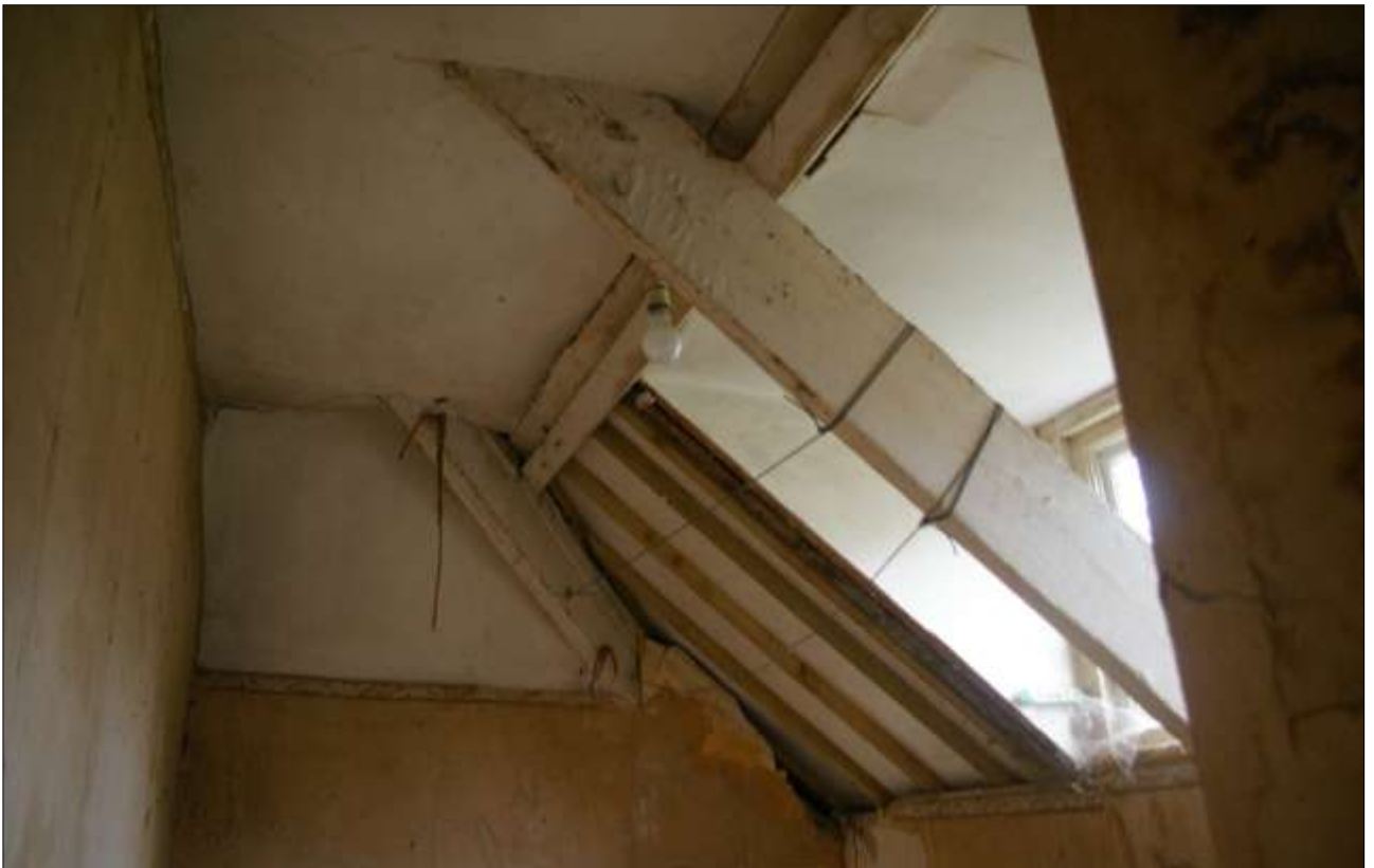
THE CEILING IN R10 SHOWING THE DORMER AND THE C21 REPLACEMENT ROOF ELEMENTS; VIEWED FROM THE NORTH.
