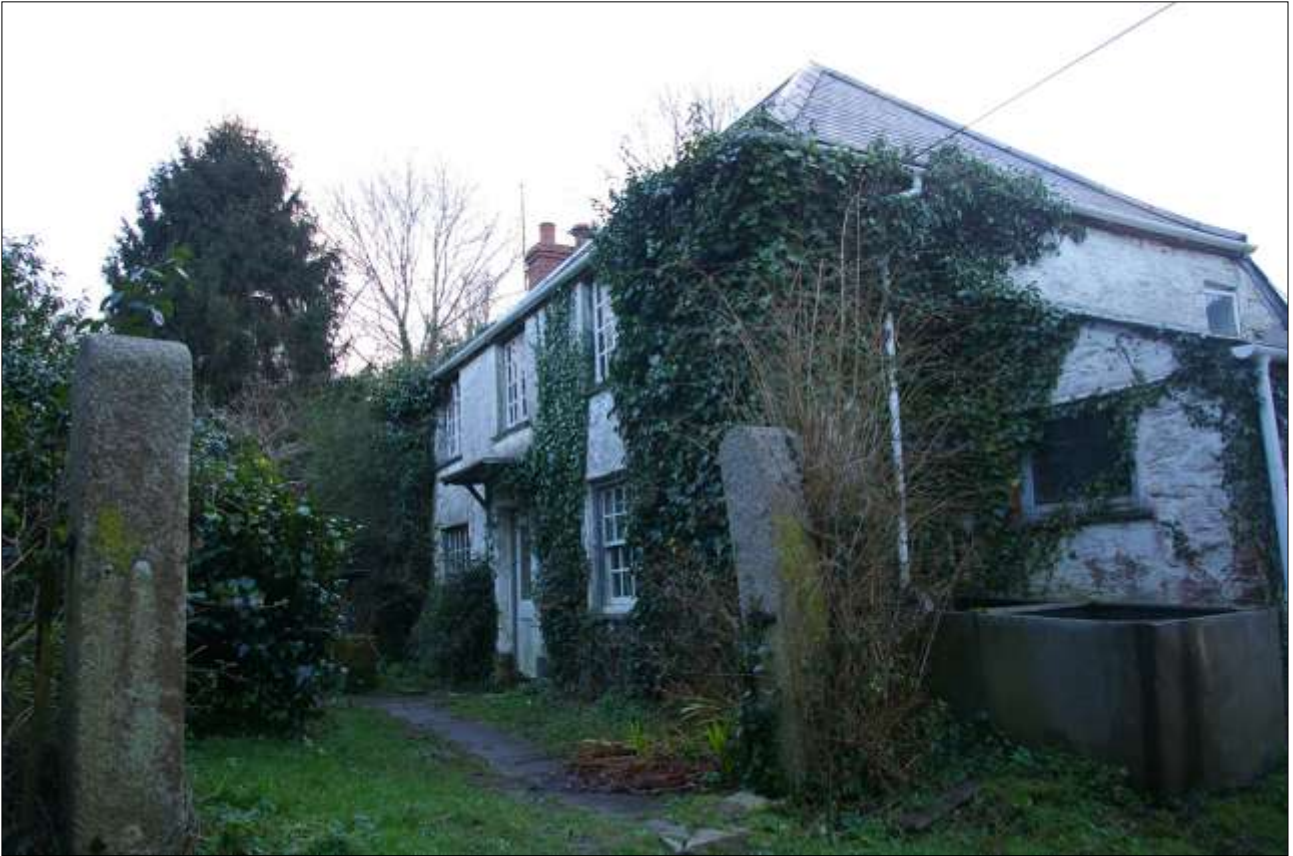
THE EAST ELEVATION, VIEWED FROM THE NORTH-EAST.
