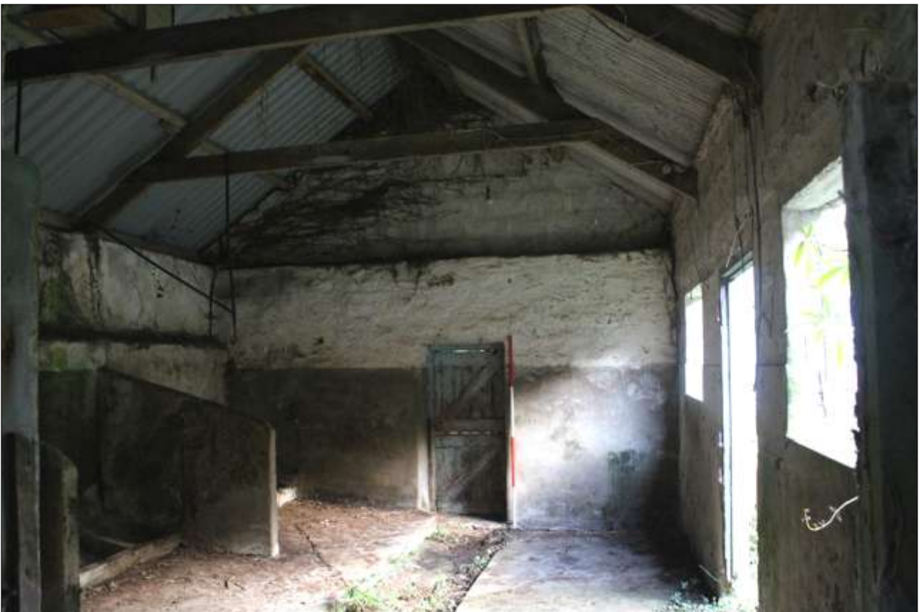
THE INTERIOR OF B3; VIEWED FROM THE WEST (SCALE 2M).
