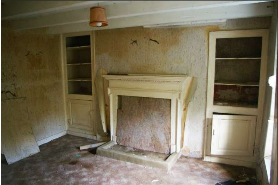
FIGURE 14: THE NORTH WALL OF R2, WITH RESET 18 TH CENTURY FIREPLACE AND 18 TH CENTURY ALCOVE SHELVES WITH CUPBOARDS; VIEWED FROM THE SOUTH-EAST (NO SCALE).
