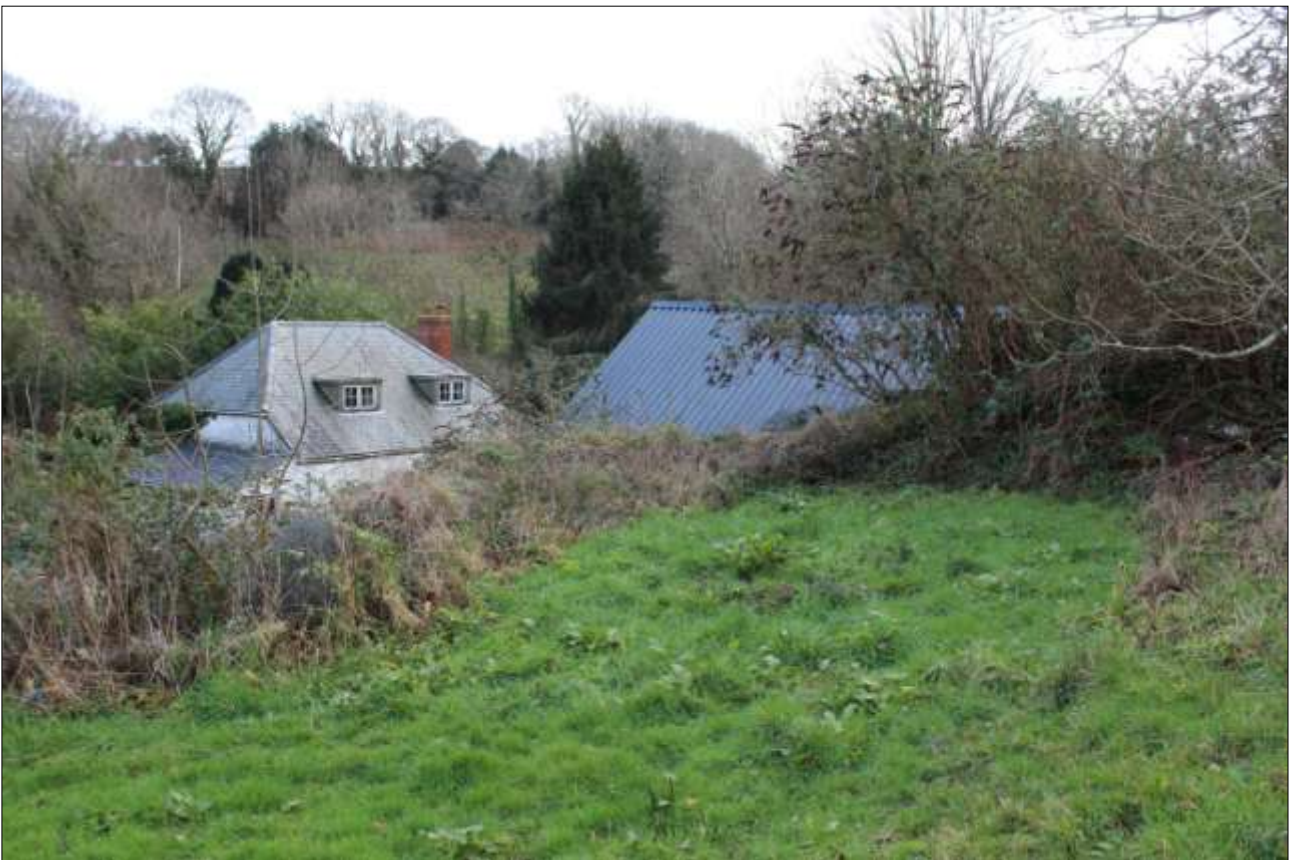
LOOKING BACK OVER THE ROOF OF FB3 (RIGHT) TOWARDS THE COTTAGE; VIEWED FROM THE NORTH-WEST.
