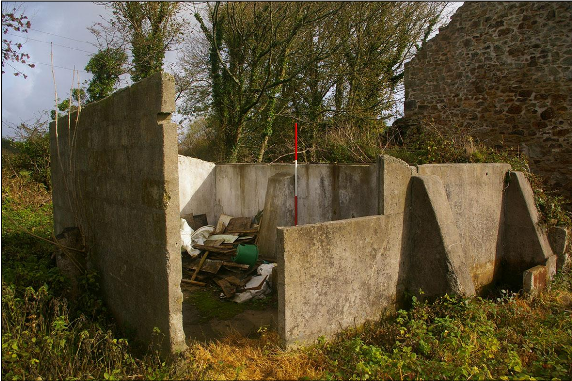
FIGURE 9: BUILDING 4; FROM THE SOUTH-WEST.
