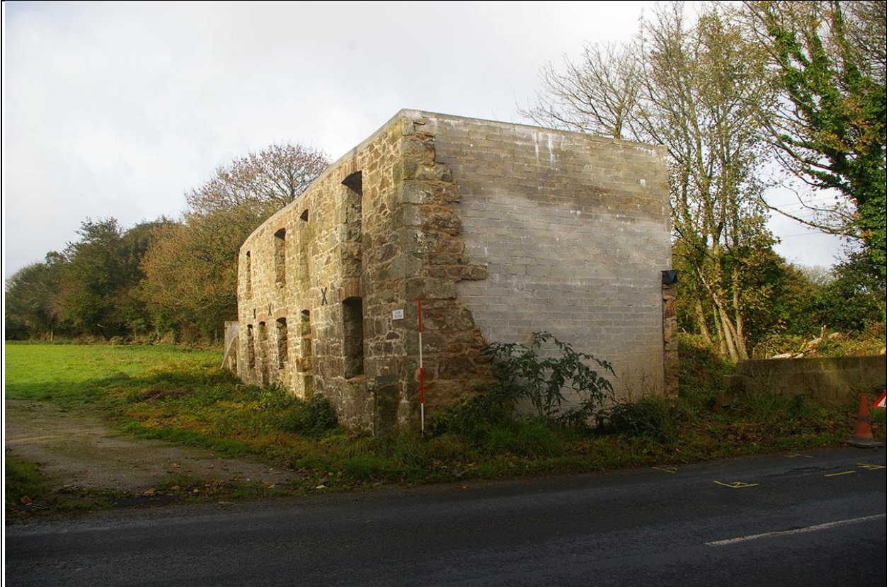
THE EAST ELEVATION OF BUILDING 2; FROM THE EAST, SOUTH-EAST.
