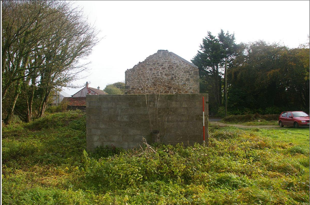
THE WEST ELEVATION OF BUILDING 4; FROM THE WEST.
