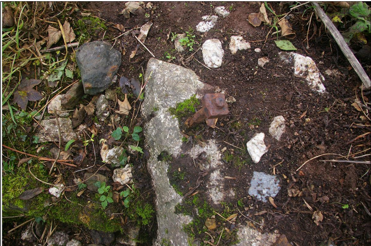
IRON BOLT FIXING ON THE SOUTH-WEST CORNER OF THE WHIM PIT; FROM THE NORTH.
