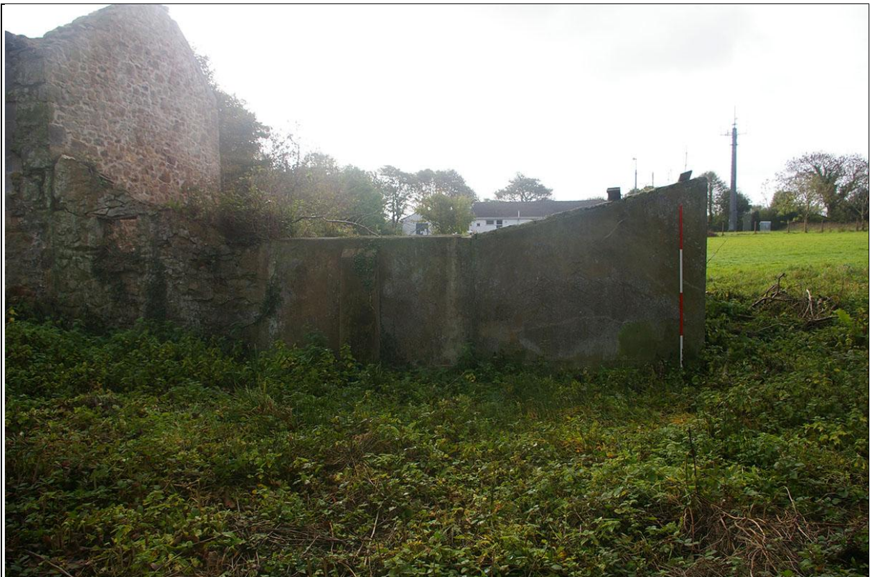
THE NORTH ELEVATION OF BUILDING 4; FROM THE NORTH, NORTH-WEST.
