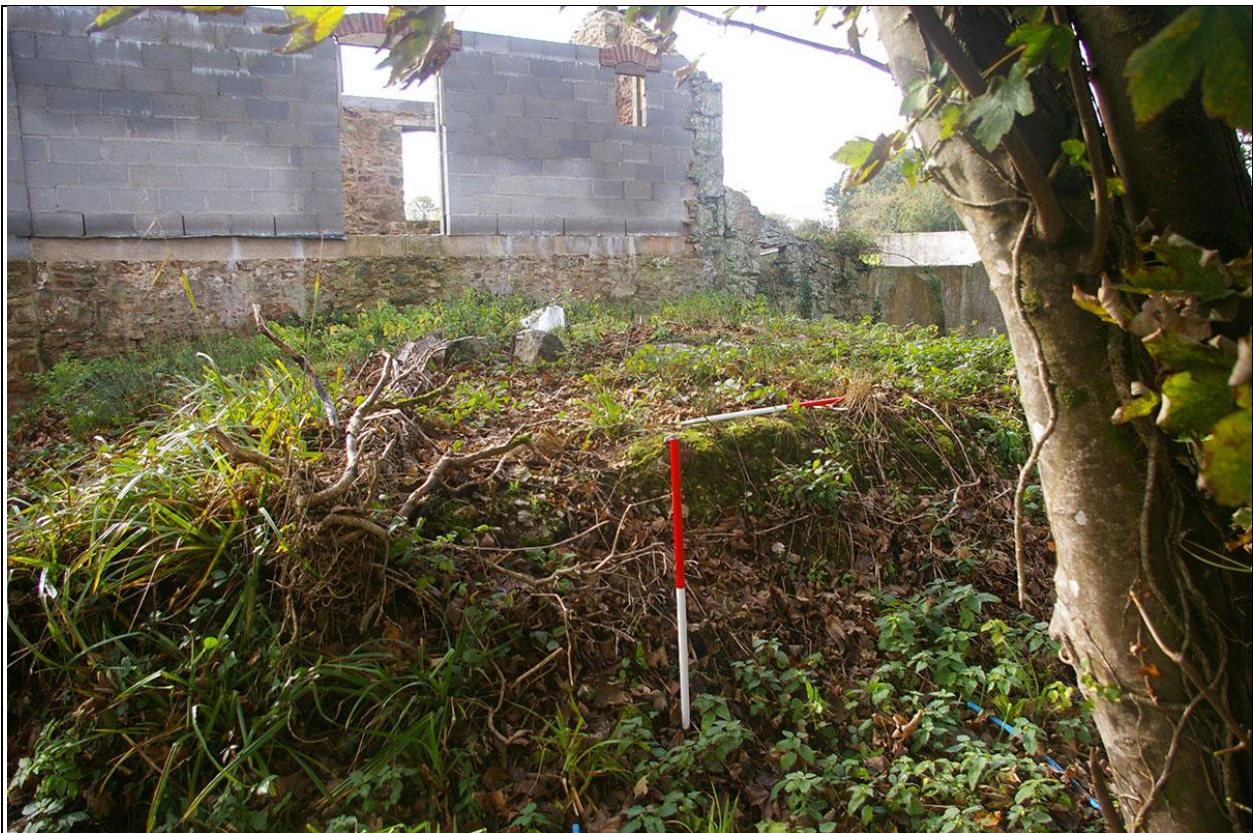
THE NORTH SIDE OF THE WHIM MOUND, WITH 2 X 1M SCALE, SHOWING THE PROFILE OF THE STEEP SLOPE; FROM THE NORTH-EAST.
