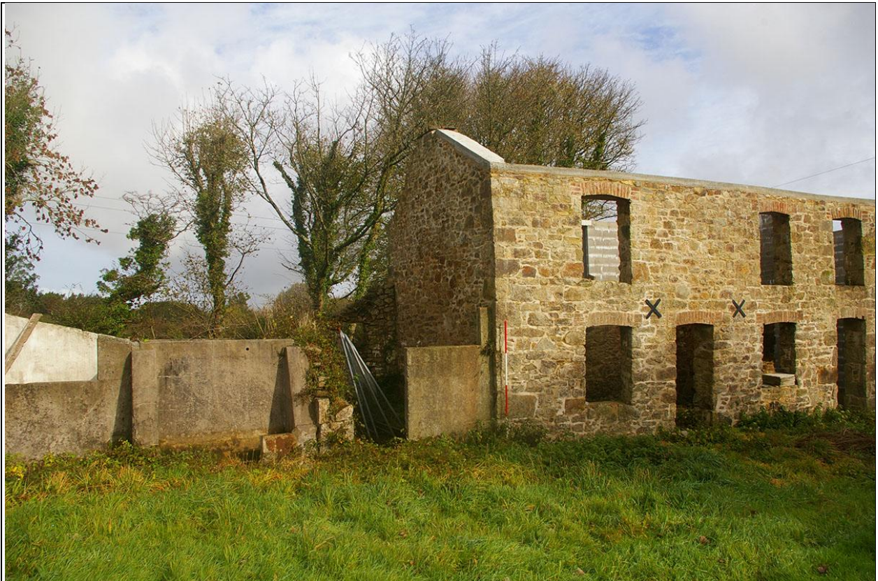
VIEW OF THE RELATIONSHIP OF BUILDINGS 3 AND 4, WITH THE WEST ELEVATION OF BUILDING 1; FROM THE SOUTH-WEST.
