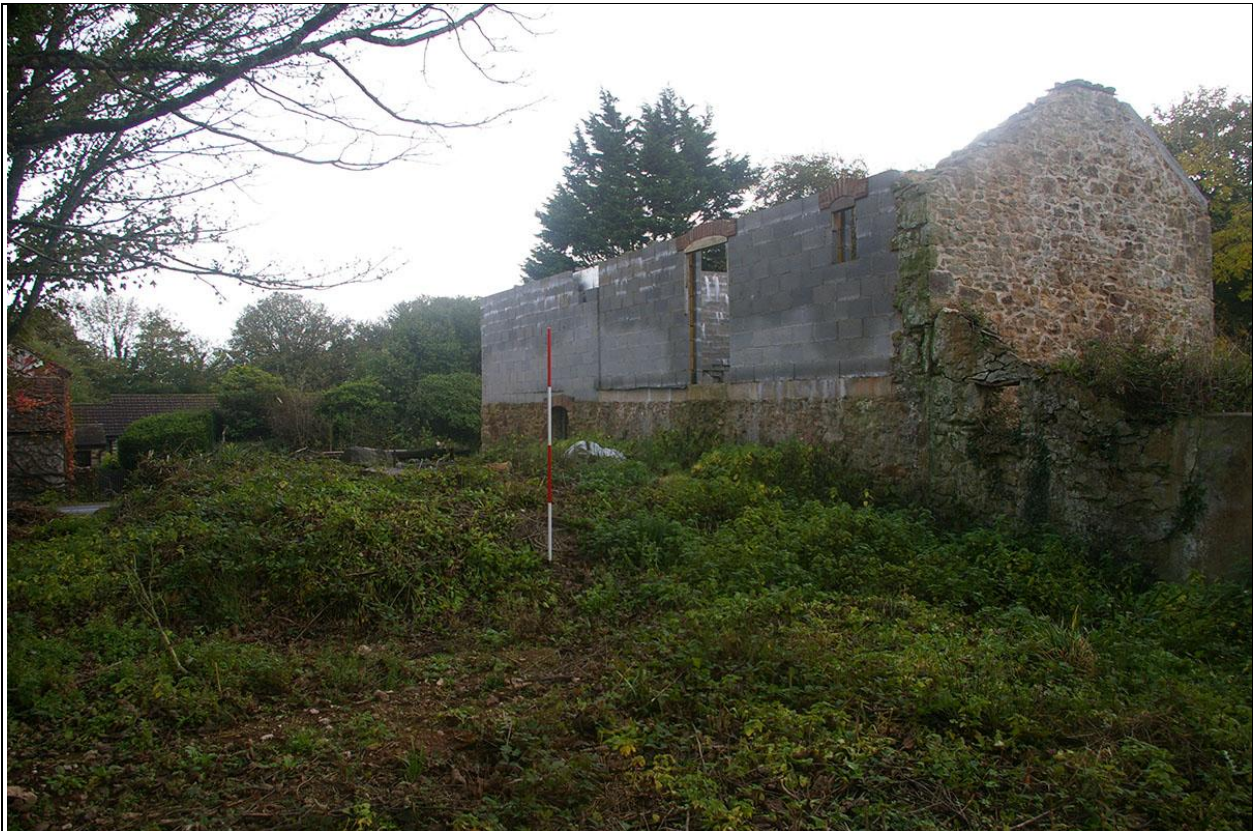
THE NORTH ELEVATION OF BUILDING 1 AND THE ATTACHED/ADJACENT WHIM MOUND; FROM THE WEST, NORTH-WEST.
