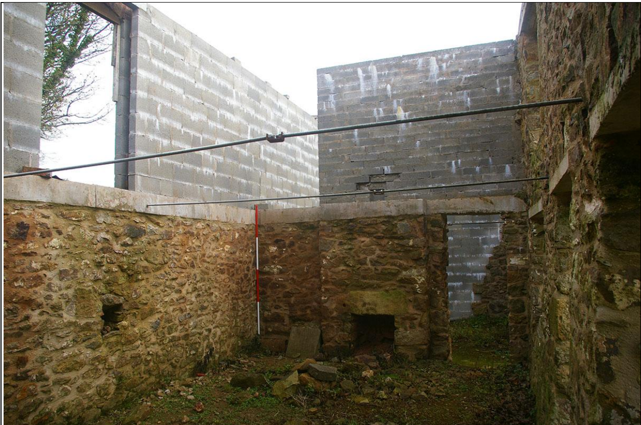
THE NORTH AND EAST WALLS, SHOWING HOW MUCH LARGER THE STONES USED IN THE EAST WALL ARE AND HOW MUCH MORE IRREGULAR THE BUILD, AS WELL AS THE LOW, SMALL BOXY FIREPLACE; FROM THE SOUTH-WEST.
