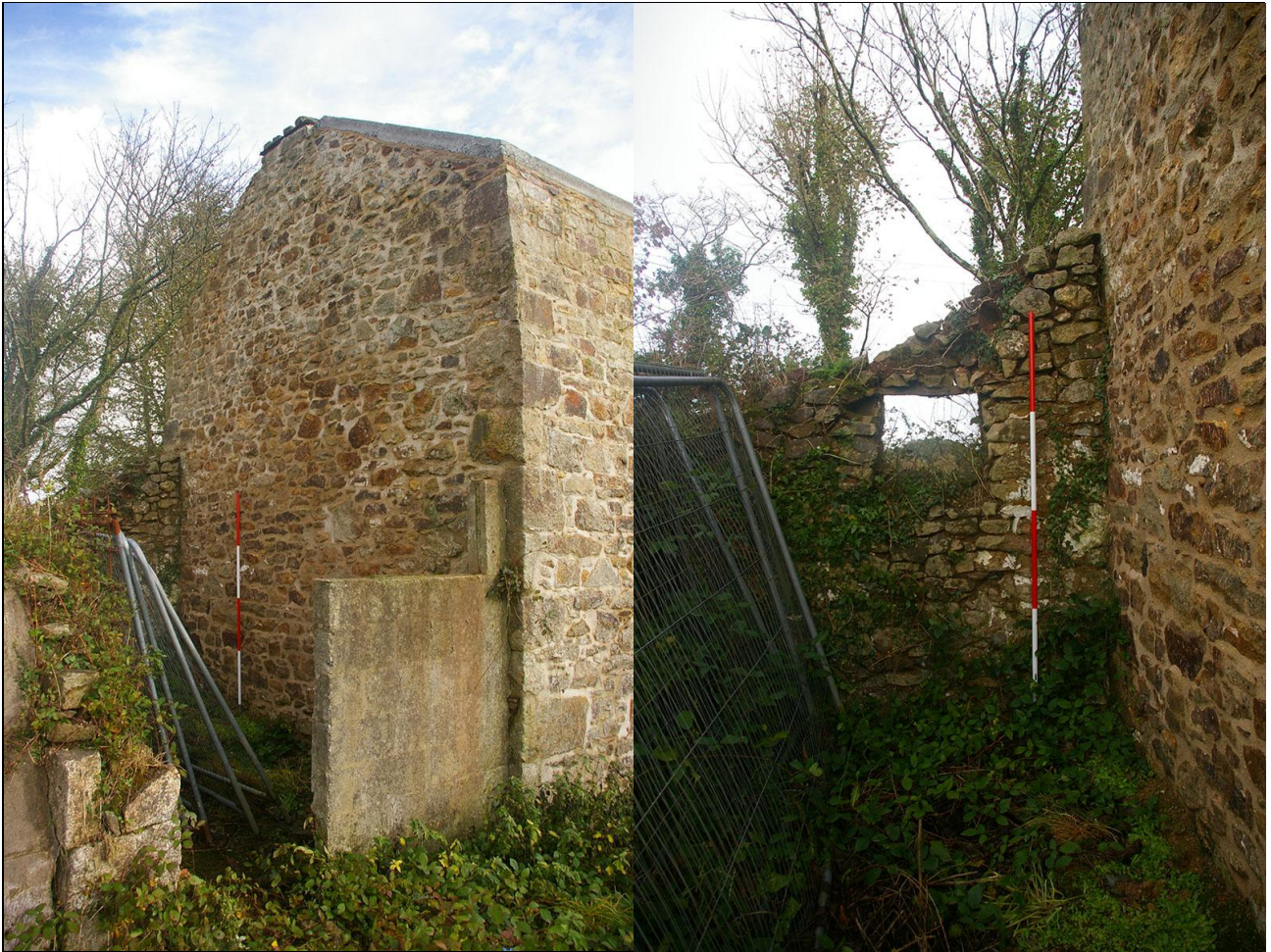
VIEW OF THE WEST GABLE OF BUILDING 1; FROM THE SOUTH-WEST.
