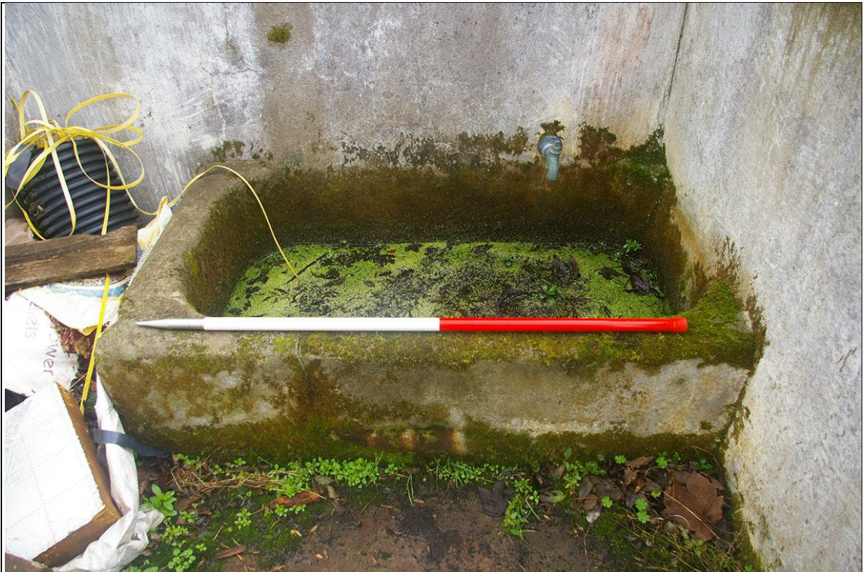
THE CISTERN IN BUILDING 4; FROM THE WEST.
