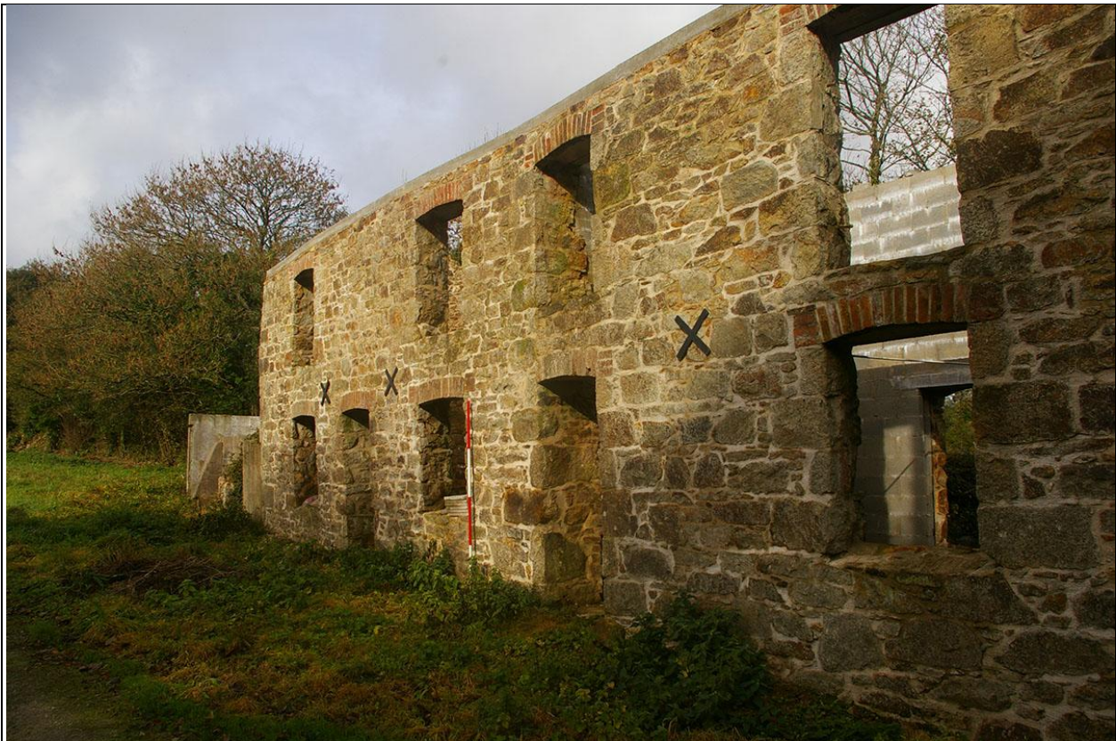
THE SOUTH ELEVATION OF THE BUILDING RANGE, BUILDINGS 1-4; FROM THE SOUTH-EAST.
