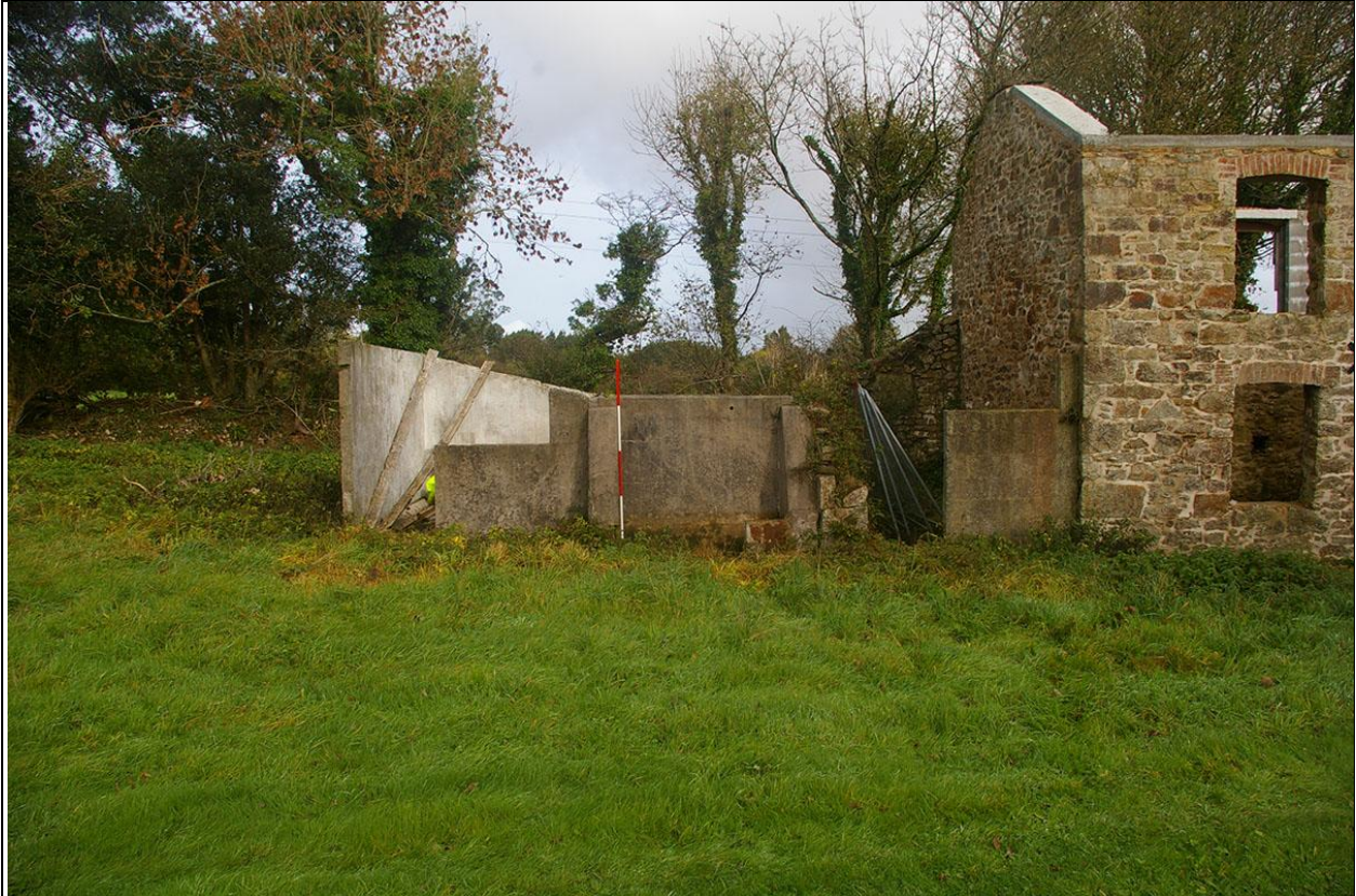
THE SOUTH ELEVATIONS OF BUILDINGS 3 AND 4; FROM THE SOUTH.
