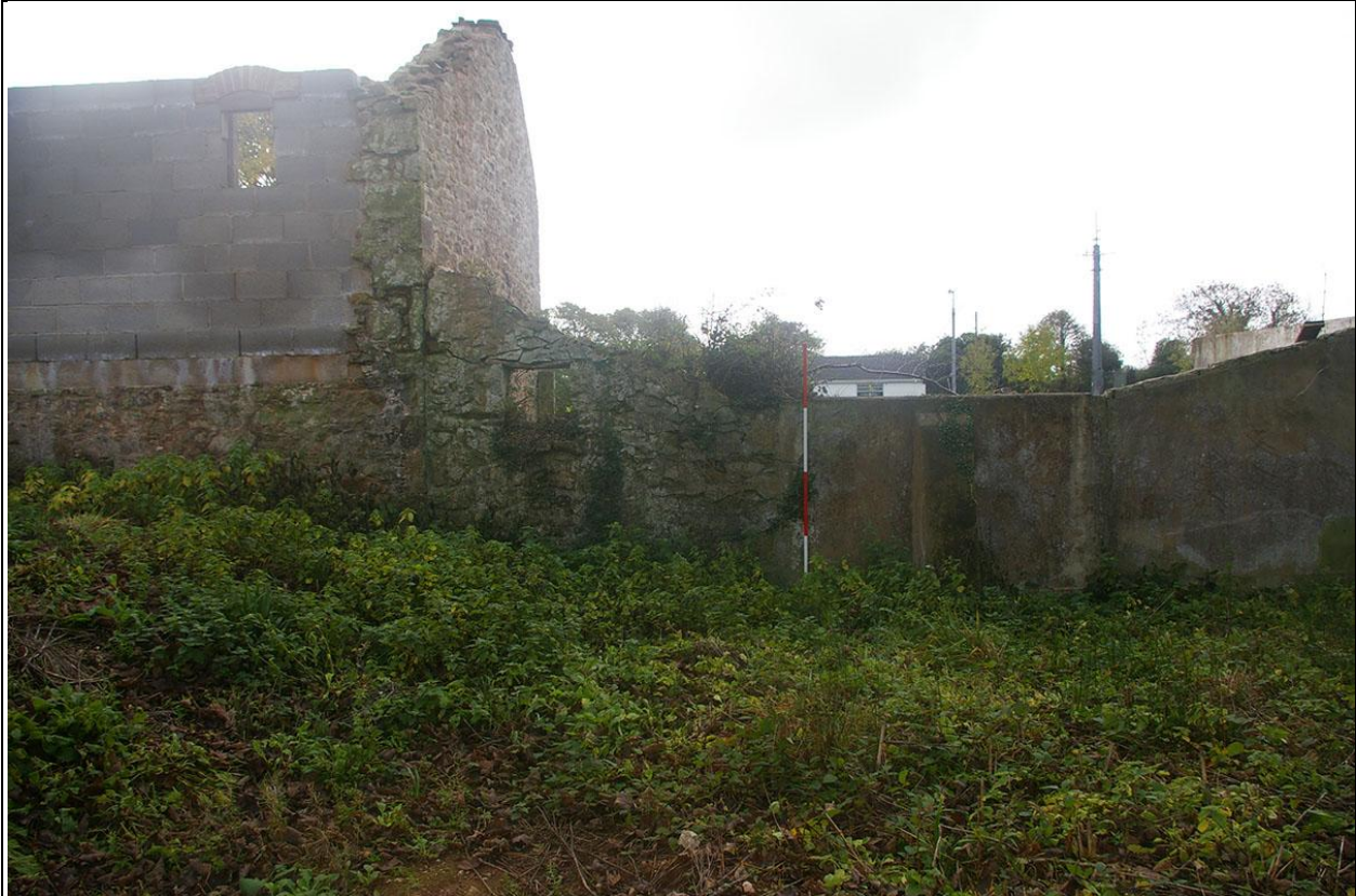
THE NORTH ELEVATION OF BUILDING 4 AND BUILDING 3; FROM THE NORTH-WEST.
